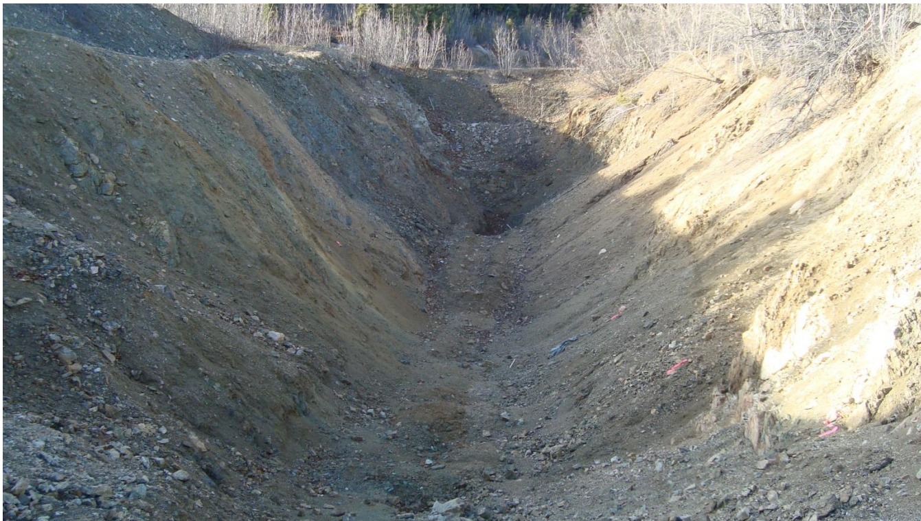
Photograph 12: View looking northwest of bulk sample excavation site in the proposed open pit area
