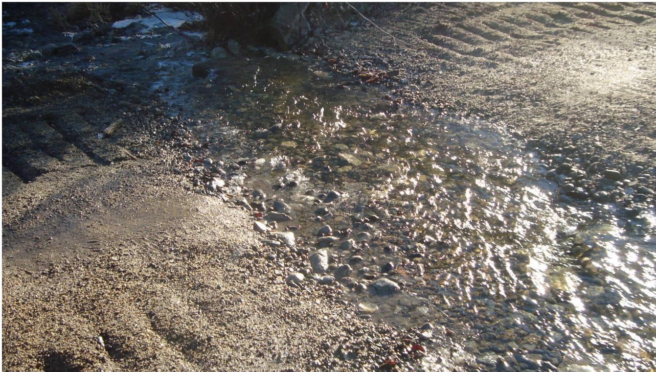
Photograph 17: View looking north of constructed 'ford' on access road at Williams Creek crossing
