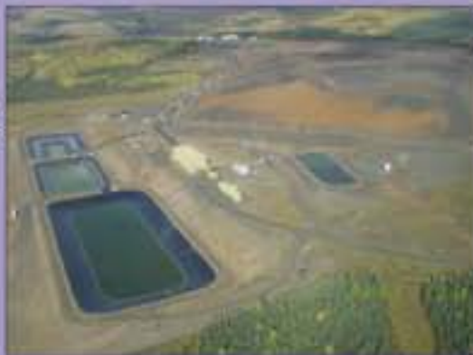
Ponds cleaned, filled, and plant grasses
