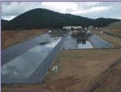
Heap Leach Facility/ Mezän tthi ts'in lake'ts'le
