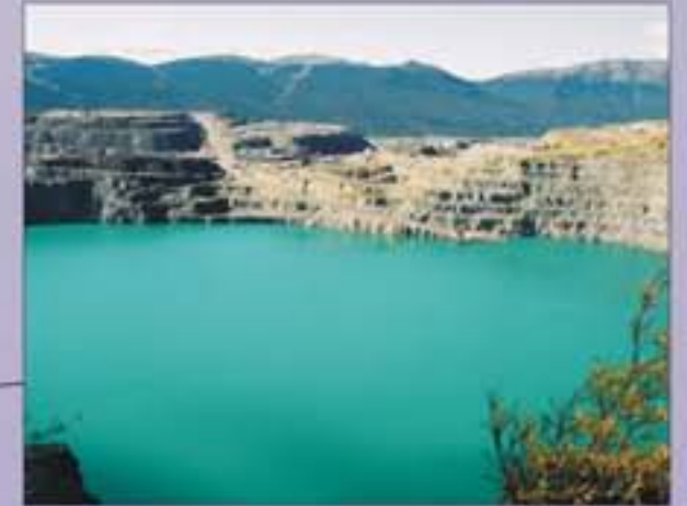
Pit - block access, allow to flood
