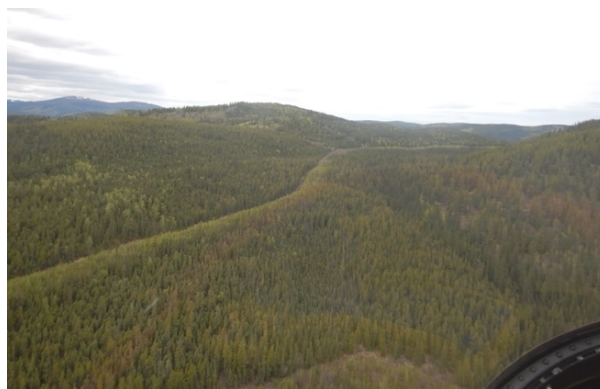
Photo-Plate 3. Section of grubbed Access Route.
