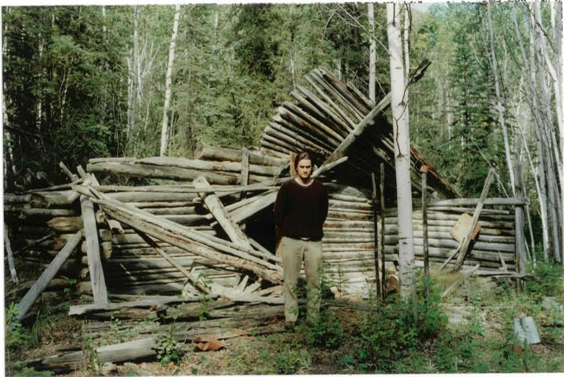
FIGURE 8. A view of log cabin structure at site 115-l/07/001, looking north.
