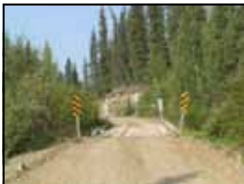
Freegold Road Crossing Creek Bridge
