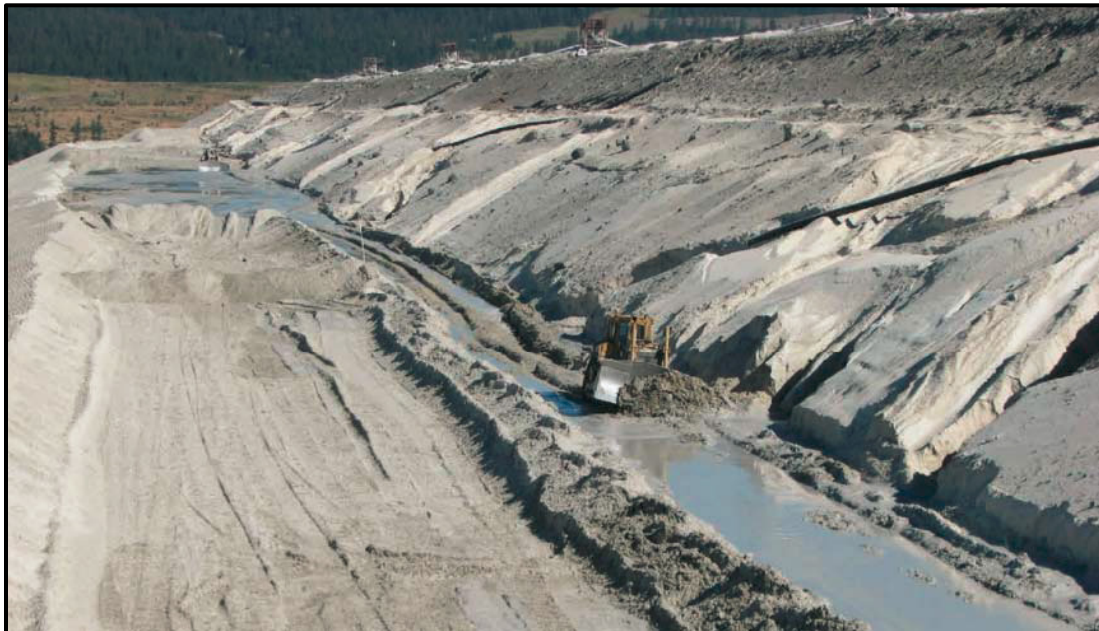
Figure B.4.8-4 Confinement Berm Construction
