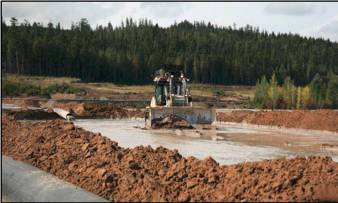
Figure B.4.8-5 Sand Cell Compaction
