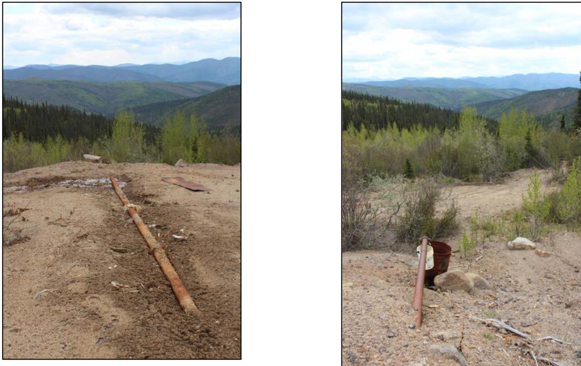
Figure A.7.3-2 Historical Adit Discharge Pipe (May 28, 2014)
