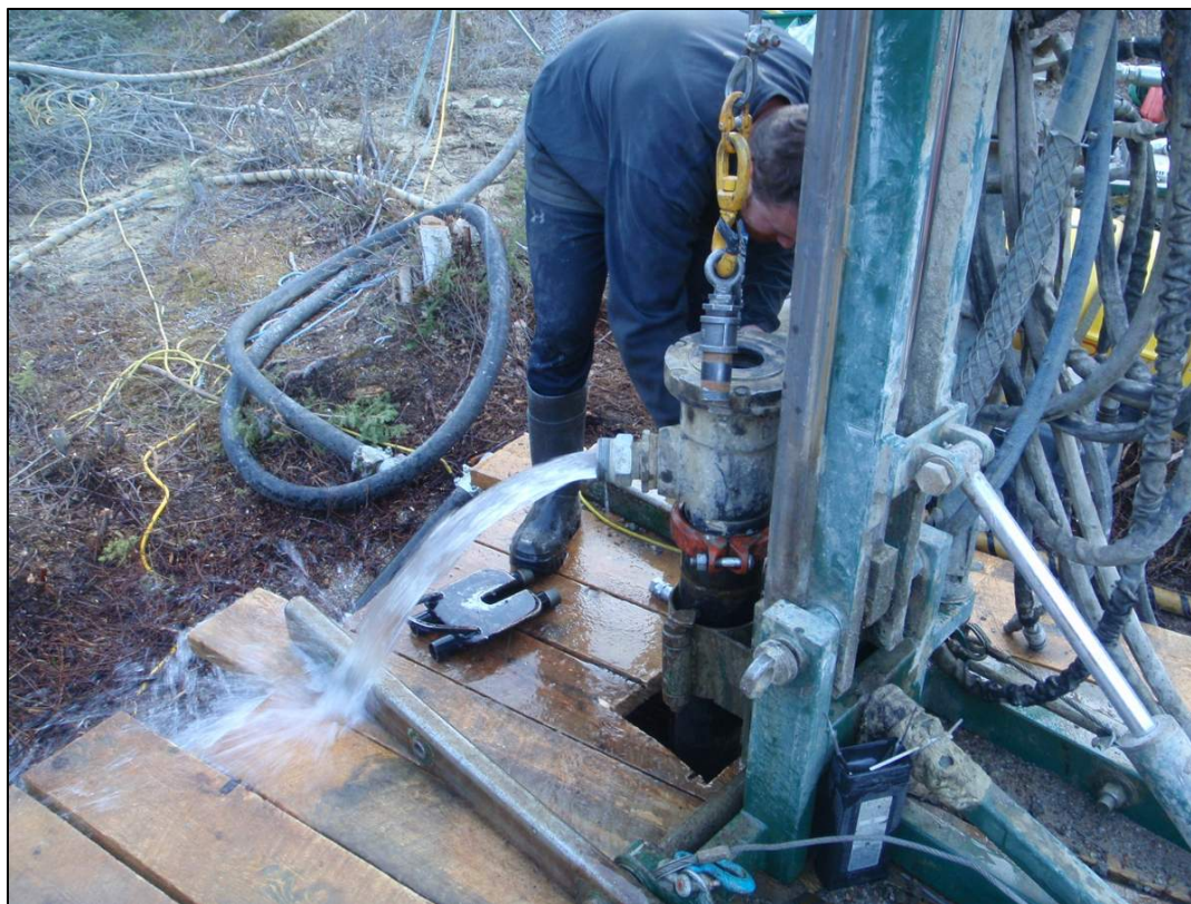
Figure 4-11: Artesian flows encountered during advancement of MW15-04WB.
