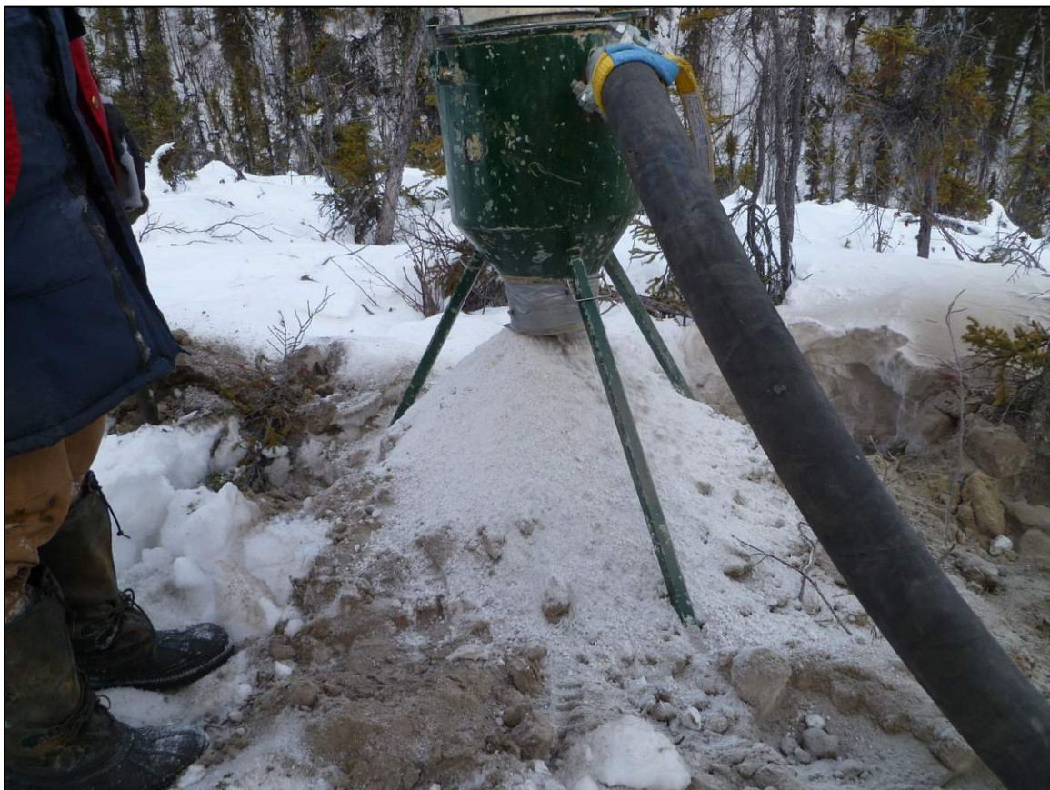
Figure 4-2: Ice “cuttings” intercepted at MW15-01T while advancing casing through colluvium.
