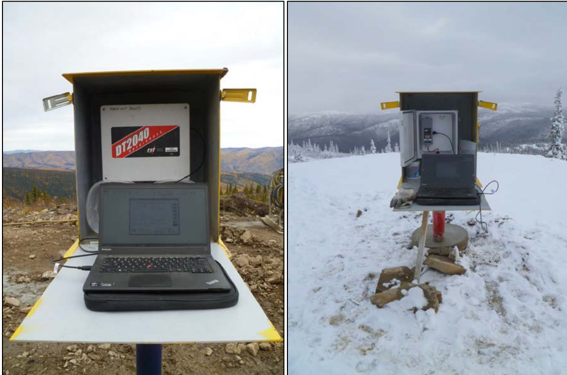
Figure 3-2: Thermistor installation at MW14-04T (left) and VWP installation at CFD-0318 (right).
