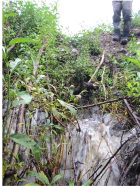
From bottom barrier looking upstream
