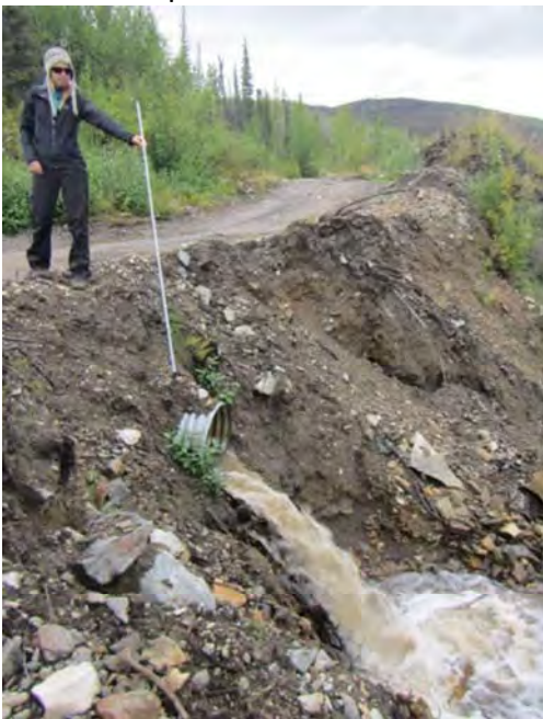
Culvert drop with metre stick
