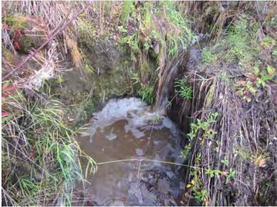
Upstream - vertical drop
