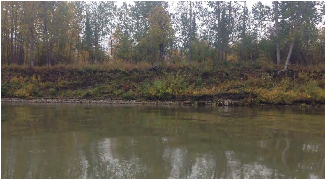
Photo 8 – Proposed Barge Landing Location on the Yukon River (south side), on September 10, 2015.
