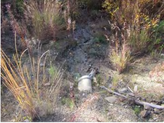
Dry culvert in abandoned channel (#220)
