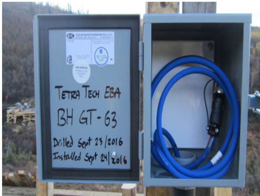
Photo 10: Ground Temperature Cable installation in Borehole GT-63. Photo taken on September 26, 2016.
