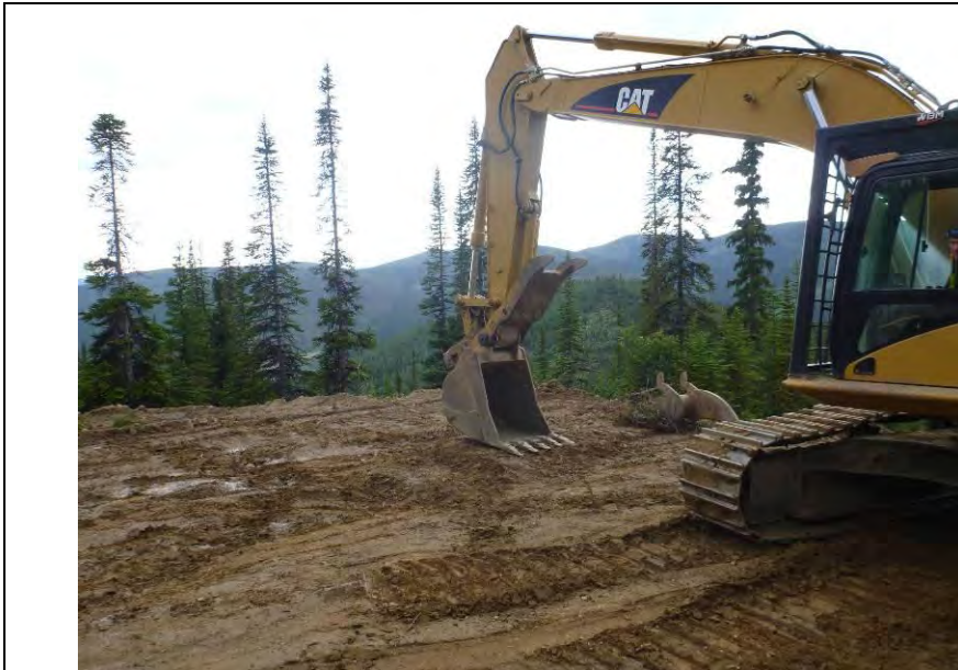
TP-BGC11-53 – Site photo; drill pad of BH-BGC11-27.
