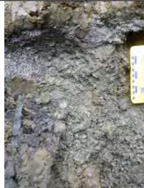
TP-BGC11-143 – Detail of pit wall 0.0-0.5 m.
