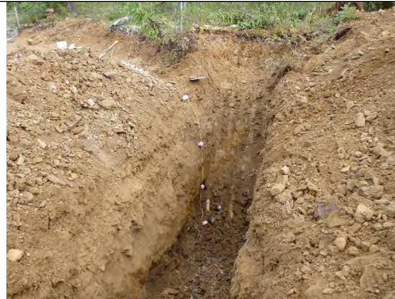
TP-BGC11-57 – Back wall of test pit; pit completed at depth of 5.0 m.
