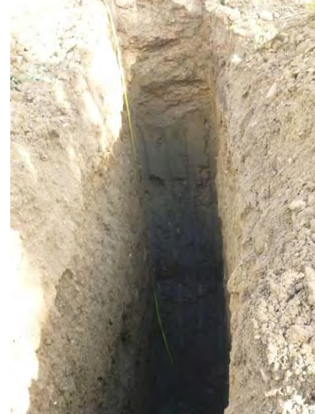
TP-BGC11-115 – Back wall of test pit; pit completed at a depth of 5.7 m.
