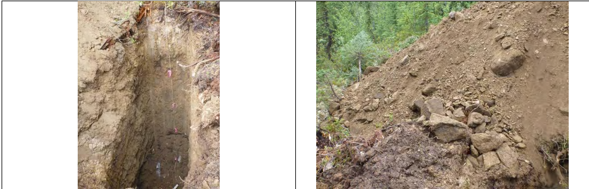
TP-BGC11-94 – Back wall of test pit; pit completed at a depth of 5.0 m.
