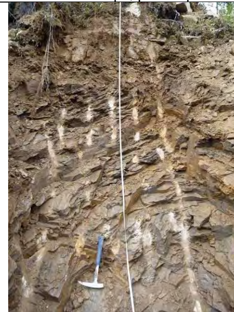
TP-BGC11-80 – Detail of pit wall.
