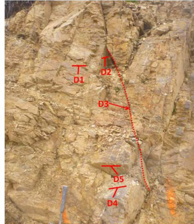
PHOTO OF STRUCTURE, UNIT D
