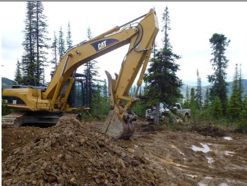
TP-BGC11-57 – Site photo; drill pad of BH-BGC11-26.
