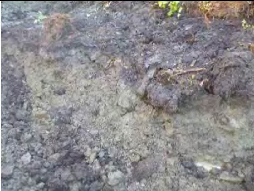
TP-BGC11-144 – Detail of back wall; pit abandoned due to seepage.
