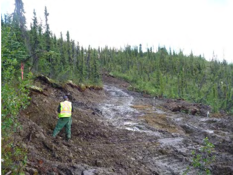
TP-BGC11-59 – Site photo; drill pad of BH-BGC11-50.
