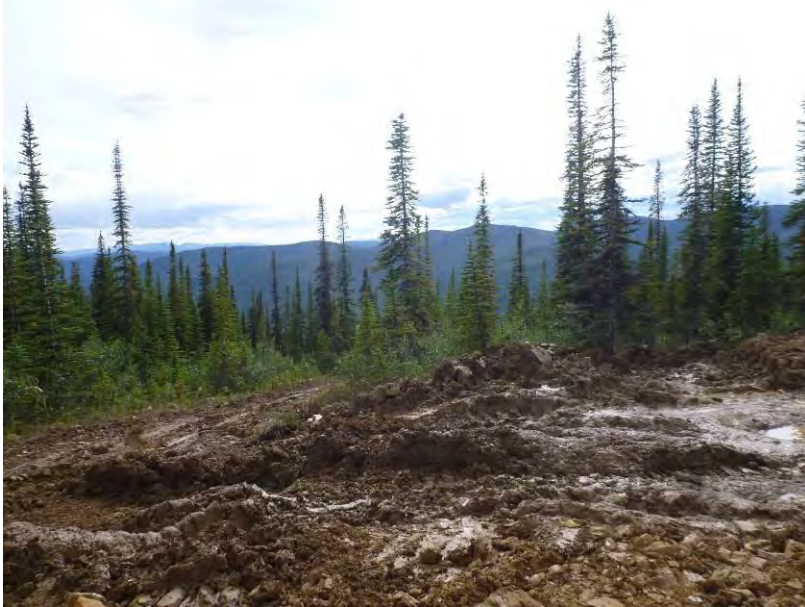
TP-BGC11-54 – Site photo; drill pad of BH-BGC11-25.
