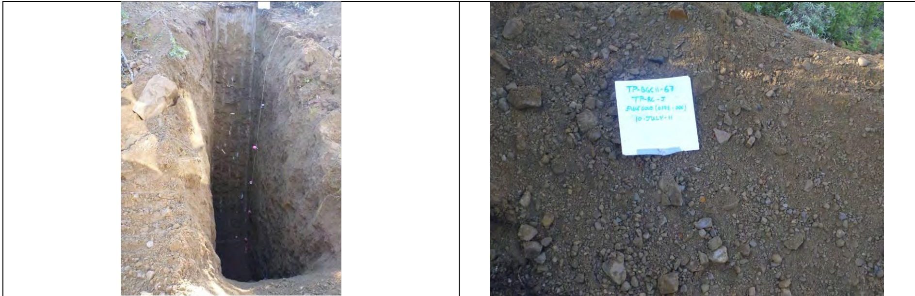
TP-BGC11-67 – Back wall of test pit; pit completed at depth of 6.5 m.
