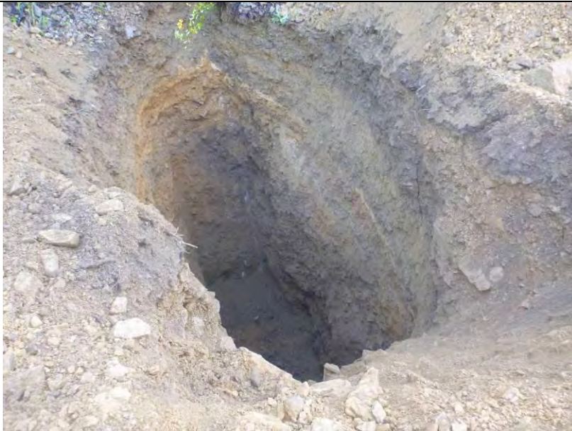
TP-BGC11-117 – Pit completed at depth of 8.0 m.
