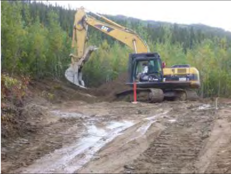
TP-BGC11-136 – Site photo; drill pad of BH-BGC11-52.
