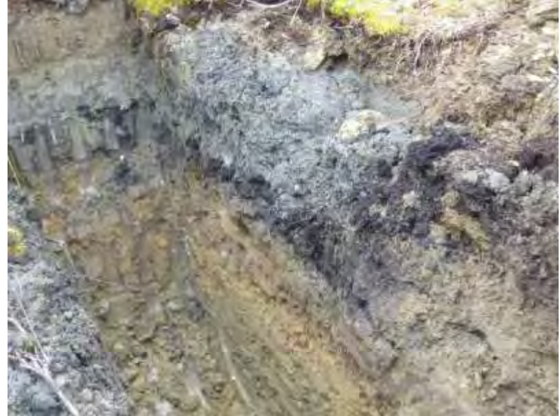
TP-BGC11-143 – Back wall of test pit; pit completed at a depth of 2.2 m.
