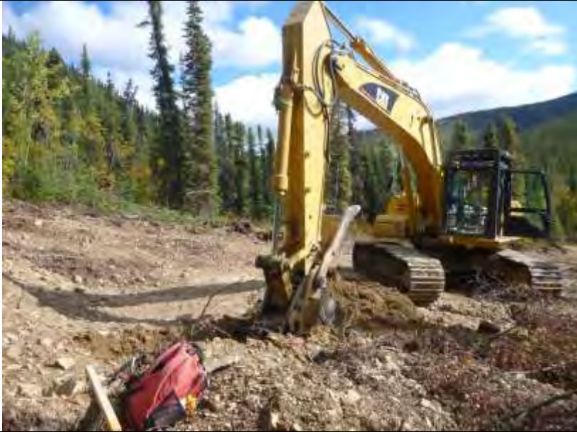
TP-BGC11-145 – Site photo; drill pad of BH-BGC11-31.
