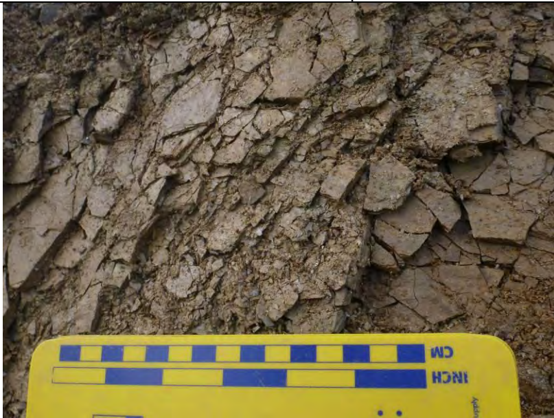
TP-BGC11-118 – Detail of highly weathered bedrock in bucket from 2.3 m.
