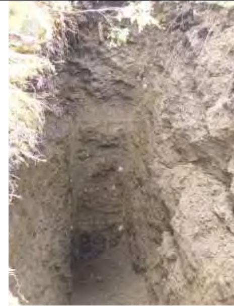
TP-BGC11-141 – Back wall of test pit; pit completed at a depth of 4.95 m.
