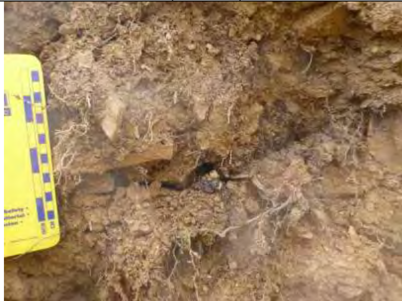
TP-BGC11-145 – Detail of wall at 0.5 m.
