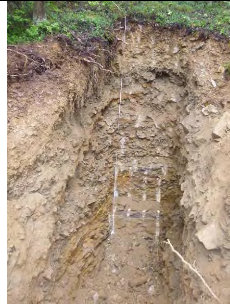
TP-BGC11-132 – Back wall of test pit; pit completed at a depth of 5.3 m.
