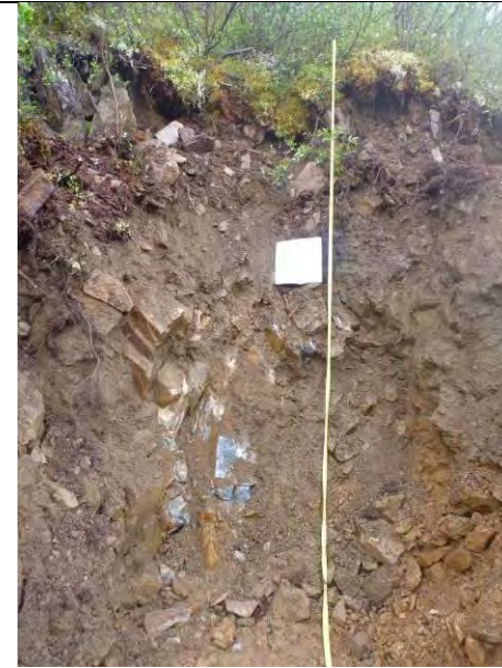
TP-BGC11-70 – Cut slope wall; pit completed at depth of 3.0 m.
