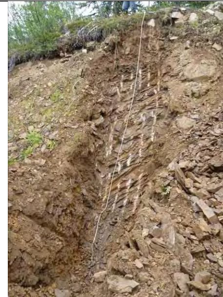
TP-BGC11-80 – Back wall of test pit; pit completed at a depth of 6.7 m.
