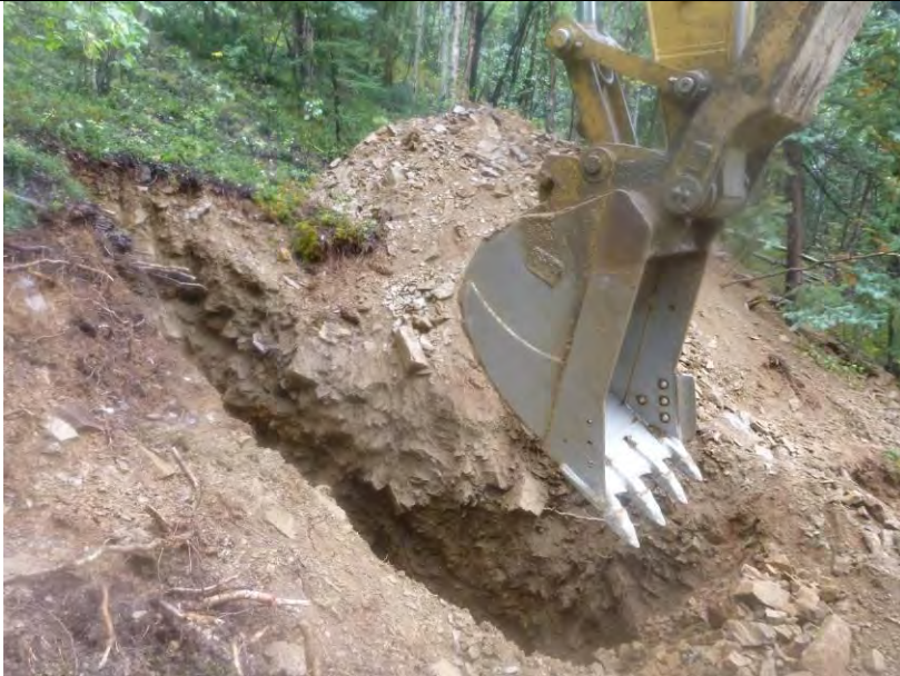
TP-BGC11-132 – Site photo after completion of test pit.
