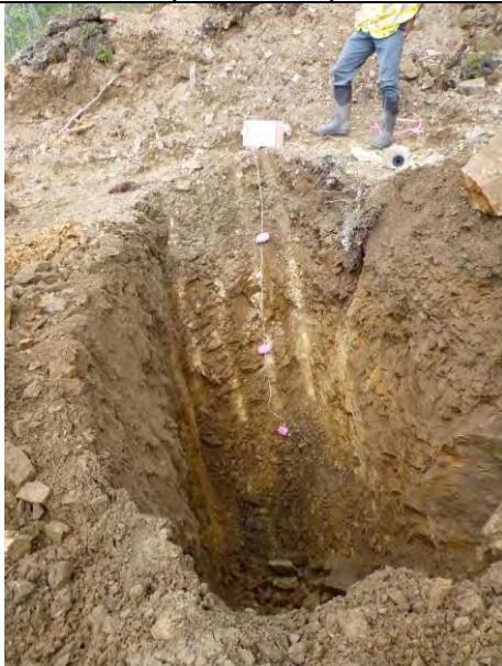
TP-BGC11-50 – Pit back wall; pit completed at a depth of 5.8 m.
