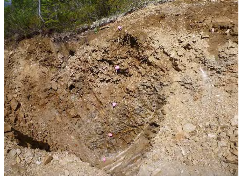
TP-BGC11-52 – Cut slope and test pit; pit completed at depth of 5.0 m.
