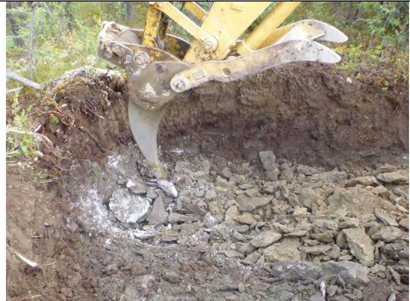
TP-BGC11-125 – Using ripper shank to penetrate frozen ground.
