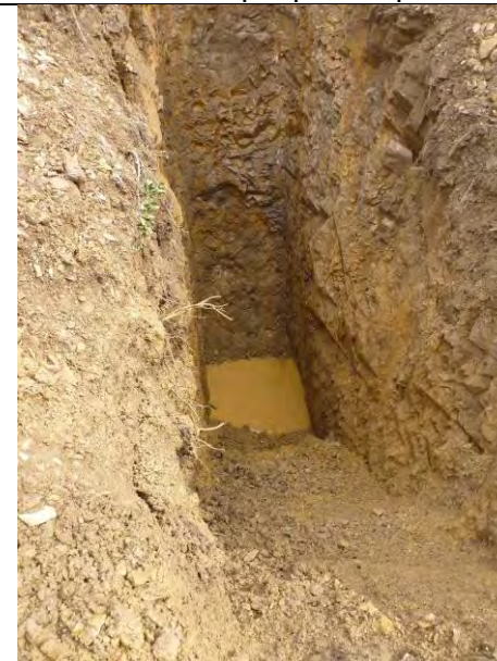
TP-BGC11-78 – Water collected in pit from seepage through the walls.
