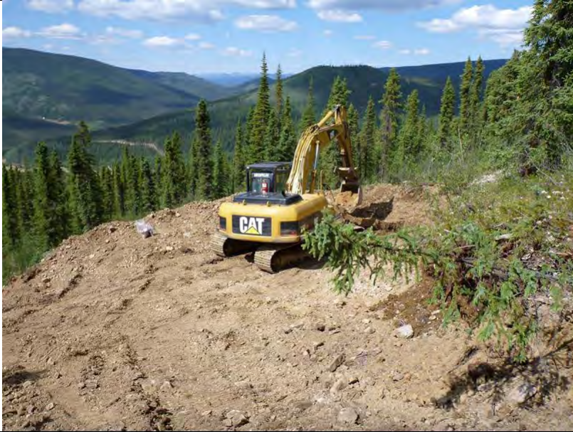
TP-BGC11-50 – Site photo; drill pad of BH-BGC11-36.
