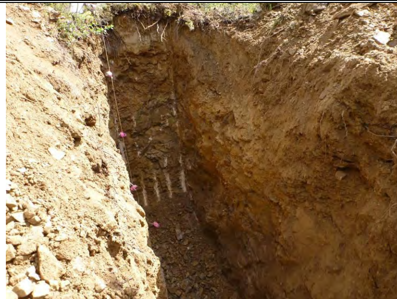
TP-BGC11-61 – Cut slope and test pit; pit completed at depth of 2.7 m.
