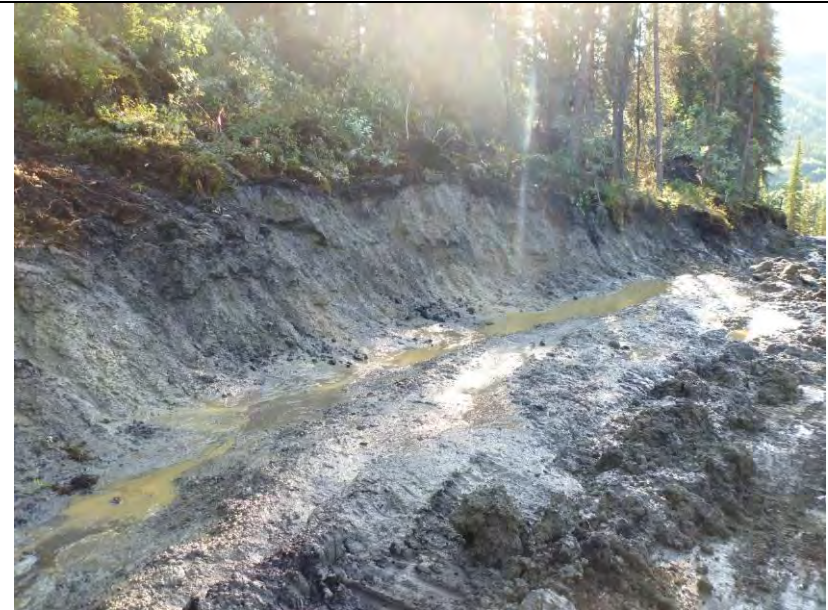
TP-BGC11-71 – Cut slope from access construction.
