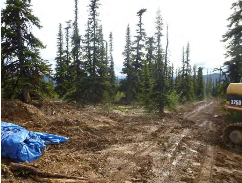
TP-BGC11-55 – Site photo; drill pad of BH-BGC11-24.
