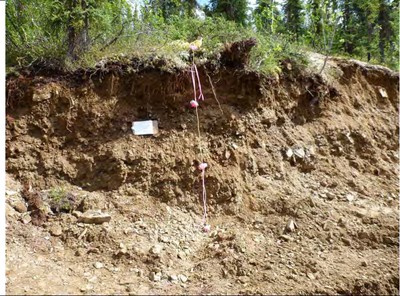
TP-BGC11-50 – Cut slope from construction of drill pad.
