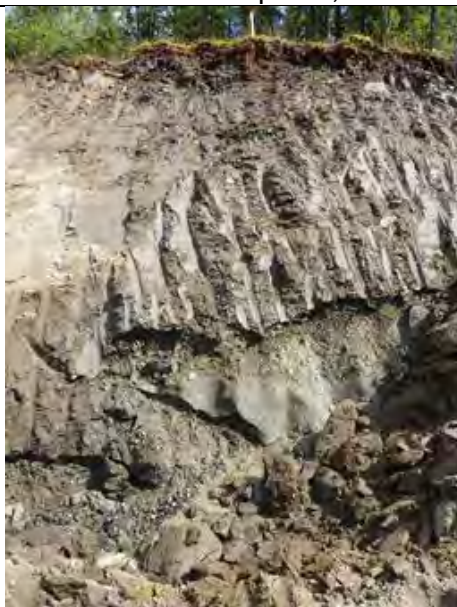
TP-BGC11-82 – Back wall of test pit; pit completed at a depth of 7.0 m.
