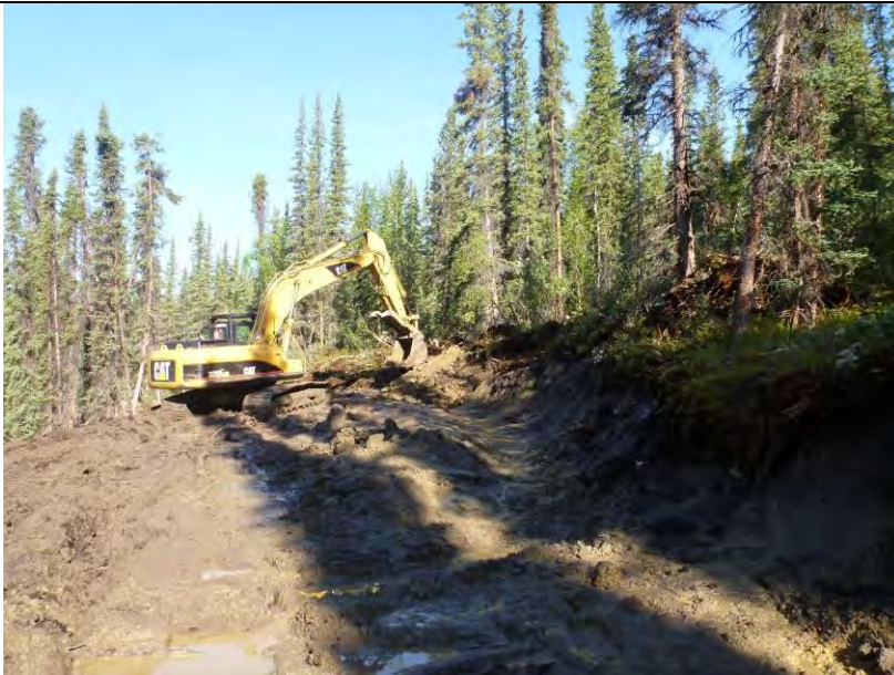
TP-BGC11-71 – Site photo; drill pad of BH-BGC11-59.
