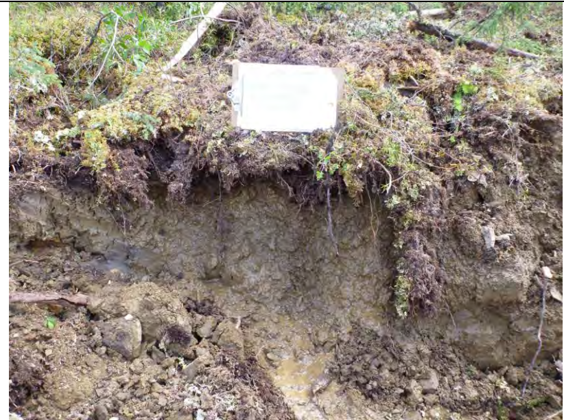
TP-BGC11-51 – Cut slope from access construction; frozen ground.
