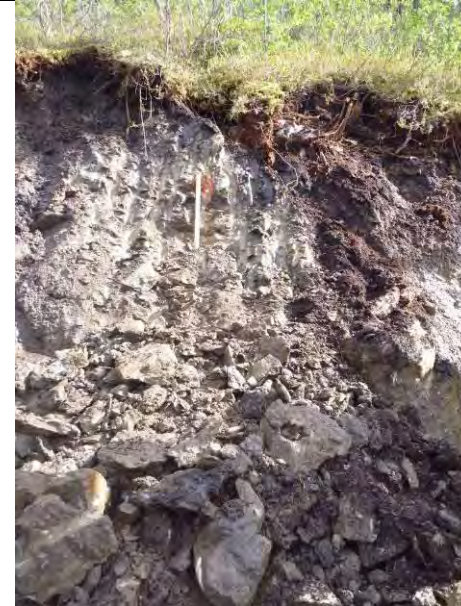
TP-BGC11-106 – Back wall of test pit; pit completed at a depth of 3.0 m.
