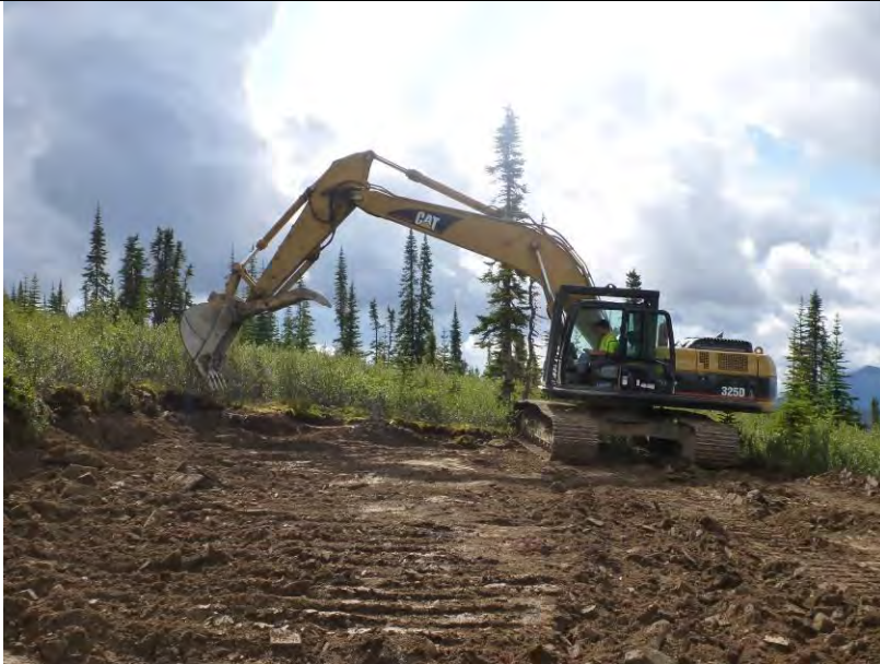
TP-BGC11-102 – Site photo; drill pad of BH-BGC11-45.
