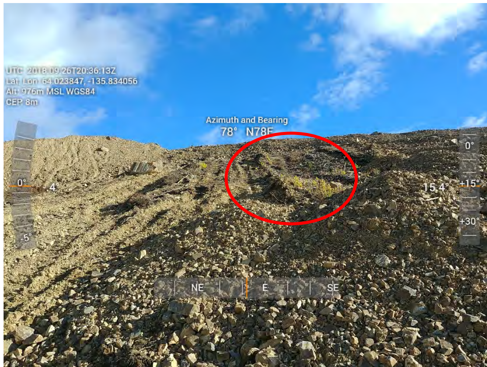
Figure 23: 90 Day Stockpile - Organics in phase 2 foundation (typical).
