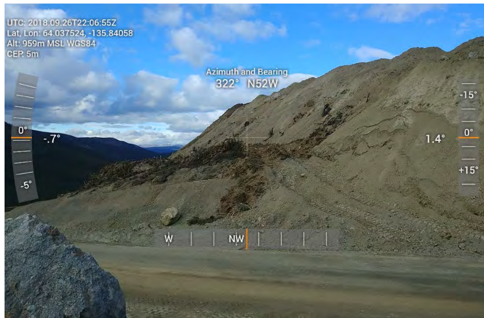
Figure 27: ADR - Common material stockpile with over steepened slopes.
