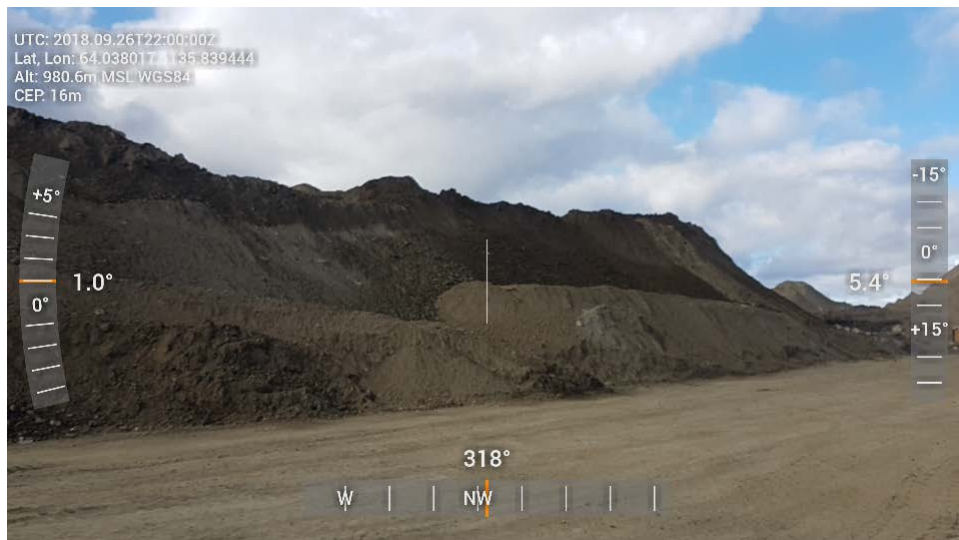
Figure 28: ADR - Common material stockpile with over steepened slopes.
