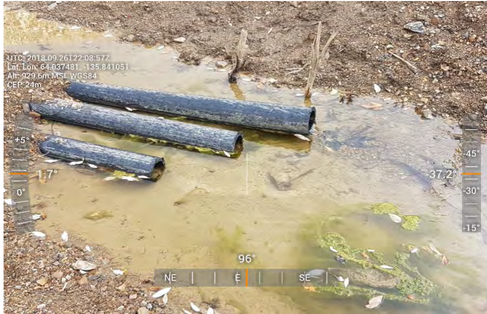
Figure 11: LDSP - Low level outlet pond.
