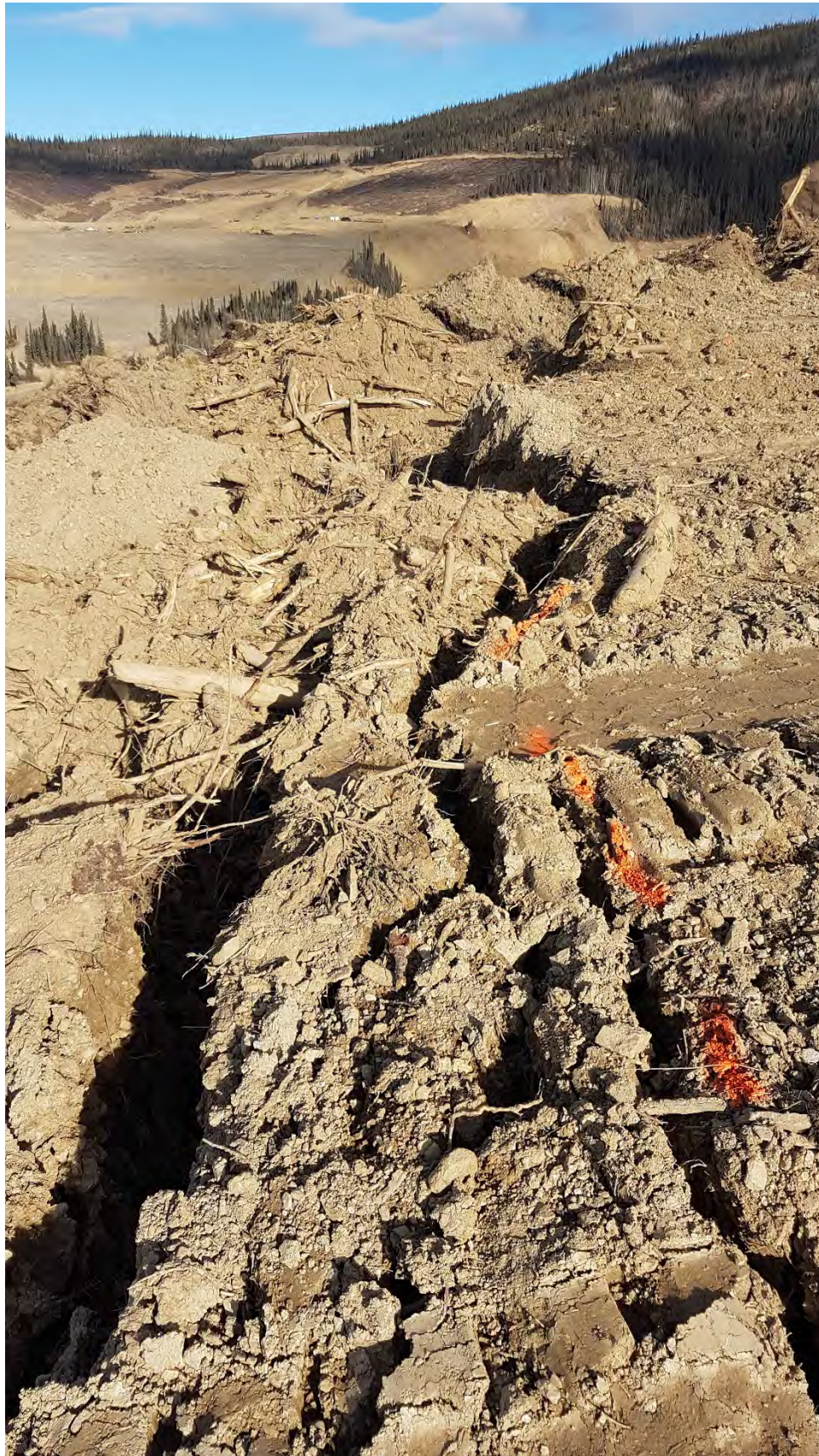
Figure 49: Stockpile B - West end tension cracking.
