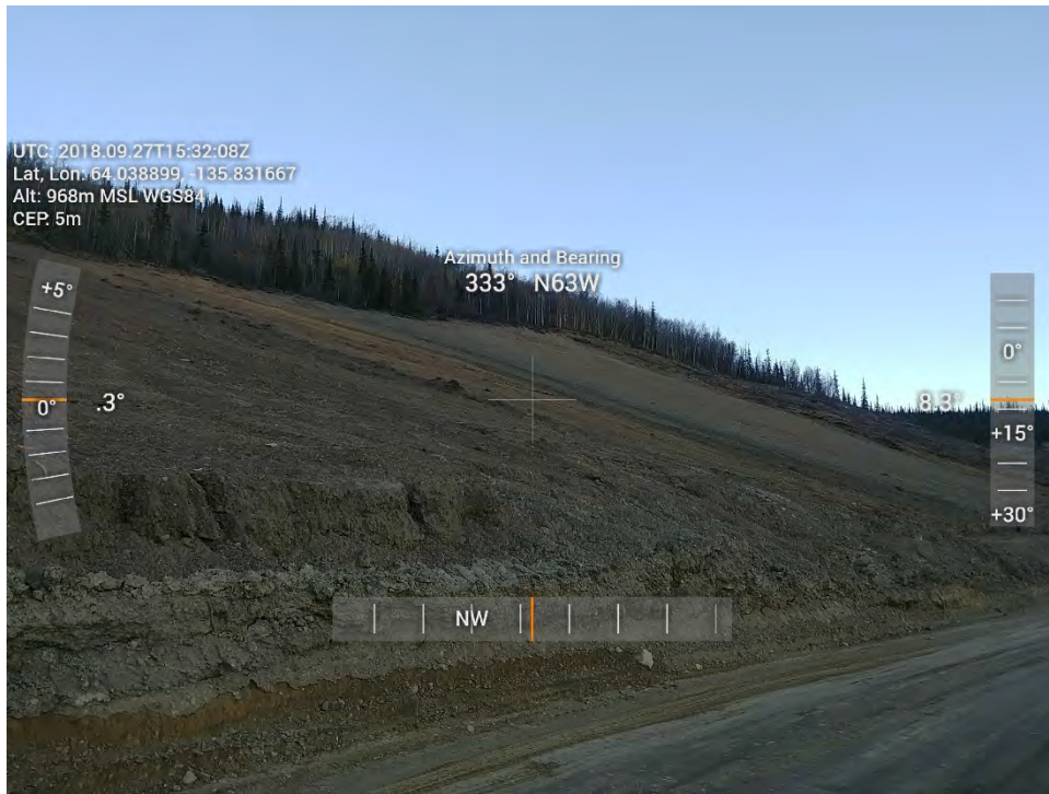
Figure 33: HLF - Phase 1B northwest slope.
