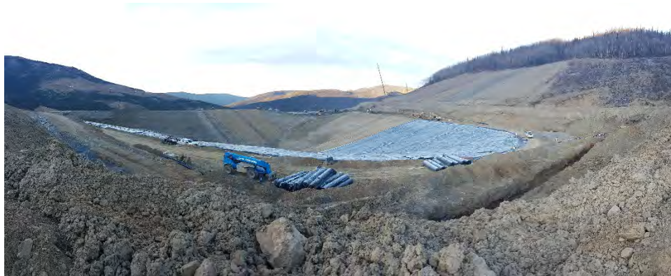
Figure 31: HLF - Construction (facing south).
