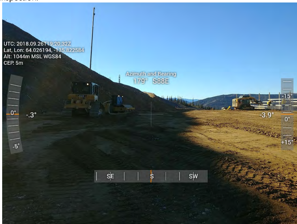
Figure 15: SC MSE - Equipment used for MSE wall construction.
