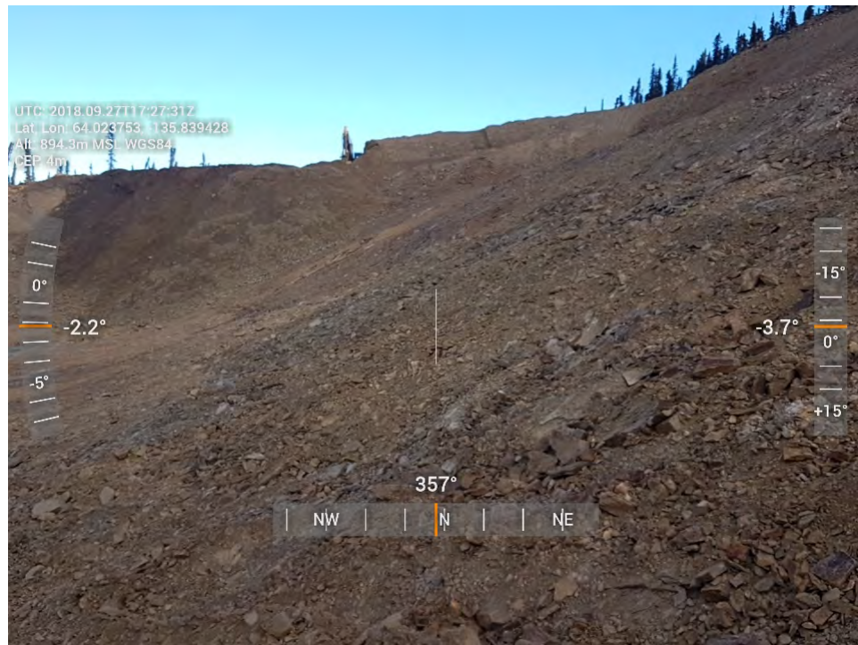
Figure 44: Stockpile A - lower slopes.
