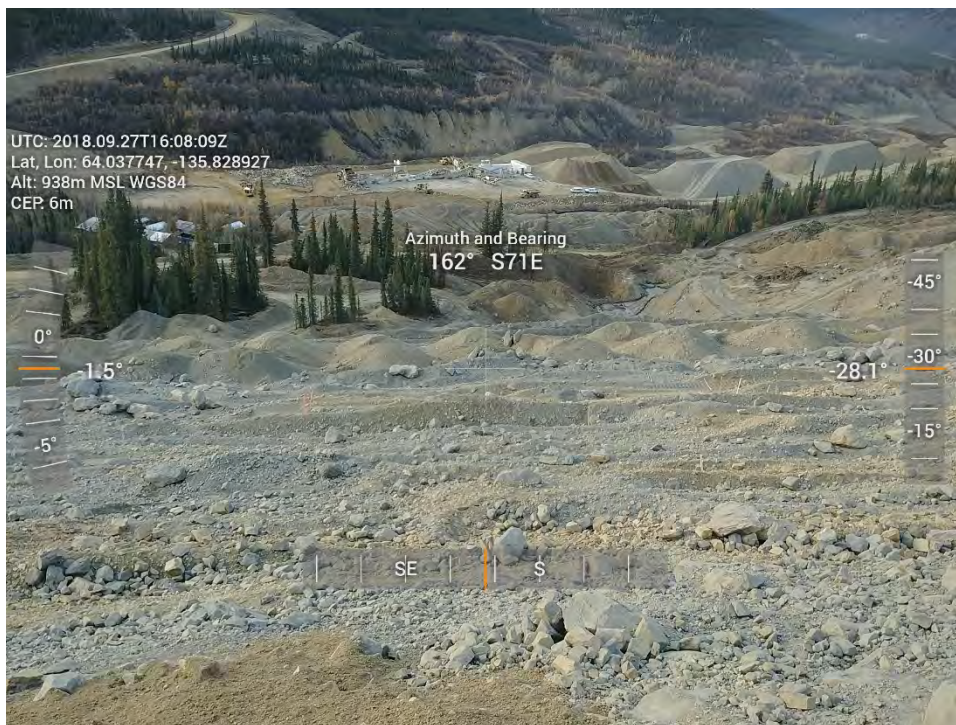
Figure 37: HLF - Free face with heaped material and perched rock.
