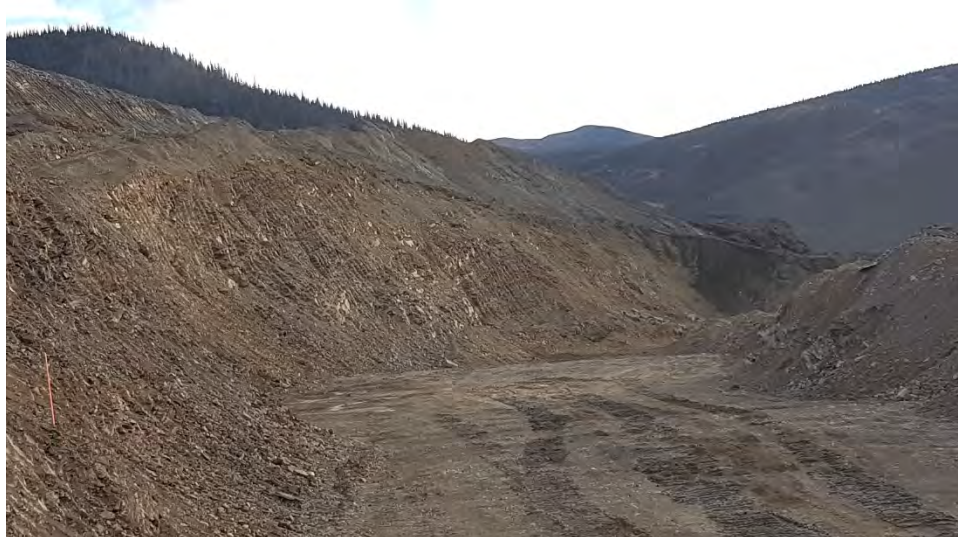
Figure 39: Event pond (facing east) – rock cuts.
