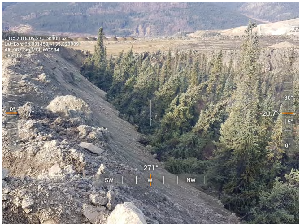
Figure 46: Stockpile B - Toe of slope encroaching on organics.
