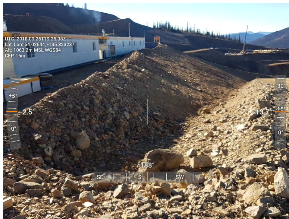
Figure 17: SC MSE - Slope below secondary crusher pad.
