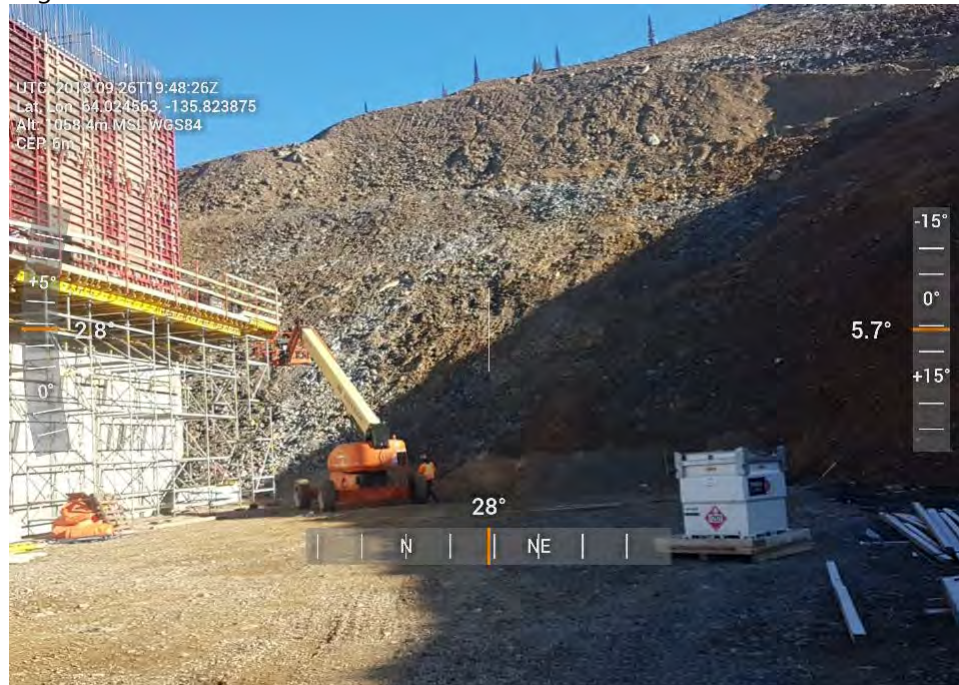
Figure 13: Slope behind primary crusher.
