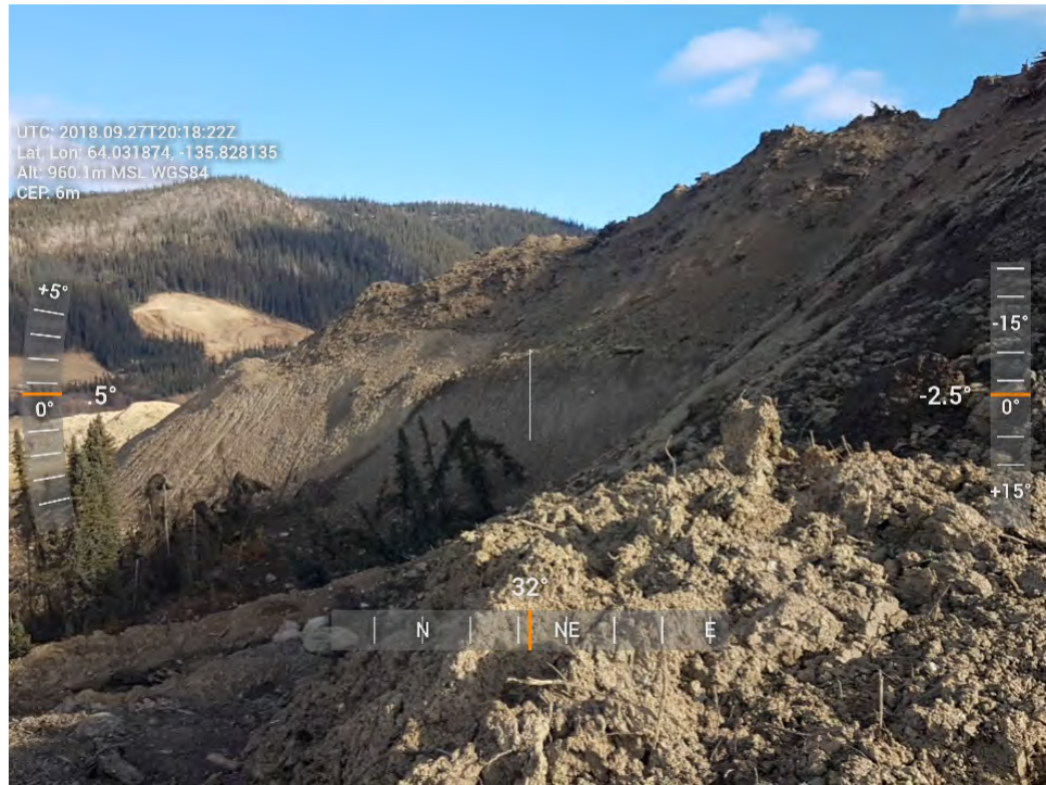
Figure 54: Stockpile B - Outside slope (Typical).
