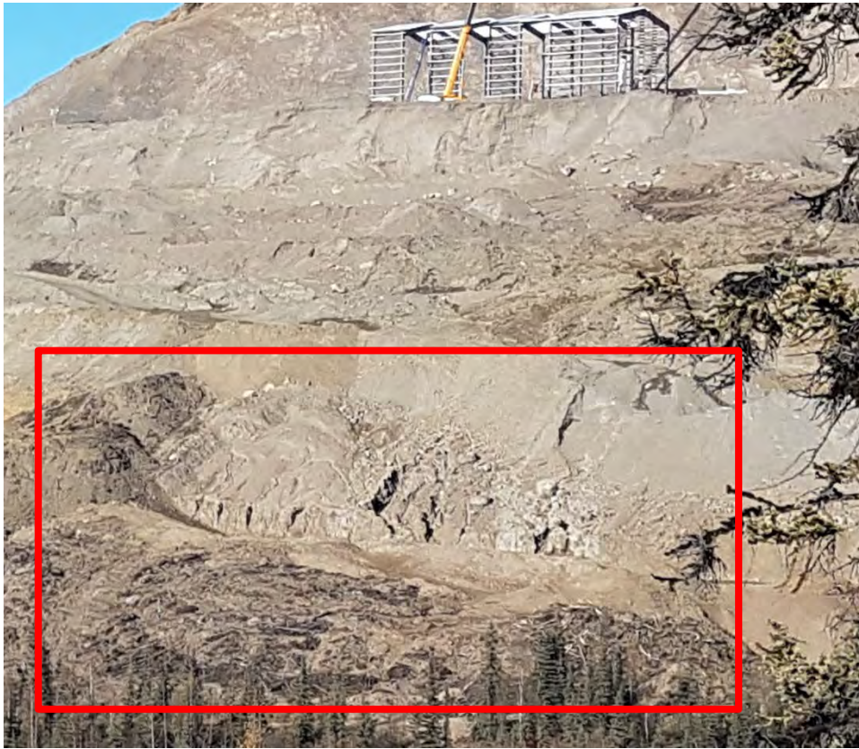
Figure 38: HLF - Erosion and material flows west of confining embankment.
