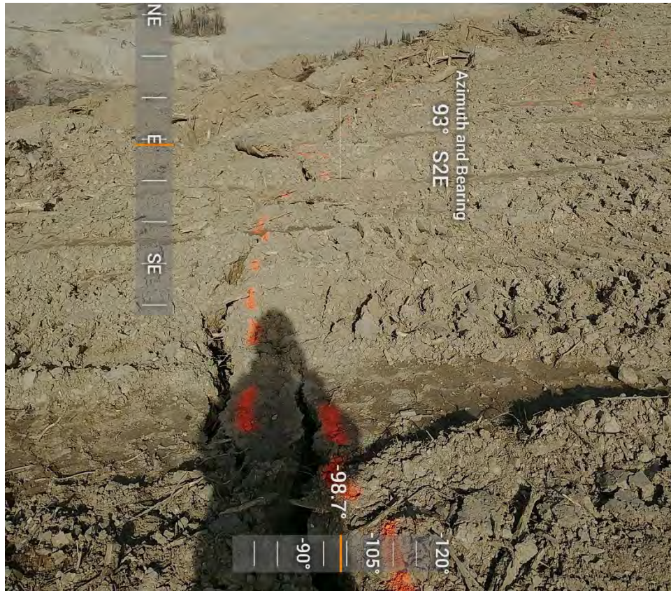
Figure 47: Stockpile B - West end tension cracking.
