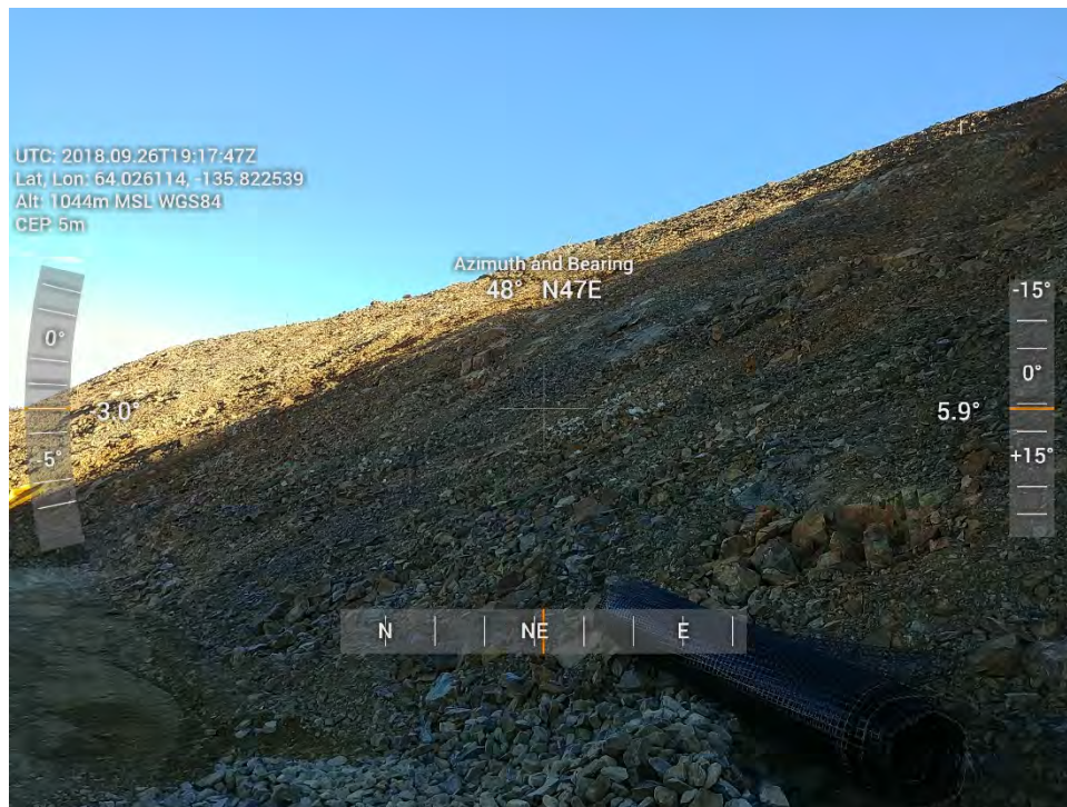
Figure 16: SC MSE - Slope behind secondary crusher MSE wall.
