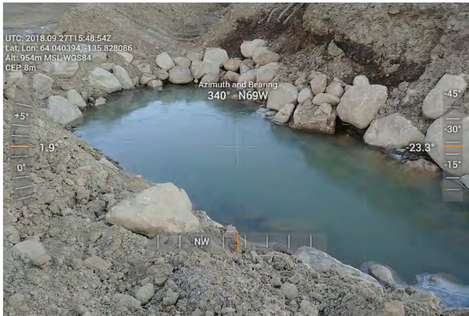
Figure 34: HLF - Ponded water above collection ditch.
