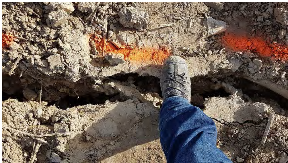
Figure 48: Stockpile B - West end tension cracking.
