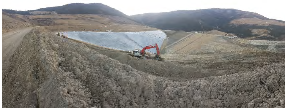
Figure 32: HLF - Construction (facing north).
