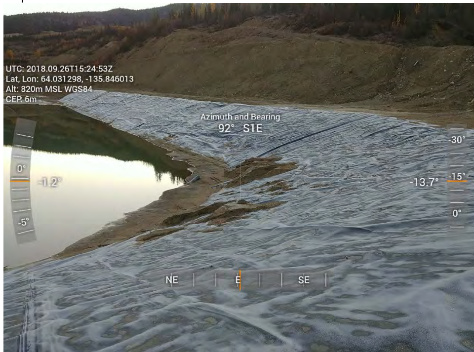
Figure 12: Sediment carried onto collection pond liner.
