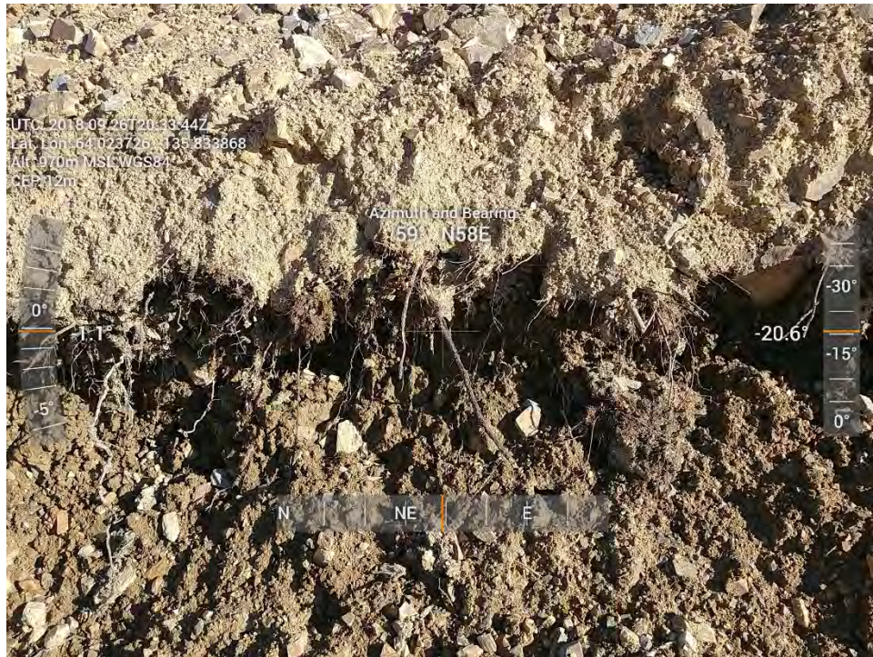
Figure 22: 90 Day Stockpile – Organic layer near west edge.
