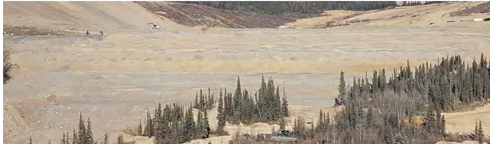
Figure 36: HLF - Free face with heaped material and perched rock.
