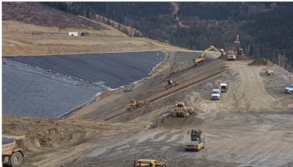
Figure 30: HFL - Confining embankment construction.
