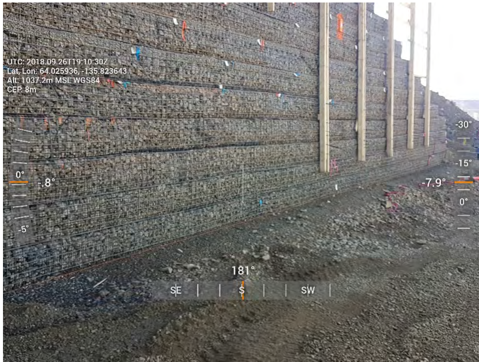
Figure 18: SC MSE - Secondary crusher MSE wall.
