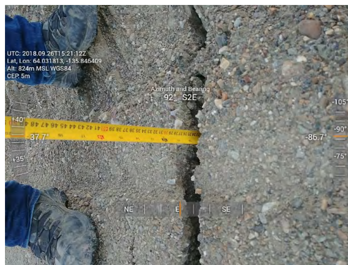
Figure 2: LDSP - Tension cracking on south dam.
