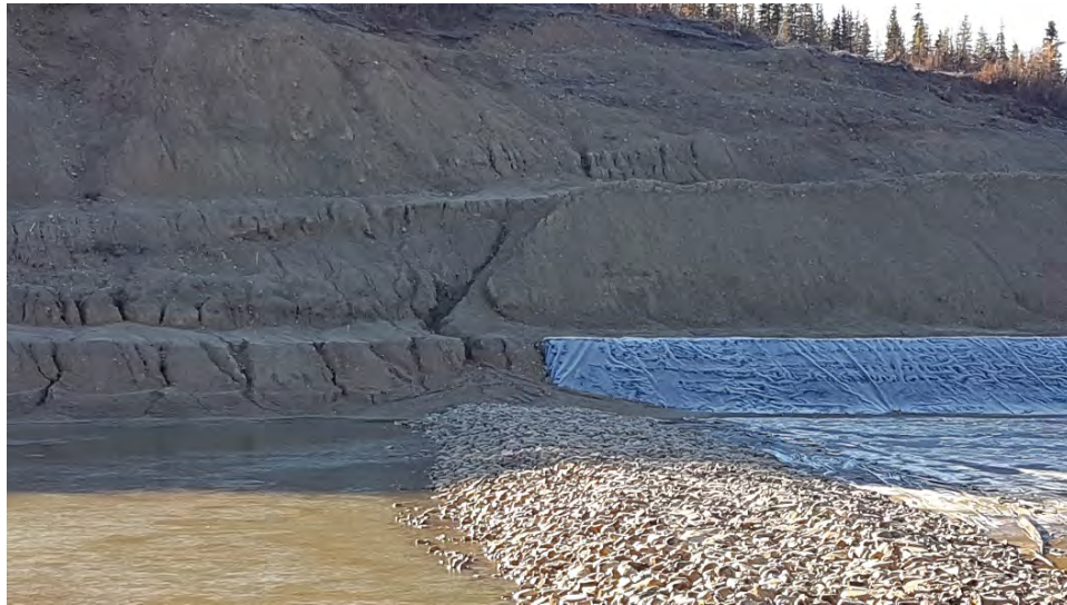
Figure 3: LDSP - Erosion at the southern side near the fore bay berm.
