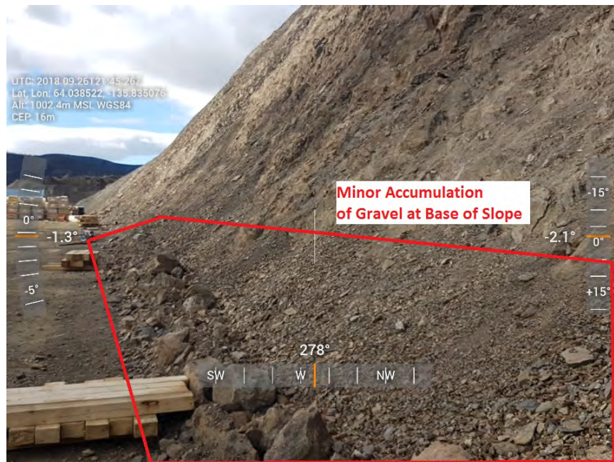
Figure 25: ADR - Minor accumulation of gravel at base of cut slope.
