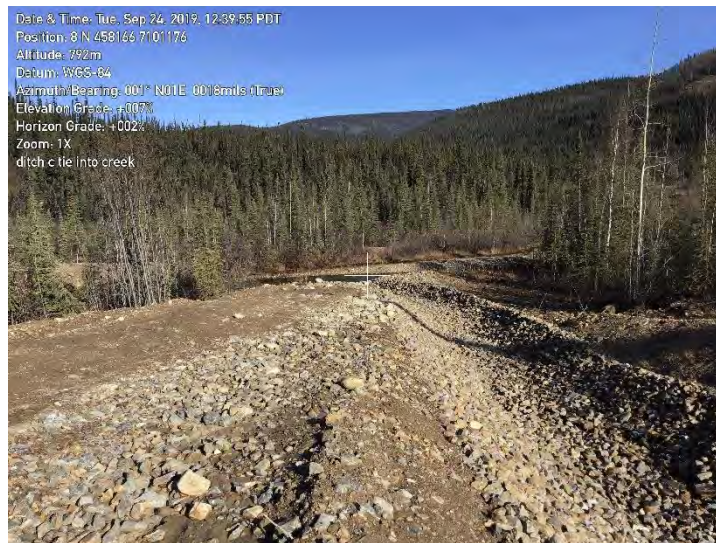
Figure 54: Ditch C Outfall to Haggart Creek
