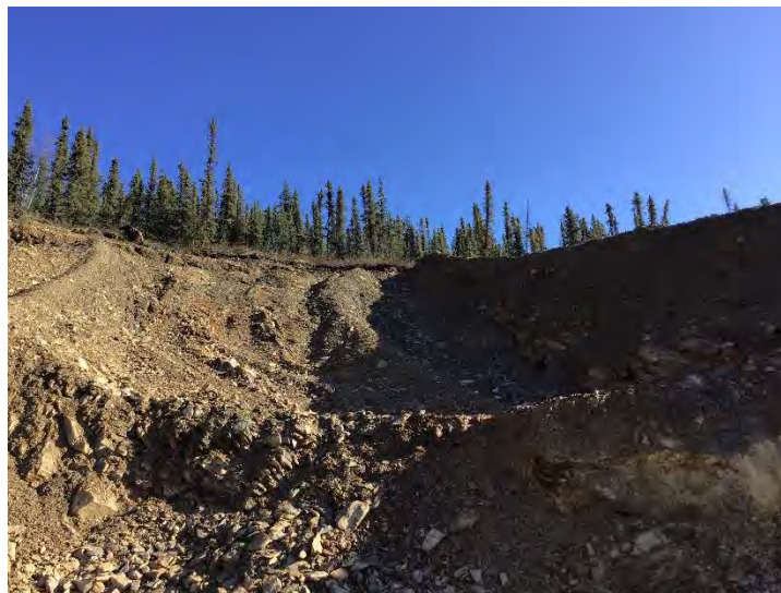
Figure 57: Sediment control sump
