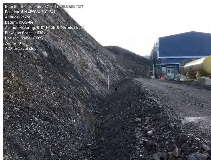
Figure 38: Typical North Toe Ditch cross section
