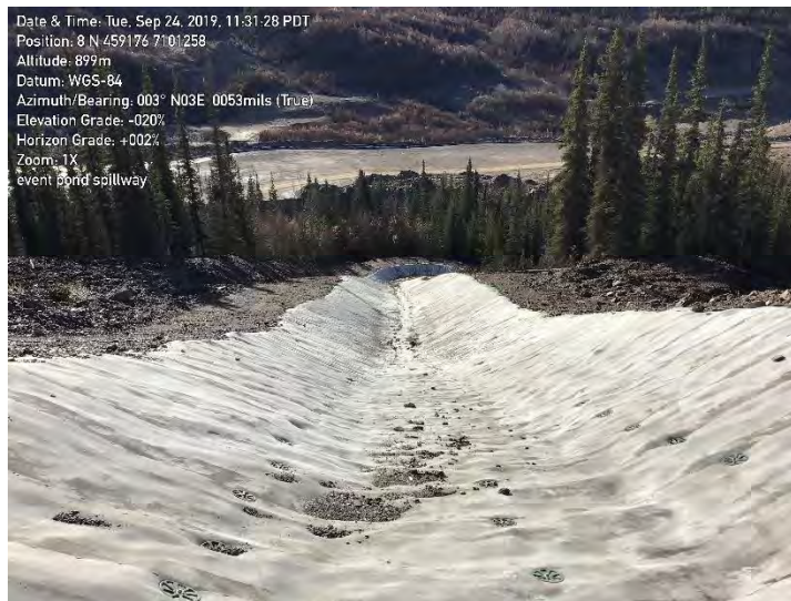
Figure 45: Events Pond Emergency spillway
