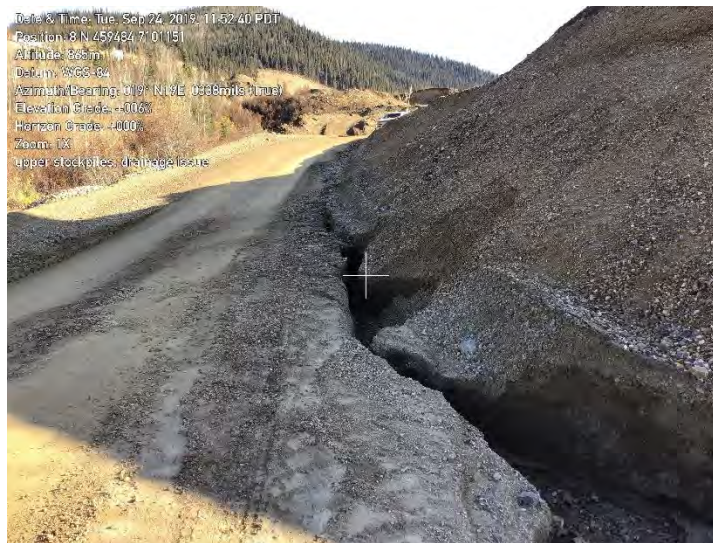
Figure 59: Scouring and gully forming adjacent to stockpiles
