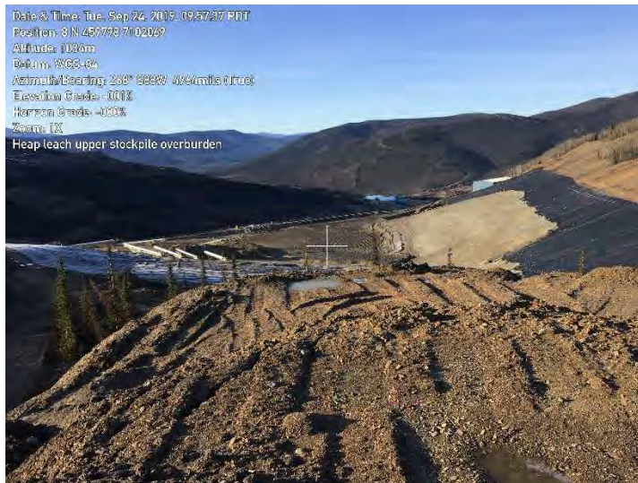
Figure 18: Top of stockpile
