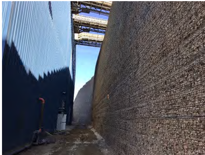
Figure 35: MSE wall behind secondary/tertiary crusher
