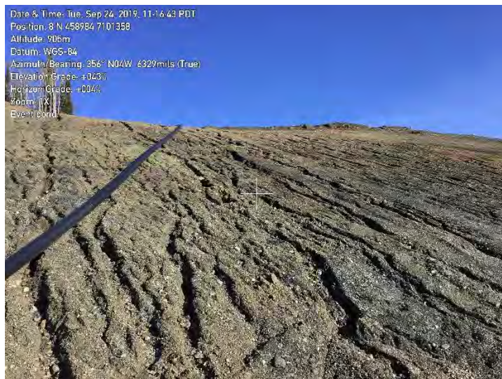
Figure 42: Slopes from heap leach spillway
