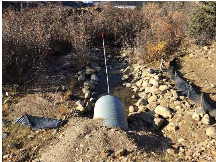
Figure 62: Dublin Gulch Culvert Outlet
