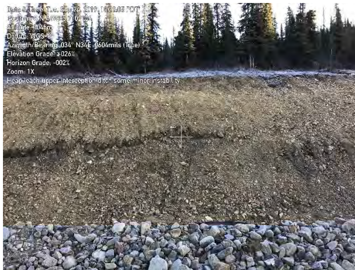
Figure 21: Sloughing slope
