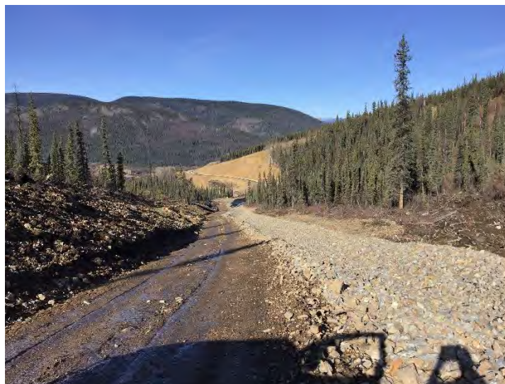
Figure 46: Looking down Ditch A
