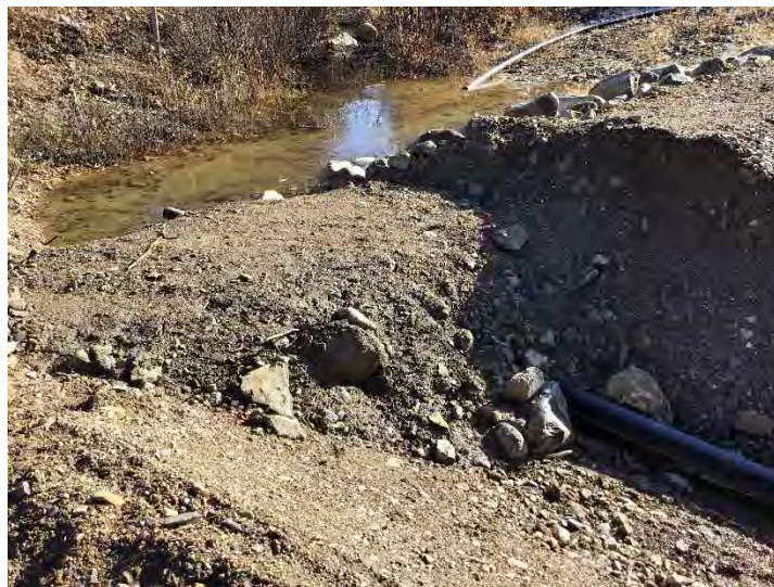
Figure 50: Top of Ditch B
