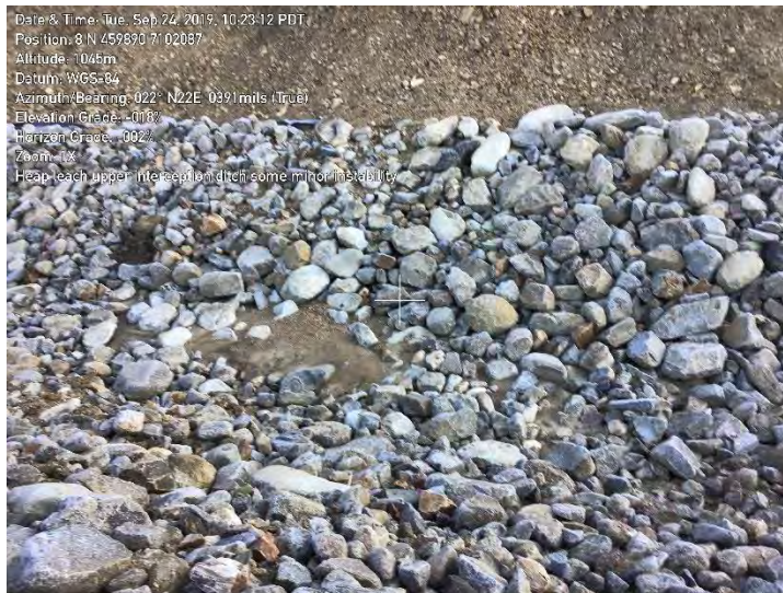
Figure 22: Material deposited into ditch
