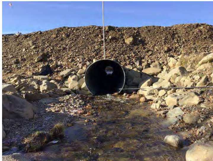
Figure 61: Dublin Gulch Culvert Inlet
