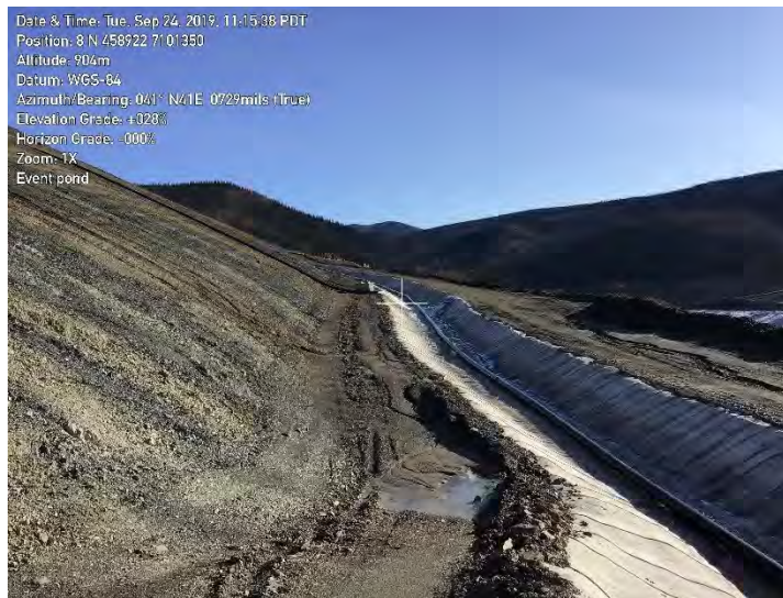
Figure 43: Slopes from heap leach spillway
