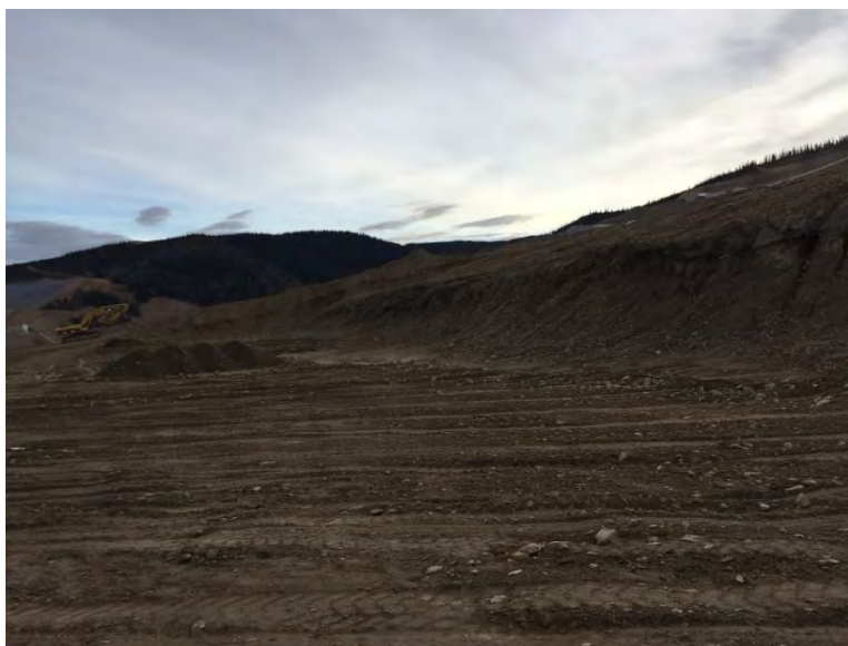
Figure 13: Secondary Stockpile Cut Slopes 2020
