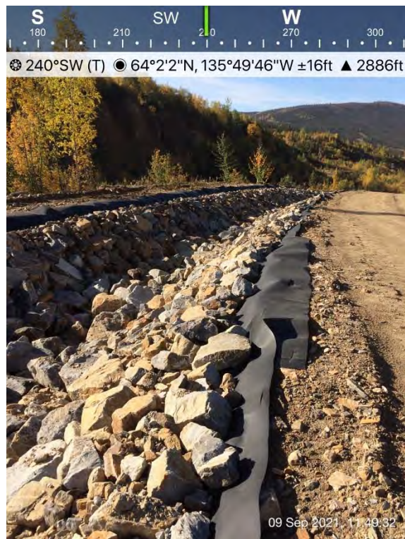
Figure 56: Ditch B (view towards LDSP)
