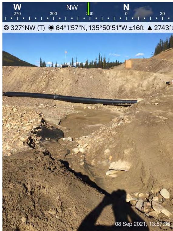
Figure 60: Dried sediment above Ditch C (2021)
