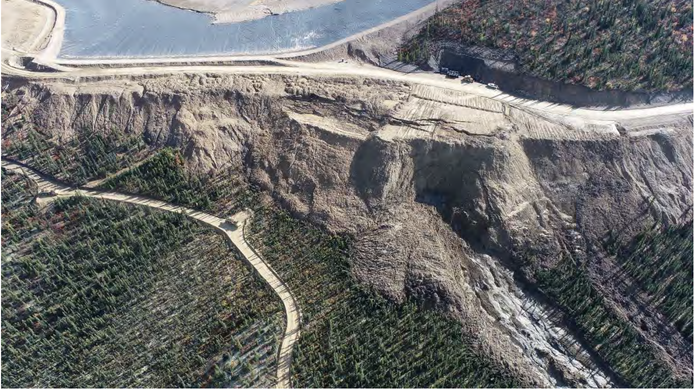
Figure 28: HLF Overburden Stockpile collapse – plan view
