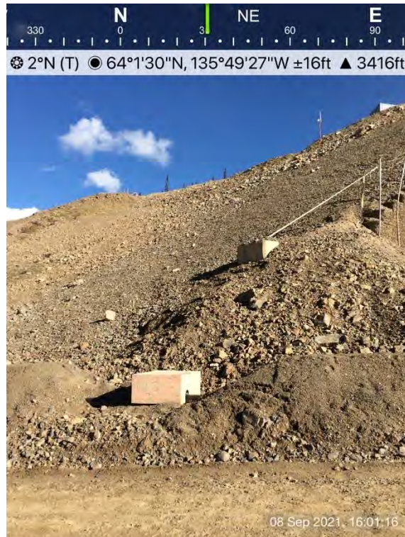
Figure 39: North-West fill slopes
