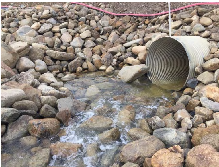
Figure 5: LDSP - 1500mm Culvert 2020 Inspection
