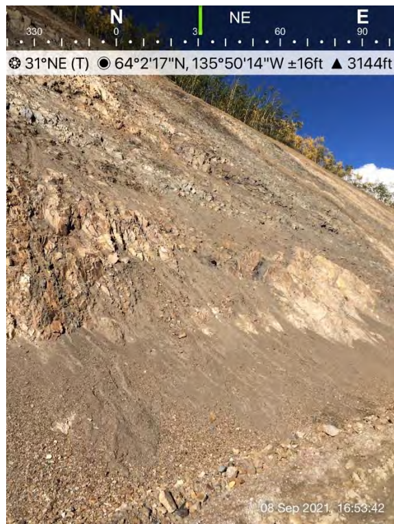
Figure 44: Slopes behind ADR (2021)
