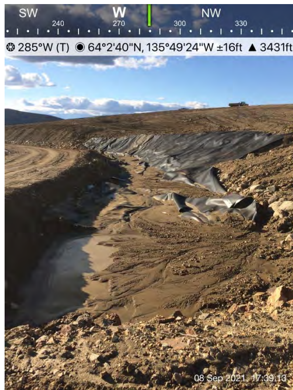
Figure 24: Material deposited in HLF Phase 1B Interceptor Ditch
