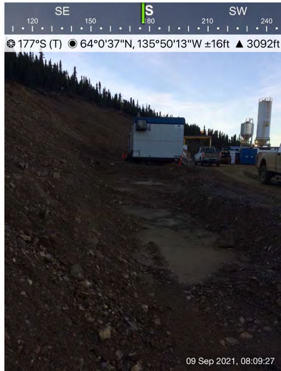
Figure 63: Orica ditch sediment build-up
