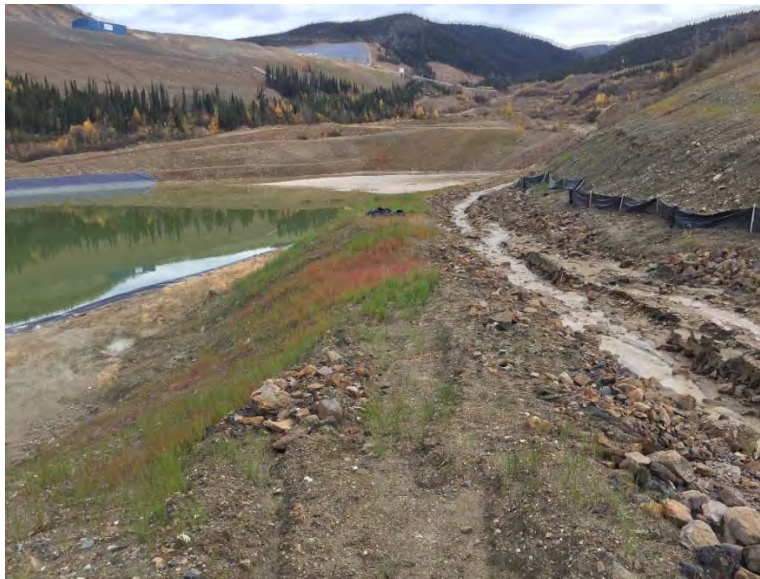
Figure 8: LDSP – Erosion on the Southwest slope 2020
