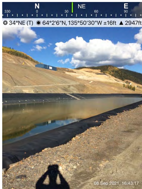
Figure 46: Overall view of event pond
