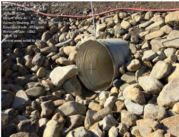
Figure 4: LDSP - 1500mm Culvert 2019 Inspection
