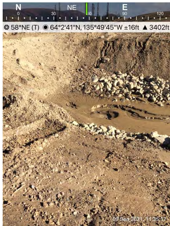
Figure 25: Phase 1B Interception Ditch buried drain pipe
