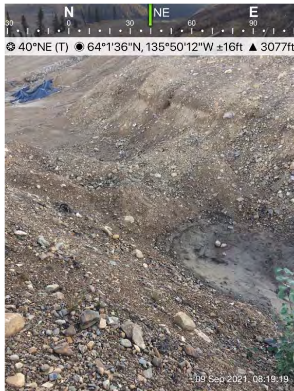
Figure 18: Unconnected Ditch Section 2021
