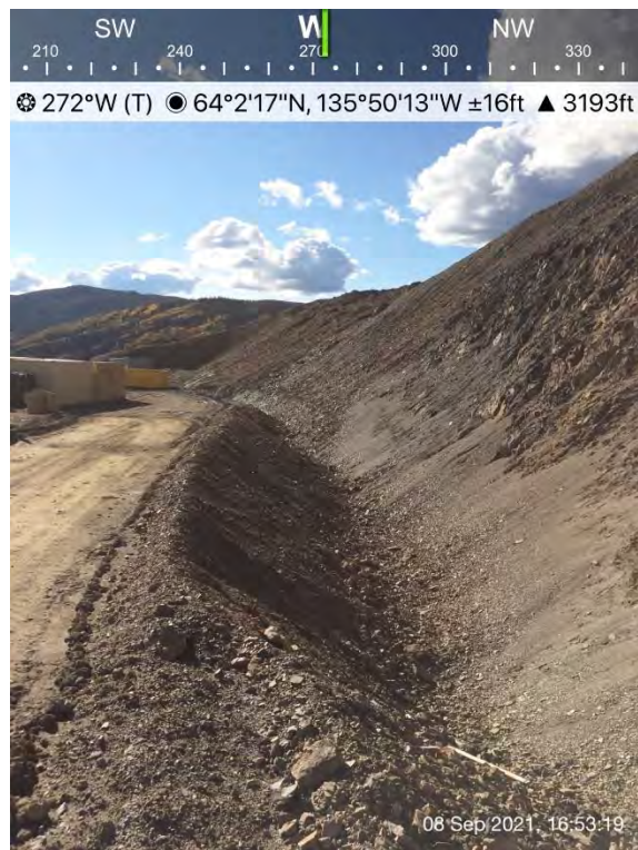
Figure 45: Typical North Toe Ditch cross section
