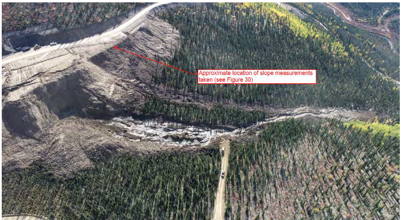
Figure 29: HLF Overburden Stockpile collapse – plan view
