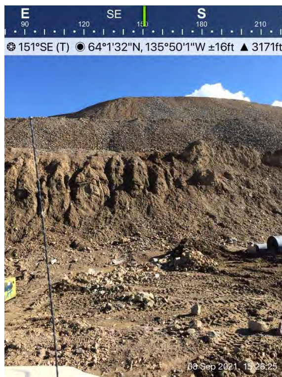
Figure 14: Secondary Stockpile Cut Slopes 2021
