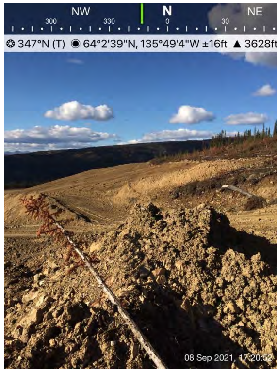
Figure 27: Phase 2 graded area
