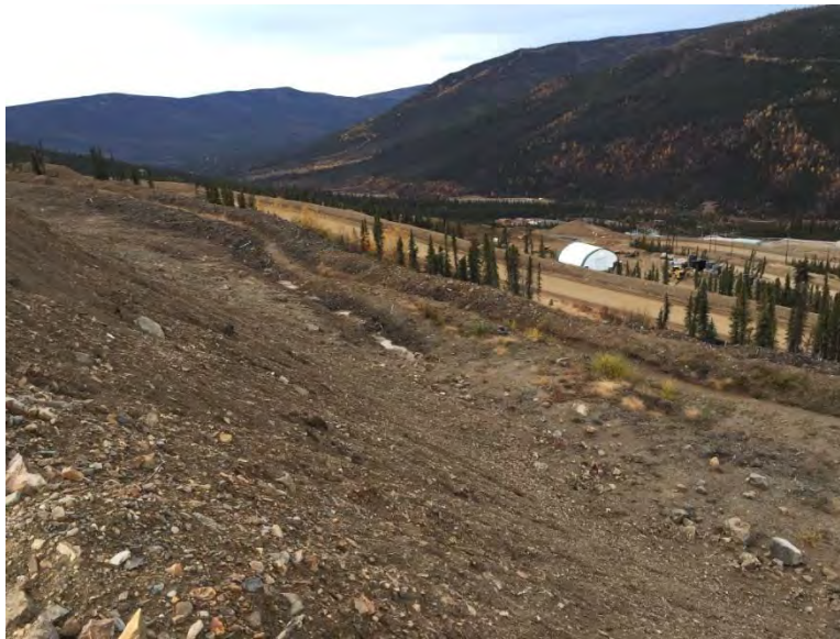
Figure 17: Unconnected Ditch Section 2020
