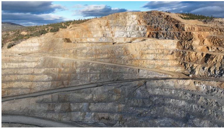
Figure 32: Open Pit Walls
