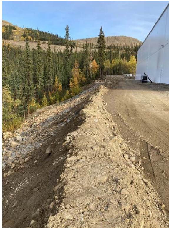
Figure 76: Water Treatment Plant Slopes
