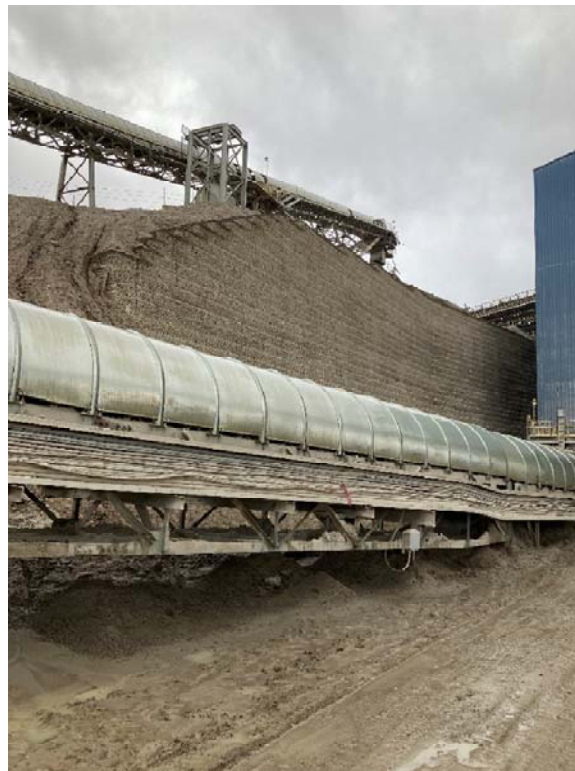
Figure 48: North side of MSE wall
