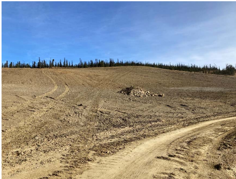
Figure 26: Phase 2 graded area
