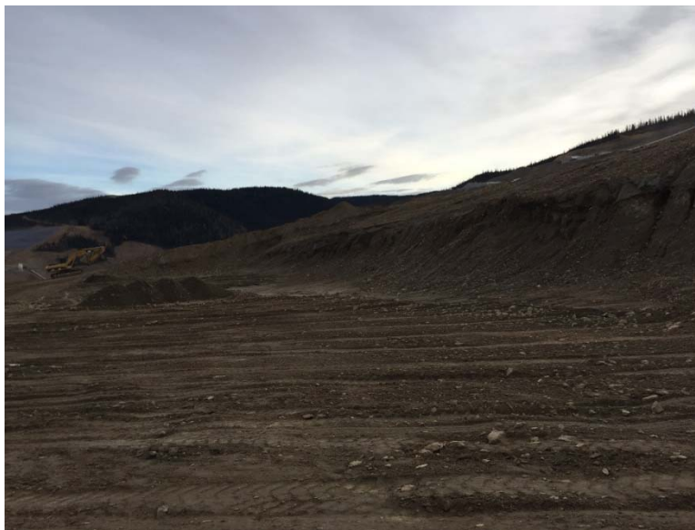
Figure 9: Secondary Stockpile Cut Slopes 2020
