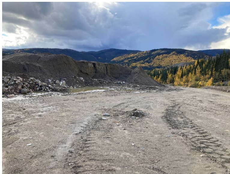
Figure 81: Additional stockpiles with steep side slopes
