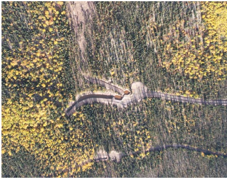
Figure 30: HLF Overburden sump system 2022
