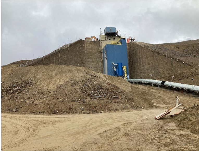
Figure 43: Primary Crusher MSE Walls
