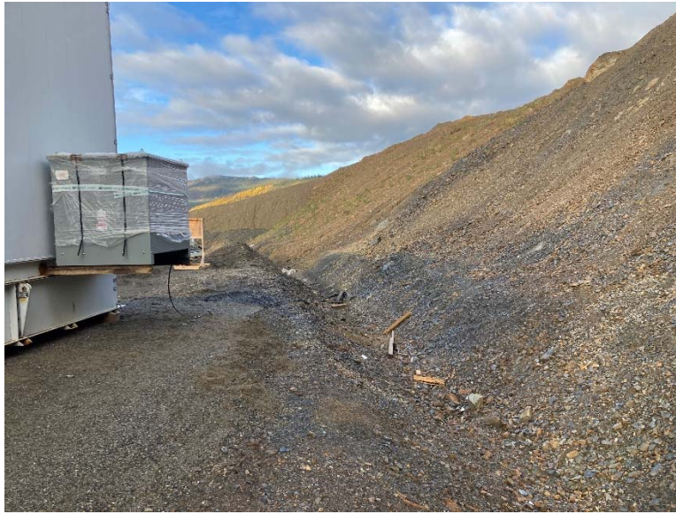
Figure 53: Typical North Toe Ditch cross section
