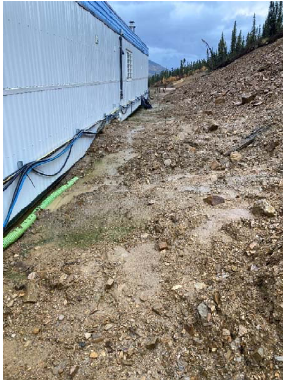
Figure 79: Orica site trailer sediment build-up
