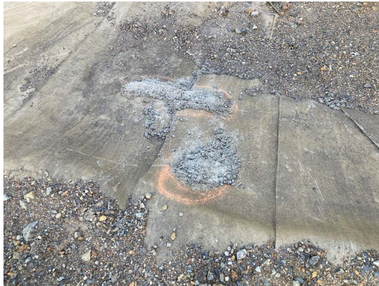
Figure 60: Heap leach spillway repairs (2022)
