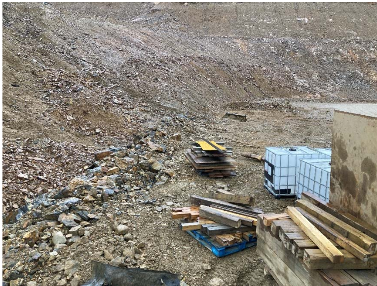
Figure 72: Truck Shop Drain Ditch Blockage
