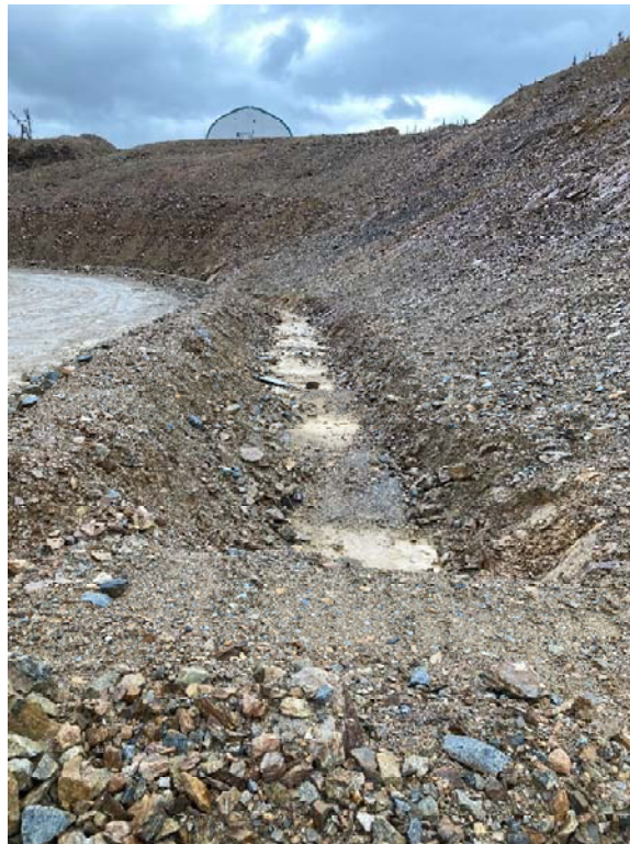
Figure 71: Truck Shop Drain Ditch
