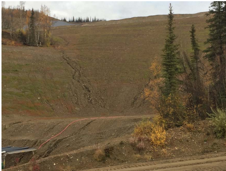
Figure 22: Scouring and rilling along toe slope of HLF (2020)
