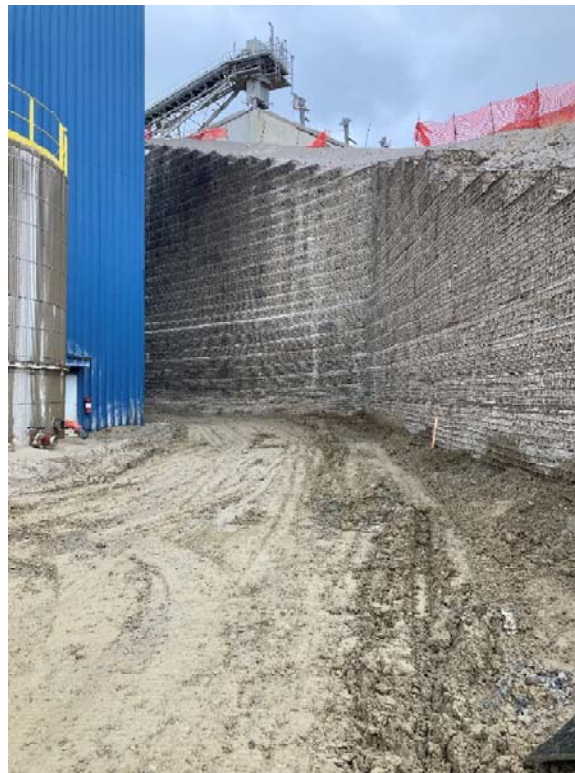
Figure 47: South side of MSE wall
