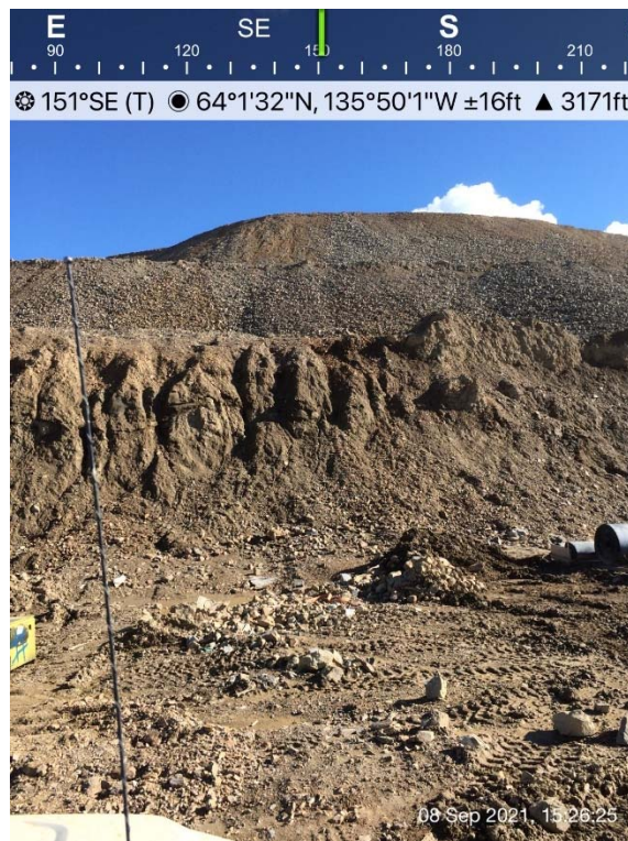
Figure 10: Secondary Stockpile Cut Slopes 2021
