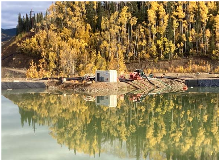
Figure 69: LDSP Pumping Station
