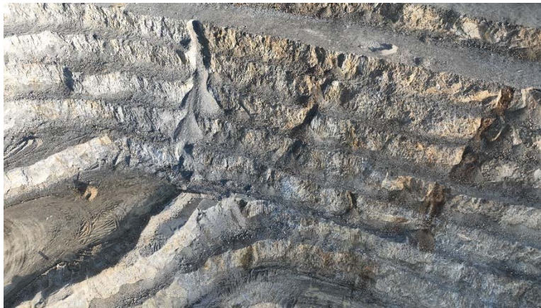
Figure 33: Erosion on Pit Walls
