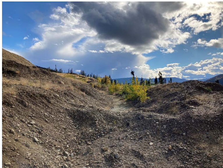
Figure 17: Unconnected Ditch Section 2022
