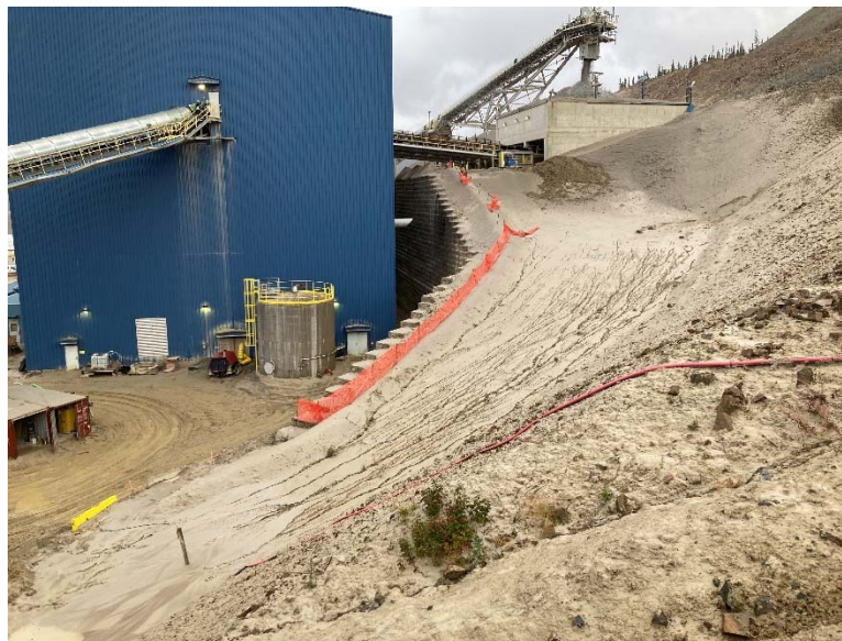
Figure 50: Cut slopes above Secondary/Tertiary Crusher 2022
