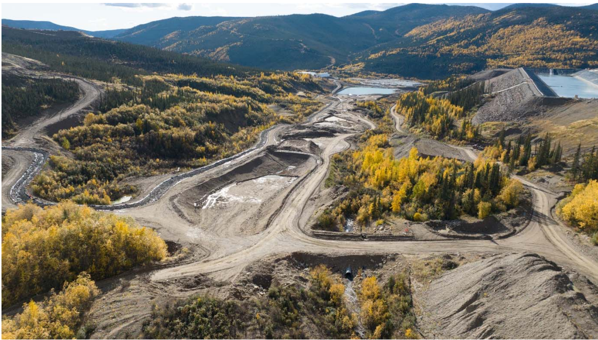
Figure 63: Emergency Pond (Aerial view)
