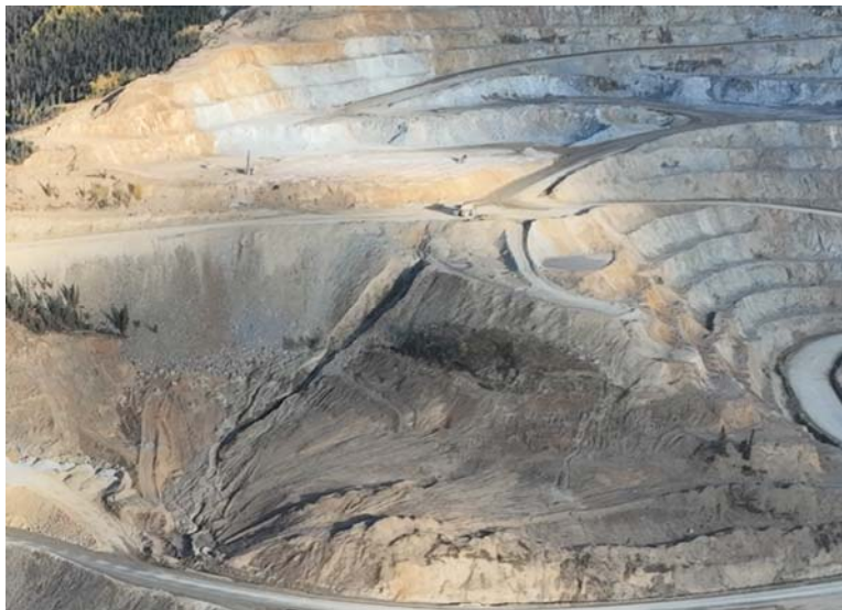
Figure 35: Open Pit Erosion – Aerial View
