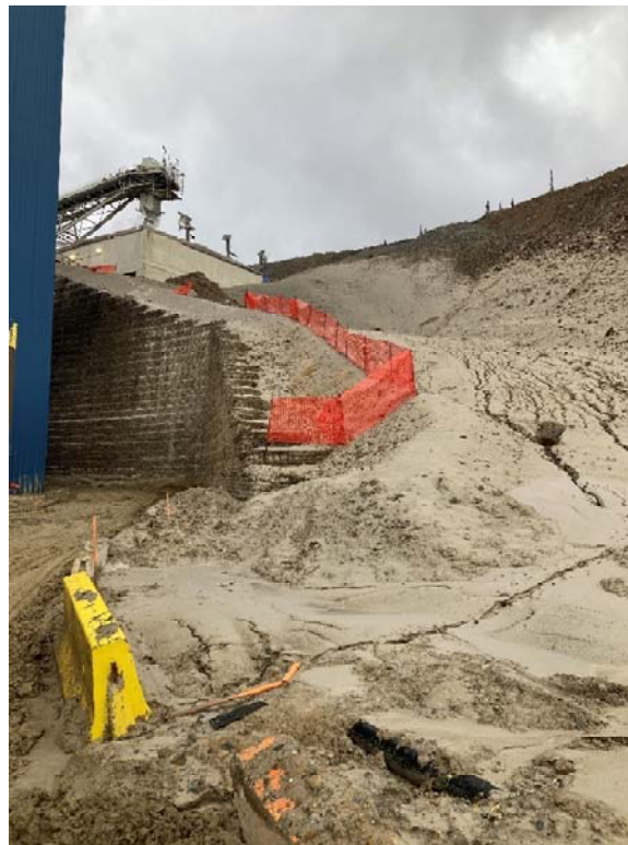
Figure 51: Cut slopes above Secondary/Tertiary Crusher 2022
