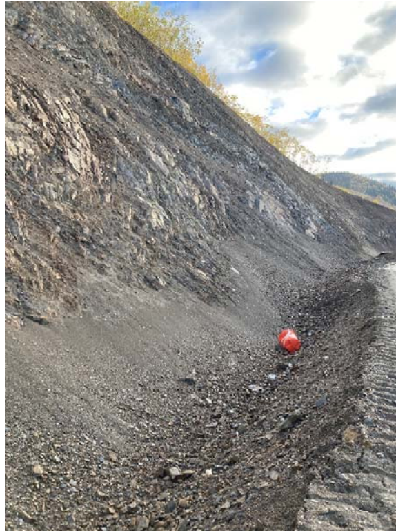
Figure 52: Slopes behind ADR (2022)
