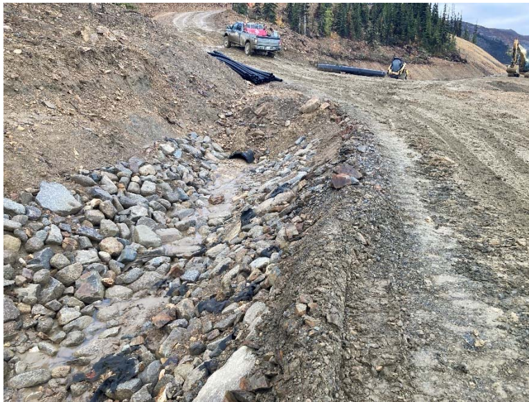
Figure 25: Material deposited in HLF Interception Ditch (2022)
