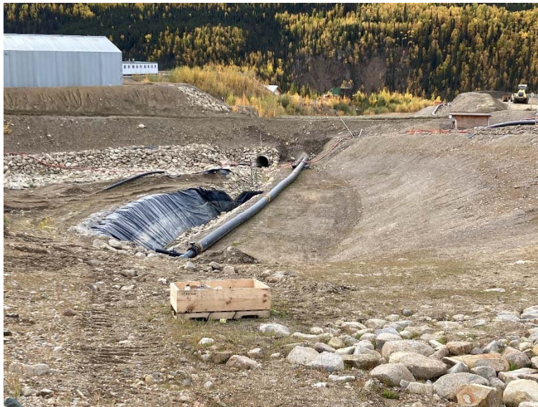
Figure 1: LDSP – Low Level Outlet Conveyance Channel
