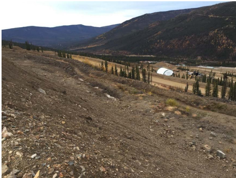
Figure 15: Unconnected Ditch Section 2020
