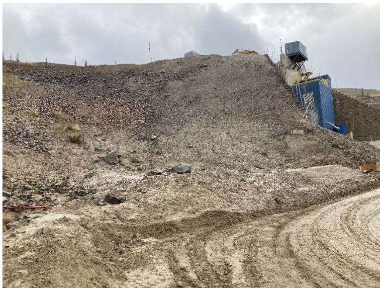
Figure 46: North-West fill slopes
