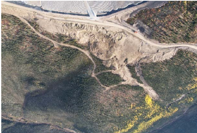
Figure 28: HLF Overburden Stockpile collapse – plan view 2022
