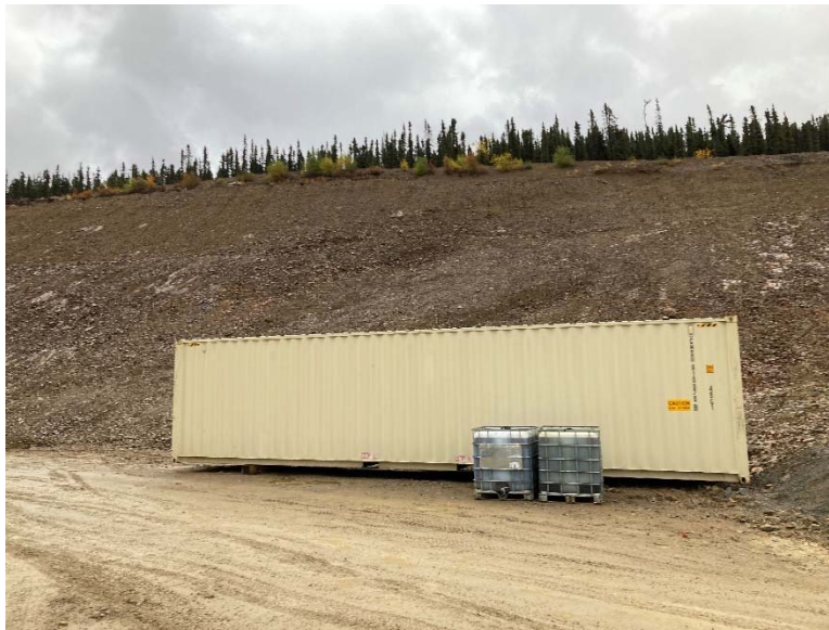
Figure 70: Truck Shop cut slopes
