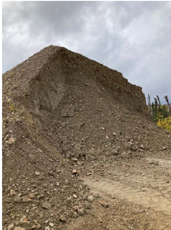
Figure 76: Additional stockpiles with steep side slopes
