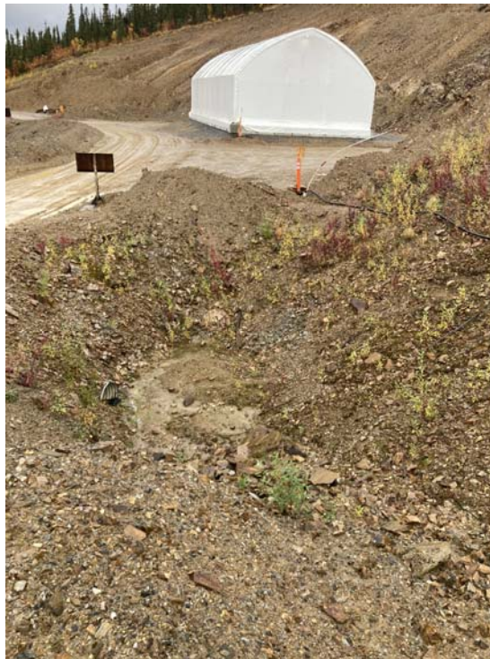
Figure 71: Orica ditch sump & drain culvert
