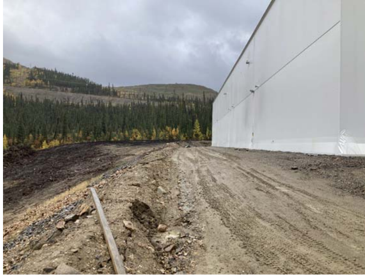
Figure 69: Water Treatment Plant Slopes
