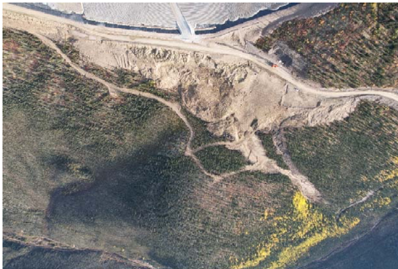
Figure 24: HLF Overburden Stockpile collapse – plan view 2022
