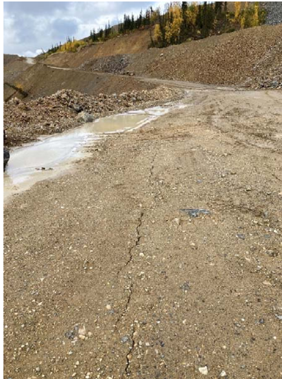
Figure 33: Platinum Gulch Dump Water Pooling (2022)
