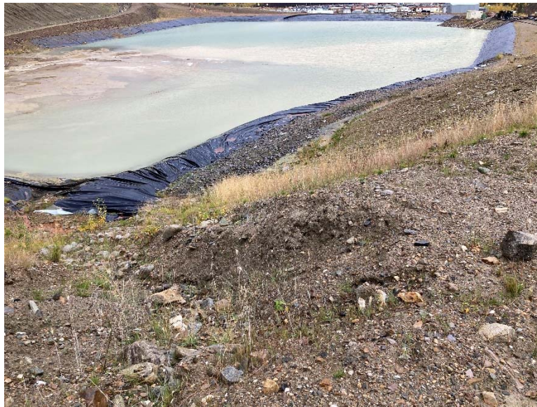
Figure 6: Erosion above the LDSP
