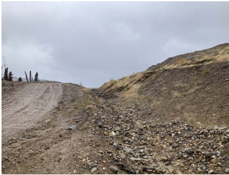
Figure 11: Perimeter Ditching 2023
