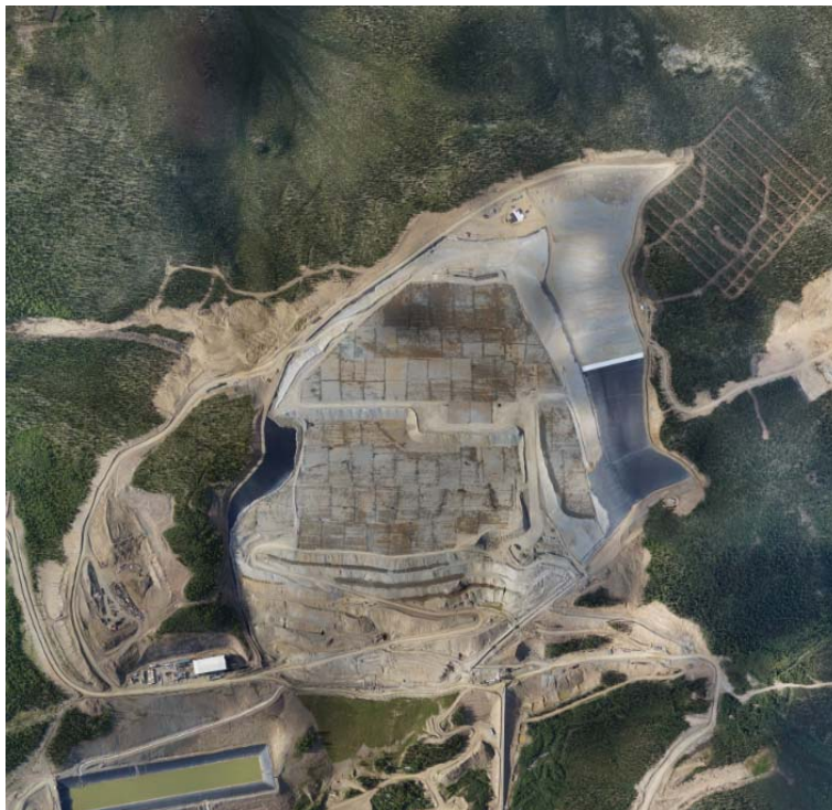
Figure 18: Heap Leach Facility Overview 2023
