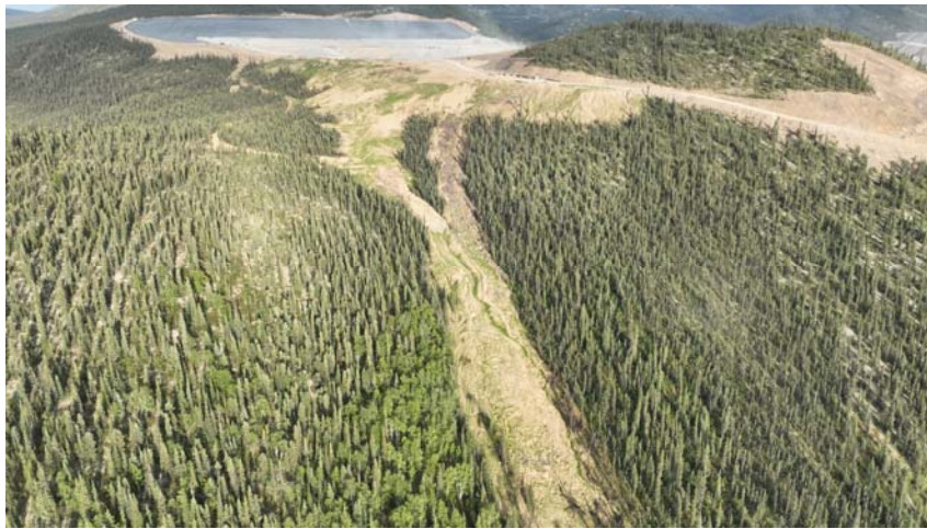
Figure 25: HLF Overburden Stockpile collapse – aerial view 2023
