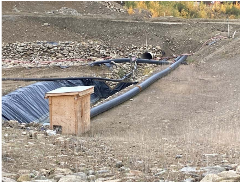
Figure 1: LDSP – Low Level Outlet Conveyance Channel
