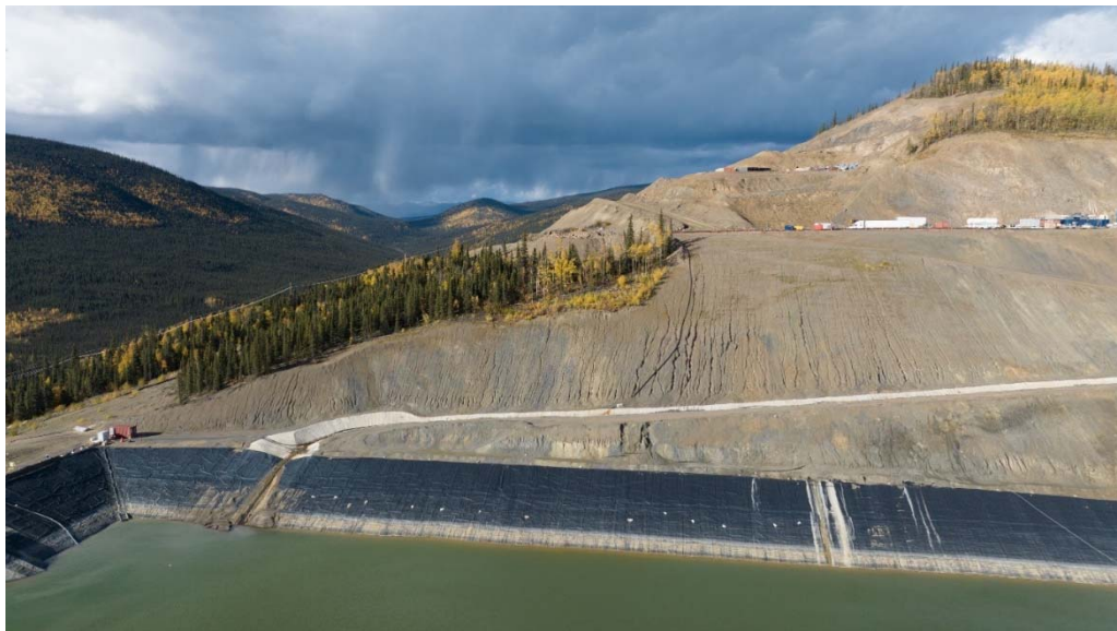
Figure 49: Rill erosion above HLF spillway (2022)
