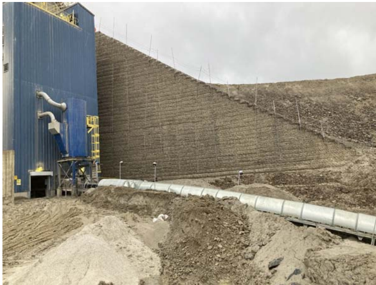
Figure 40: Primary Crusher South-East Wall
