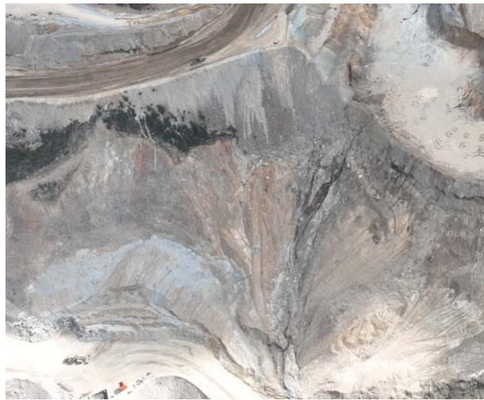
Figure 30: Open Pit Erosion – Aerial View 2023
