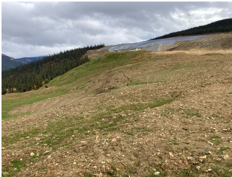
Figure 26: HLF Overburden Stockpile collapse – slope cracking 2023
