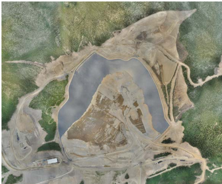
Figure 16: Heap Leach Facility Overview 2021
