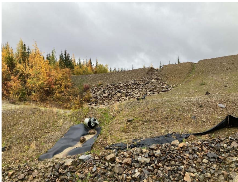
Figure 5: LDSP – Some flow from adjacent culvert 2023
