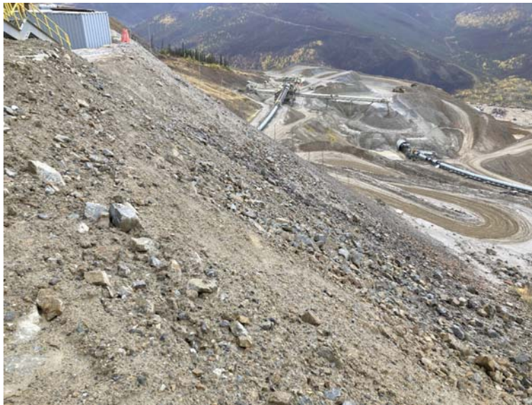
Figure 41: North-West fill slopes
