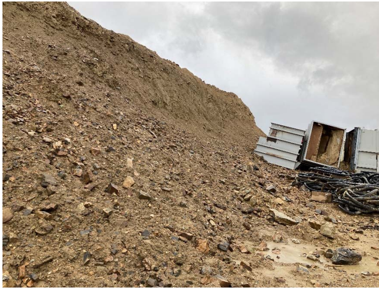
Figure 8: Secondary Stockpile Cut Slopes 2022
