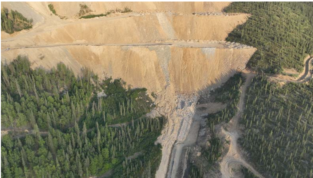
Figure 32: Platinum Gulch Dump (Aerial View)
