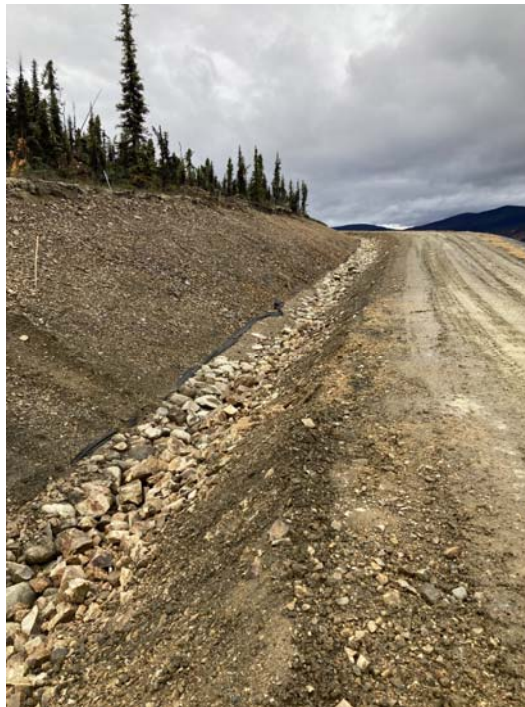
Figure 22: HLF Interception Ditch (2023)
