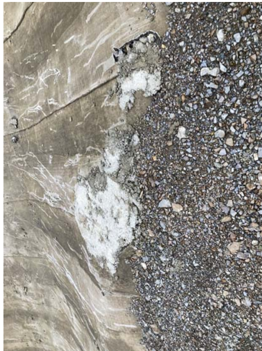
Figure 56: Heap leach spillway repairs (2023)
