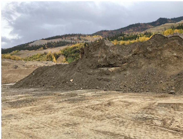
Figure 75: Some stockpiles with steep side slopes
