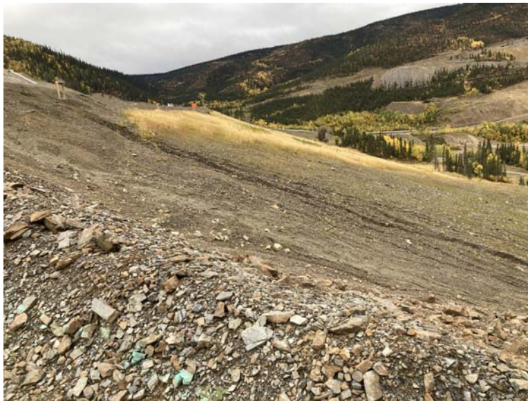
Figure 21: Seeded grass on toe slope of HLF (2023)
