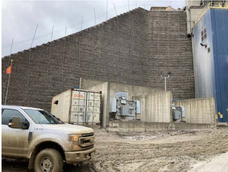
Figure 39: Primary Crusher North-West Wall
