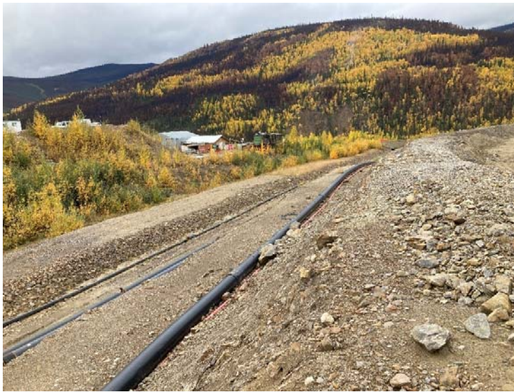
Figure 64: Ditch C with WTP Pipeline
