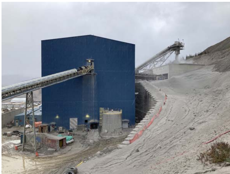
Figure 42: South side of MSE wall
