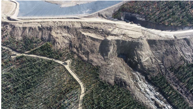
Figure 23: HLF Overburden Stockpile collapse – plan view 2021
