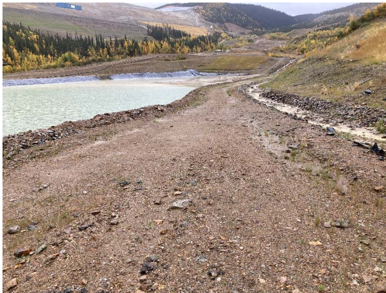
Figure 3: LDSP – Cracking on the Southwest slope 2023
