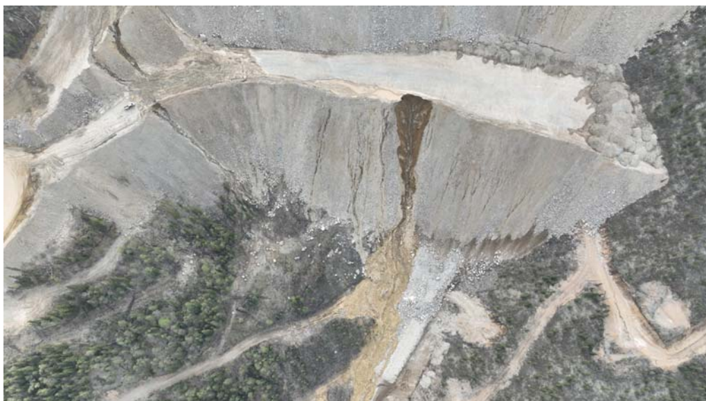
Figure 35: Platinum Gulch Dump Erosion Event (Spring 2023)
