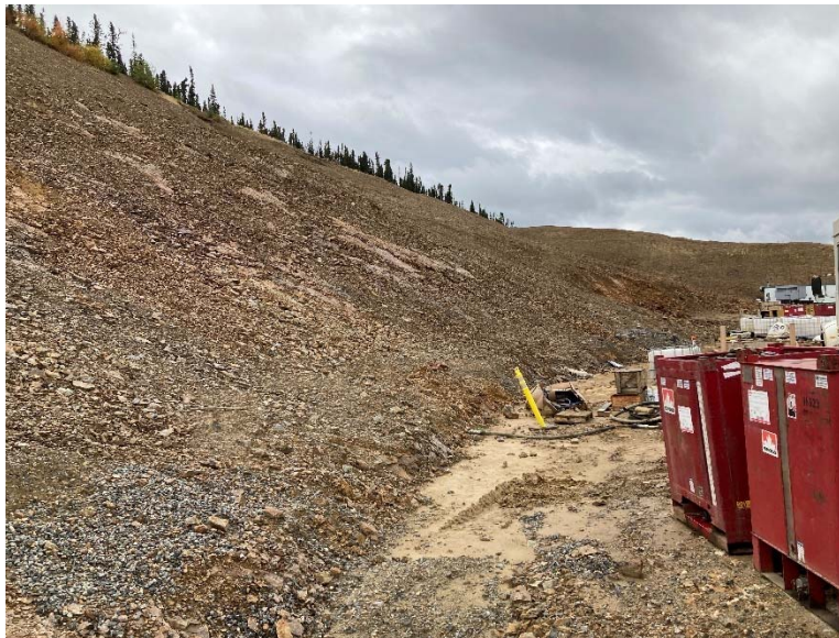
Figure 65: Truck Shop cut slopes
