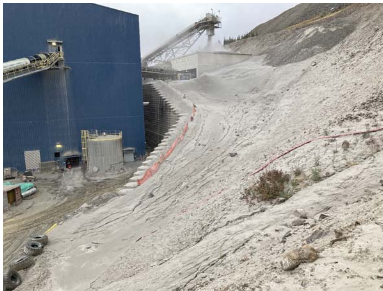
Figure 45: Cut slopes above Secondary/Tertiary Crusher 2023
