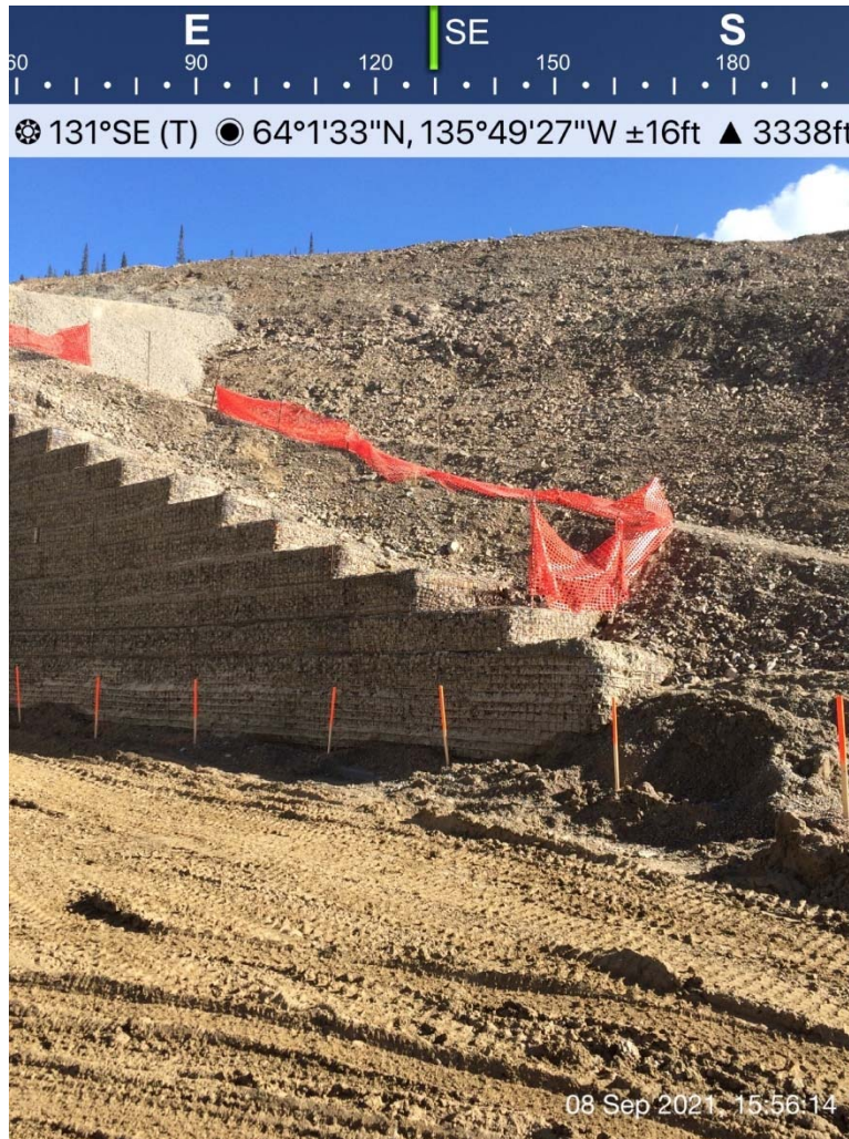
Figure 43: Cut slopes above Secondary/Tertiary Crusher 2021
