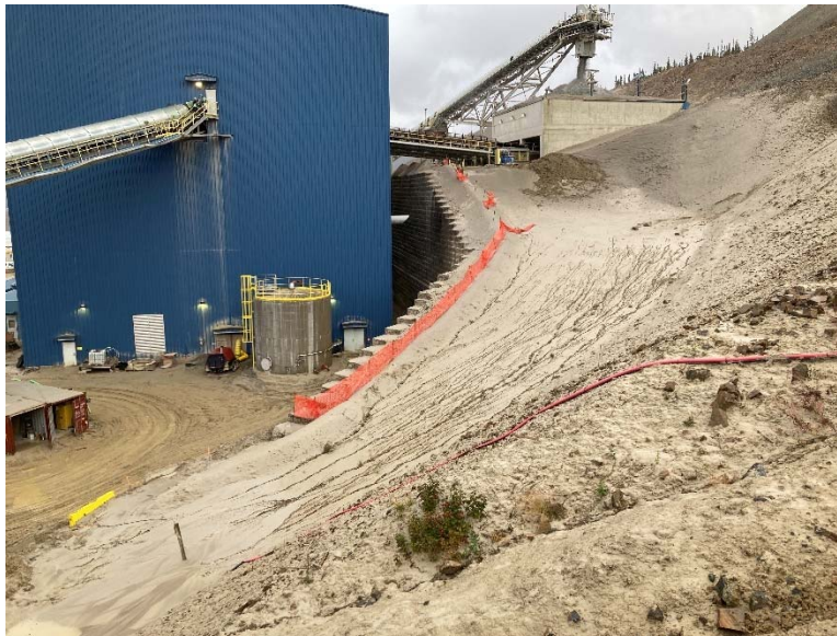
Figure 44: Cut slopes above Secondary/Tertiary Crusher 2022
