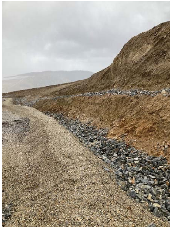
Figure 9: Secondary Stockpile Cut Slopes 2023
