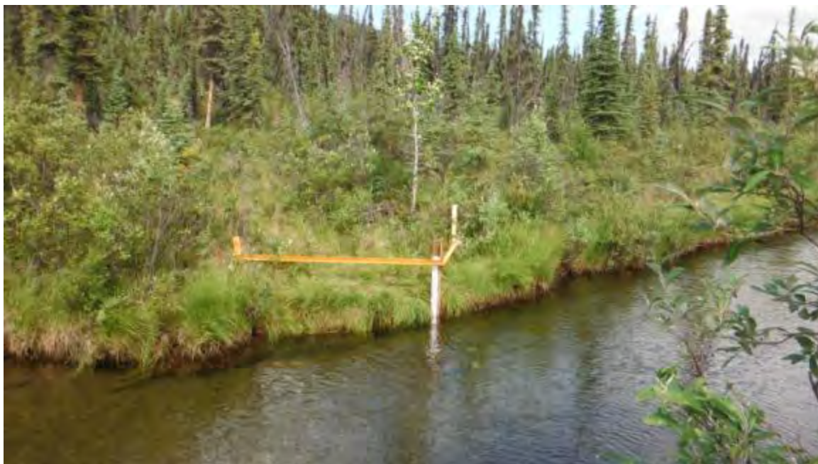
Figure 5 - W-22 after repairs, August 4 2013
