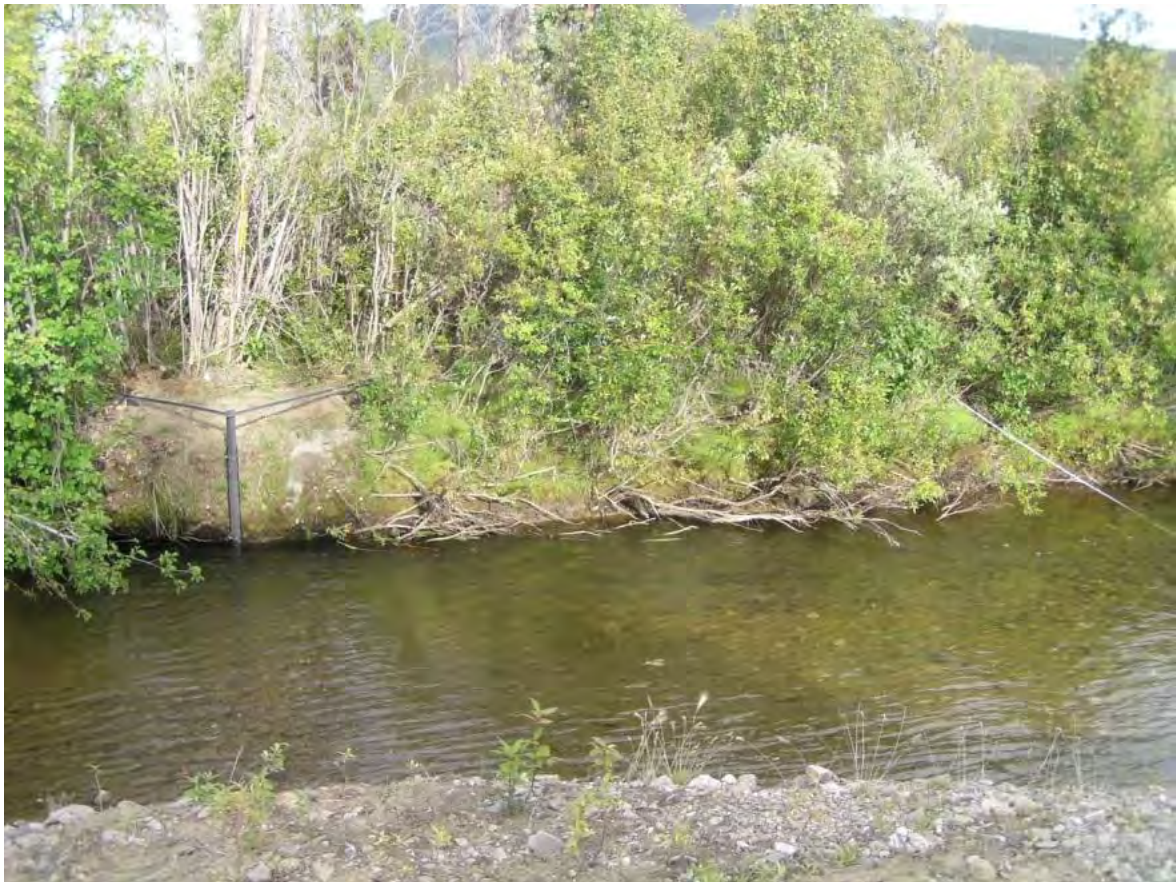
Figure 10 – W-5 during construction August 2007
