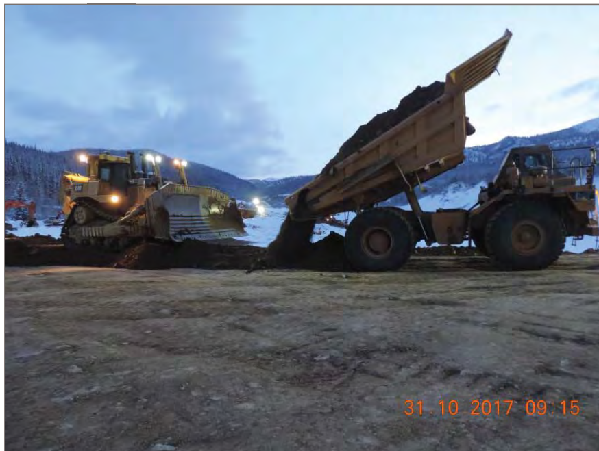
Photo 2: Cat D10T Dozer receives subgrade fill material from Cat 773 Rock Truck
