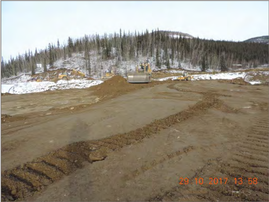
Photo 4: Dozer spreading second lift of sub grade
