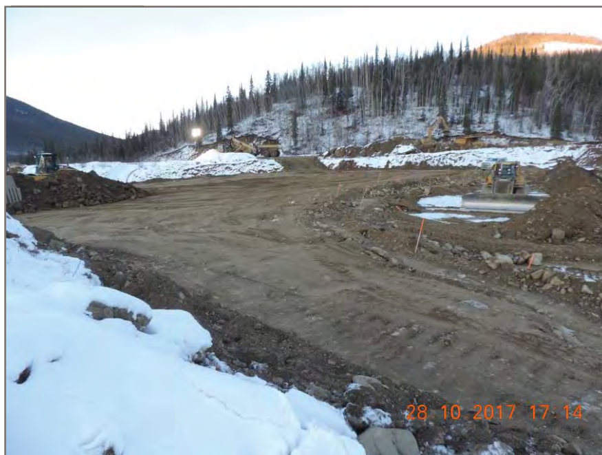
Photo 6: Progress from day shift on Dam. Elevation: 809.3
