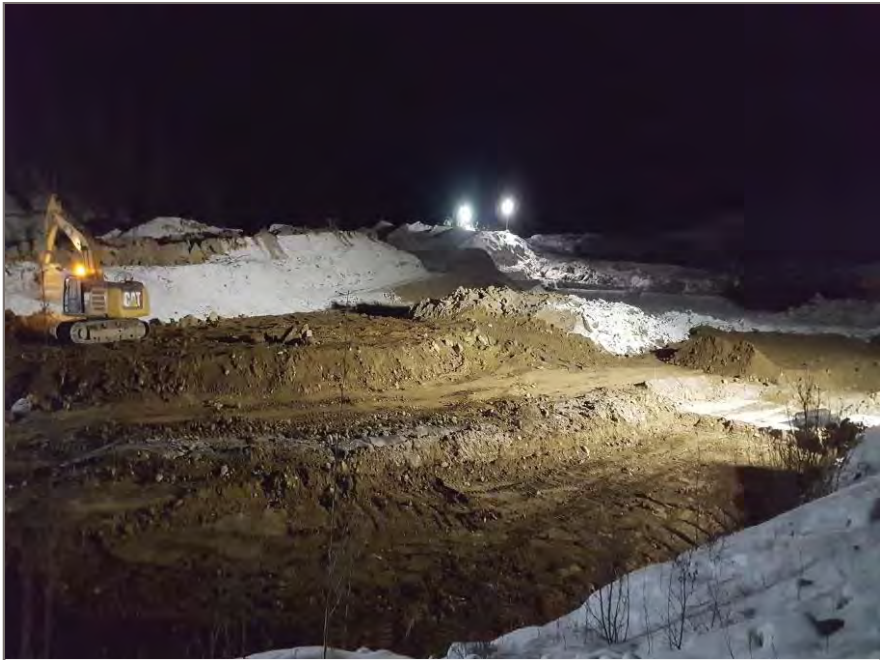
Photo 3: Excess material located north of excavation being cut to 808.00m
