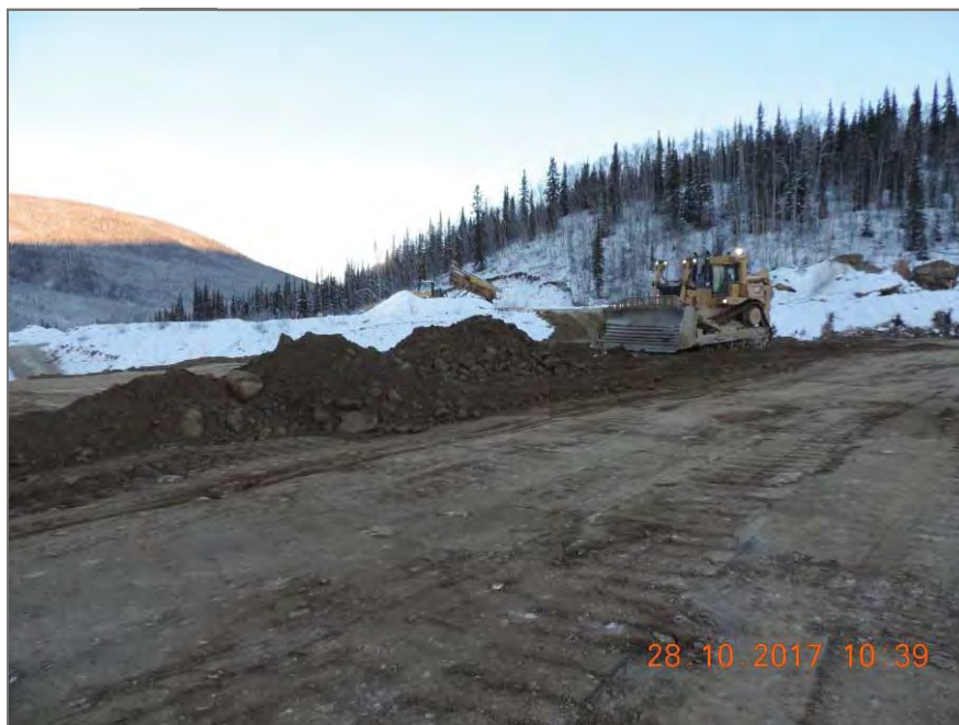
Photo 2: Cat D10T dozer spreads sub grade material on floor of Dam
