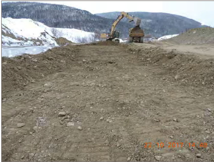
Photo 3: Unsuitable sub grade fill material excavated out
