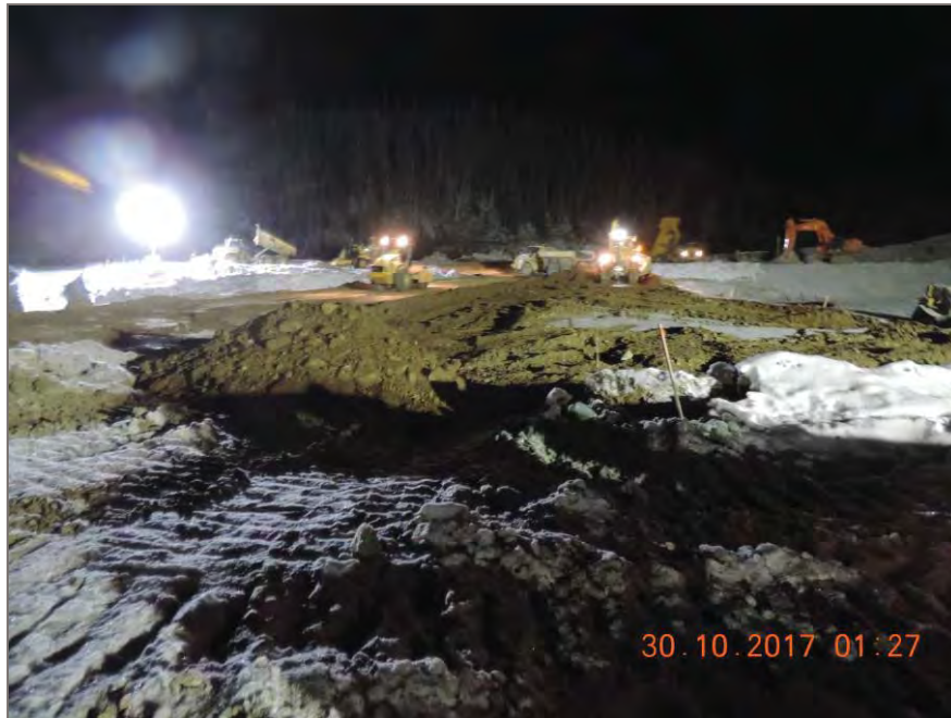
Photo 1: Stripping of insufficient lift material on East side of dam.
