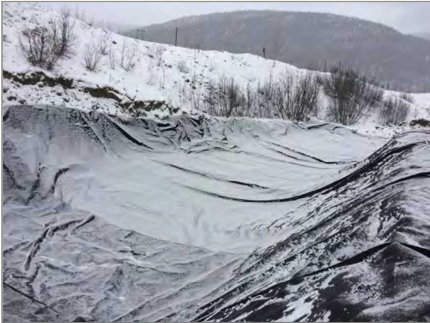
Photo 3: View from north embankment looking southwest at geotextile placed throughout sub-excavation.
