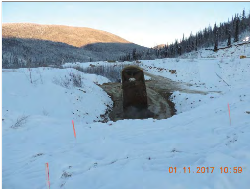
Photo 4: First load of subgrade on foundation for Spill Way construction
