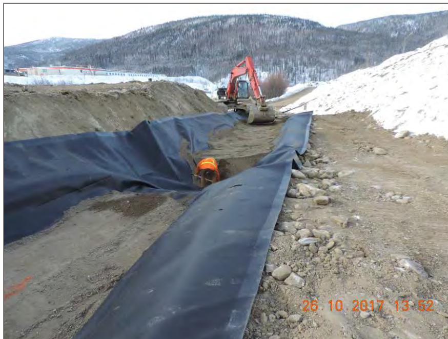
Photo 2: Bedding Sand placed onto liner
