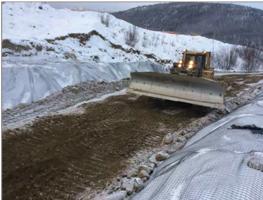
Photo 4: Scarifying lift to ensure adequate bond to next lift in-pogress.
