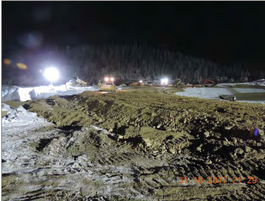
Photo 1: Compaction pit run using a smooth drum packer at grade 812.5m.
