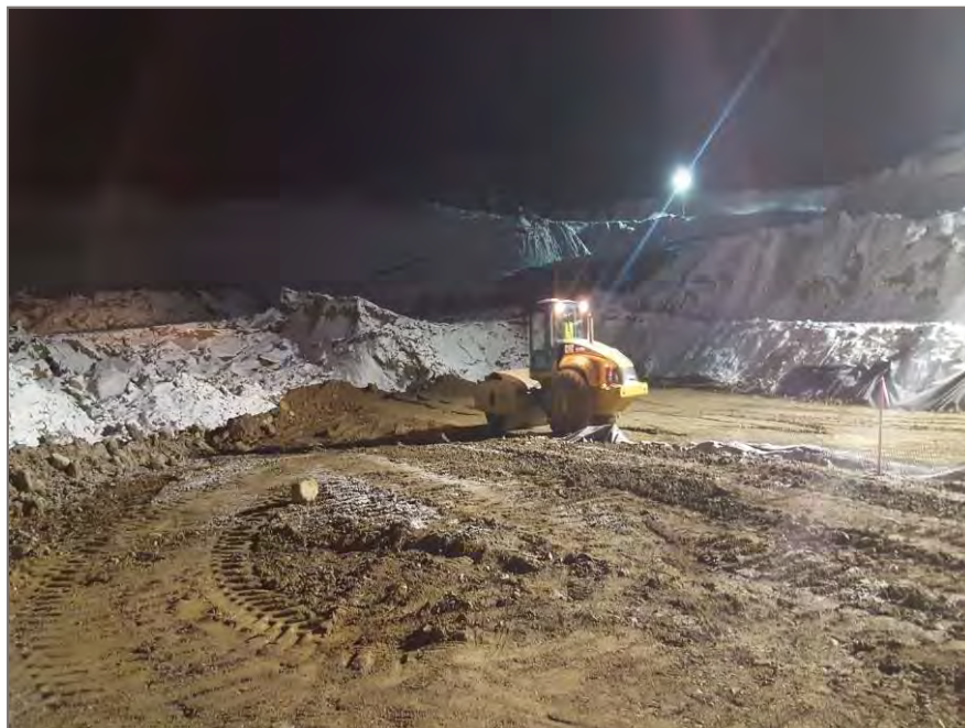
Photo 2: Compaction of bridge lift east side of excavation.
