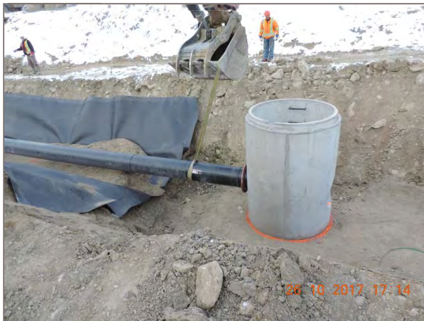
Photo 6: Placing Pipe Invert into center of Man Hole
