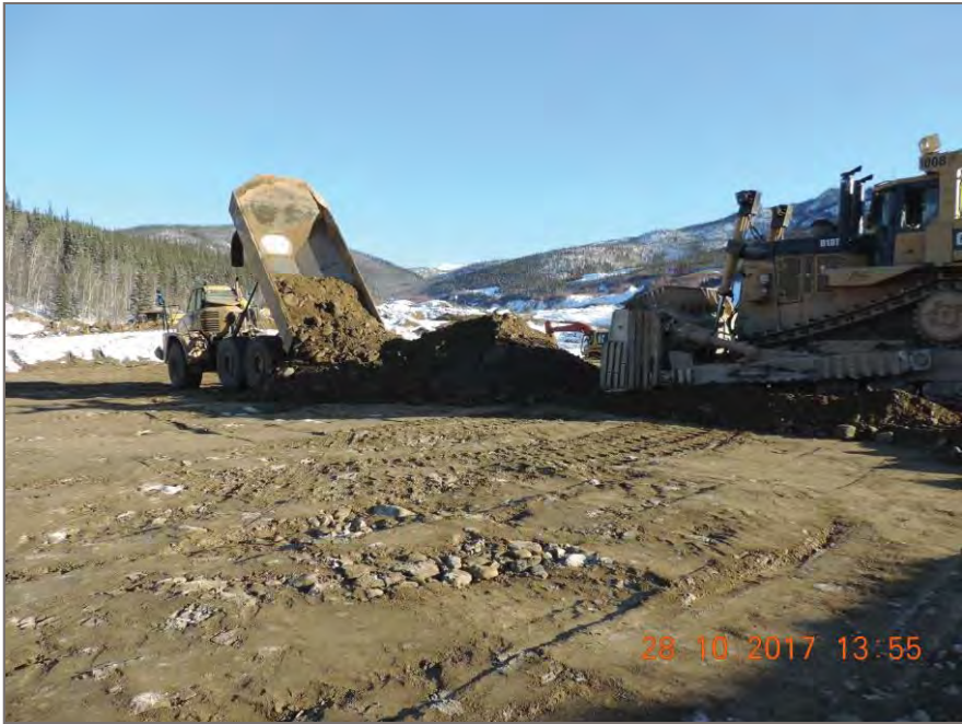
Photo 3: Rock truck placing fill on Dam, first lift on day shift
