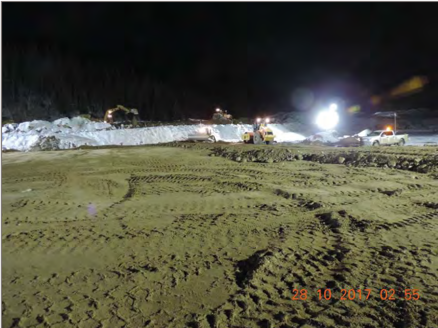
Photo 3: Compaction of pit run on second lift at 809.0 m grade.
