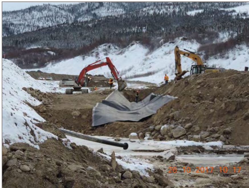
Photo 1: Liner installed to LLO Trench
