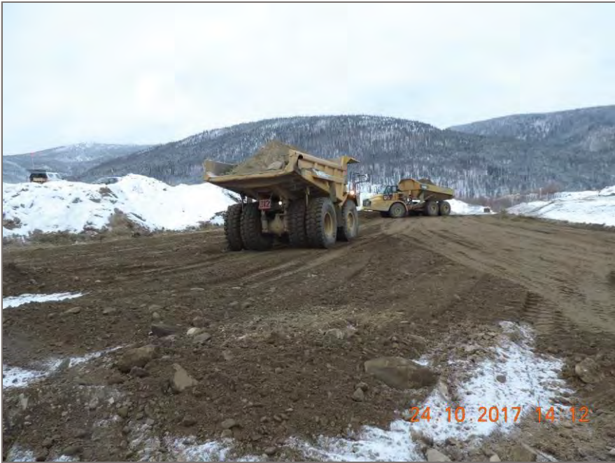
Photo 3: Cat 773D Rock Truck used for compaction of bridge lifts
