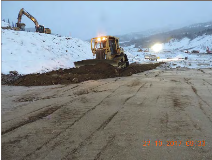
Photo 1: Backfilling sub grade material in LLO Pipe area after Pipe install
