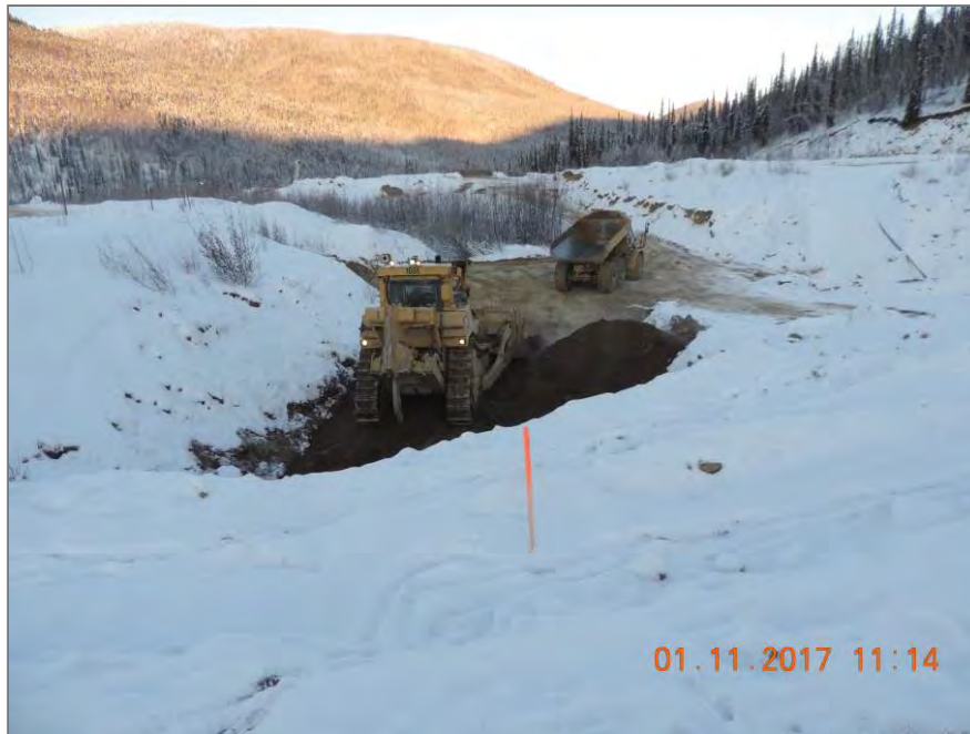
Photo 5: Cat D10T Dozer spreading fill on Spill Way
