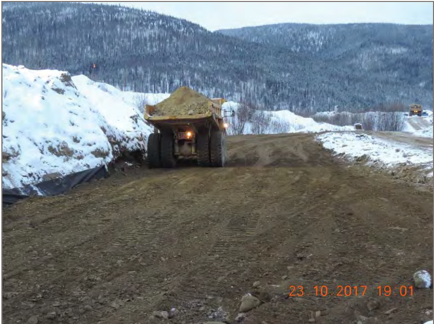
Photo 7: Packing second lift with Cat 773 rock Truck
