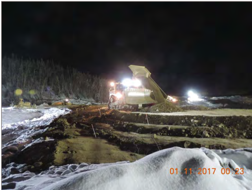
Photo 2: Placement of pit run material at grade 812.8m.
