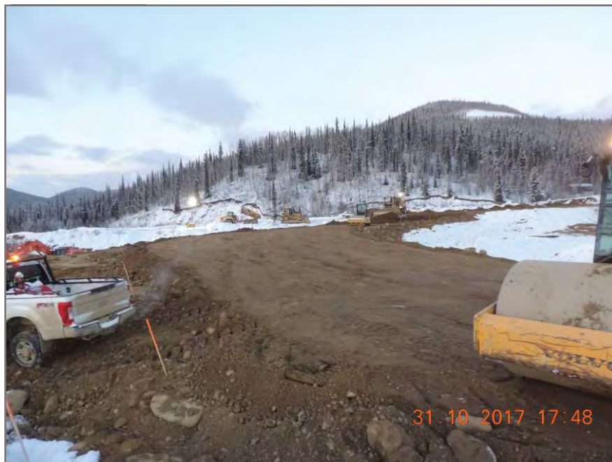
Photo 6: Progress from day shift on Dam fill complete at Elevation: 812.2
