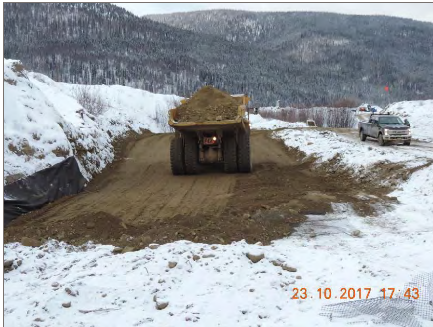
Photo 5: Cat 773 Rock Truck used for compaction
