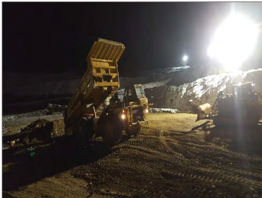
Photo 4: Placement of suitable pitrun within berm.
