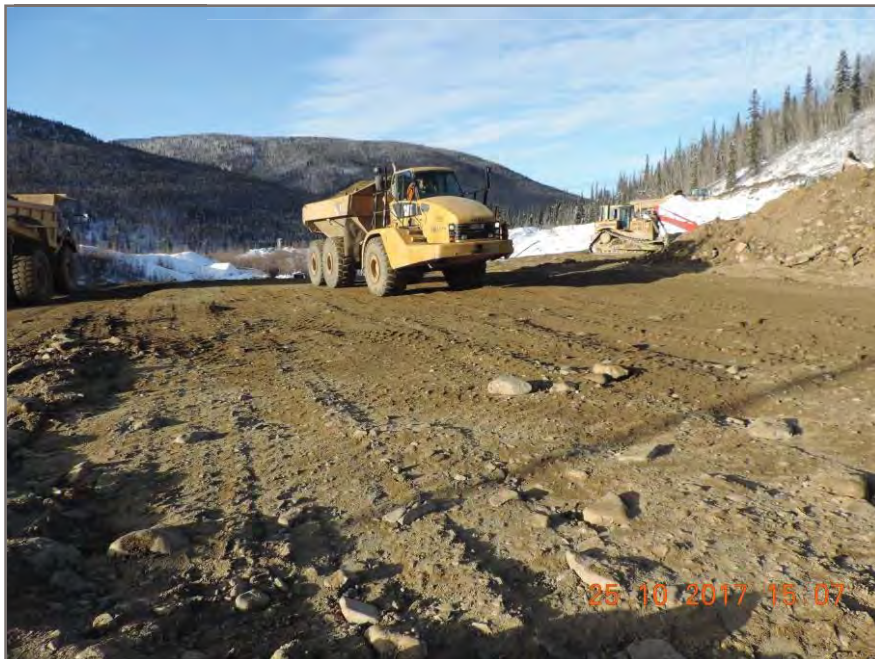
Photo 6: Packing with Cats 740B and 773 Rock Trucks on grade
