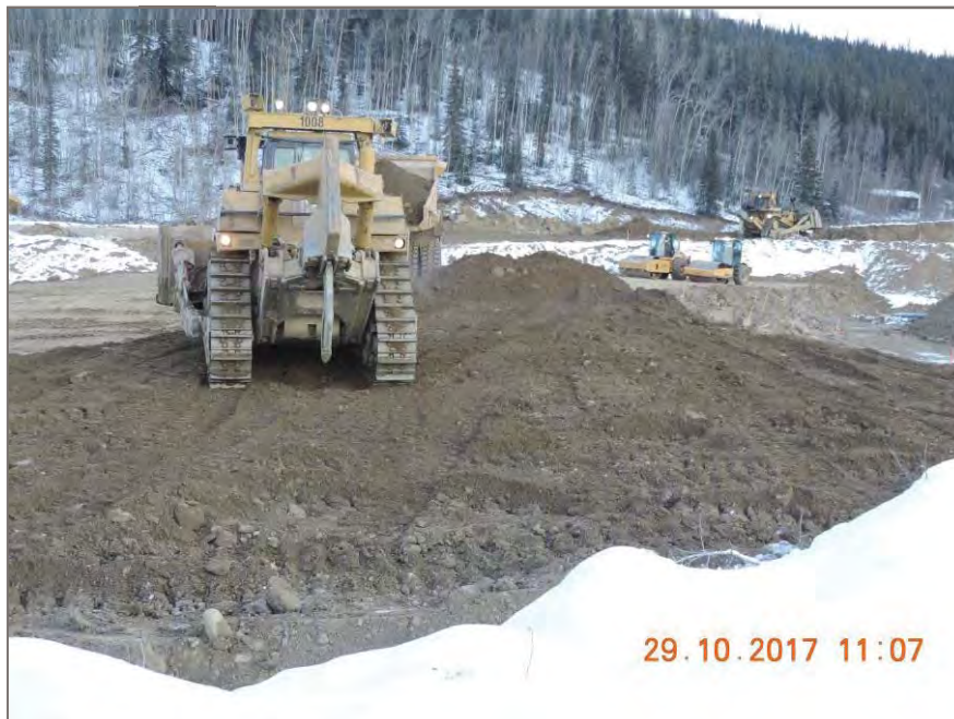
Photo 2: Cat D10T Dozer spreads sub grade fill material
