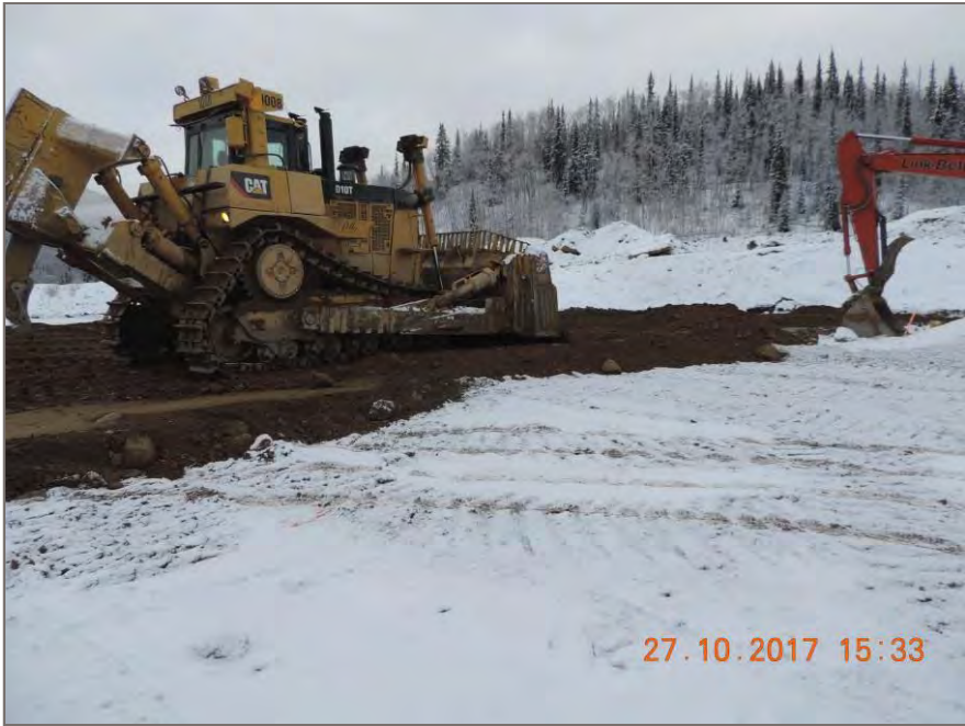
Photo 3: Cat D10T Dozer spreading backfill
