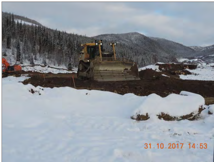
Photo 5: Dozer back blading smooth fill lift for even compaction with packers
