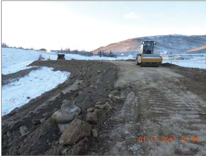
Photo 3: 1-Single Smooth Drum packer works subgrade material on final lift Elevation: 813.5
