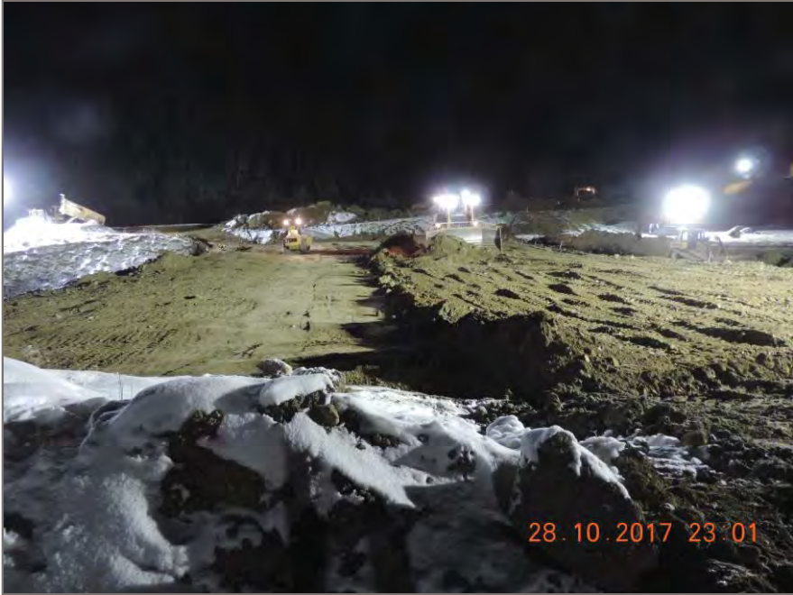
Photo 3: Compaction of pit run on second lift at 809.9 m grade.
