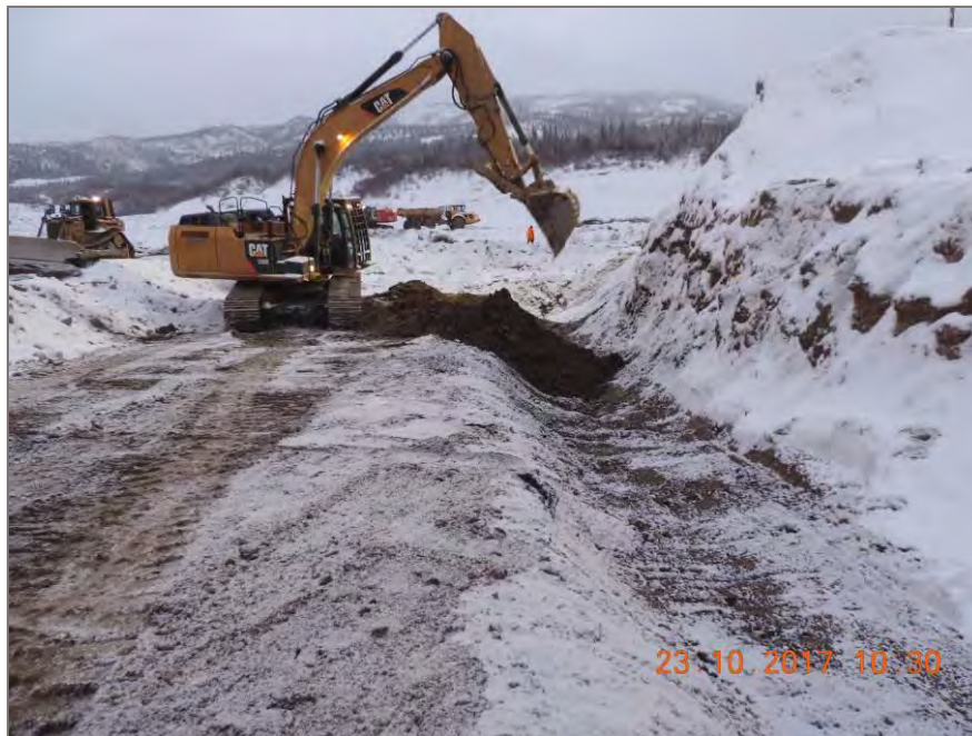
Photo 1: Excavator removes over saturated unsuitable berm material
