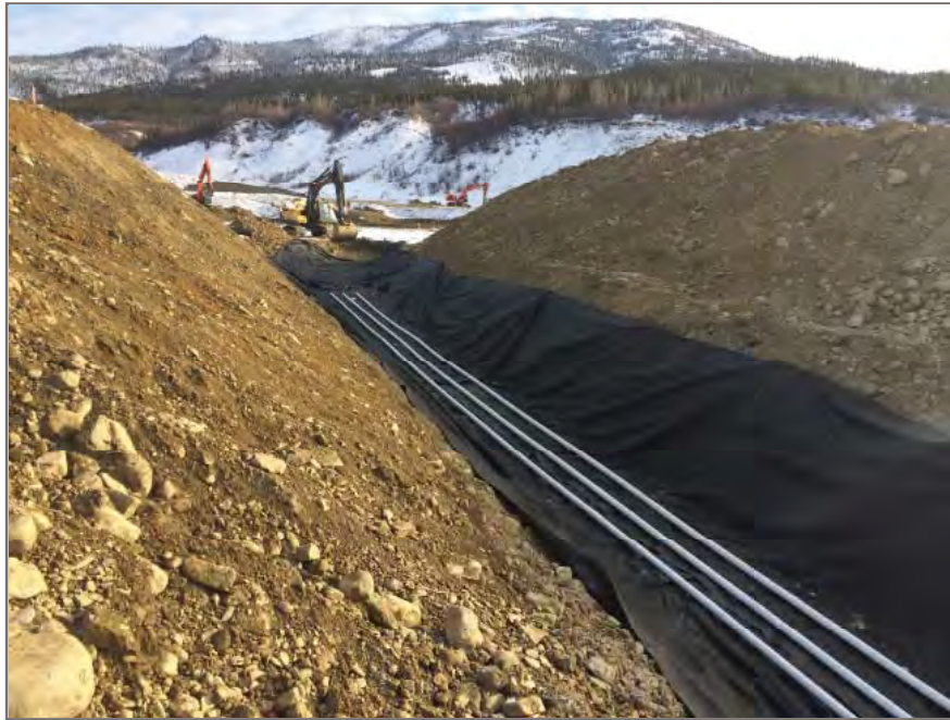
Photo 3: Continued installation of perforated pipe for underdrain.
