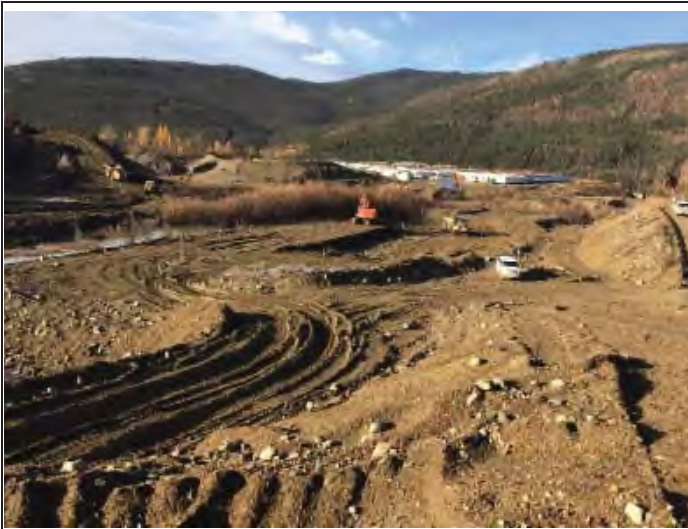
Photo 1 Excavation along west dam
