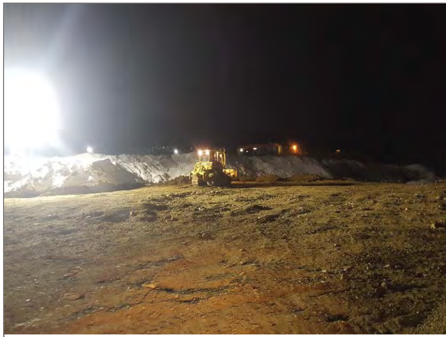
Photo 1: Placement of pit run within dam footprint
