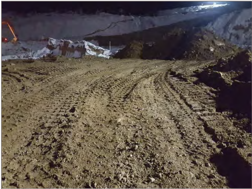
Photo 4: CAT 740 tracking placed material
