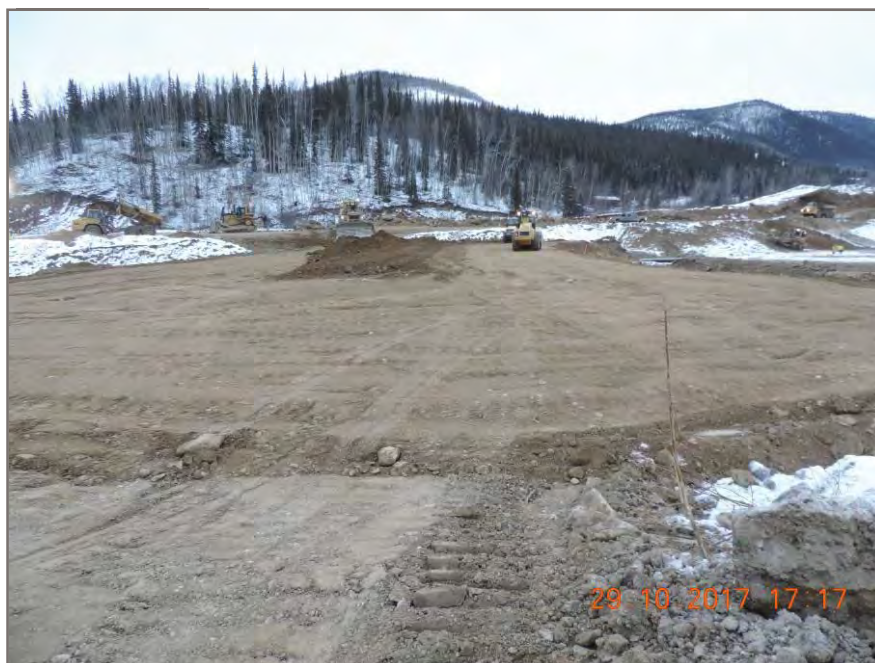
Photo 6: Progress from day shift on Dam fill complete at Elevation: 810.4
