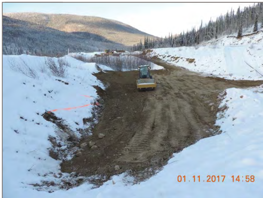
Photo 6: Packer working fill on Spill Way
