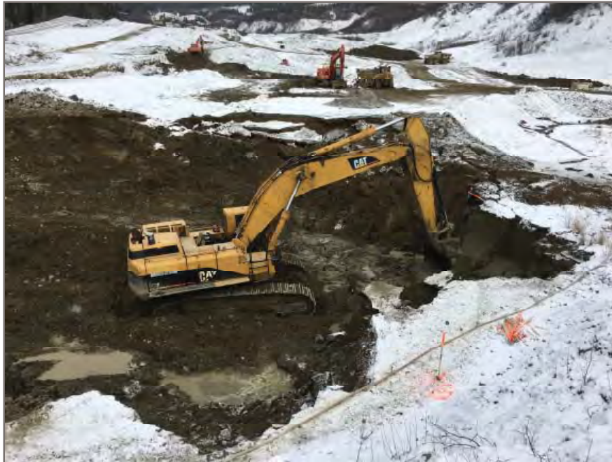
Photo 3: View of sub-excavation within southwest area of embankment.
