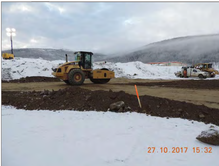
Photo 2: Single smooth drum packing sub grade fill
