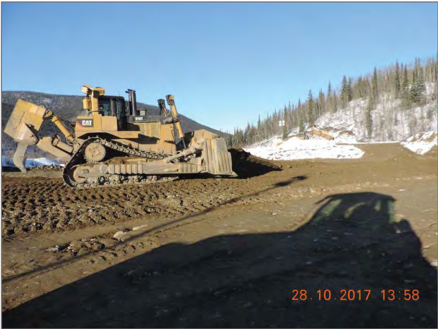
Photo 4: Spreading second lift of sub grade
