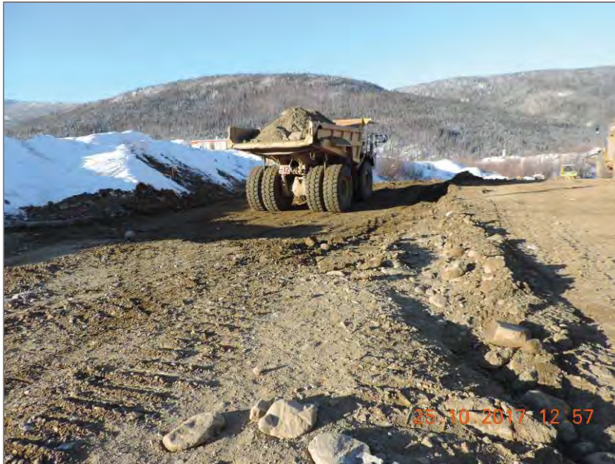
Photo 5: Packing replacement lift after excavation.
