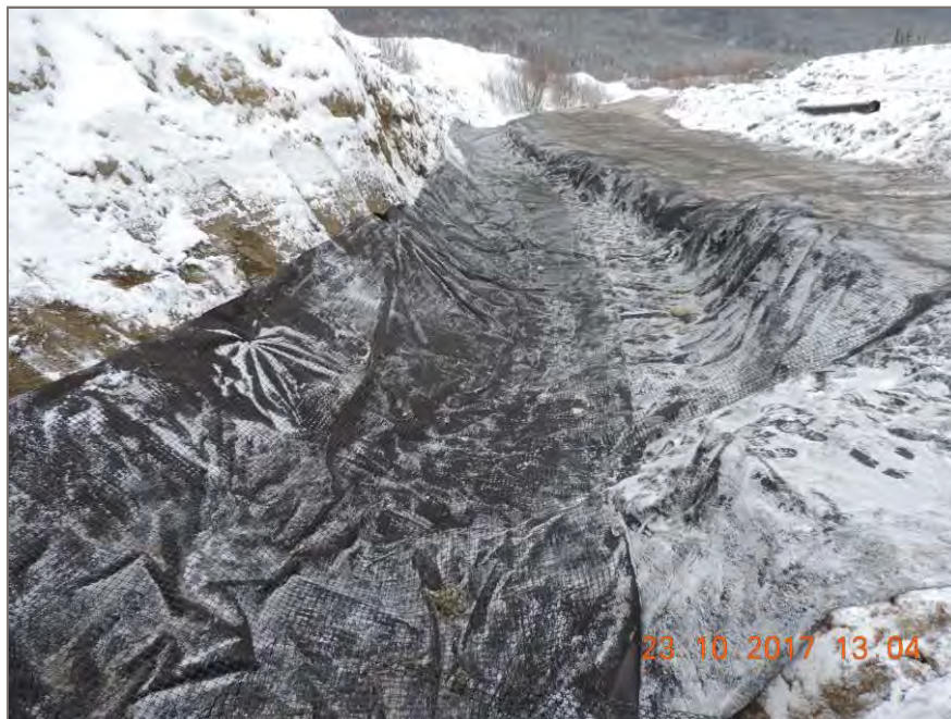
Photo 2: Filter Fabric with Geogrid laid on bottom of berm
