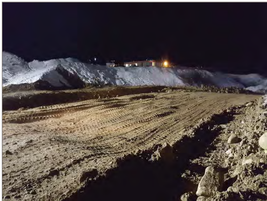
Photo 2: Unstable material removed
