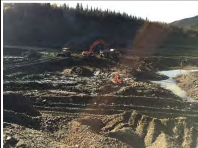
Photo 3 Excavation of spoils in forebay area
