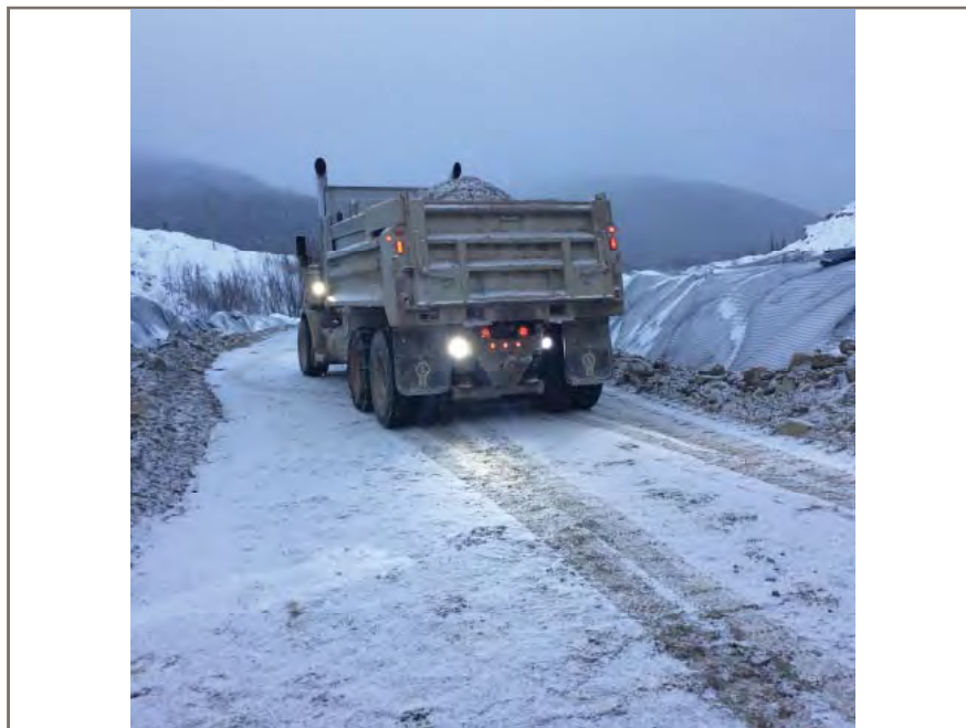
Photo 2: Proof-roll of bridge lift in-progress.
