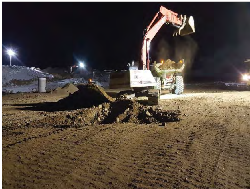
Photo 2: Removal of unstable material within berm
