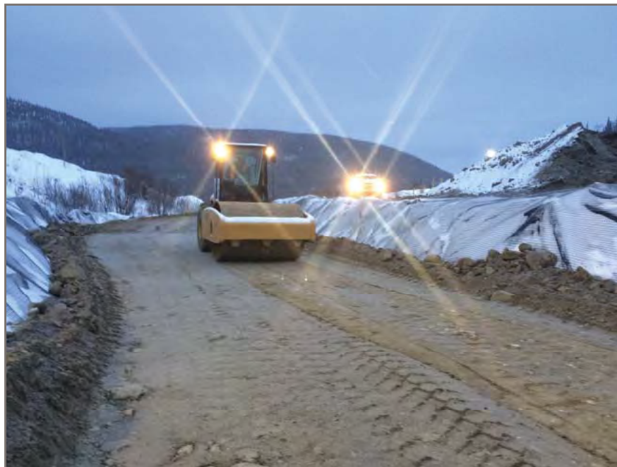
Photo 1: Compaction of bridge lift in progress.
