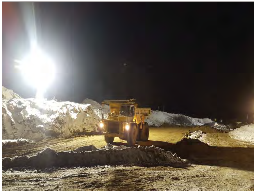
Photo 1: Loaded CAT 773D used for compaction
