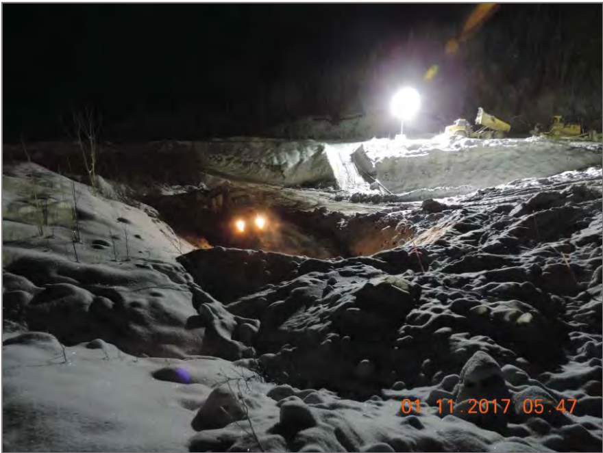
Photo 4: Initial placement of backfill at base of spill way.
