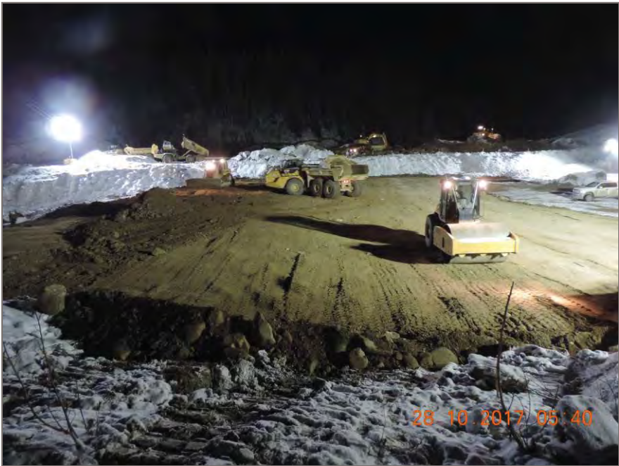
Photo 4: Placement and compaction of pit run.
