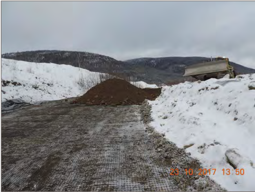
Photo 3: Geogrid placed on prior lift for support
