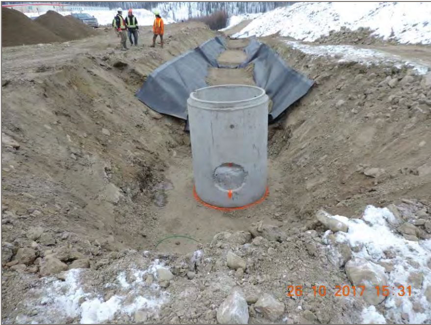
Photo 3: Man Hole installed into place
