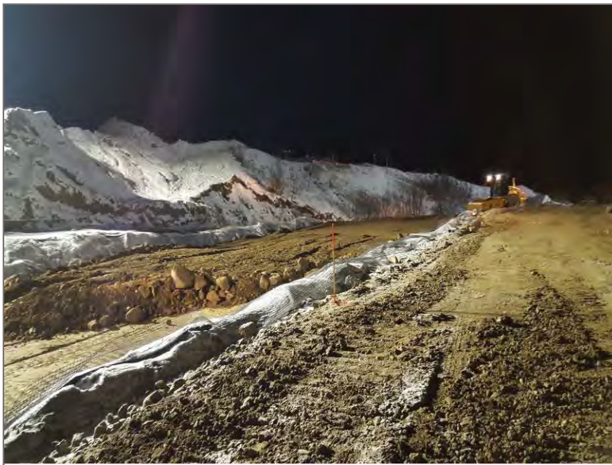
Photo 4: Placement and compaction of pitrun within excavation
