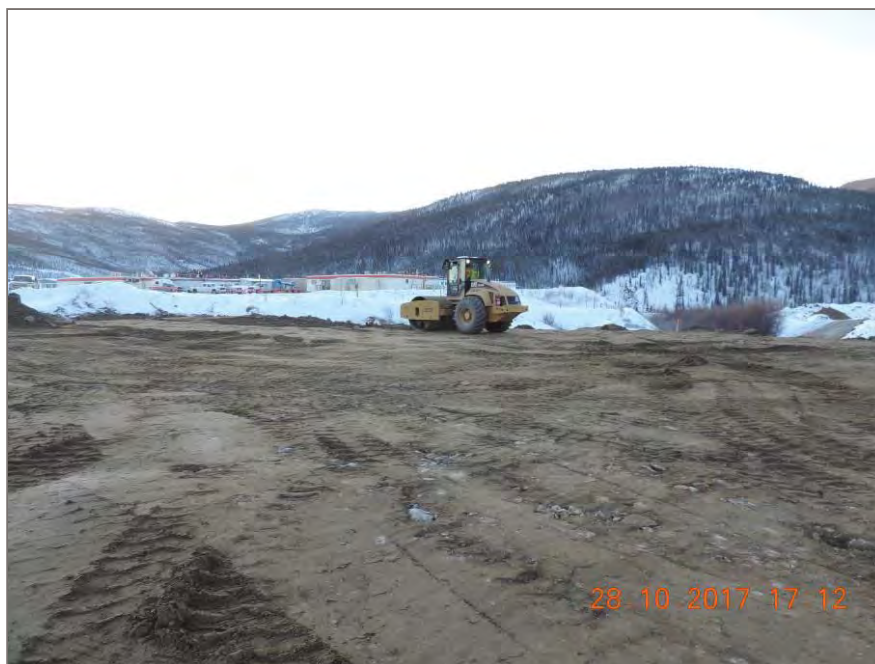
Photo 5: Single smooth drum packer working on second lift
