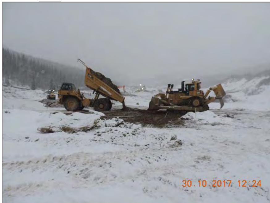
Photo 2: Cat D10T Dozer spreads subgrade fill material from Cat 773 Rock Truck
