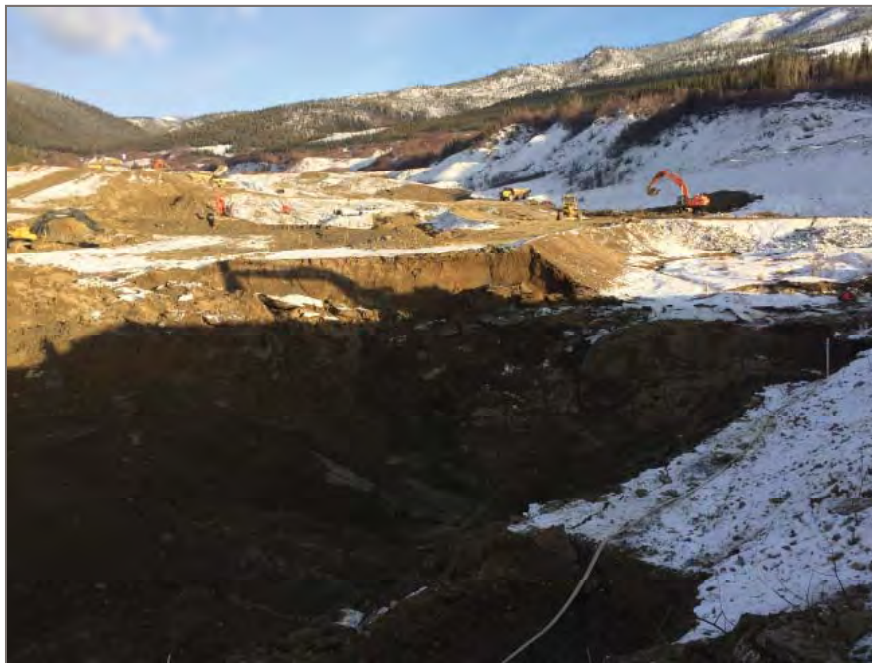
Photo 4: Continued sub-excavation within south end of control pond embankment area.
