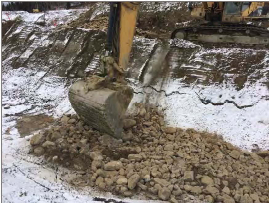
Photo 2: Attempting to push the rock into the subgrade with the cutting edge of the bucket.
