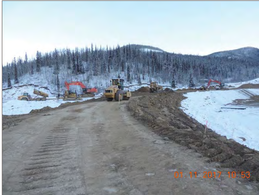
Photo 1: Pelly continues backfill of South Dam of Lower Dublin Control Pond
