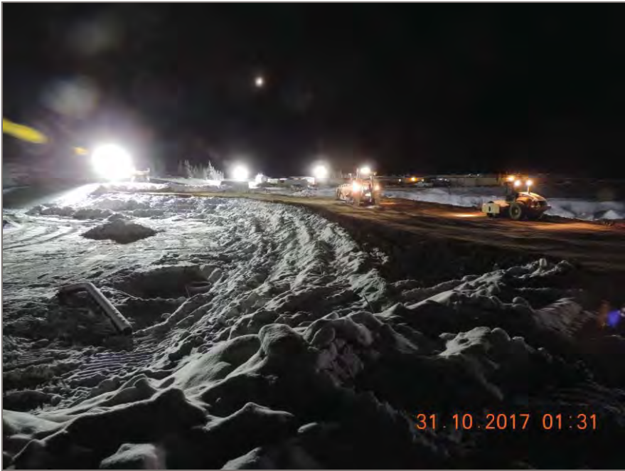
Photo 3: Extent of dam backfill at grade 811.3m, East side.
