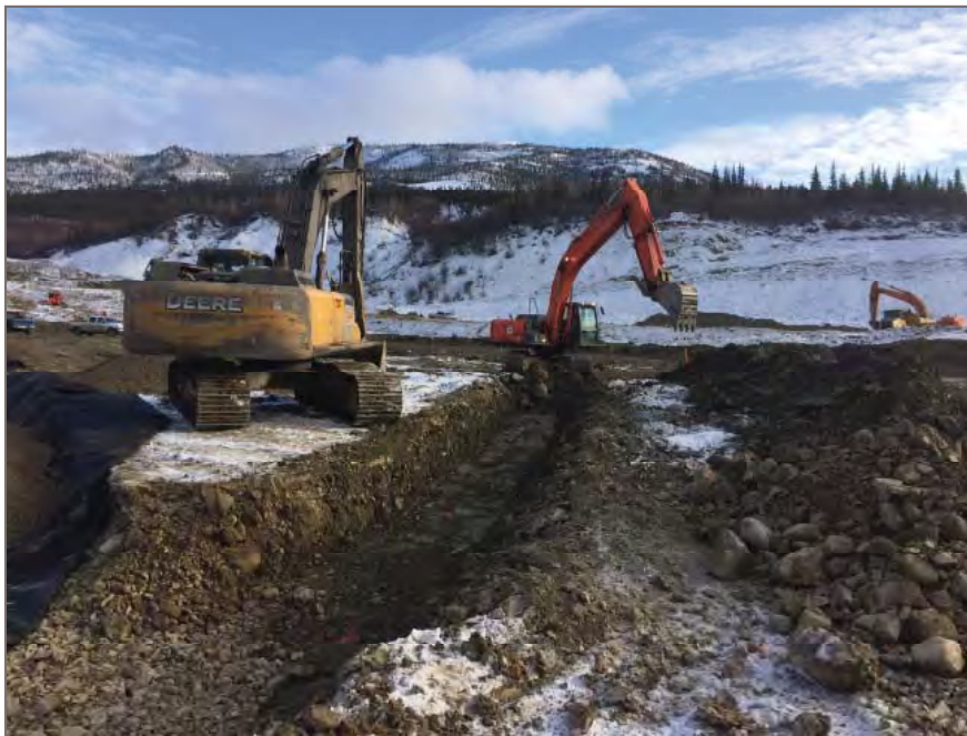
Photo 4: Excavation of underdrain
