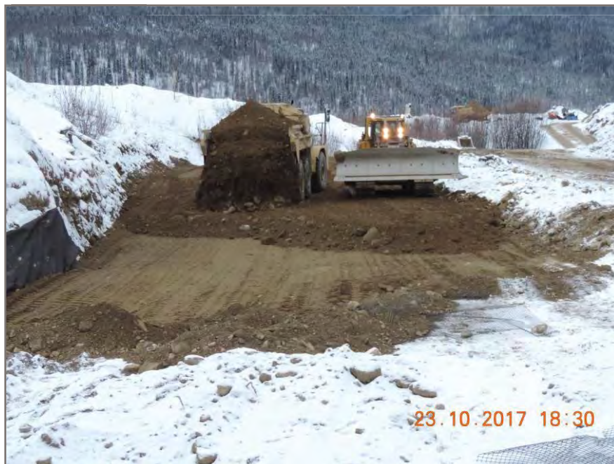
Photo 6: Second lift placed and spread
