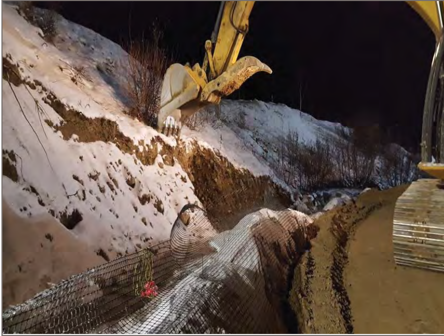
Photo 3: Removal of sluffed and frozen material in south west bank
