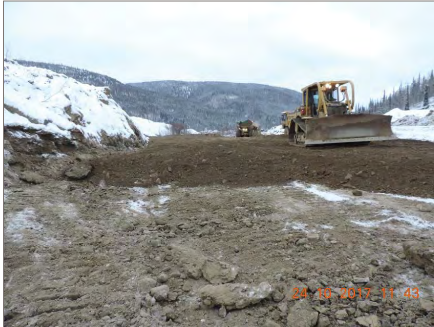
Photo 1: 400-500mm bridge lift spread
