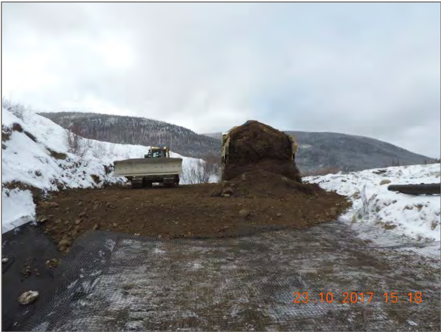
Photo 4: Suitable backfill material placed on Geogrid
