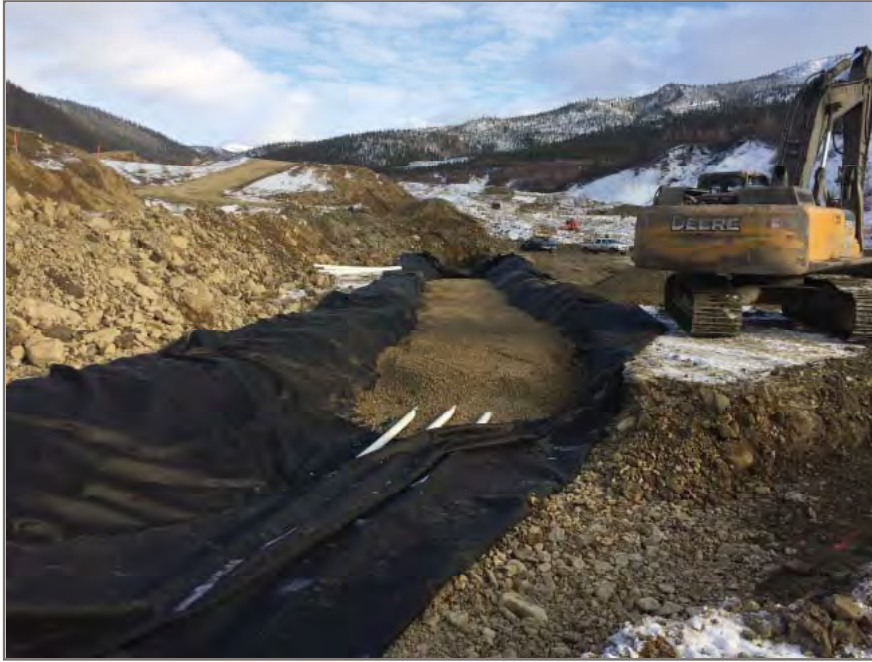
Photo 3: Continued installation of perforated pipe for underdrain.
