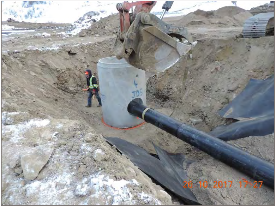
Photo 7: HDPE Pipe install complete and ready for Grout and backfill
