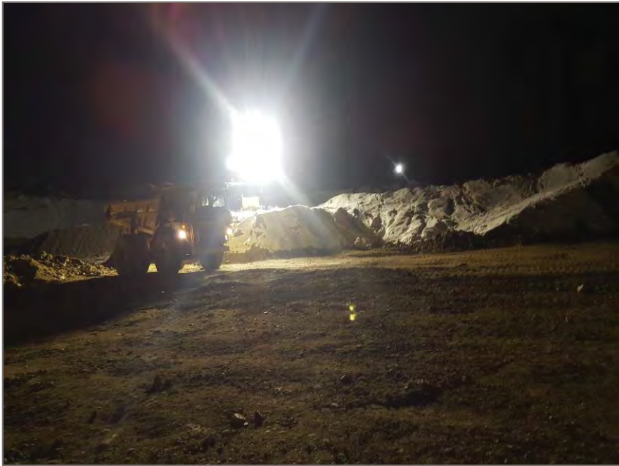
Photo 3: Compaction of material
