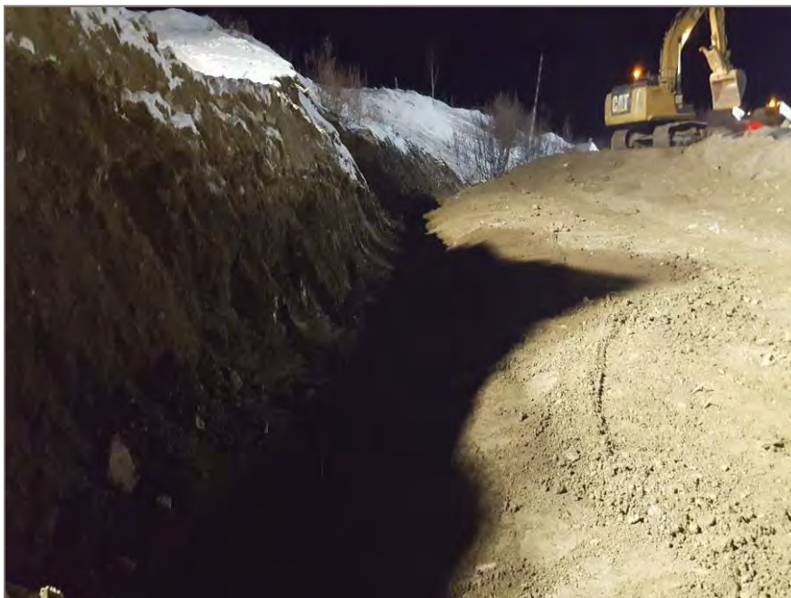
Photo 2: Material removed from bank and straight walled.
