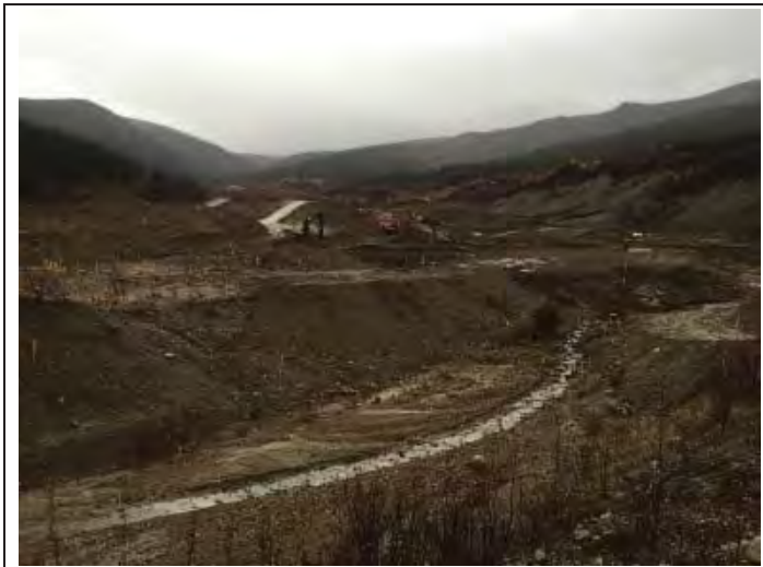
Photo 1 East view of pond excavation.
