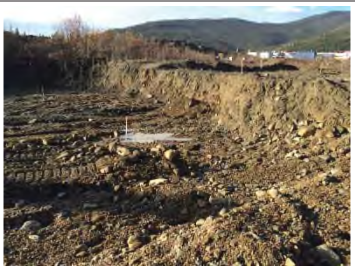
Photo 2 Northwest corner of west dam excavation. Note material present in subgrade
