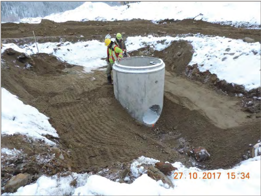
Photo 4: Backfilling around Man Hole at LLO Pipe
