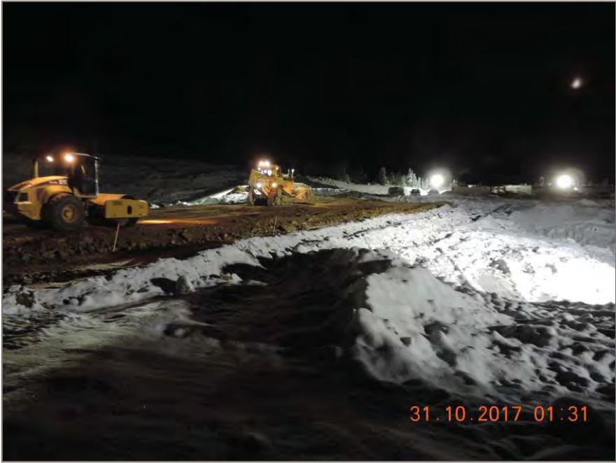
Photo 4: Extent of dam backfill at grade 811.3m, West side.
