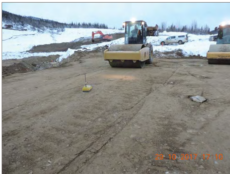
Photo 5: Moisture Density testing on sub grade fill
