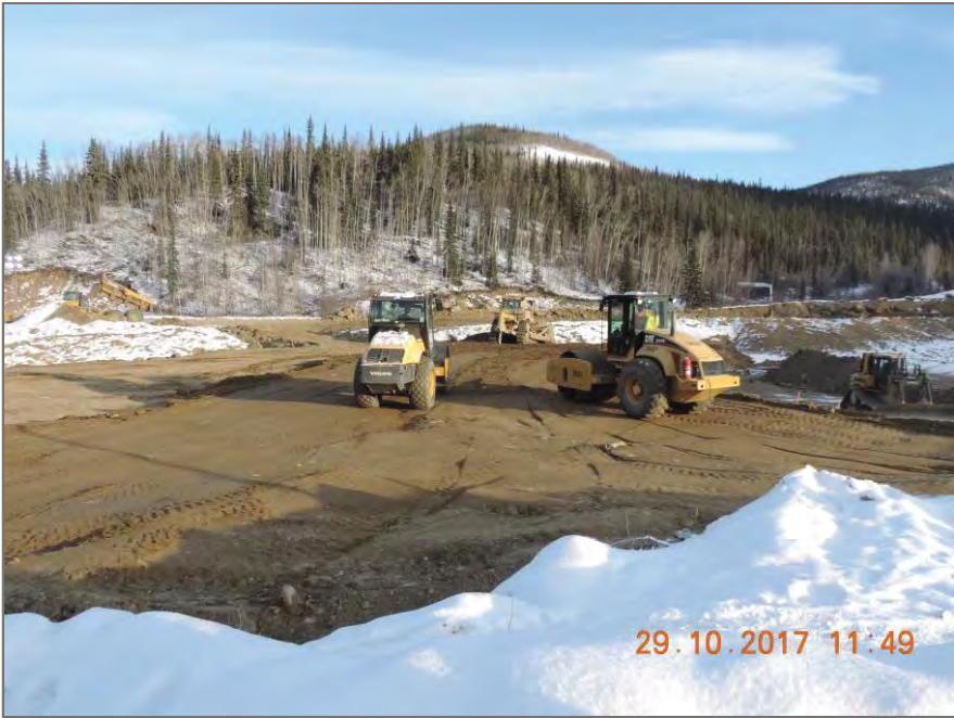
Photo 3: 2-Single Smooth Drum packers working on pad
