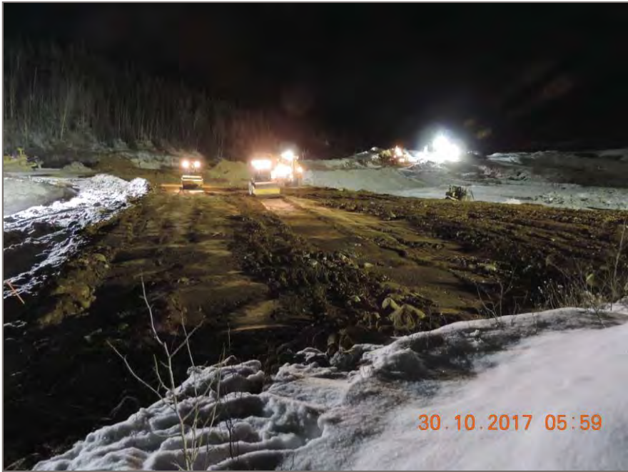
Photo 3: Compaction of placed material on 810.7m lift.
