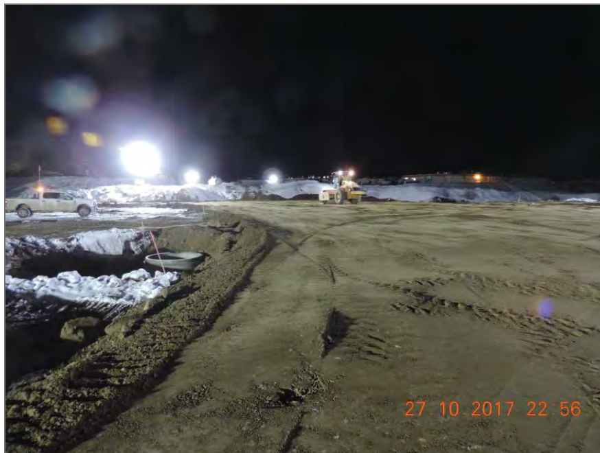
Photo 1: Compaction of pit run on 808.7 m grade lift.
