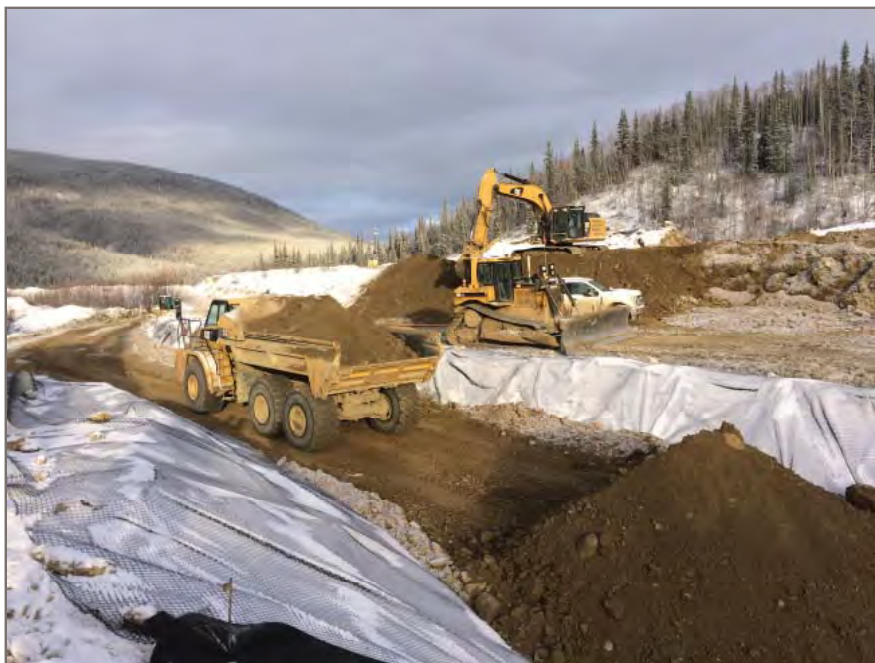
Photo 6: View from south embankment looking northwest at fill placement in-progress.
