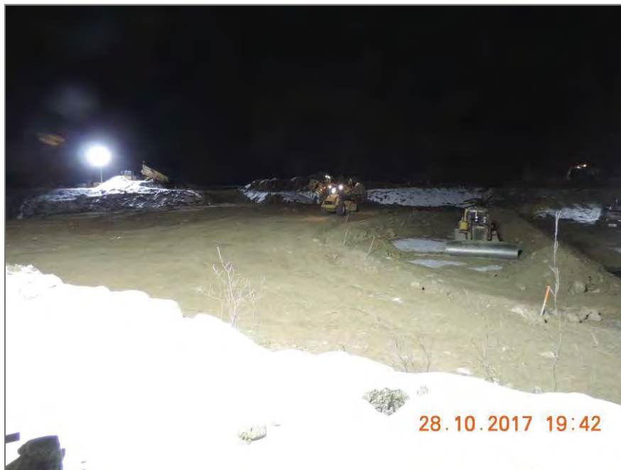
Photo 2: Placement of pit run base material for south dam on first lift.
