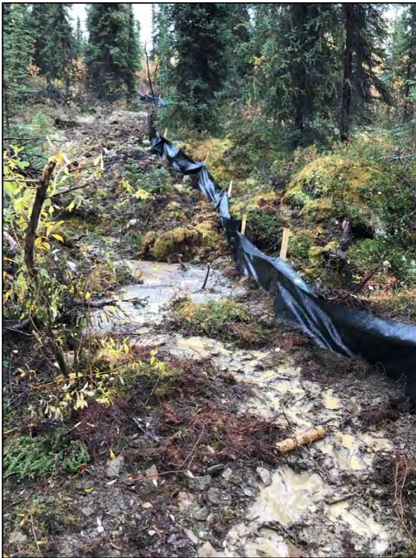
Figure 3.11-1: Silt Fence Downgradient of HLF Embankment
