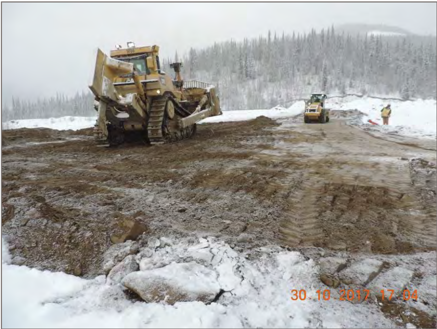
Photo 4: Dozer spreading second lift of subgrade
