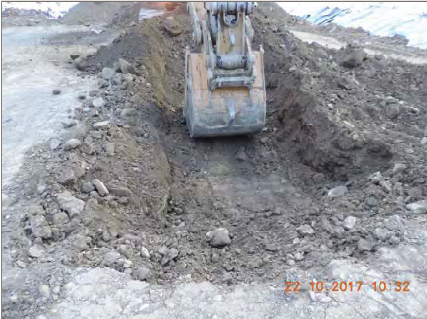
Photo 2: Test of material placed through night shift show organics and high clay content.
