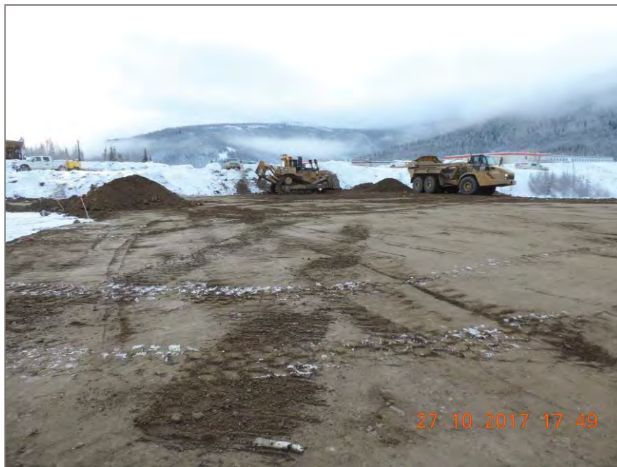
Photo 5: Pelly continues backfilling throughout day shift
