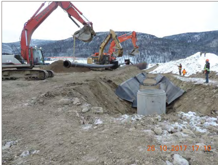
Photo 5: Positioning HDPE Pipe to Trench Bed with three excavators
