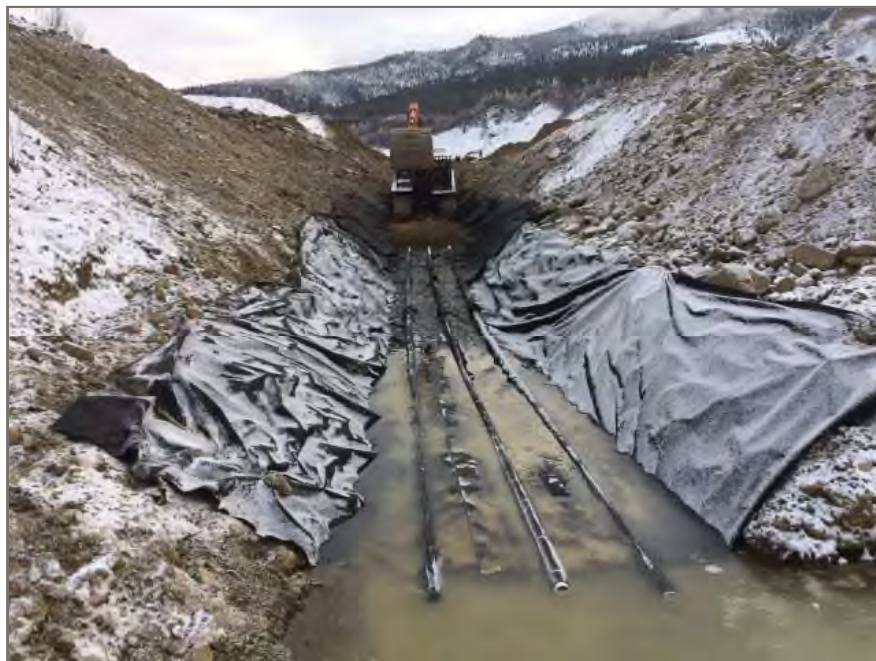
Photo 2: Placement of 20 mm minus drain rock in progress within underdrain area
