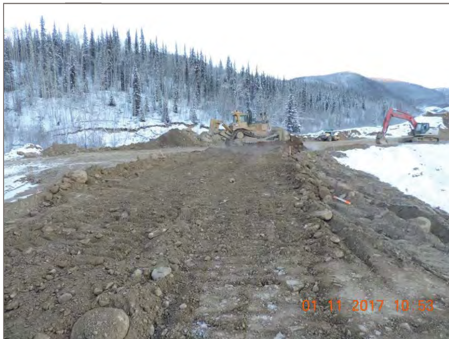
Photo 2: Cat D10T Dozer spreads subgrade fill on South Dam
