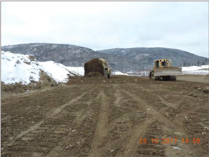
Photo 4: Second lift placed with prior lift scarified prior to backfill
