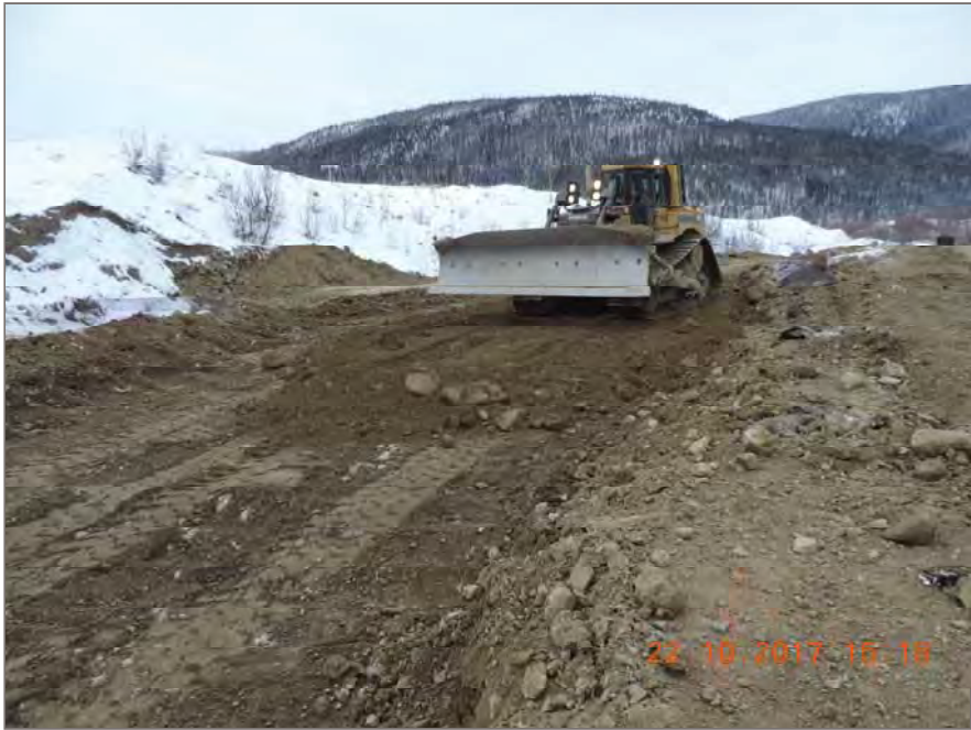
Photo 5: New sourced material placed, spread and compacted.
