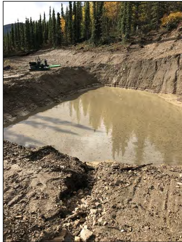
Figure 3.11-2: Temporary HLF Runoff and Exfiltration Basin
