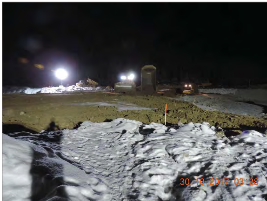
Photo 2: Replacement of material along stripped lift.
