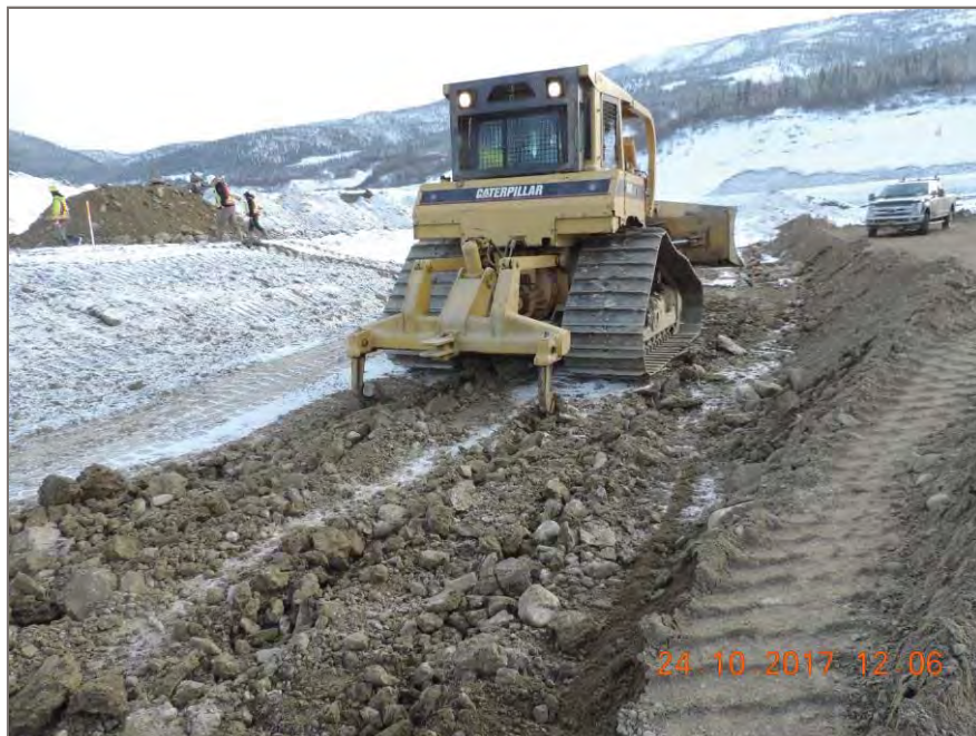
Photo 2: Backfill area ripped with removal of exiting snow removed before backfill
