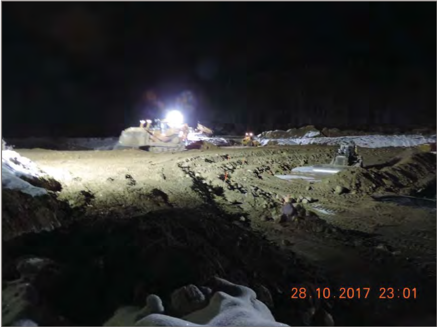
Photo 4: Extent of dam embankment to date.
