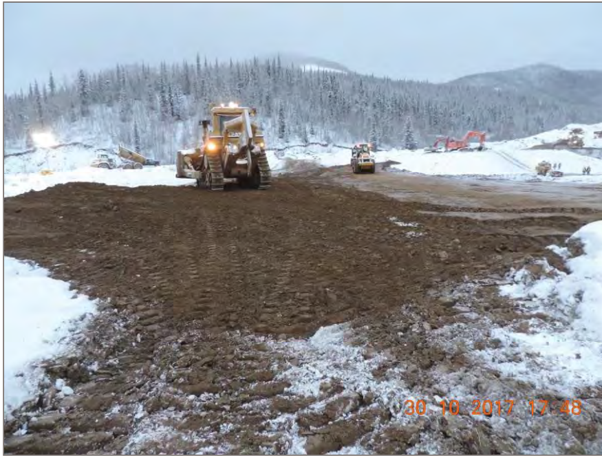
Photo 5: Progress from day shift on Dam fill complete at Elevation: 811.0
