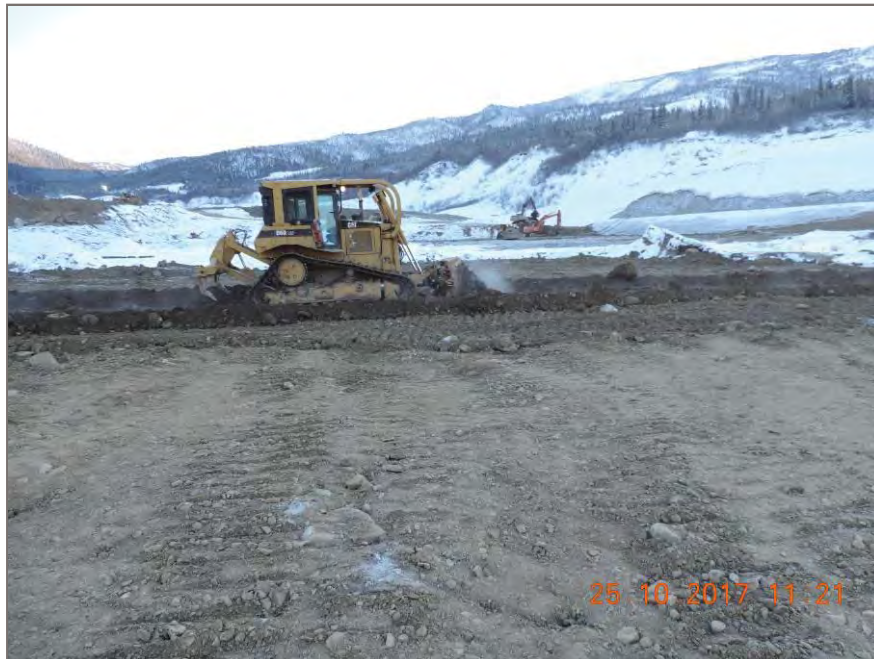
Photo 2: Over-sized lift placed cut back to 300mm lift thickness before compacting
