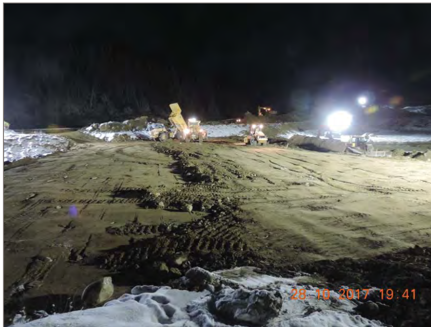
Photo 1: Compaction and placement of pit run on 809.6 m grade lift.
