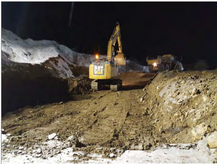
Photo 1: Removal of unsuitable material within berm
