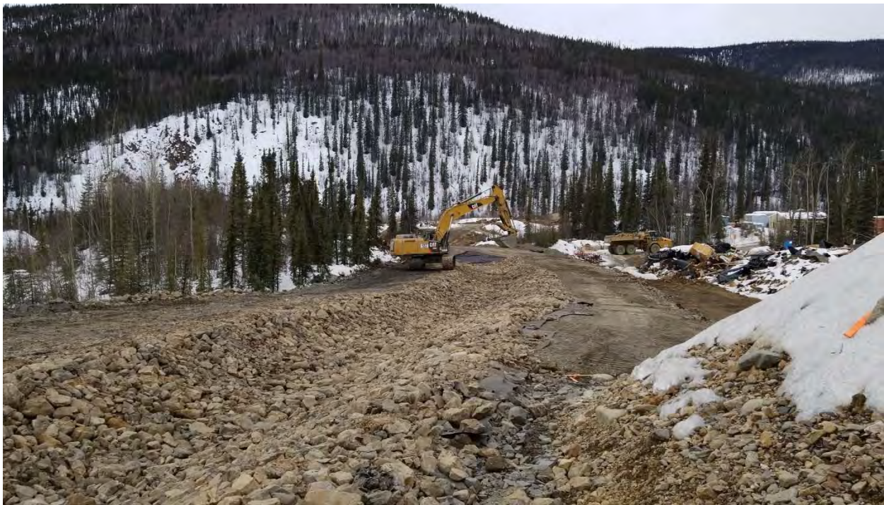
Figure 22. Ditch C Riprap Placement near STN 0+400 Looking Downstream
