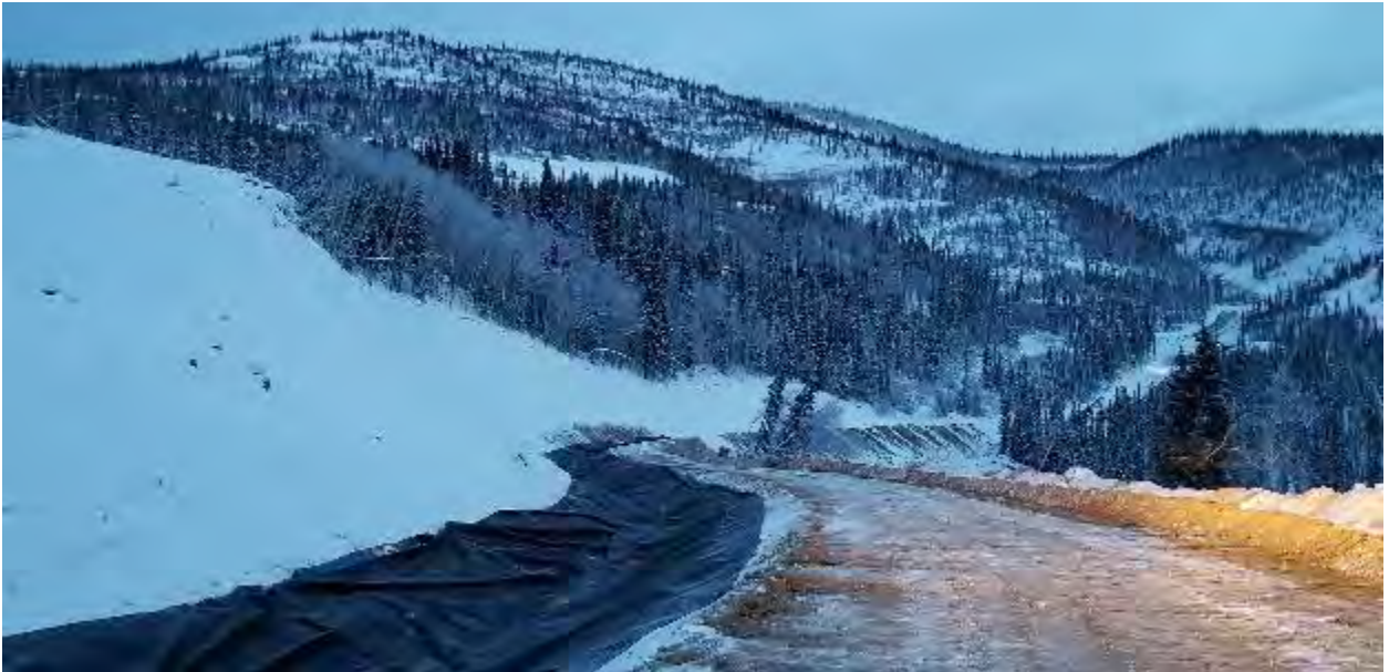
Photo 2 - 18.12.13 - Ditch A station 0+700
