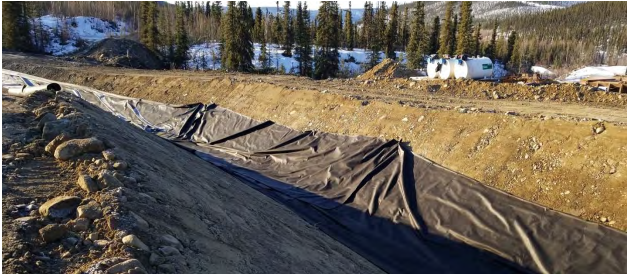
Figure 21. Ditch C Liner Placement near STN 0+500
