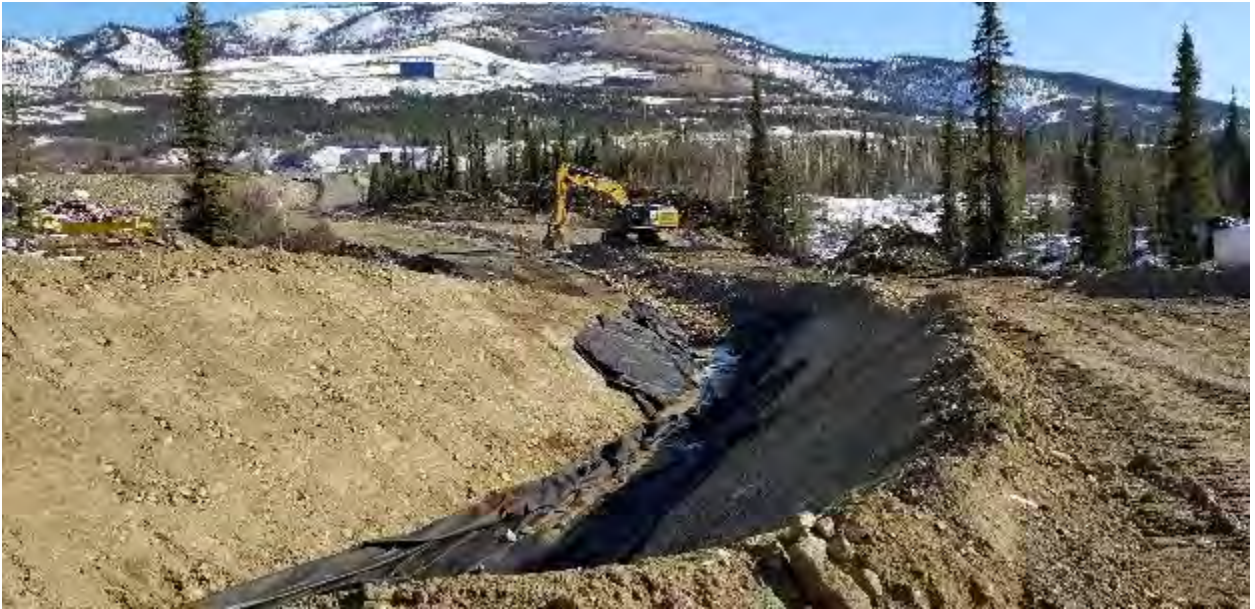
Photo 86 - 20190330 Ditch C Prep for Rip Rap
