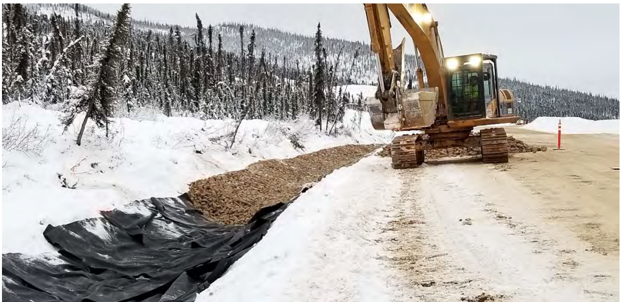
Figure 3. Ditch A Riprap Placement near STN 0+800 Looking upstream
