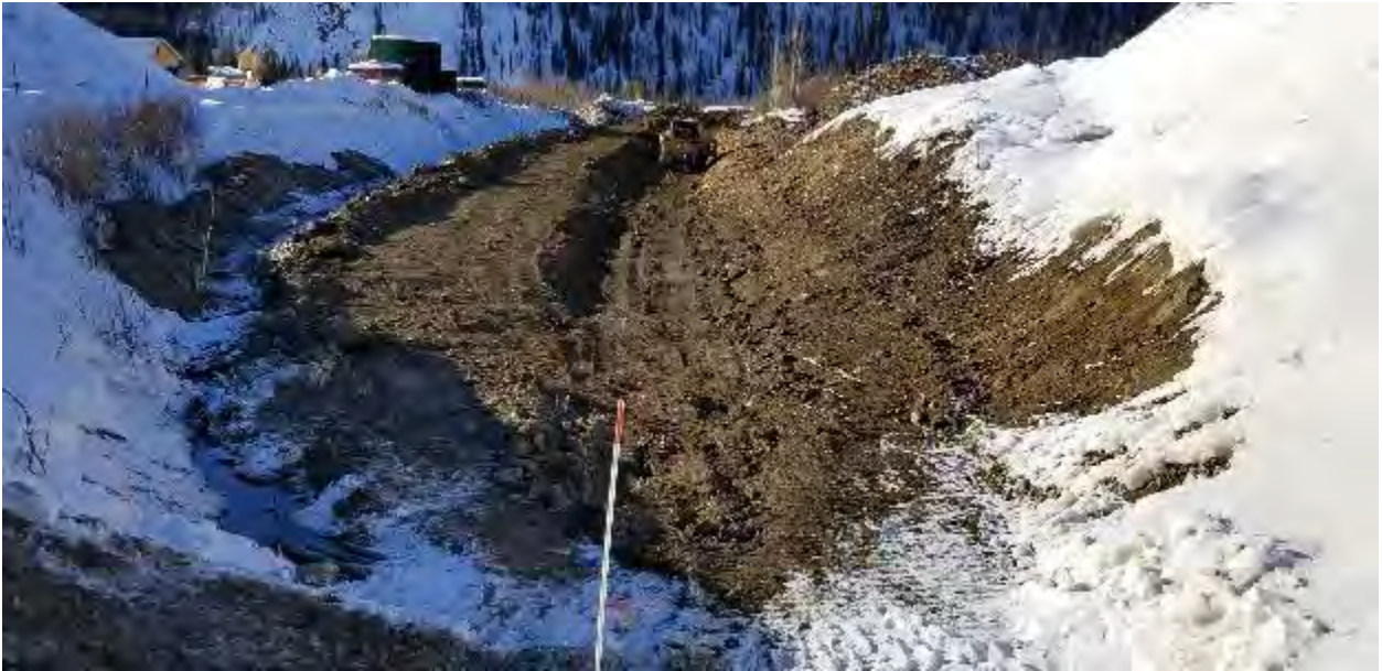
Photo 80 - 20190312 Ditch C Construction
