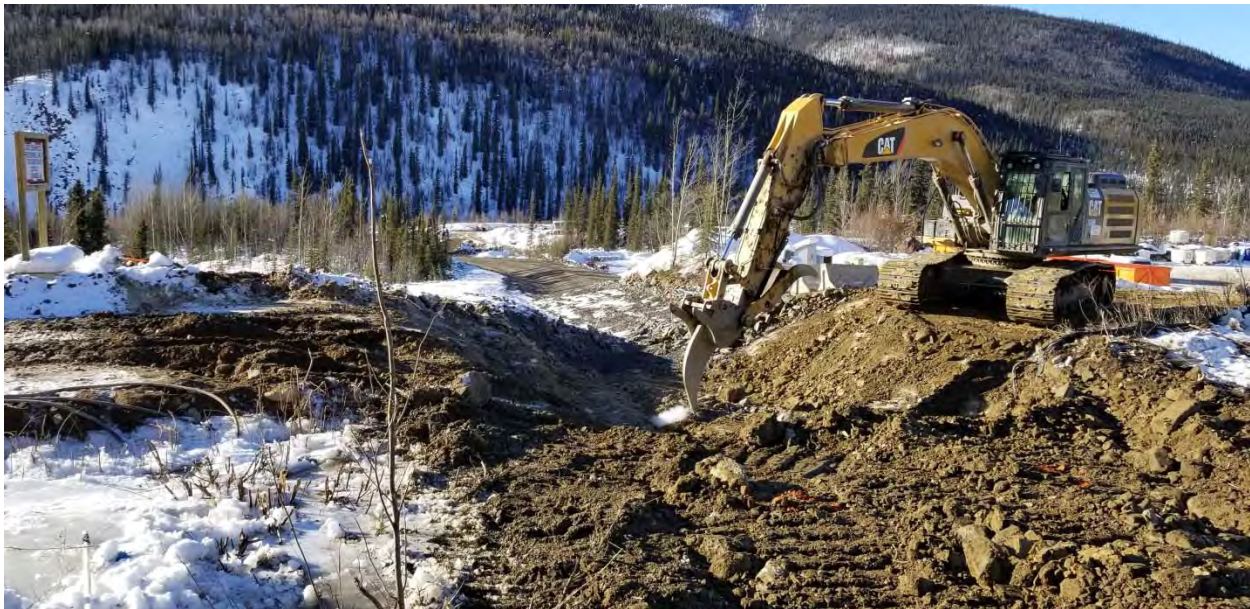
Figure 16. Ditch C Ripping for Culvert Placement near STN 0+200
