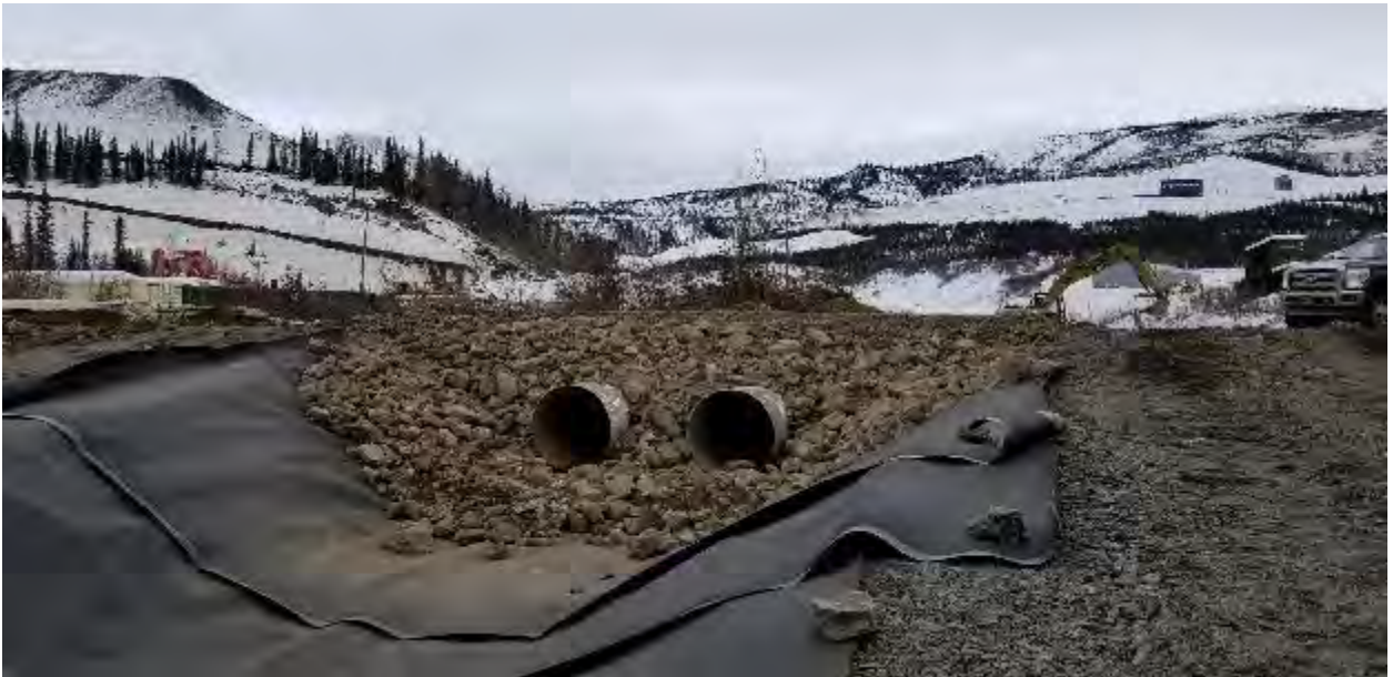
Photo 83 - 190316 Ditch C Culvert Install on Shop Road
