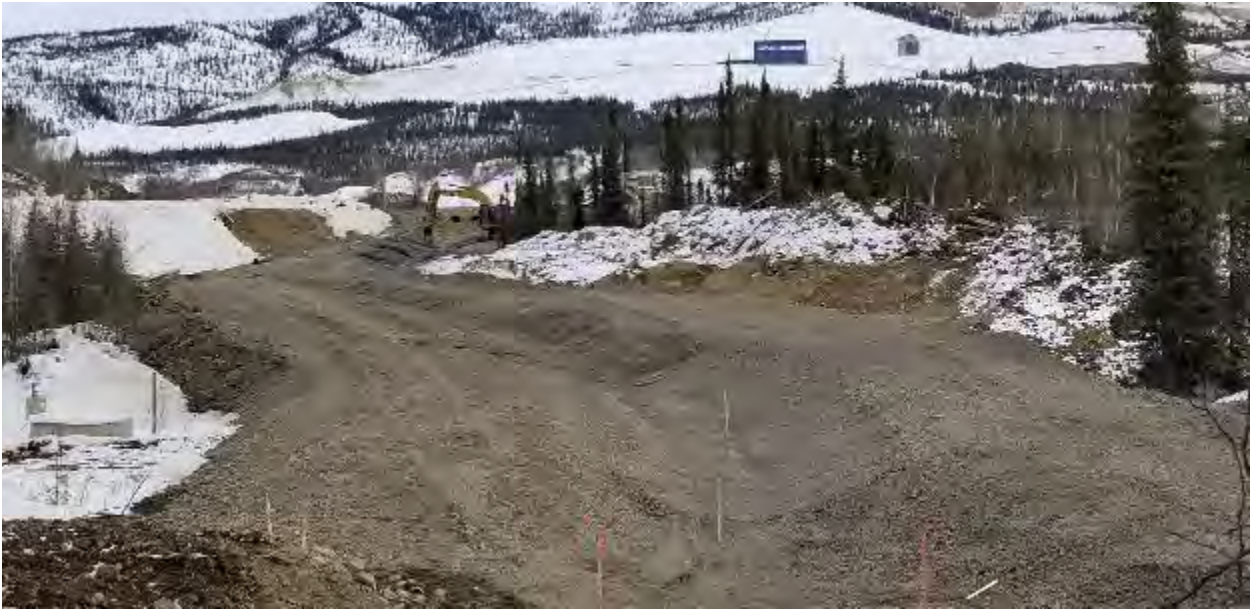
Photo 84 - 20190317 Ditch C Rip Rap Install
