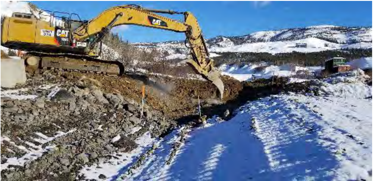
Photo 81 - 190312 - Ditch C Ripping and Excavating for Shop Road Culvert Crossings
