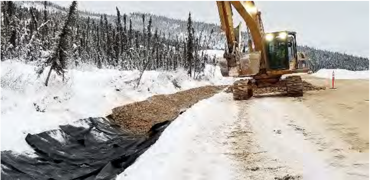
Photo 45 - 20181121 Ditch A Riprap Placement
