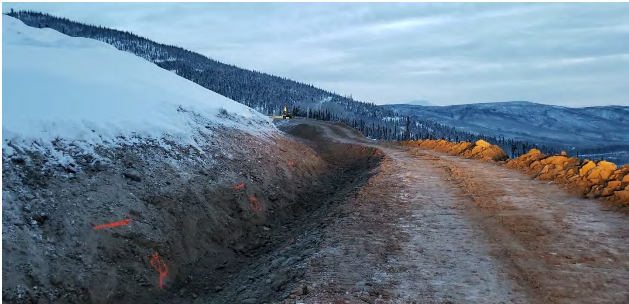
Figure 1. Ditch A Shaping near STN 0+450 Looking Upstream
