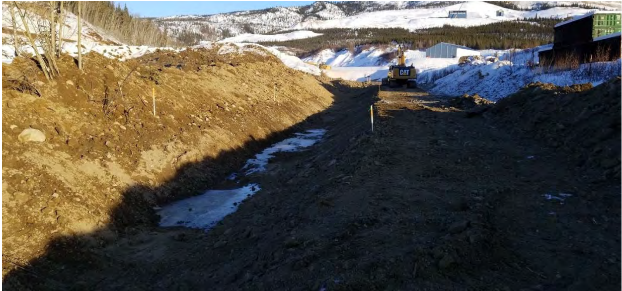
Figure 17. Ditch C Shaping near STN 0+100 Looking Upstream
