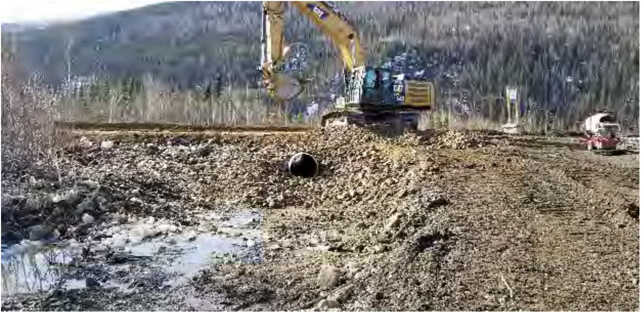
Photo 105 - 20190401 New 900mm Culvert for Eagle Offset
