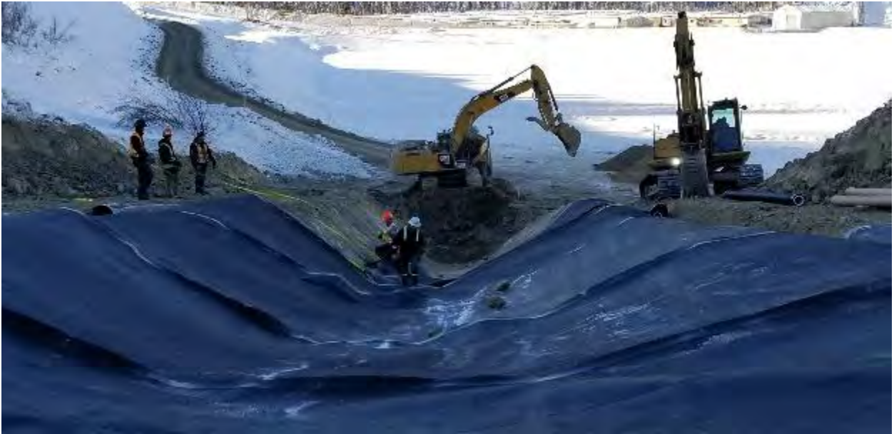
Photo 57 - 20190226 Ditch B Liner Installation to Control Pond
