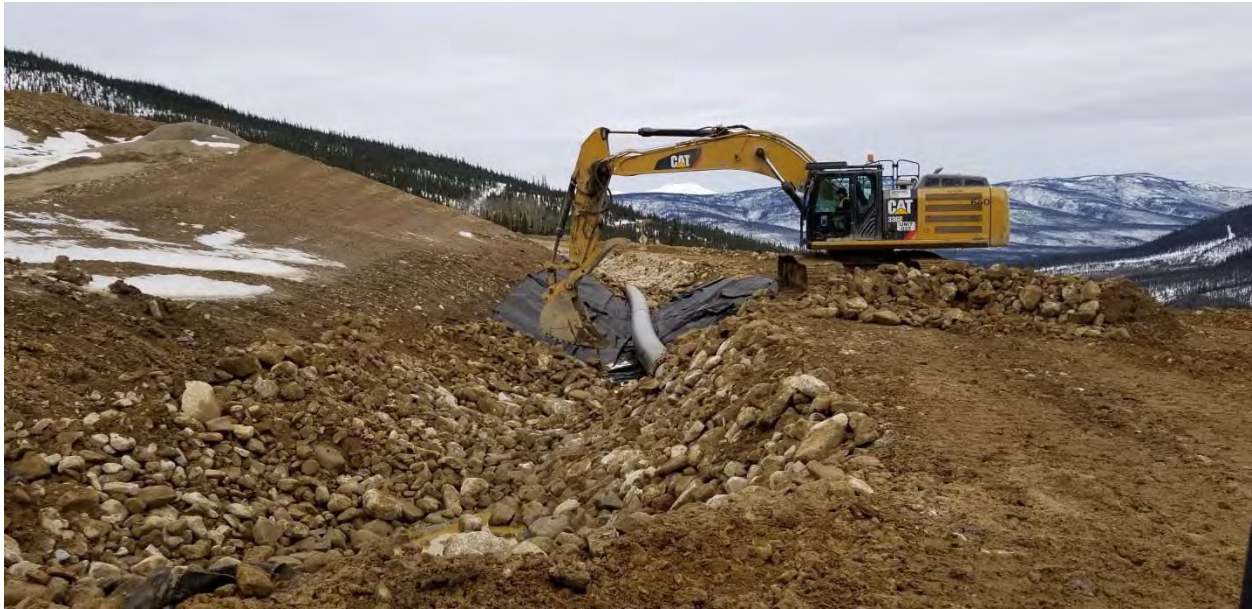
Figure 8. Placement of Final Riprap on Ditch A near STN 0+550
