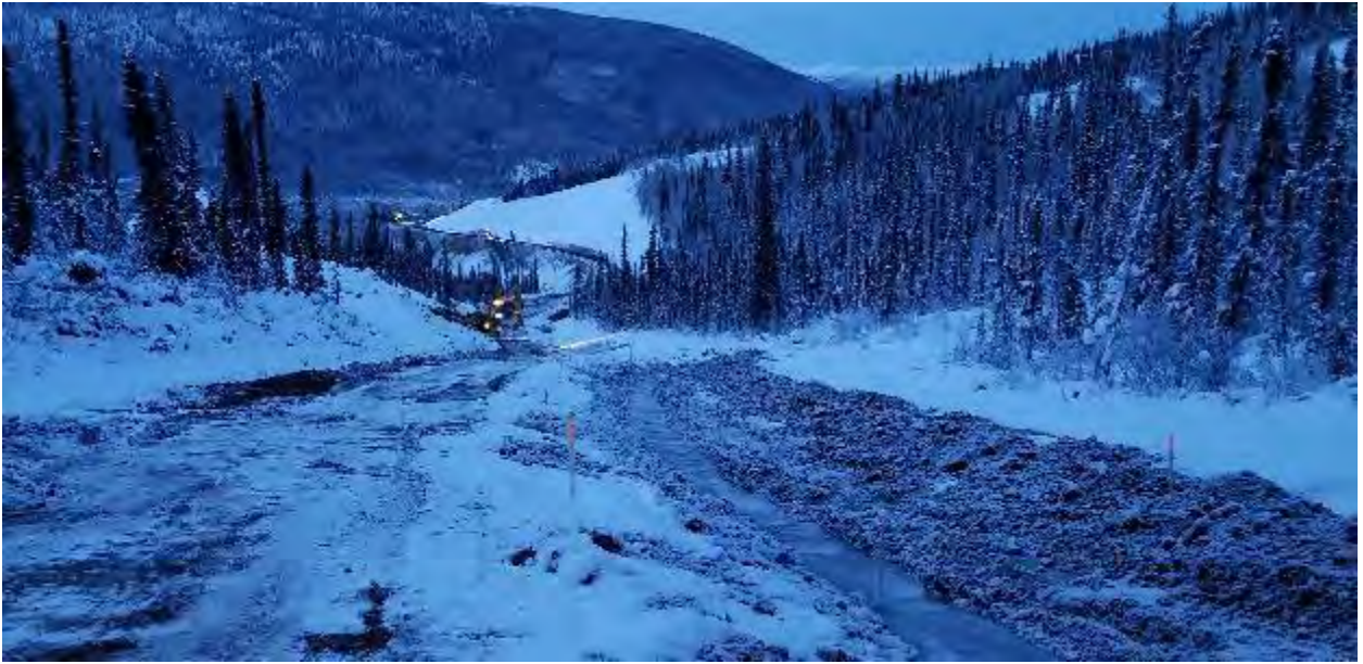
Photo 1 - 18.12.13 - Ditch A station 0+100
