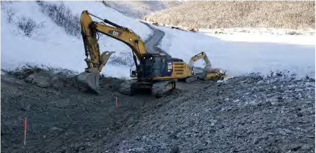
Photo 55 - 190216 - Ditch B Excavation to Control Pond Forebay
