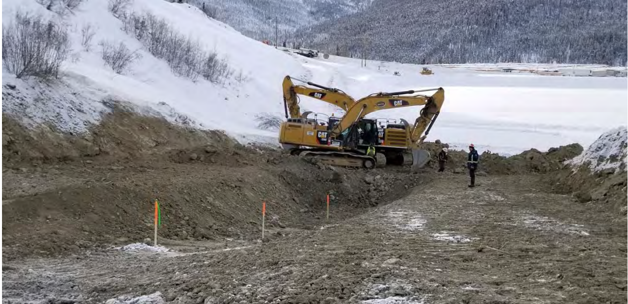
9. Ditch B Shaping near STN 0+260 Looking Downstream
