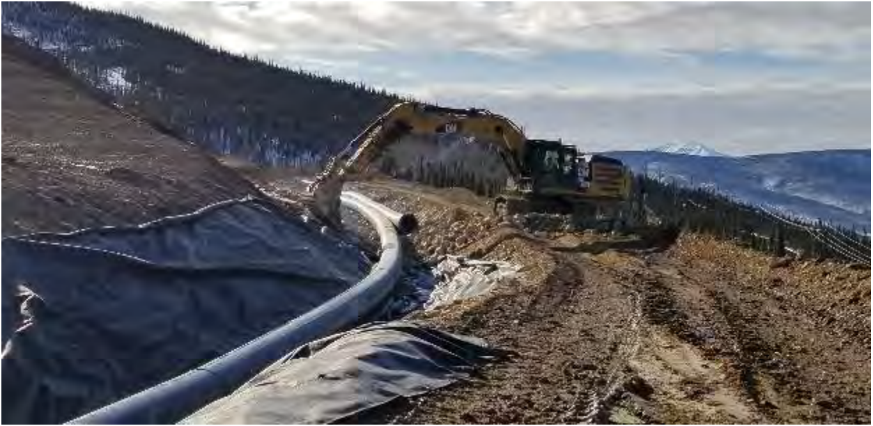
Photo 10 - 19.03.28 -Ditch A Final Rip Rap Placement
