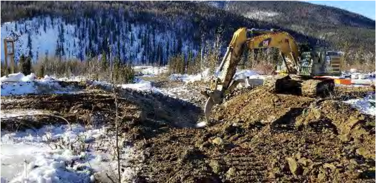
Photo 82 - 20190312 Ditch C Ripping and Excavating for Shop Road Culvert Crossings
