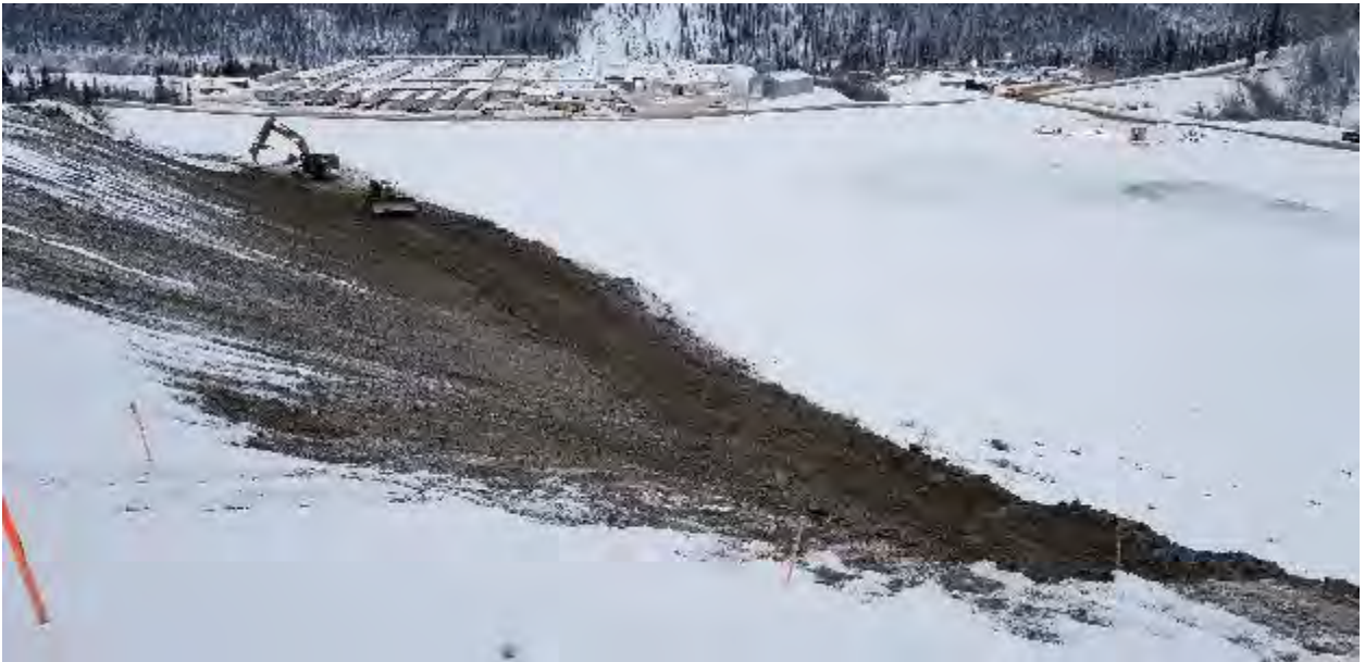
Photo 41 - 20181124 Ditch A Earthworks
