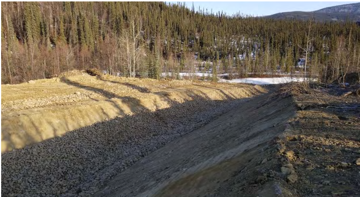
Figure 24. Ditch C Completion near STN 0+550 Looking Downstream
