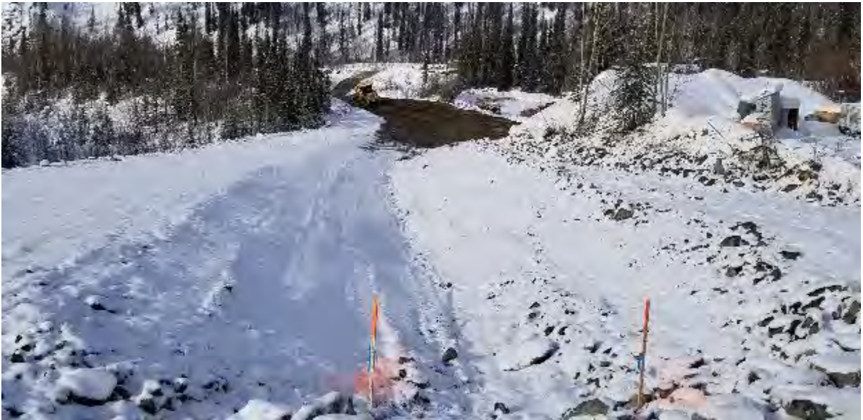
Photo 79 - 20190311 Ditch C Construction
