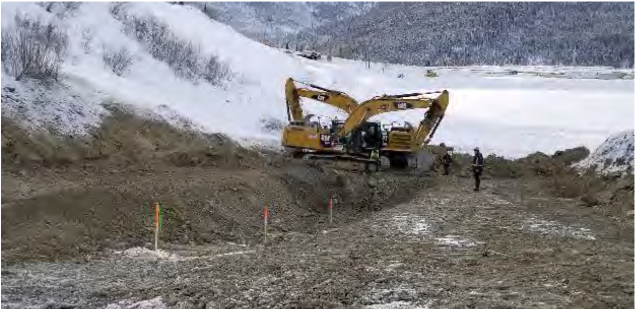
Photo 56 - 190219 - Ditch B Excavation to Control Pond Forebay
