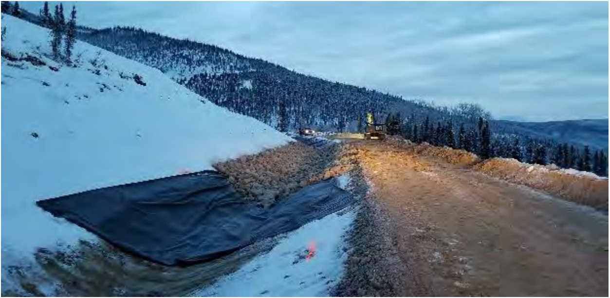
Photo 3 - 18.12.13 -Ditch A station 0+800
