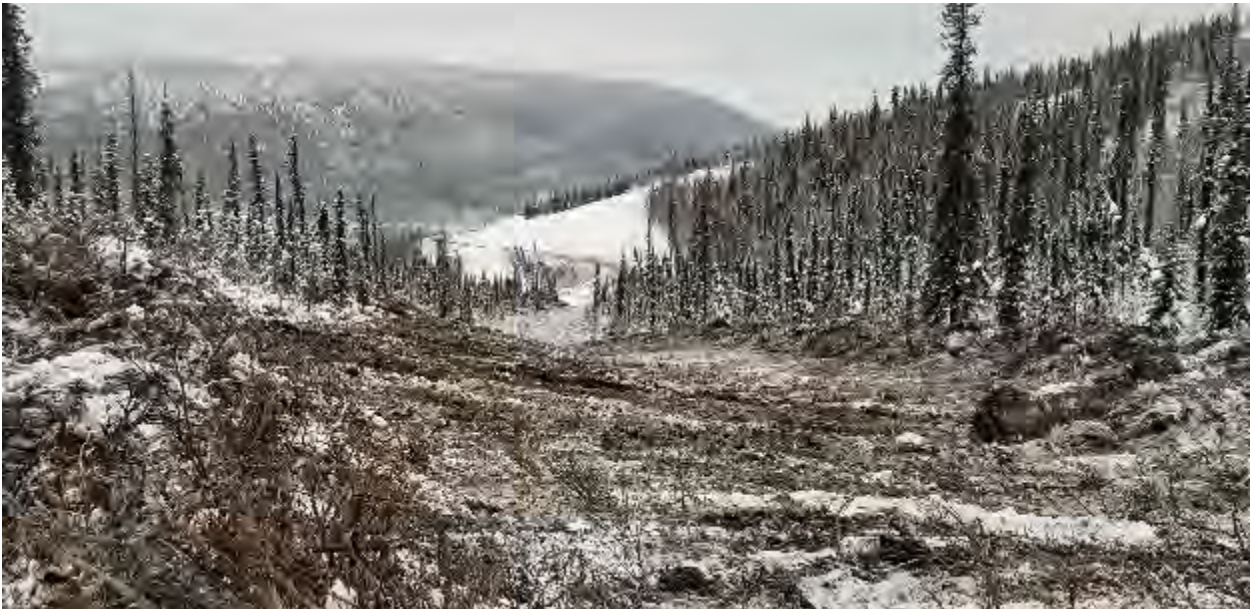
Photo 37 - Ditch A Clearing and Ground prep
