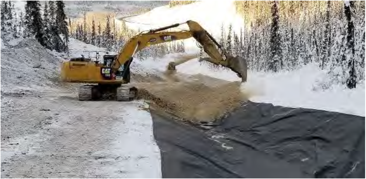
Photo 44 - 20190127 Ditch A Riprap Placement
