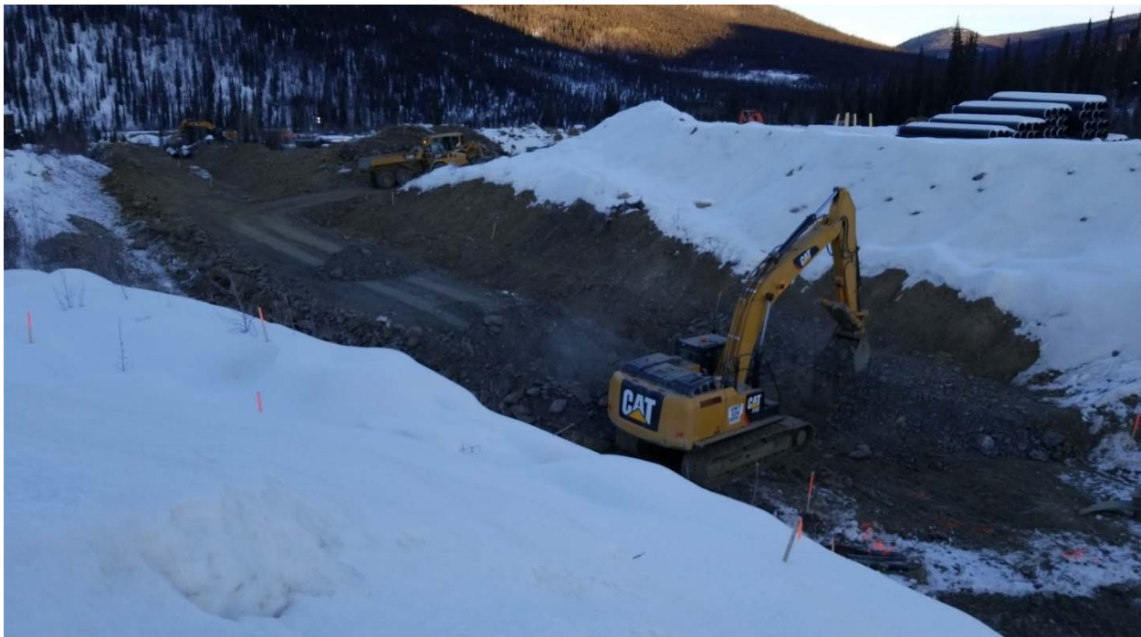
Figure 20. Ditch C Shaping near STN 0+350
