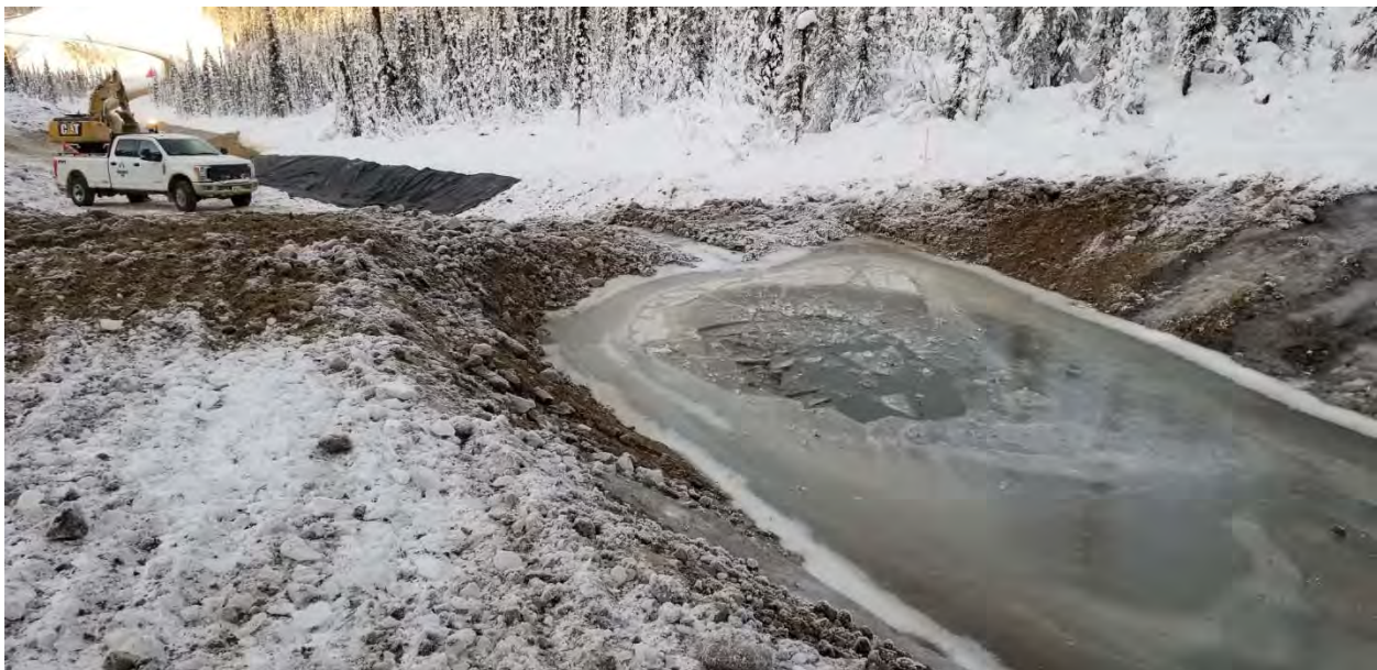
Figure 5. Ditch A Sump Before during Shaping and Before Lining
