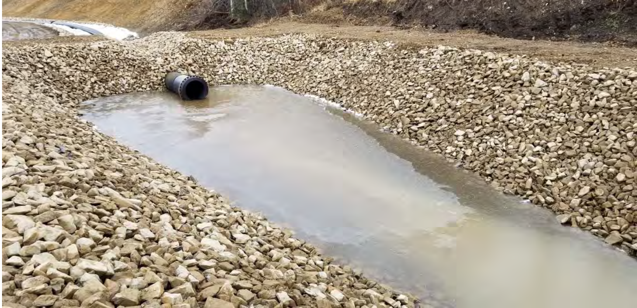
Figure 6. Ditch A Sump After lining and Riprap Installed
