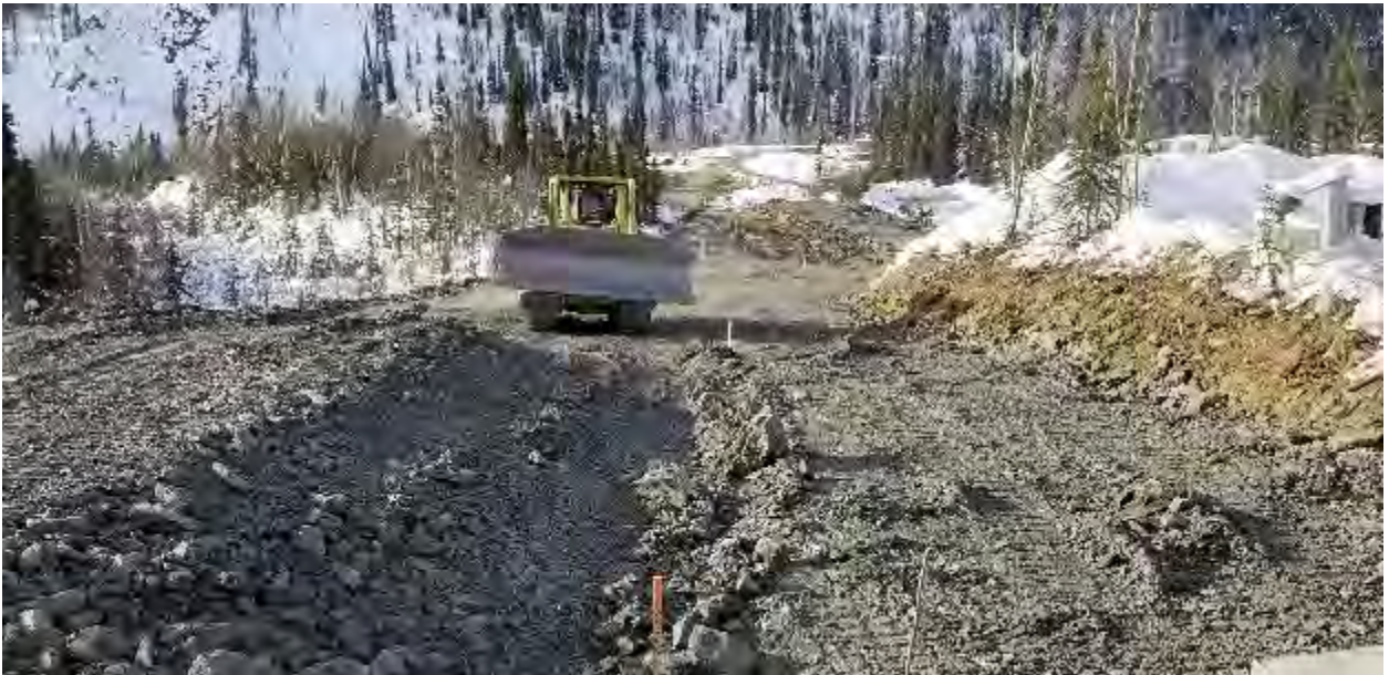
Photo 77 - 20190308 Ditch C Construction
