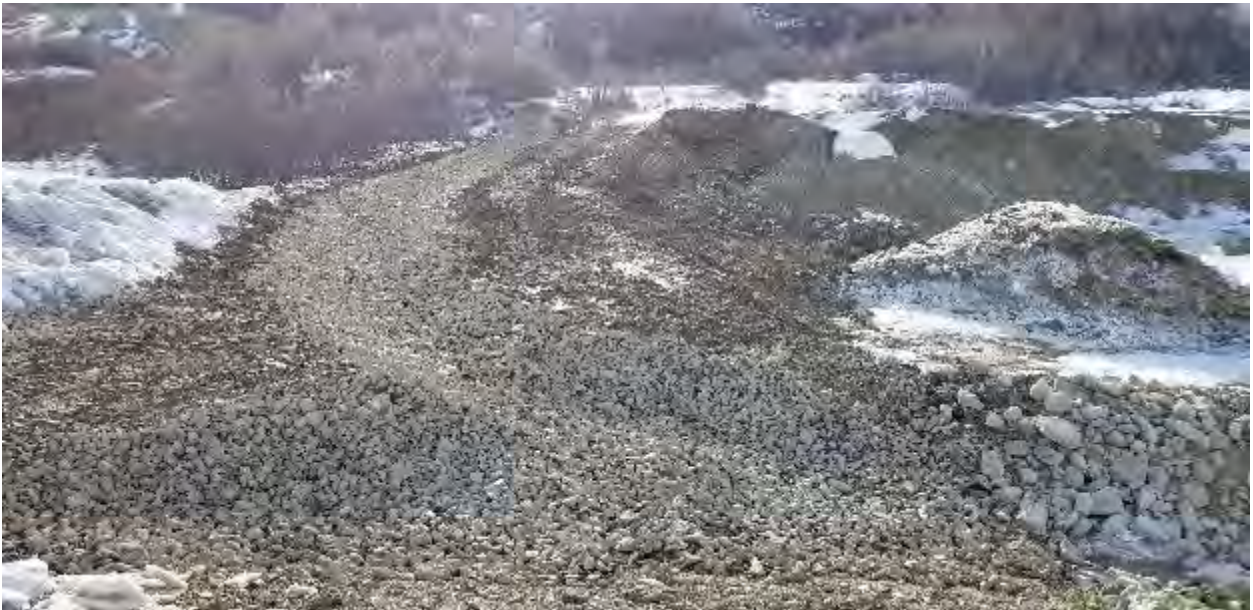
Photo 58 - 20190419 Suttles to Ditch B Diversion Complete
