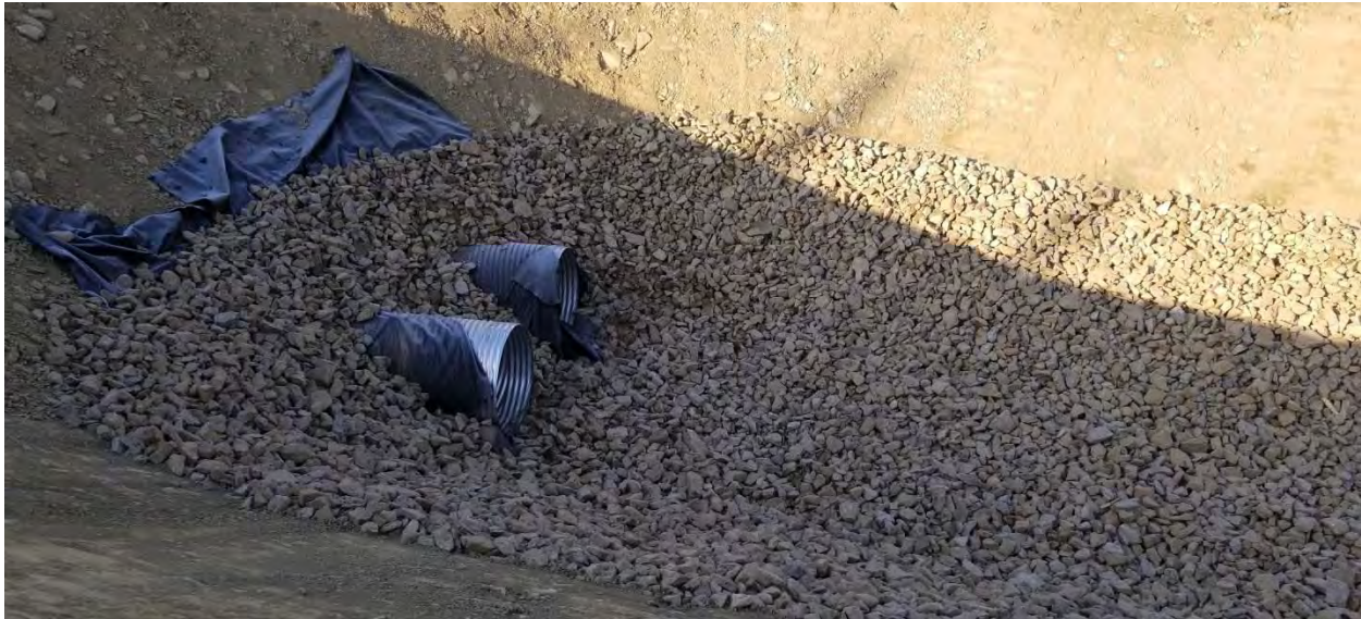
Figure 23. Ditch C Completion of Dual Culverts near STN 0+460
