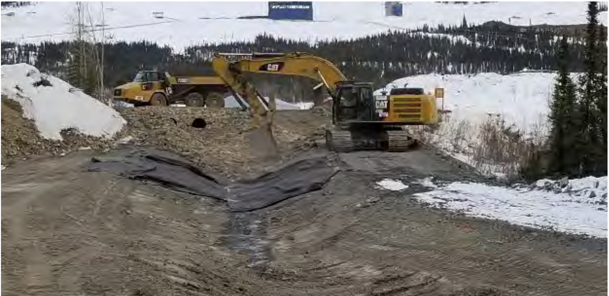
Photo 85 - 20190317 Ditch C Rip Rap Install
