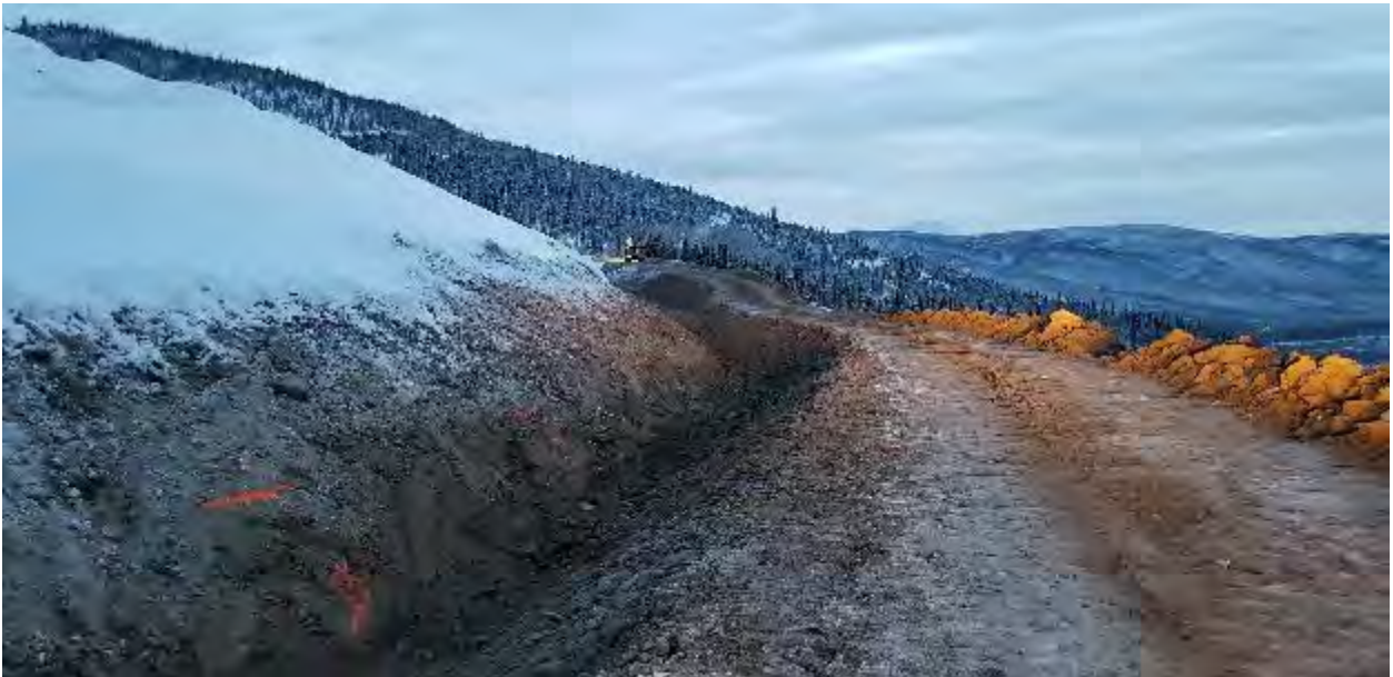
Photo 4 - 18.12.13 -Ditch A station 0+900 - Finished Cut
