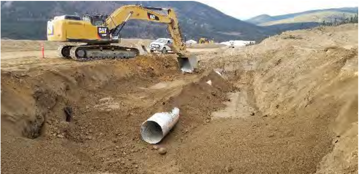
Photo 39 - Ditch A Culvert Placement
