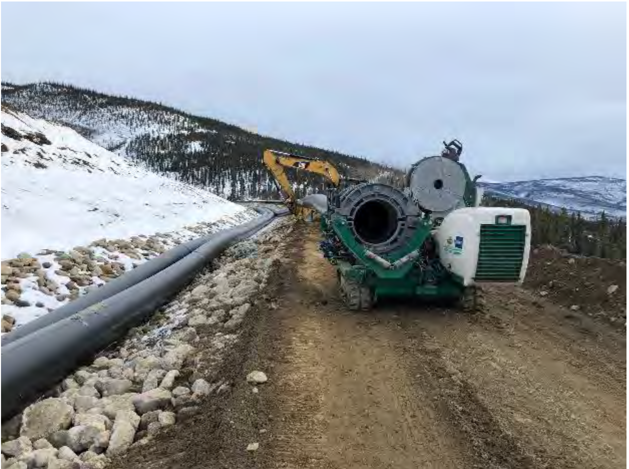
Photo 9 - 19.03.19 - Fusing pipe for Ditch A
