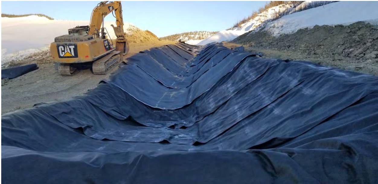
12. Ditch B Non-Woven Geotextile Lining Placement near STN 0+000 Looking Upstream
