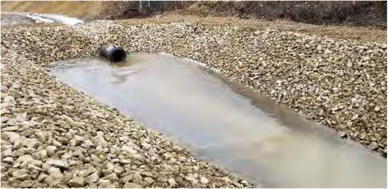
Photo 38 - 20190419 Ditch A Collection Sump Complete
