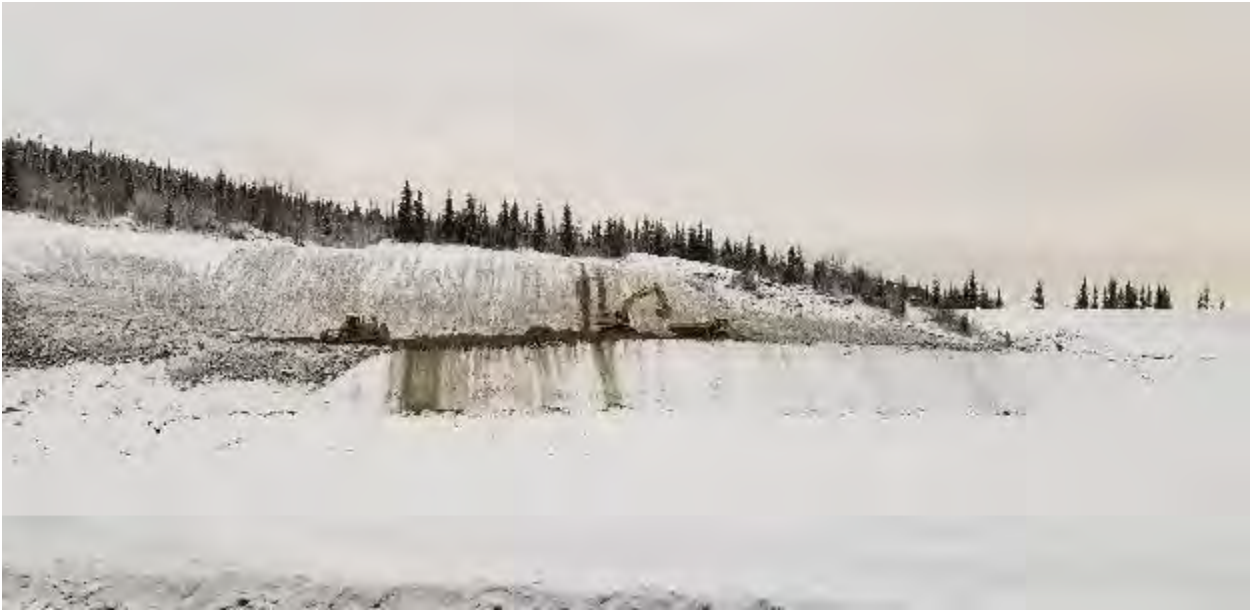
Photo 42 - 20181125 Ditch A Earthworks
