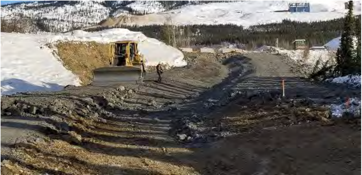
Photo 78 - 20190309 Ditch C Construction
