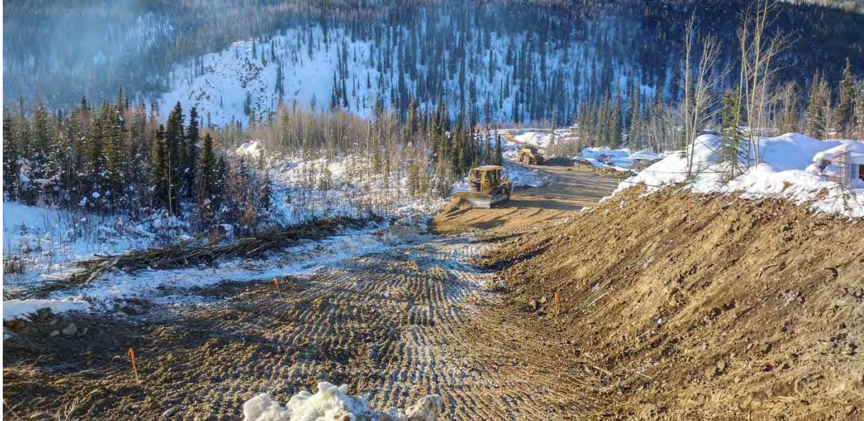
Figure 15. Ditch C Shaping near STN 0+300 Looking Downstream
