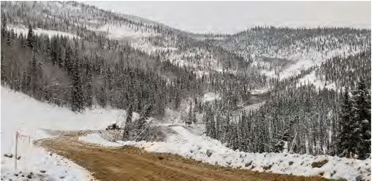
Photo 43 - 20181201 Ditch A Earthworks
