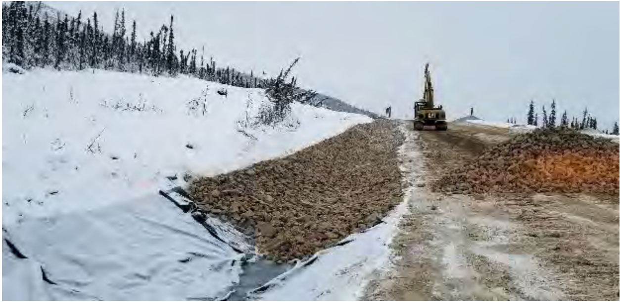
Photo 46 - 20181124 Ditch A Riprap Placement
