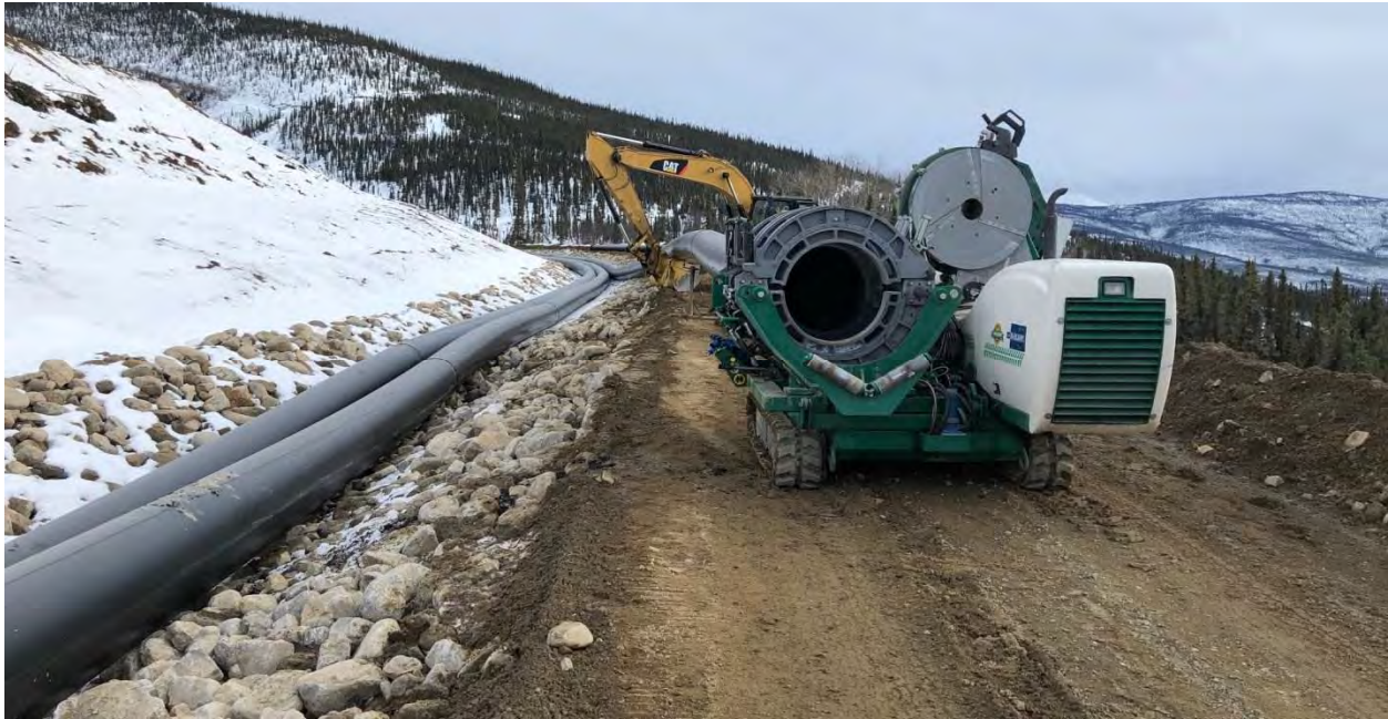
Figure 4. Fusing Machine and Temporary Placement of Contact Water Pipeline near STN 0+550
