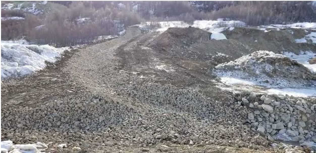
14. Ditch B Suttles Gulch Capture Completion
