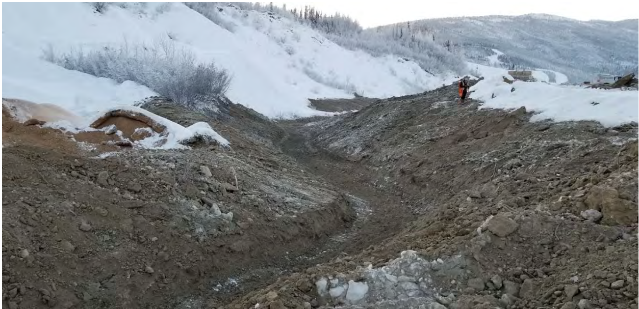
10. Ditch B Shaping near STN 0+160 Looking Upstream
