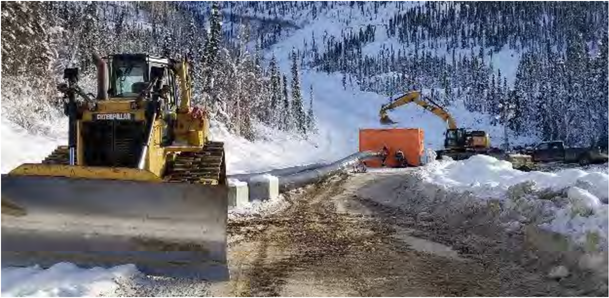
Photo 6 - 19.02.20 - Fusing 28 Inch Pipe for Ditch A
