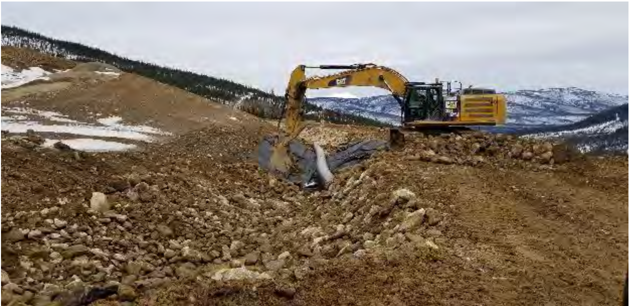
Photo 11 - 19.03.28 -Ditch A Final Rip Rap Placement
