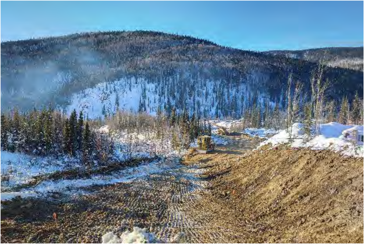
Photo 76 - 190303 Ditch C Stripping and Grubbing
