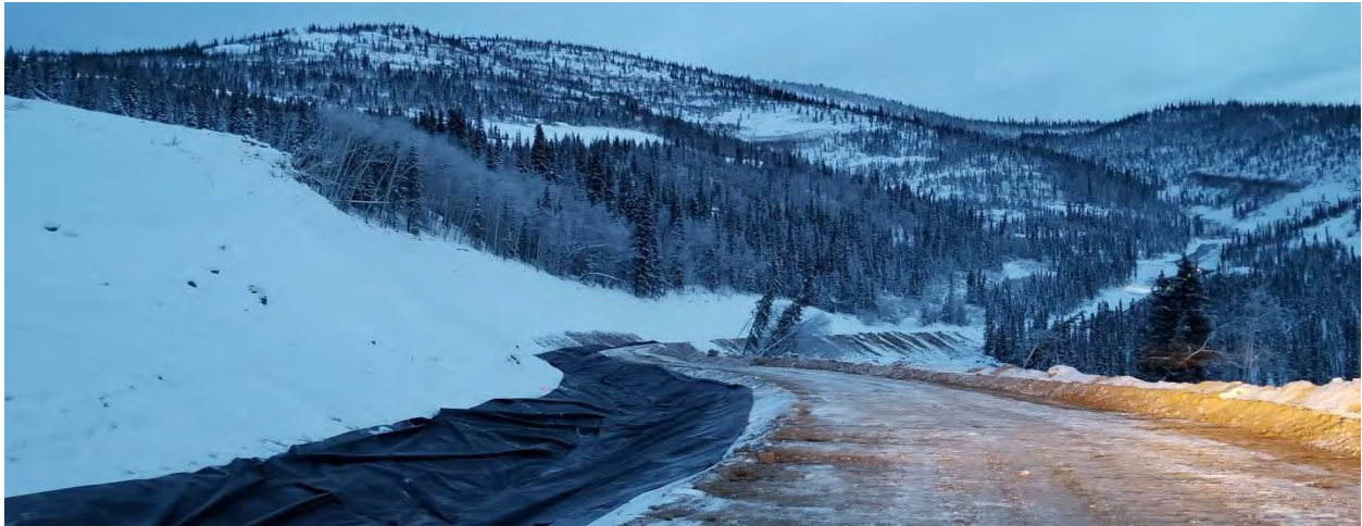
Figure 2. Ditch A Non-Woven Geotextile Lining near STN 0+375 Looking Upstream
