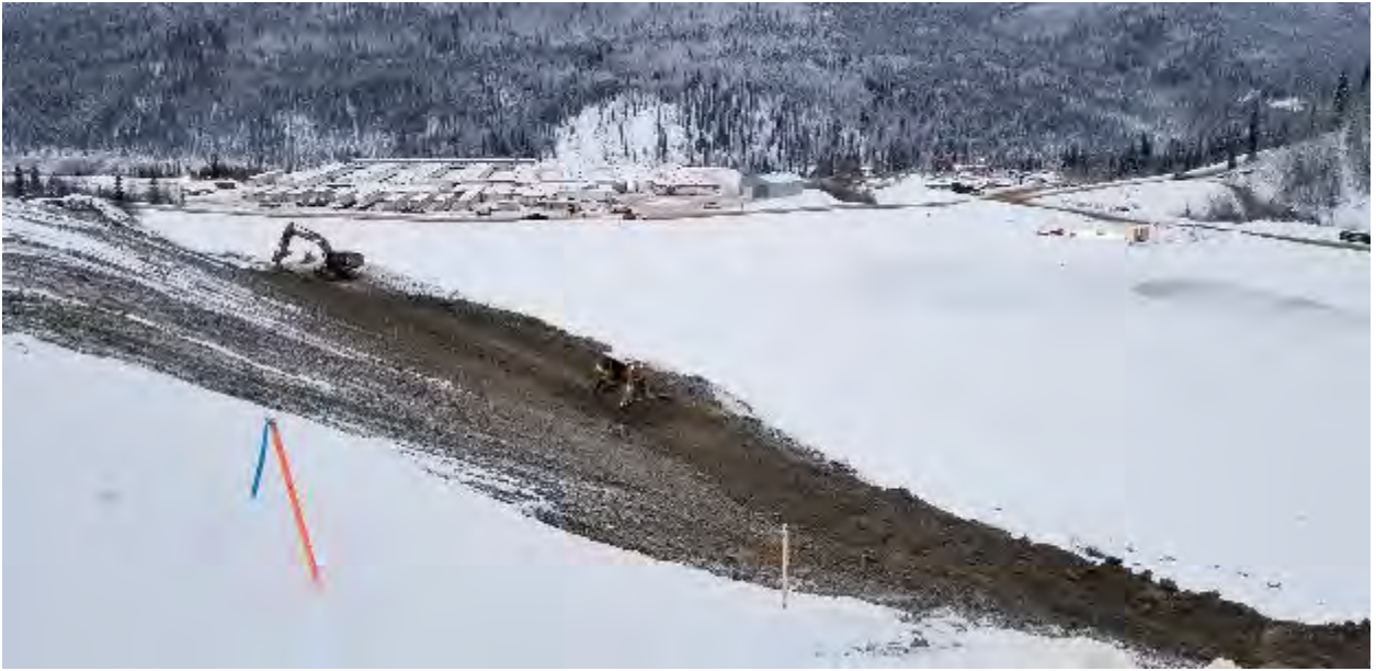
Photo 40 - 20181124 Ditch A Earthworks
