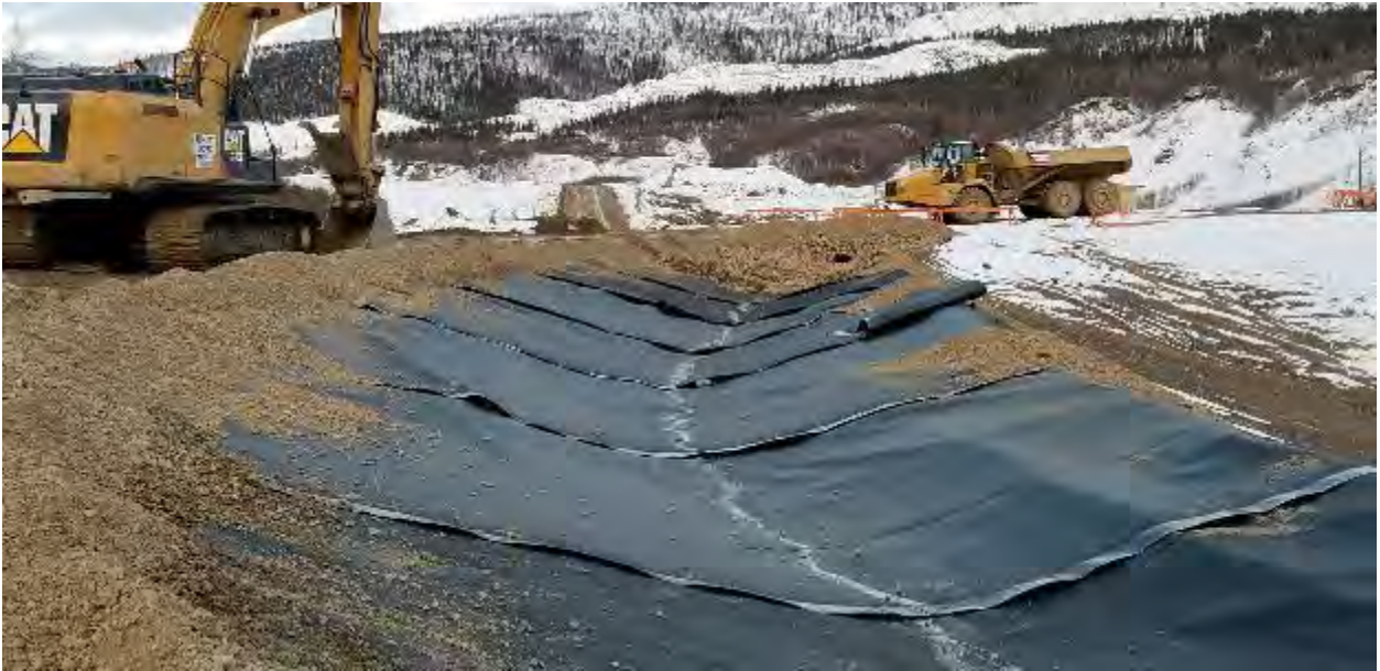
Photo 106 - 20190424 Eagle Offset Diversion Ditch
