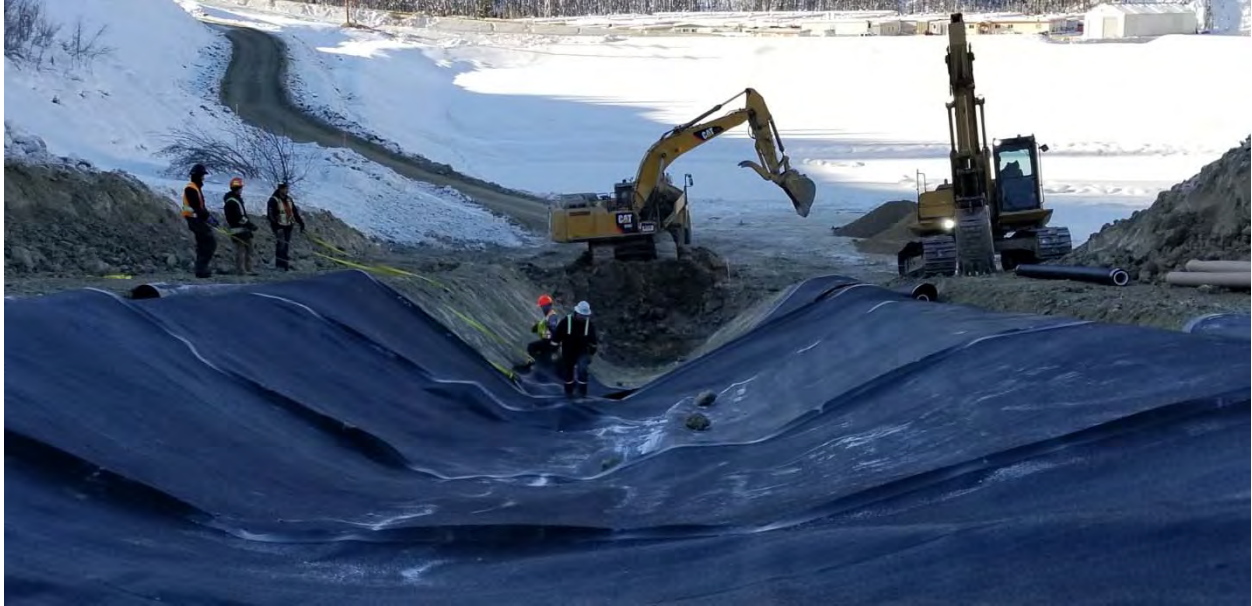
11. Ditch B Non-Woven Geotextile Lining Placement near STN 0+280 Looking Downstream
