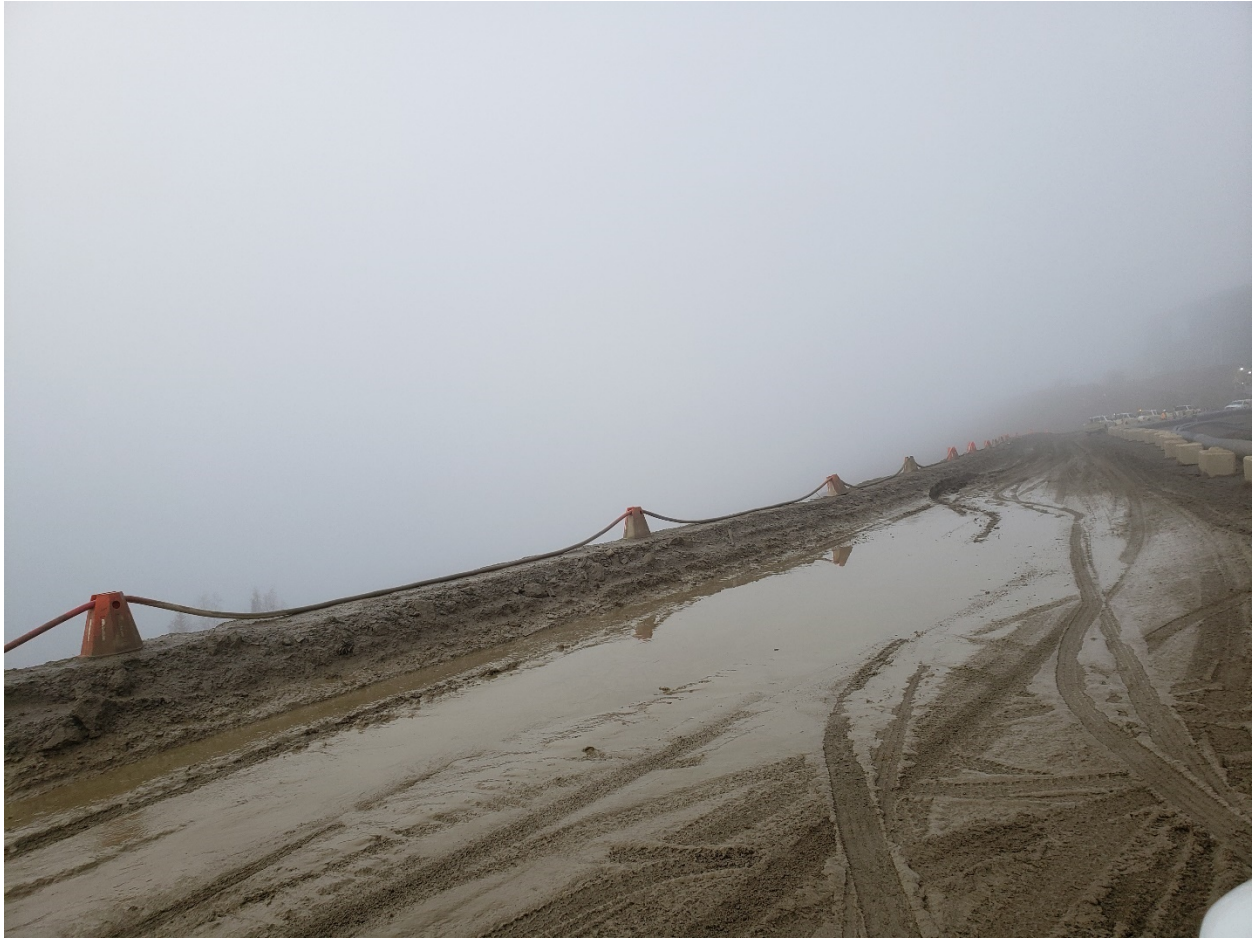
Photo 13. HLF Dam crest looking west.
