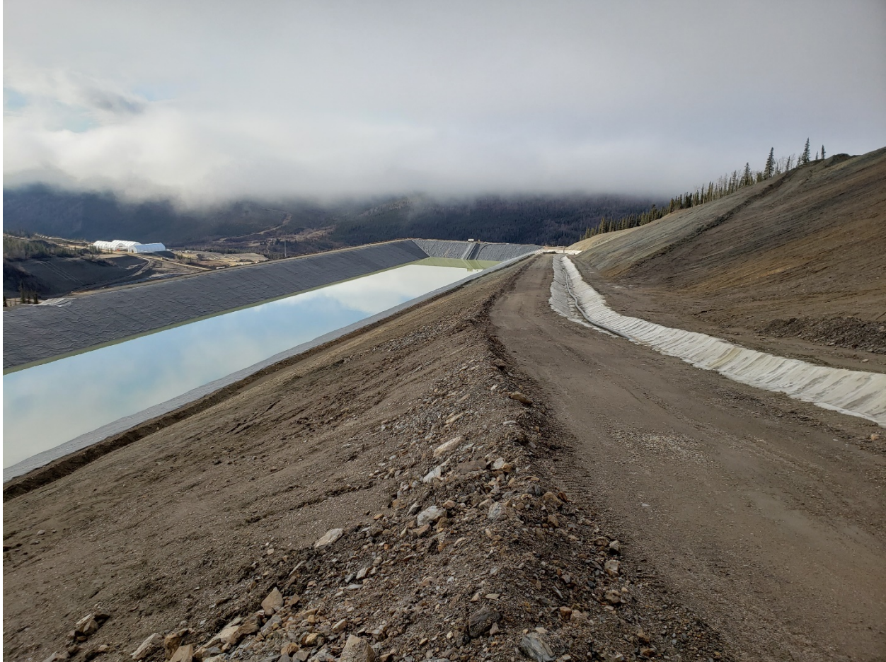
Photo 1. Event Pond and HLF spillway looking west.
