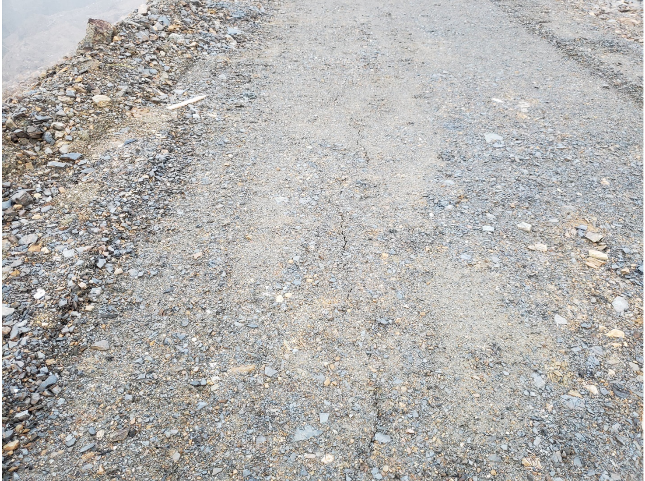
Photo 6. Event Pond south embankment crest looking west.
