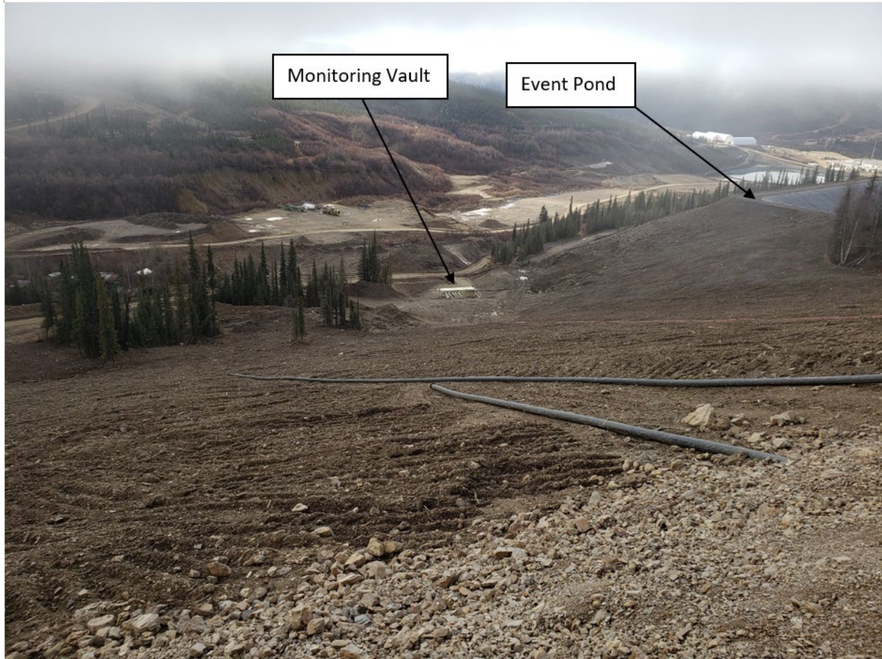
Photo 16. HLF Dam Slope looking south from crest.
