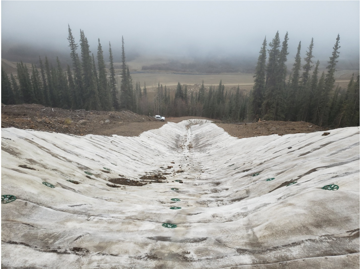
Photo 7. Event Pond Emergency spillway looking south from crest.
