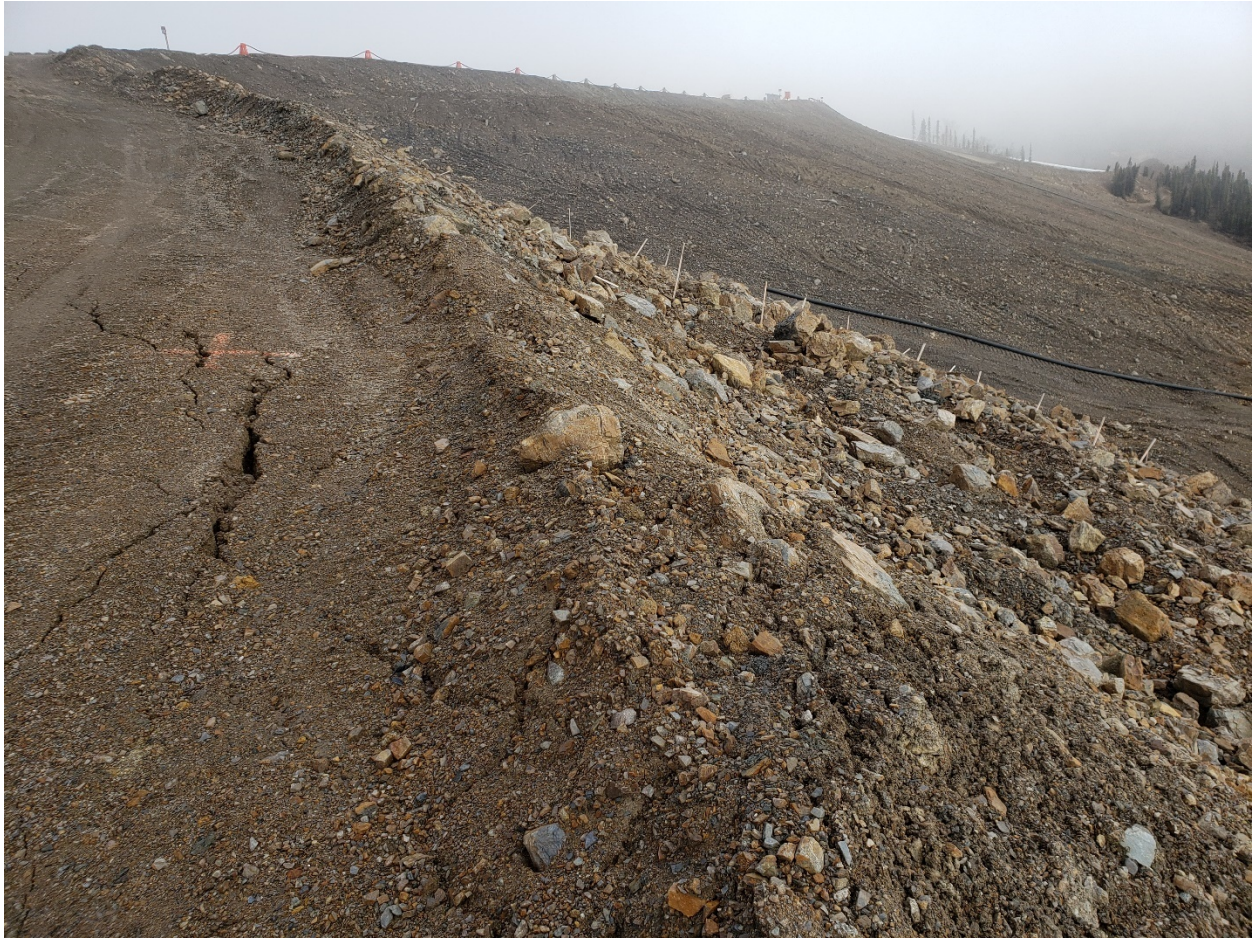
Photo 3. Upper portion of HLF spillway access road.
