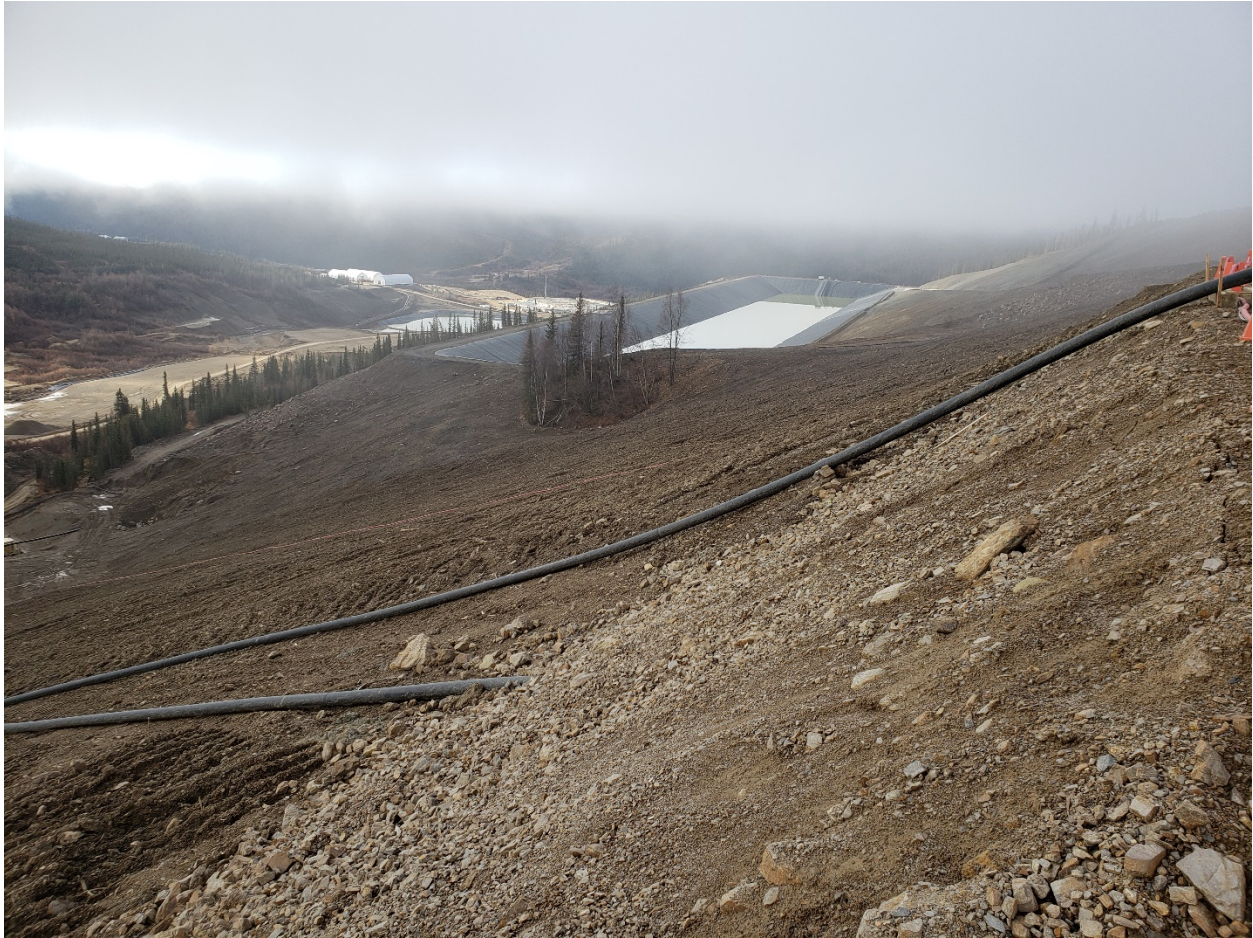
Photo 14. HLF Dam Slope looking west from crest.
