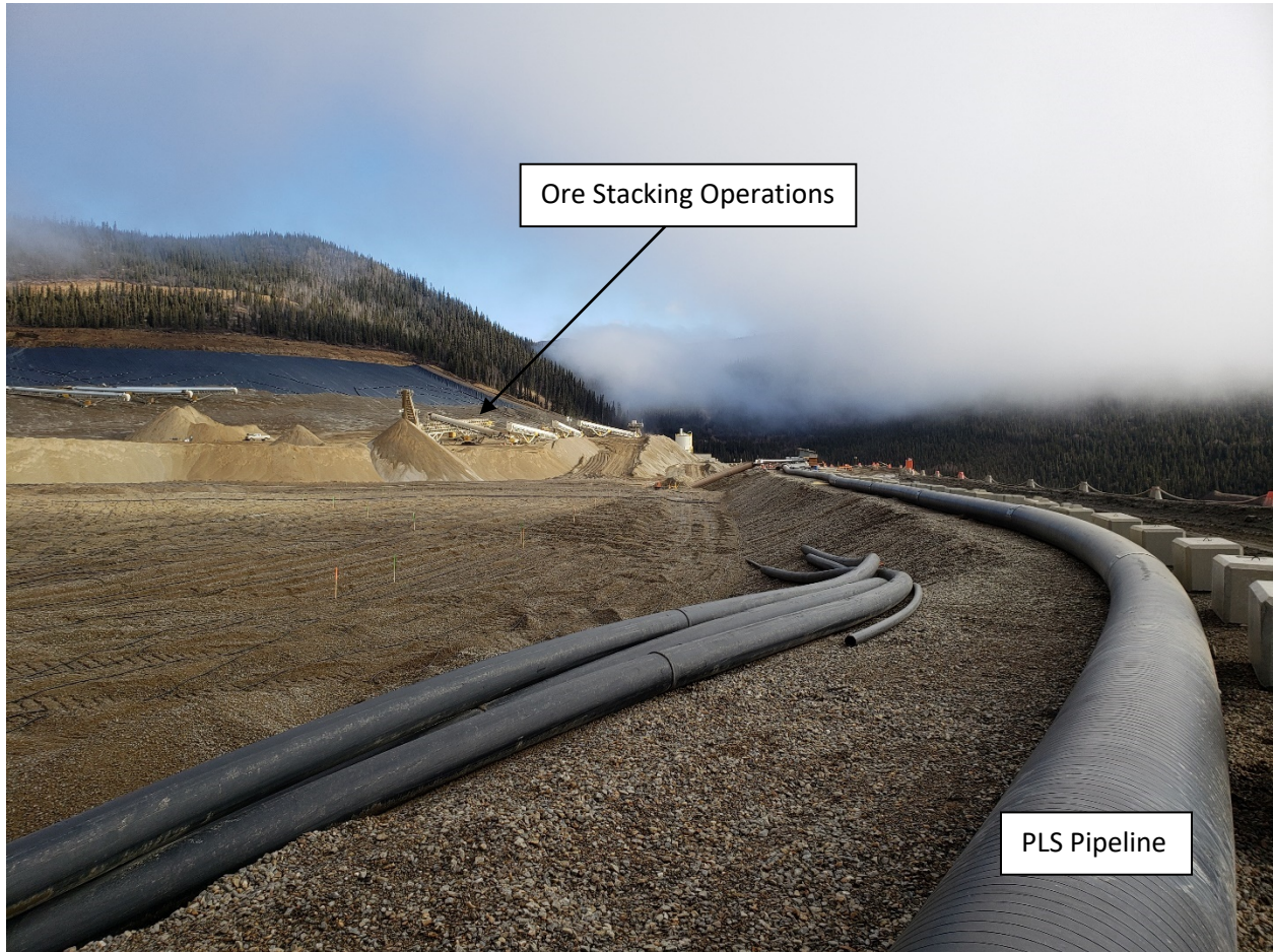
Photo 19. HLF Phase 1 Pad looking east from dam crest.
