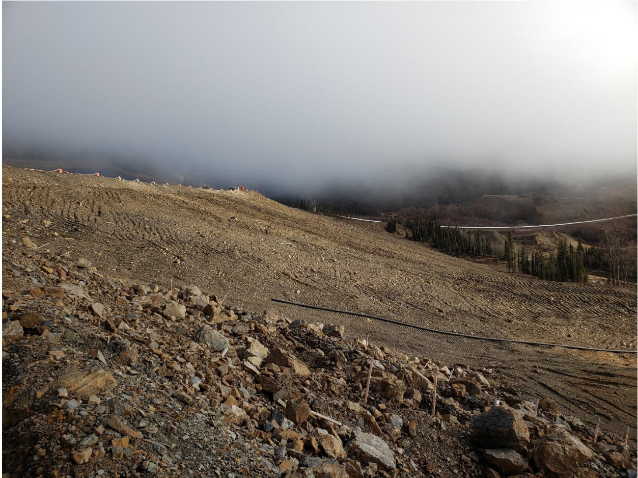
Photo 18. HLF Dam Slope looking east from spillway access road.
