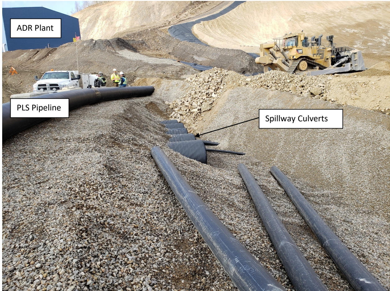
Photo 21. HLF Spillway culverts looking west from dam crest.
