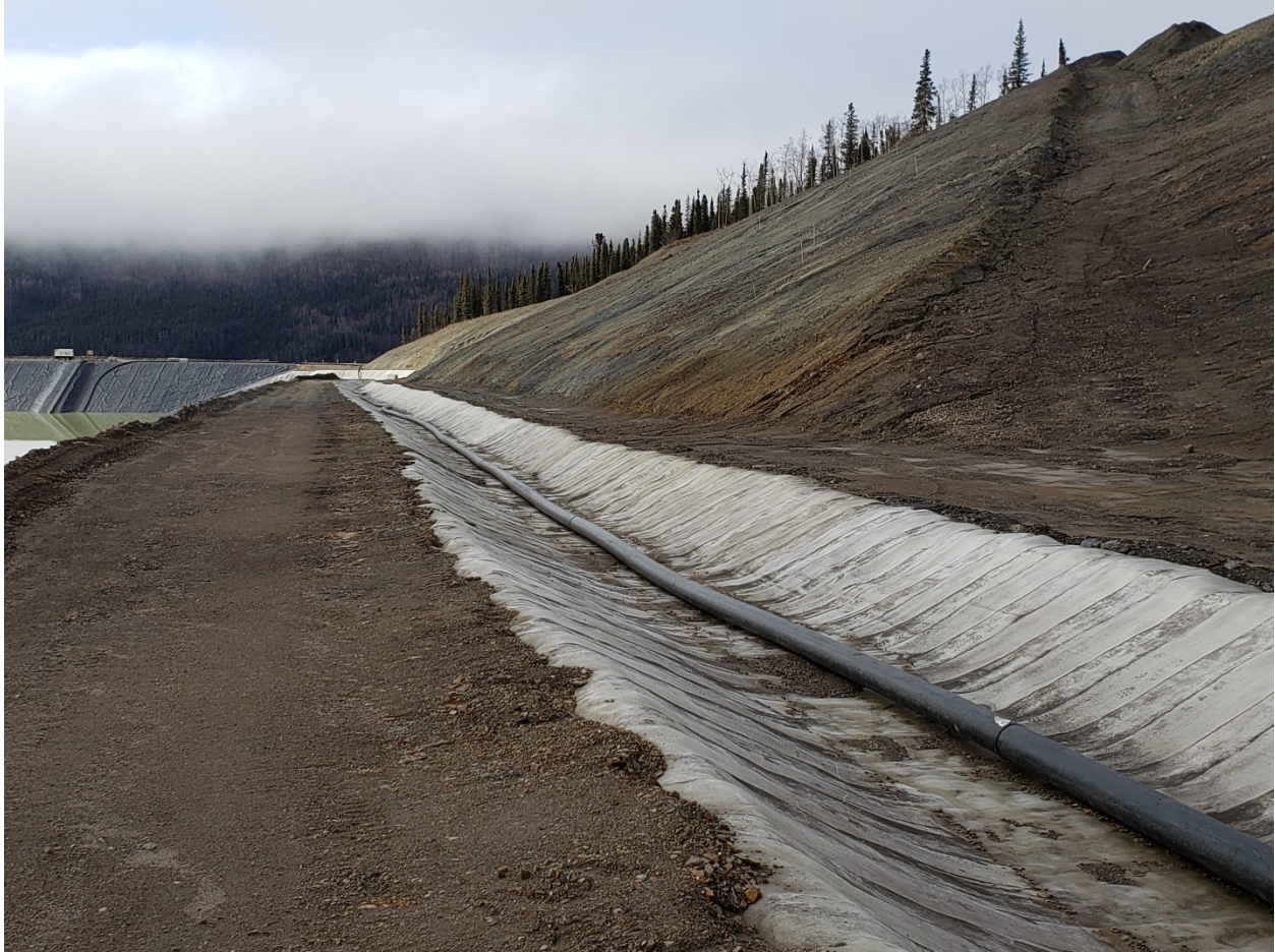
Photo 4. Upper portion of HLF spillway looking west.
