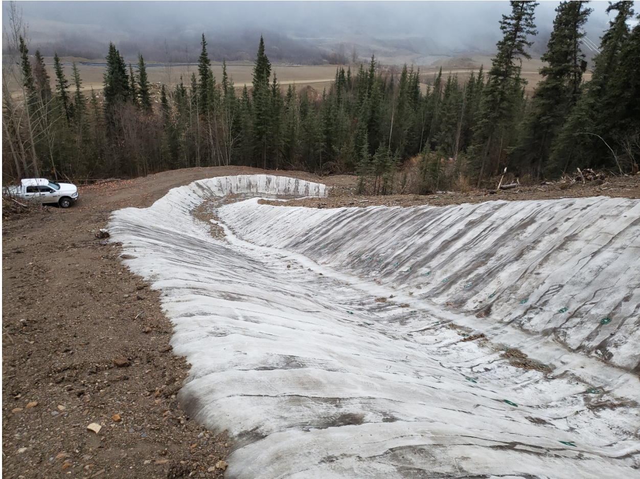
Photo 9. Bottom portion of Event Pond Emergency spillway looking south.
