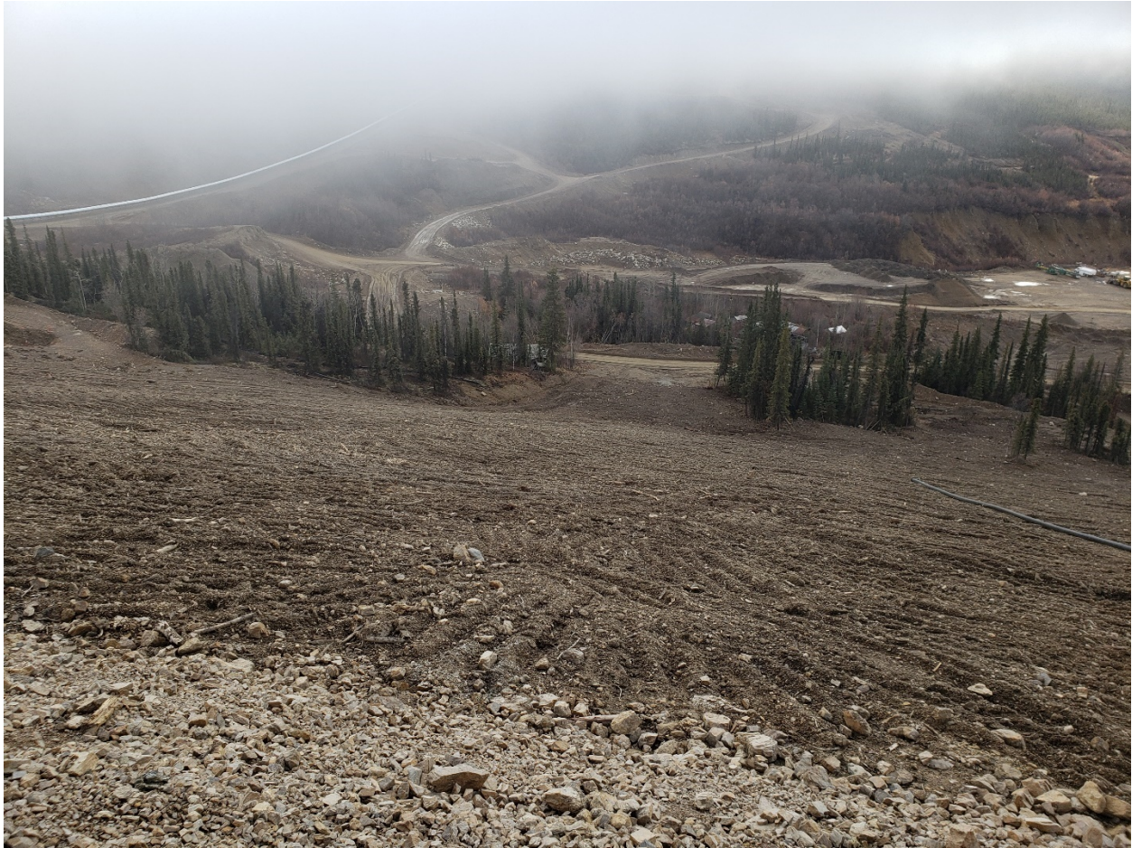
Photo 17. HLF Dam Slope looking south from crest.
