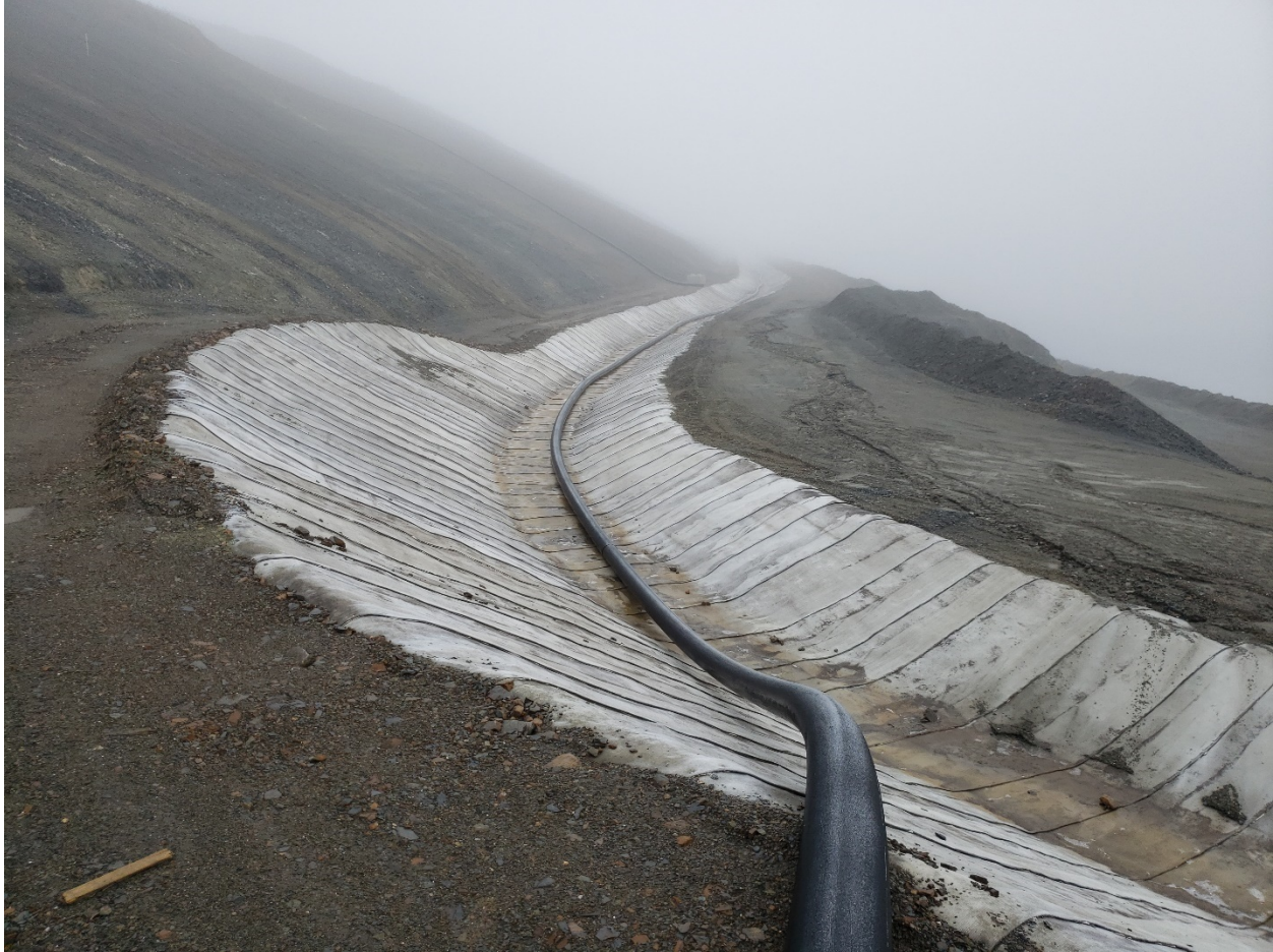
Photo 5. Bottom portion of HLF spillway looking east.
