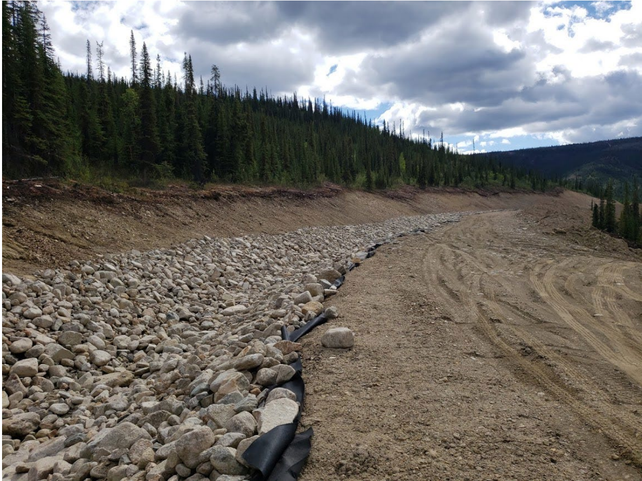
Photo 22. HLF Phase 1 interceptor ditch looking east.
