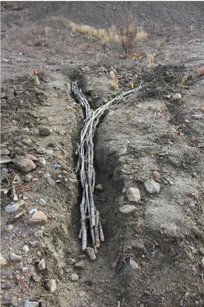
Photo #3: Y pole drain prior to burial.
