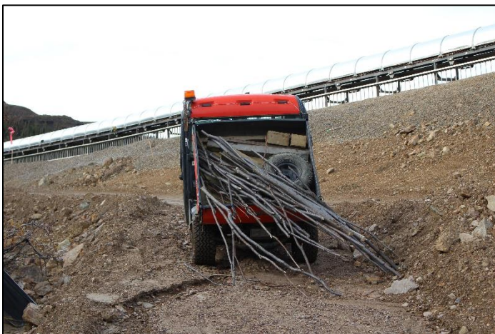
Photo #9: Staging willows at Site #5.
