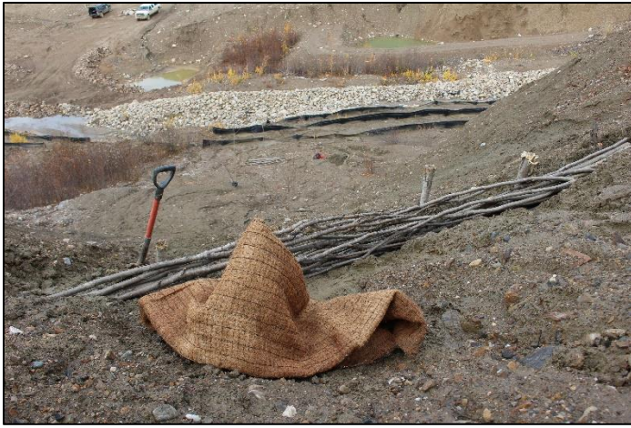
Photo #5: wattle fence prior to coco mat installation
