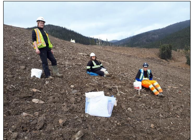
Photo #10: Seeding the heap leach embankment
