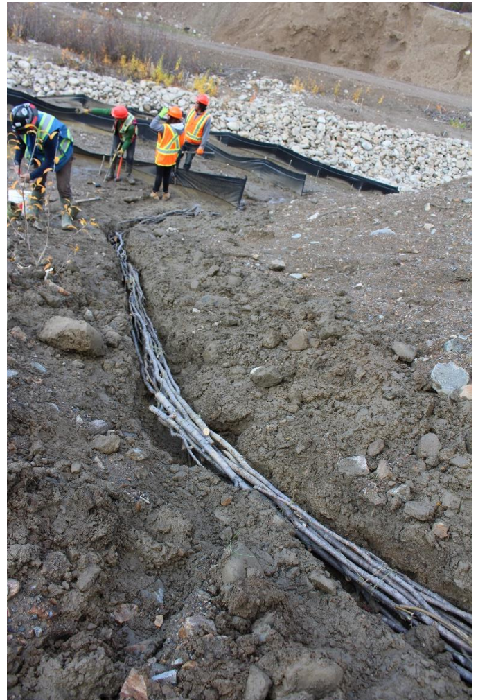
Photo #4: long pole drain prior to burial.
