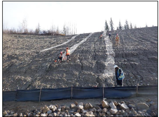
Photo #8: laying down the jute mats on the cutbank
