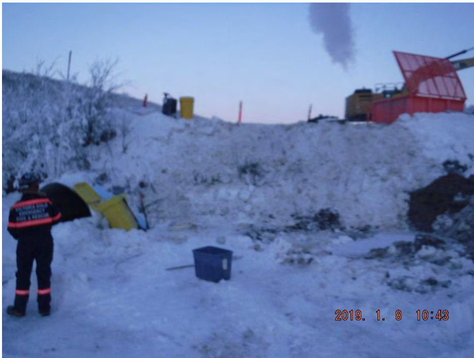
Photo 3-8: Recovery of Contaminated Materials - January 8, 2019
