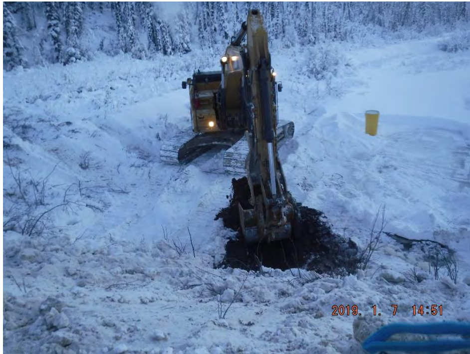
Photo 3-4: Excavation of Contaminated Material - January 7, 2019
