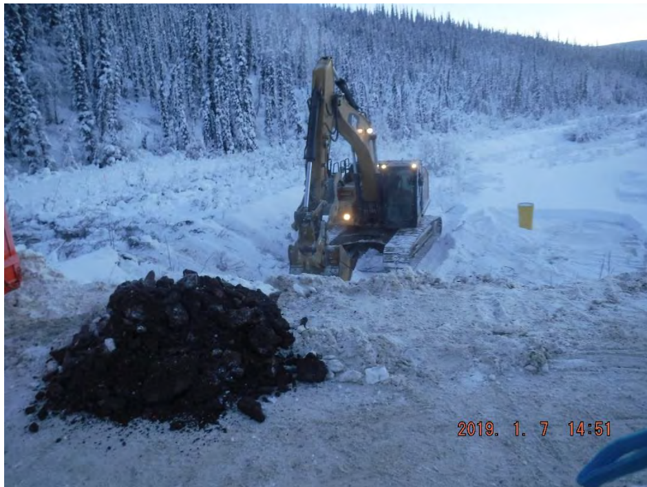
Photo 3-5: Excavation of Contaminated Material - January 7, 2019
