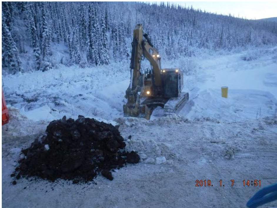
Photo 3-5: Excavation of Contaminated Material - January 7, 2019
