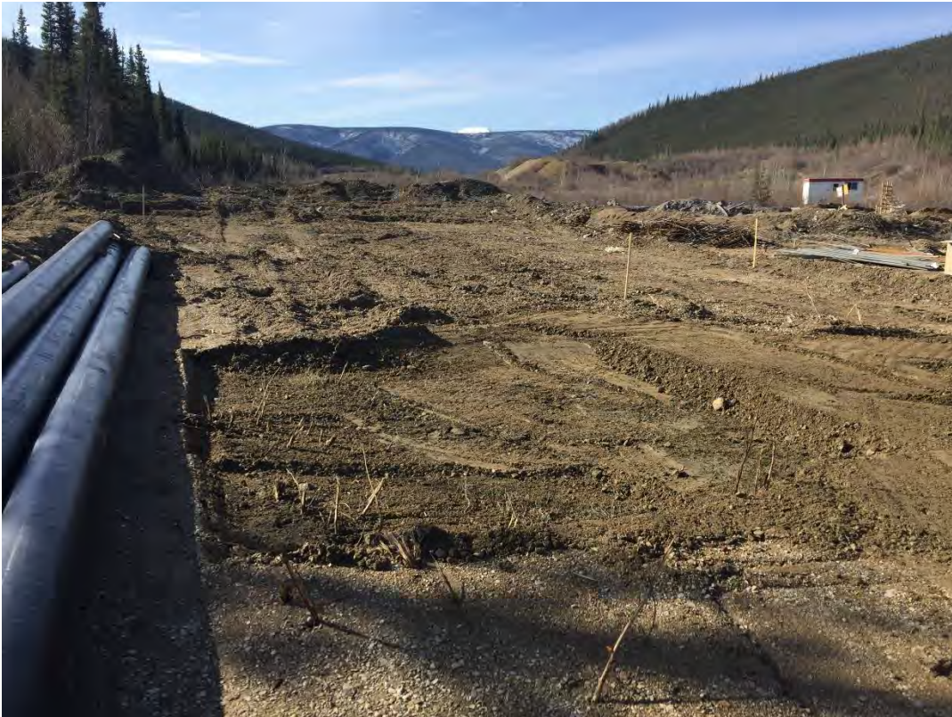
Photo 3-2: May 12, additional sampling of Staging 6 area after additional excavation.
