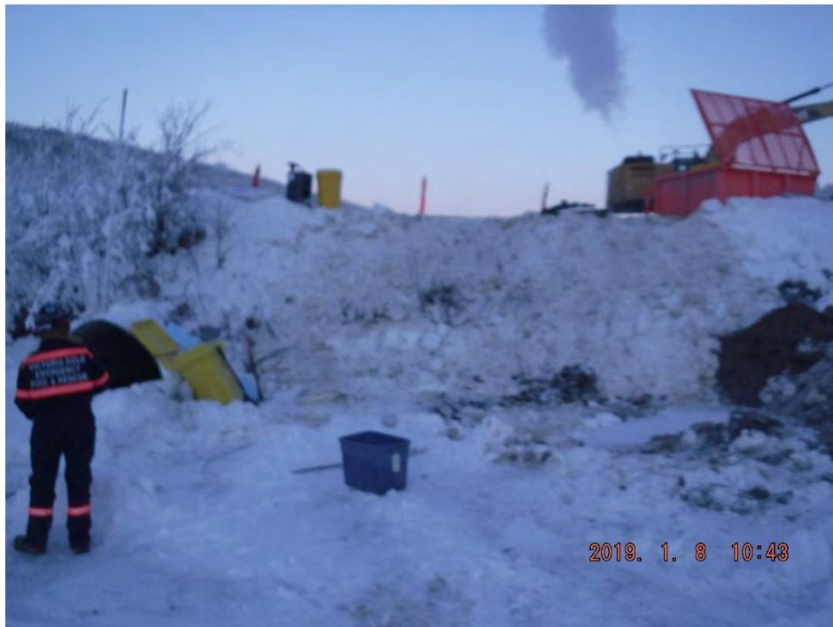
Photo 3-8: Recovery of Contaminated Materials - January 8, 2019
