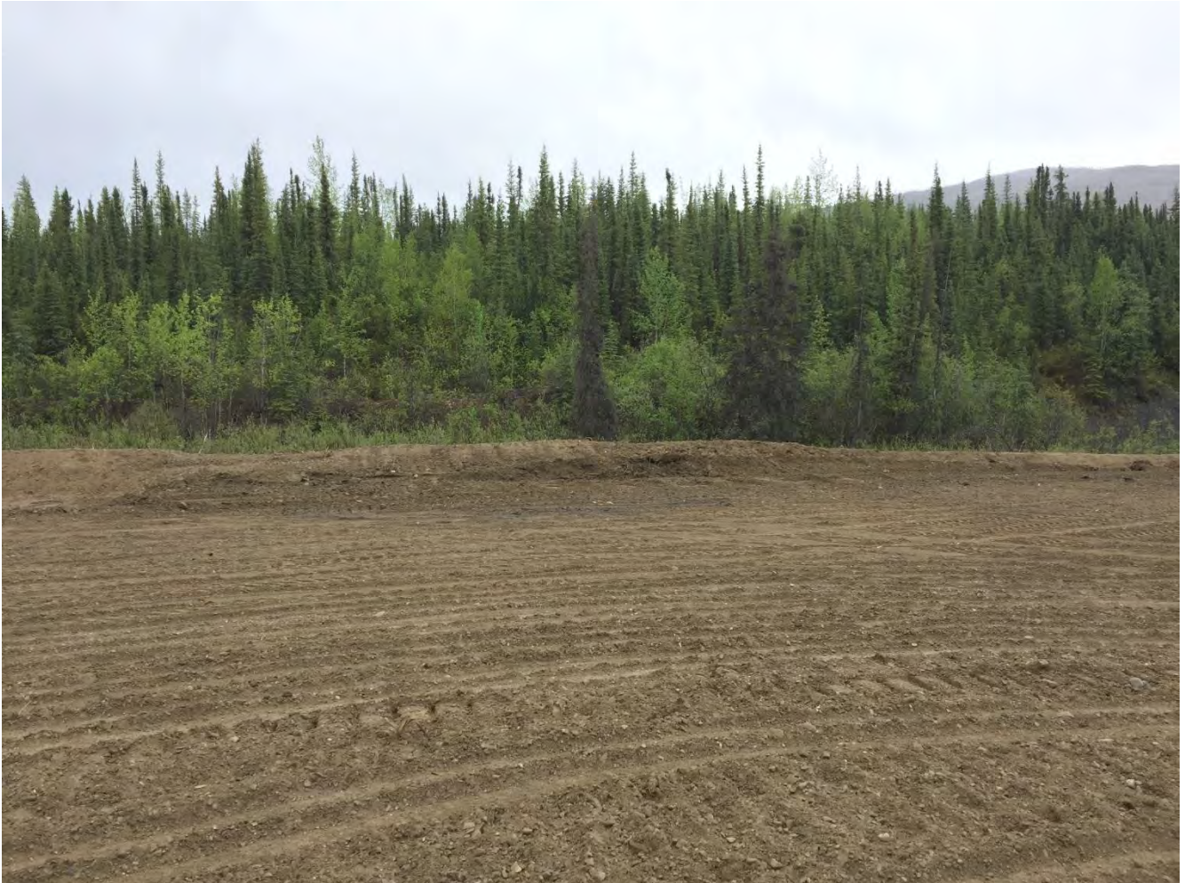
Photo 3-4: May 30, Previous location of Temporary Berm, re-contoured
