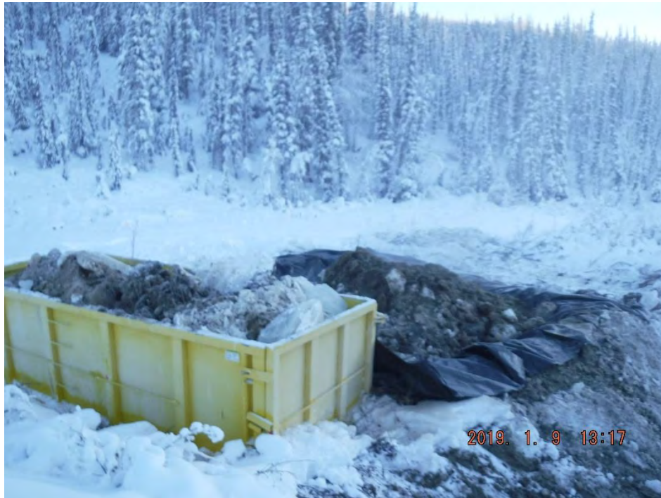
Photo 3-12: Temporary Lined Sump - January 9, 2019
