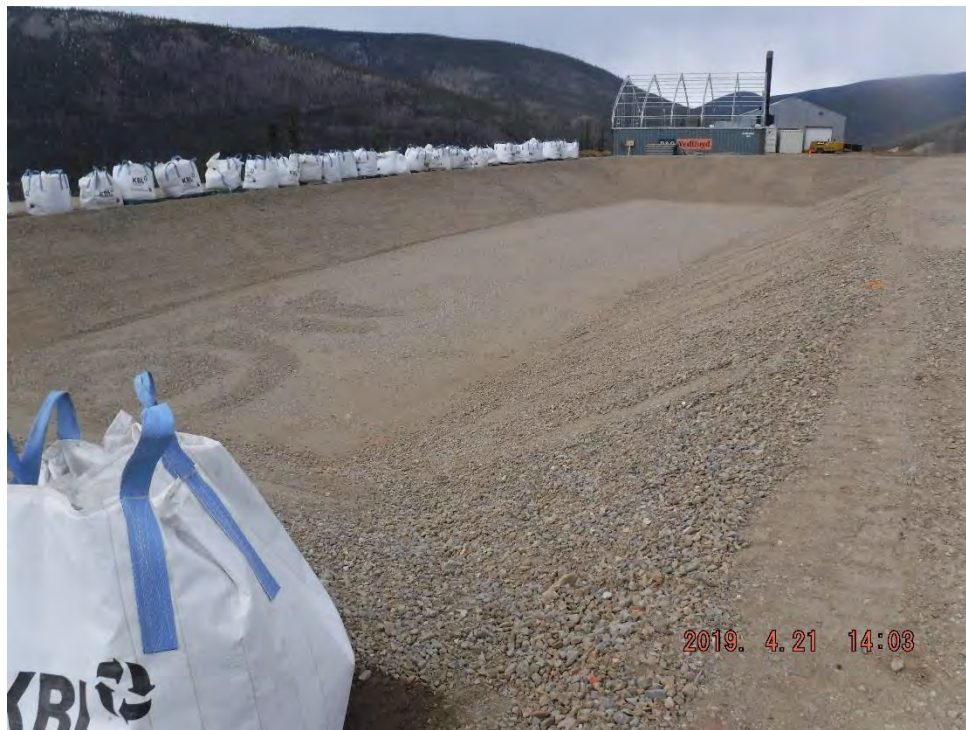
Photo 2-3: Super Sacks Staged for Placement in LTF
