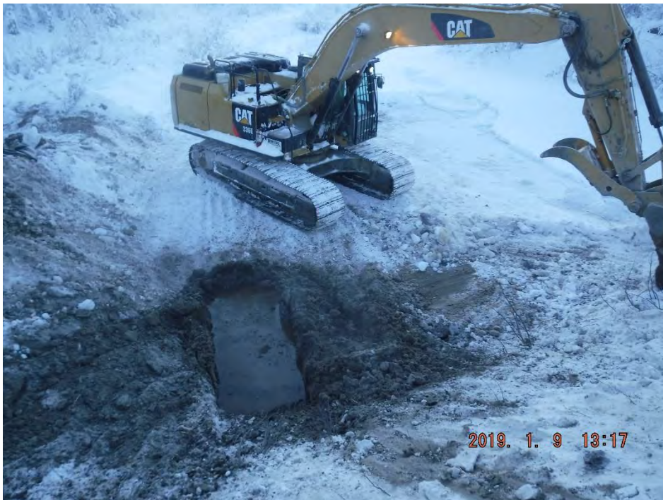
Photo 3-11: Recovery of Contaminated Materials - January 9, 2019
