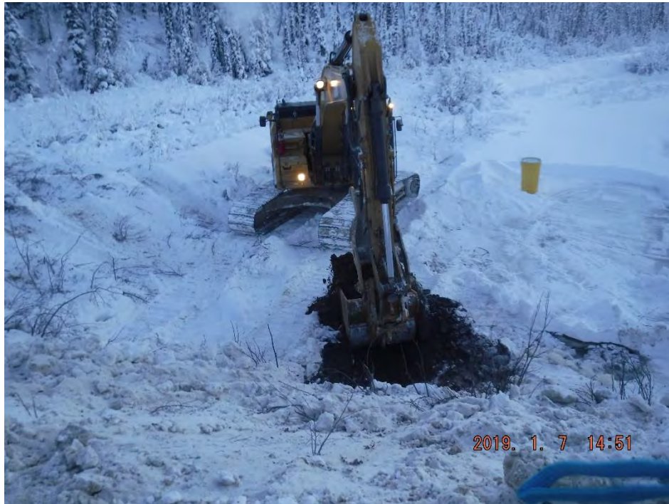
Photo 3-4: Excavation of Contaminated Material - January 7, 2019
