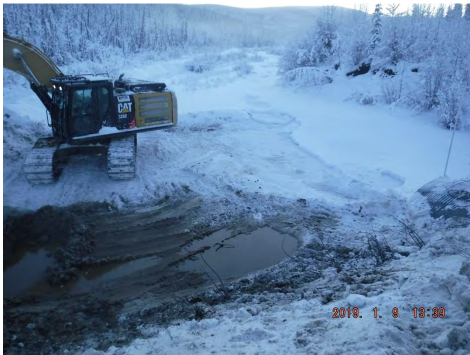
Photo 3-13: Recovery of Contaminated Materials and Seepage Water - January 9, 2019
