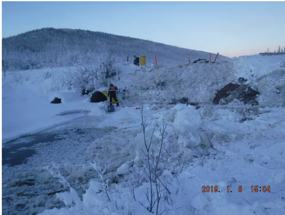
Photo 3-9: Recovery of Contaminated Materials - January 8, 2019
