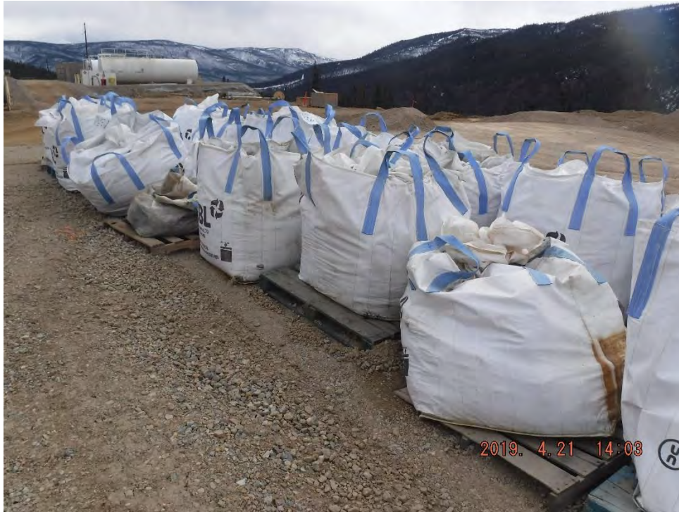
Photo 2-4: Super Sacks Staged for Placement in LTF
