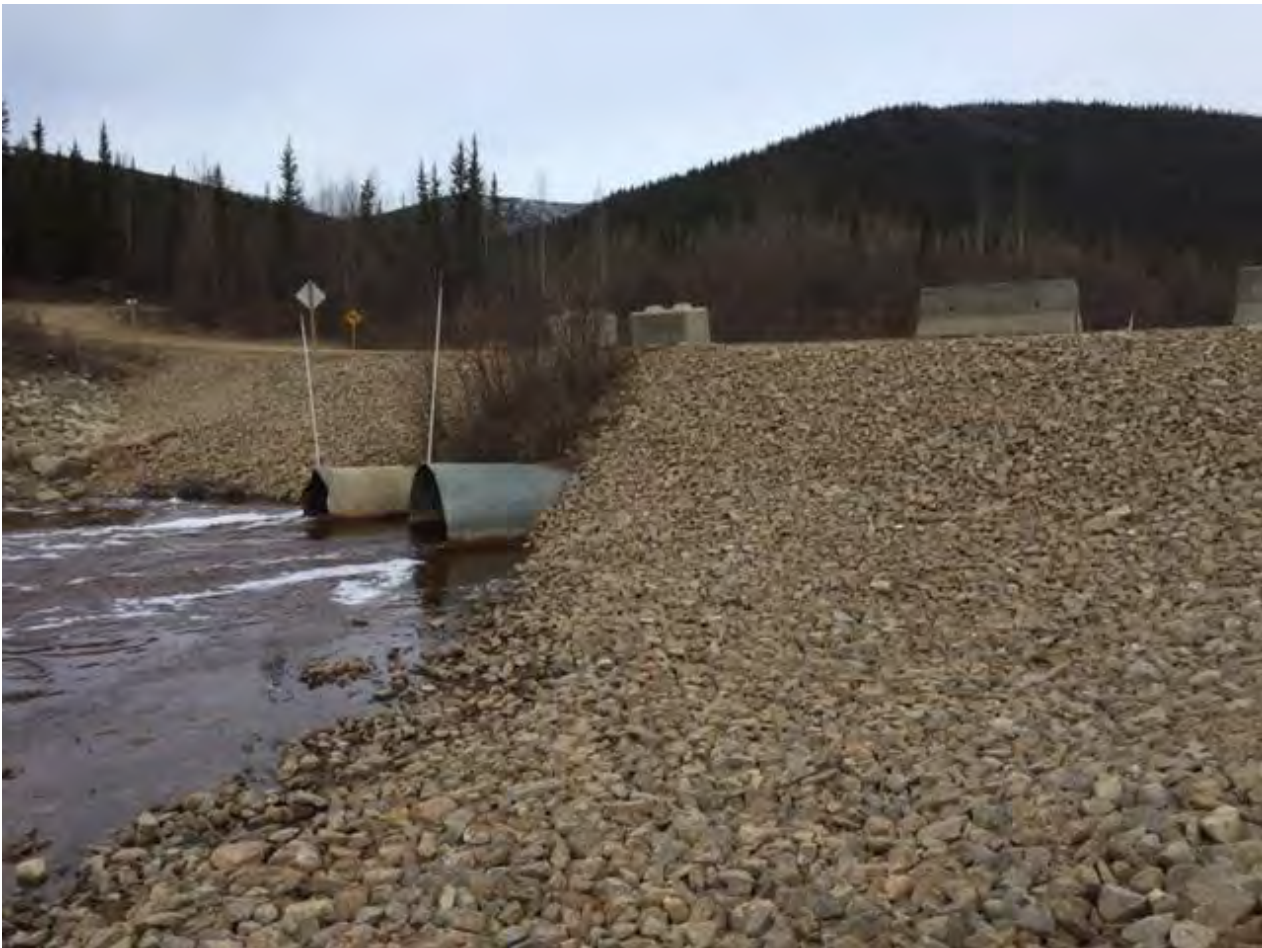
Photo 3-1: Site Stabilization with Rip Rap - May 10, 2019
