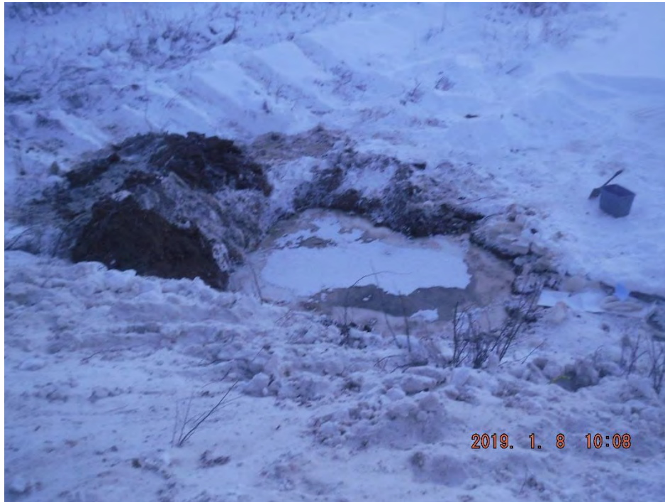
Photo 3-6: Excavation of Ice - January 8, 2019
