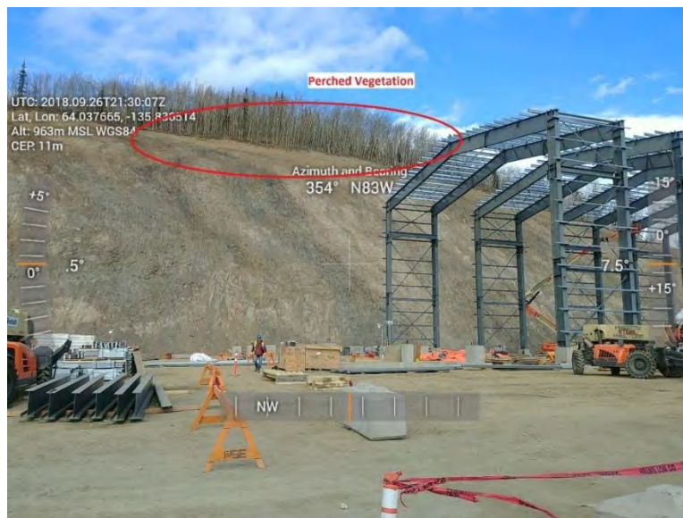
Figure 37: Slopes behind ADR (2018)
