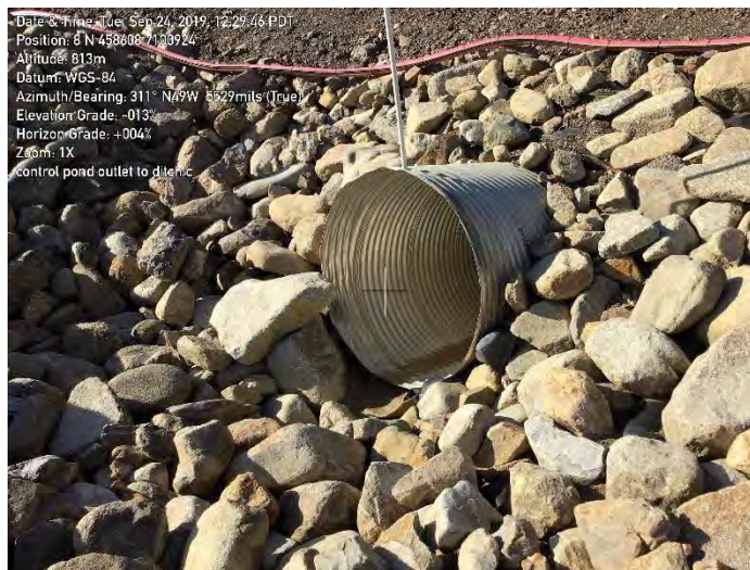
Figure 4: LDSP - 1500mm Culvert 2019 Inspection
