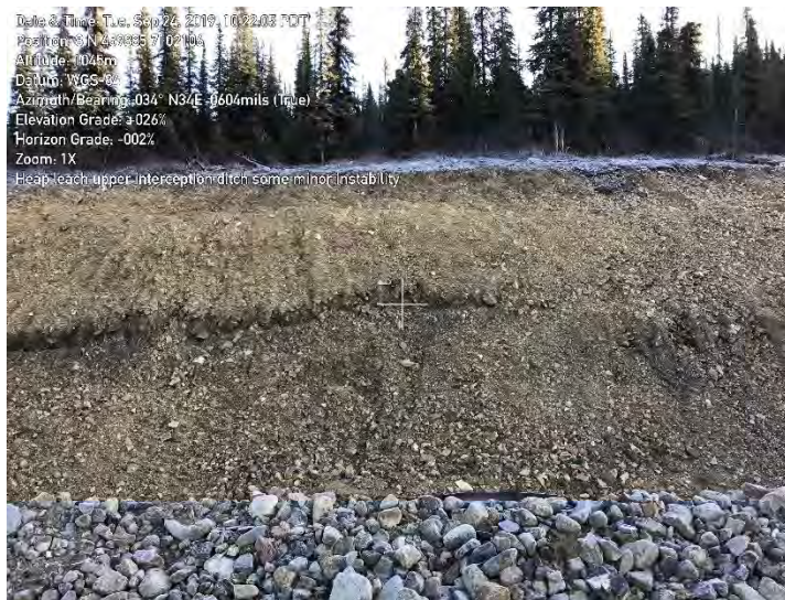
Figure 21: Sloughing slope
