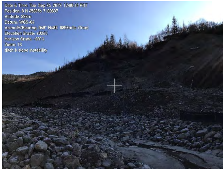
Figure 51: Silt fencing constructed in areas of erosion on cut slopes
