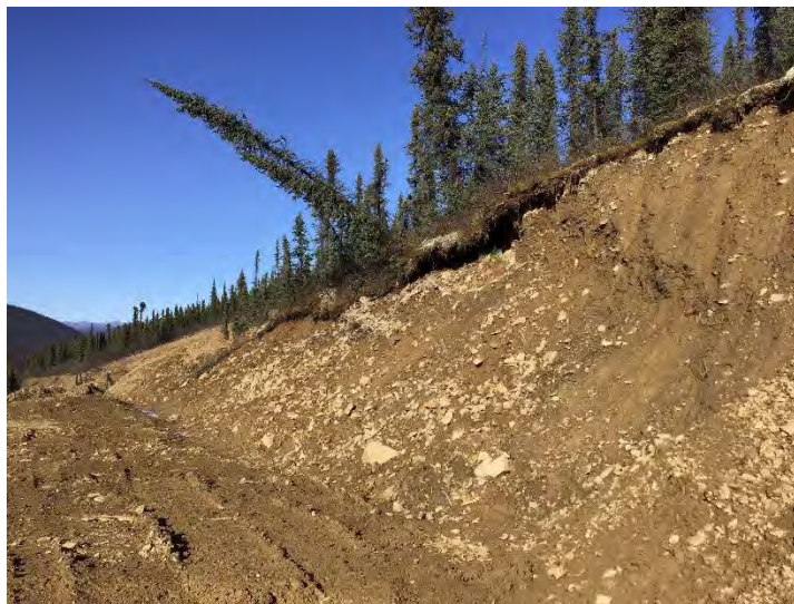
Figure 56: Section of over-steepened slope
