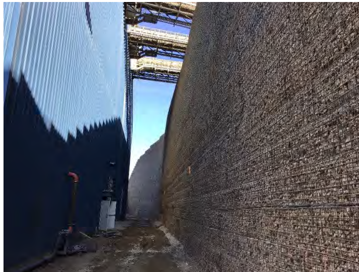
Figure 35: MSE wall behind secondary/tertiary crusher
