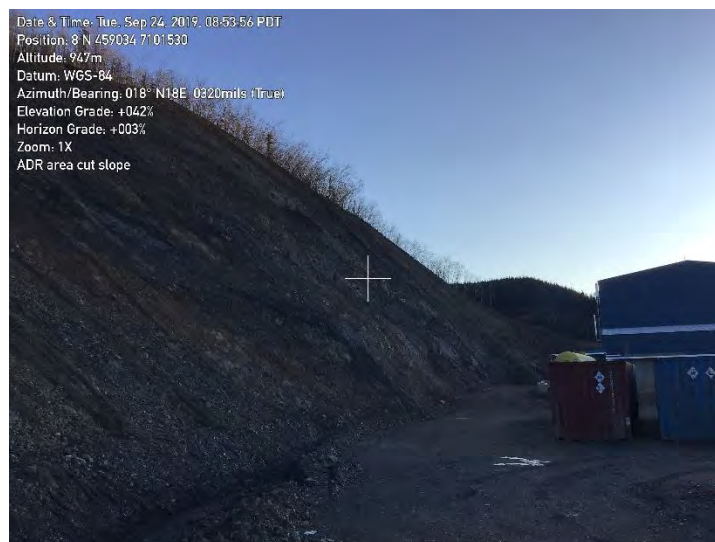
Figure 36: Slopes behind ADR (2019)
