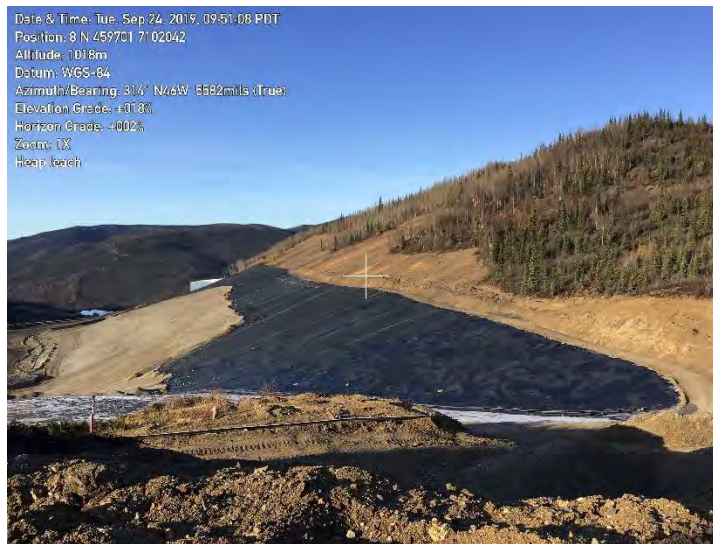
Figure 15: Some erosion/sloughing on slopes above the existing HLF pad
