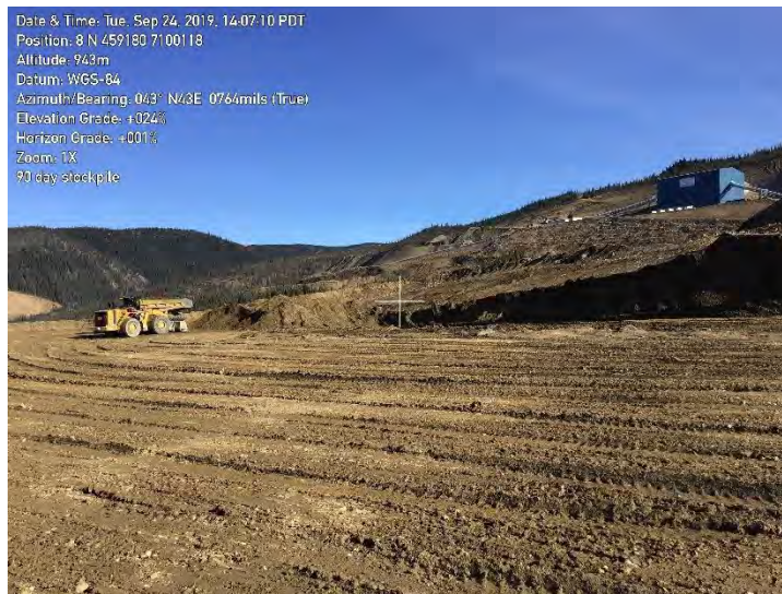
Figure 7: 90 Day Stockpile under construction
