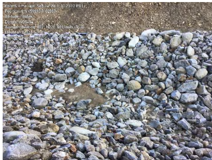
Figure 22: Material deposited into ditch
