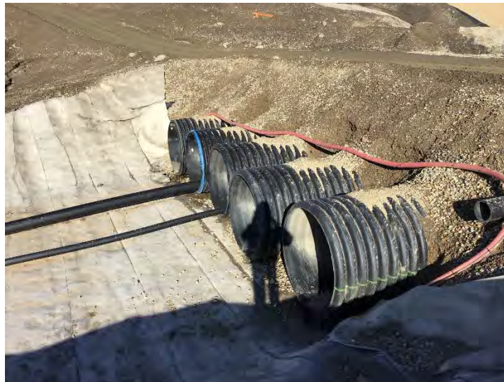
Figure 44: Culverts installed under HLF embankment access road crossing
