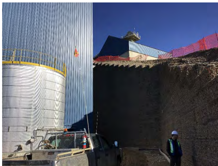
Figure 34: South side of MSE wall
