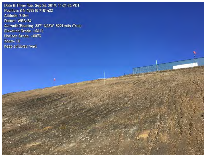
Figure 41: Slopes from heap leach spillway
