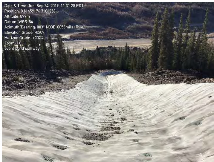
Figure 45: Events Pond Emergency spillway
