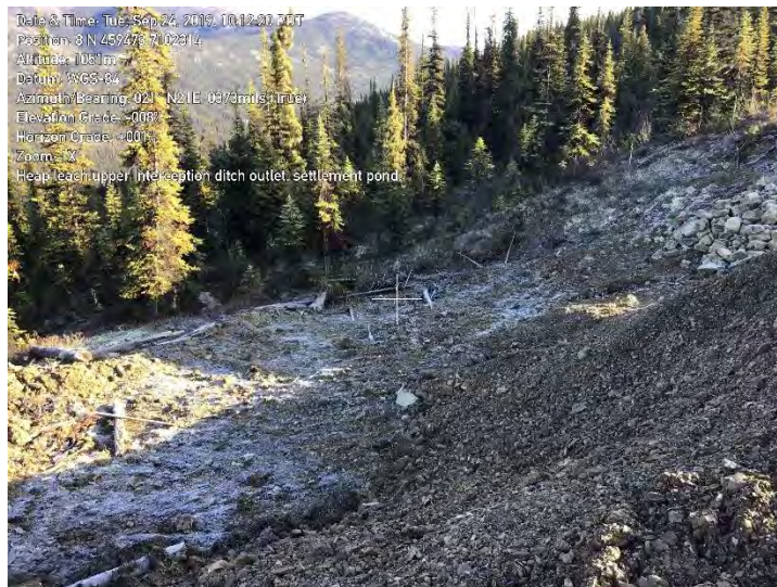
Figure 20: Outlet of HLF Phase 1 Interceptor Ditch
