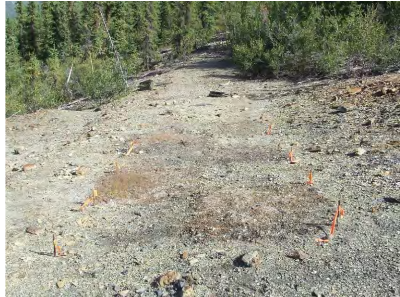
Photo #70: Waste Rock, Block #3, August 2014.
