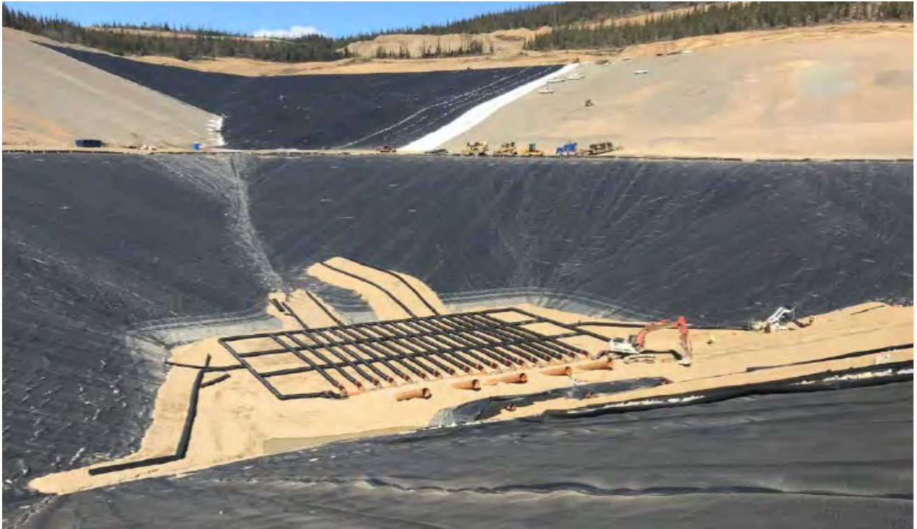
Photo 2.1-21: HLF PLS Piping Installation - May 10, 2019
