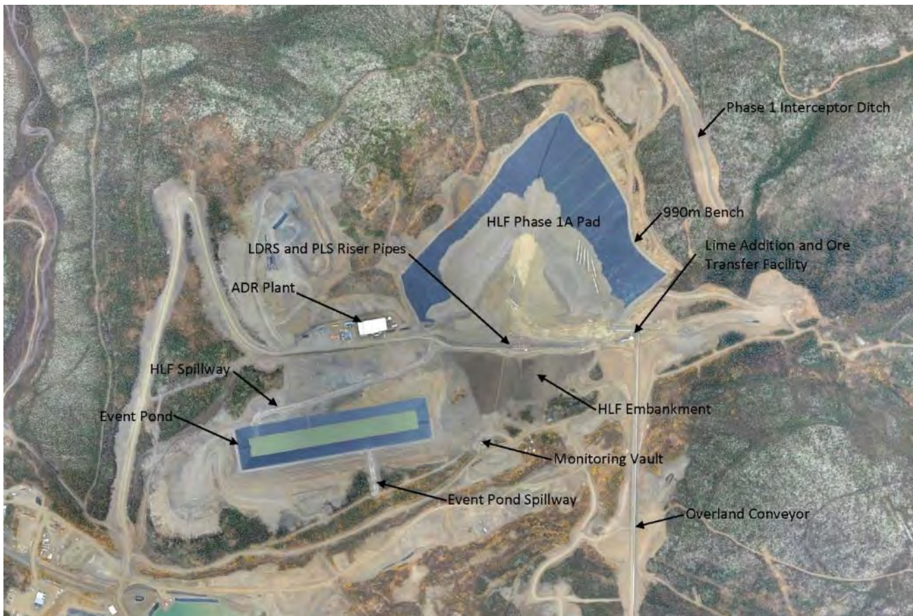
Figure 4.3-1: Drone Photo Map of HLF and Process Facilities - September 16, 2019
