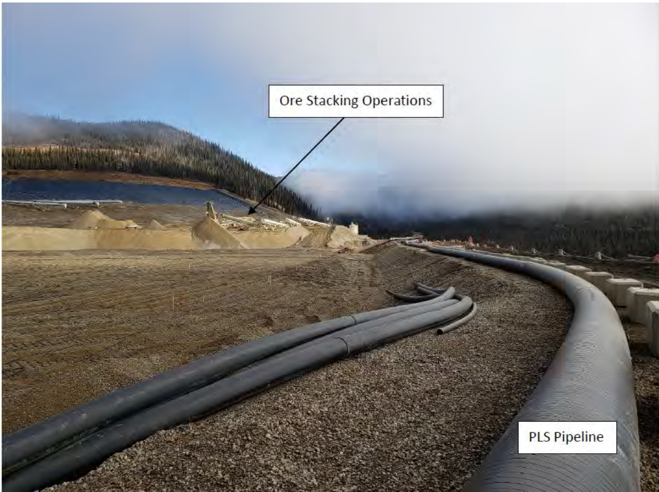
Photo 4.3-3: HLF Phase 1 Pad Looking East from Dam Crest
