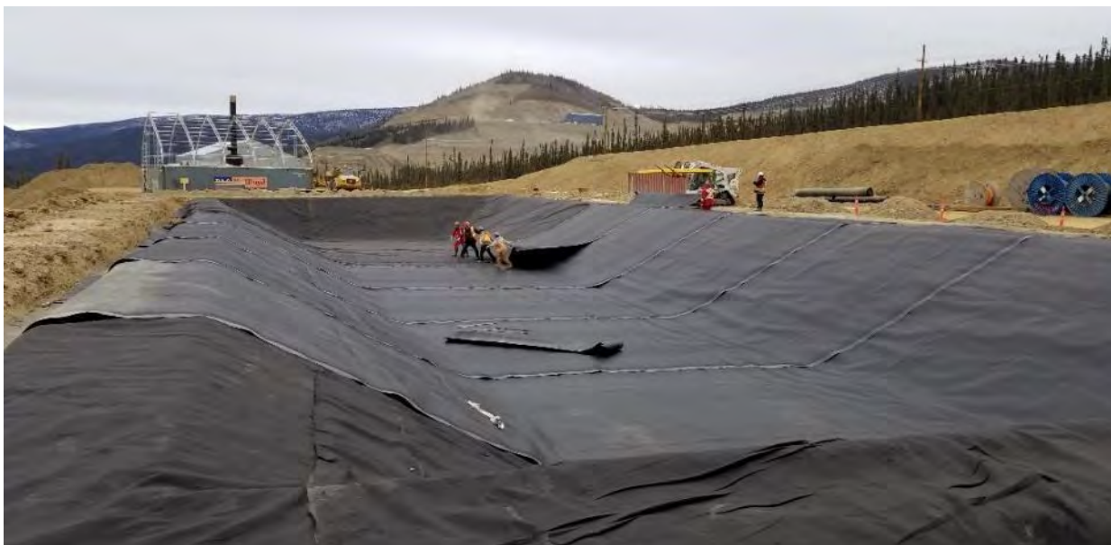
Photo 2.1-26: Land Treatment Facility Liner Installation - April 6, 2019
