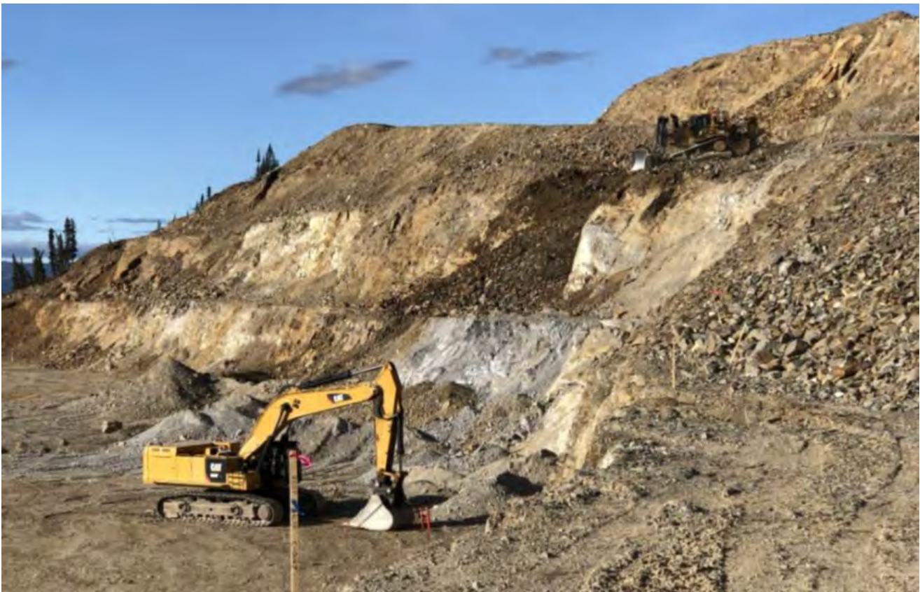
Photo 4.1-2: Remediation Activities on Localized Wedge Failures on the 1275 and 1285 Benches - June 18, 2019
