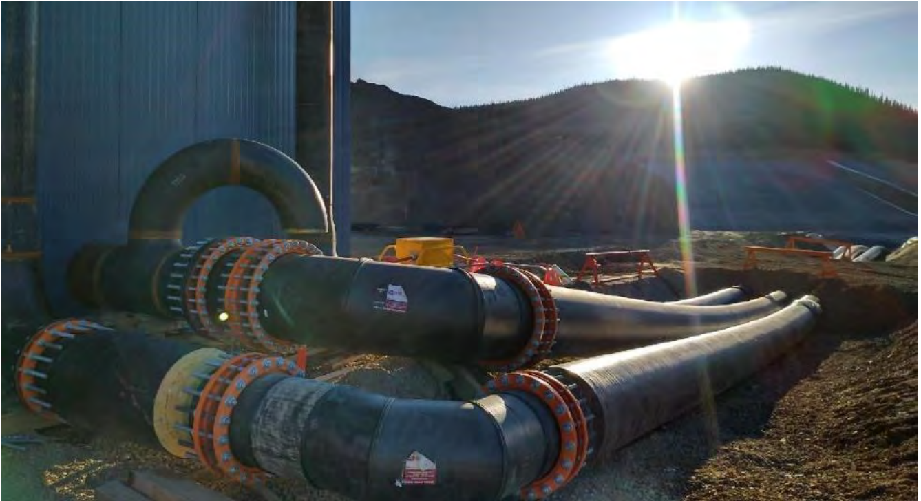
Photo 2.1-6: ADR to HLF Pipe Installation - May 28, 2019
