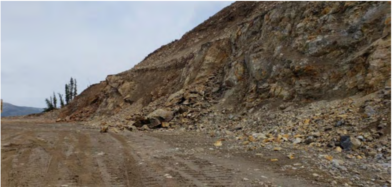
Photo 4.1-1: Localized Wedge Failures on the 1285 Bench - June 9, 2019
