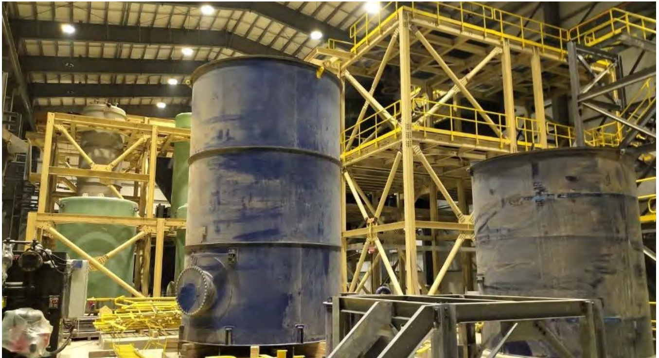
Photo 2.1-4: ADR Steel Erection - January 15, 2019
