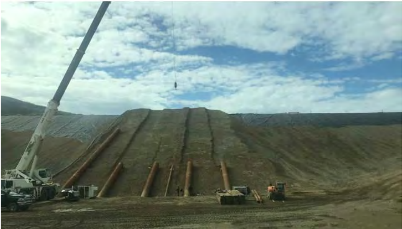
Photo 4.3-7: PLS Steel Casings Installation - June 14, 2019
