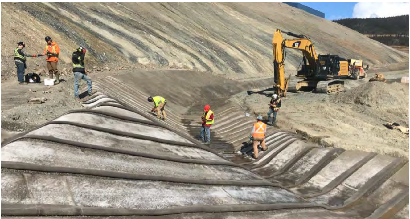
Photo 2.1-22: HLF Spillway Lining Construction - May 13, 2019
