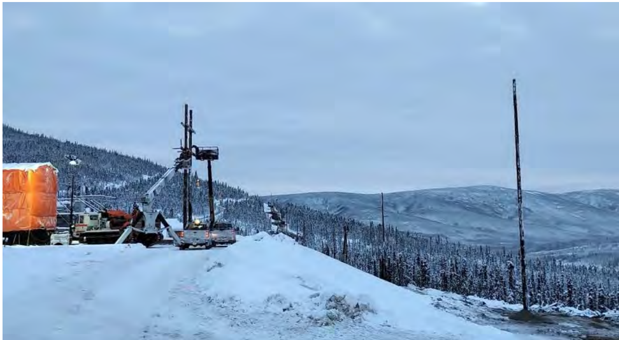
Photo 2.1-23: Powerline Installation at Project Site - January 21, 2019
