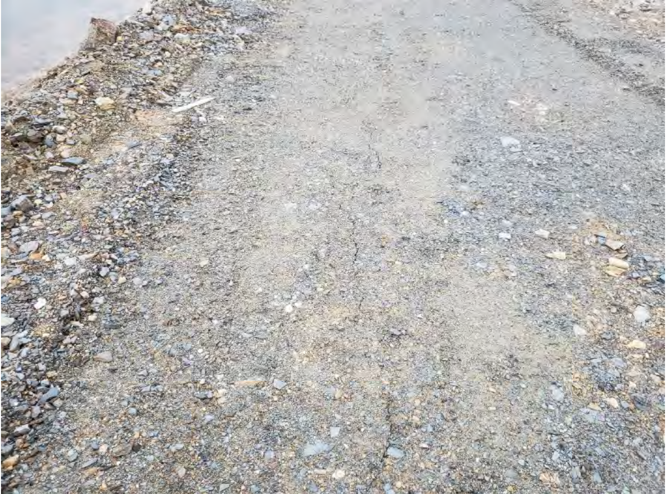
Photo 4.3-5: Event Pond South Embankment Crest Looking West
