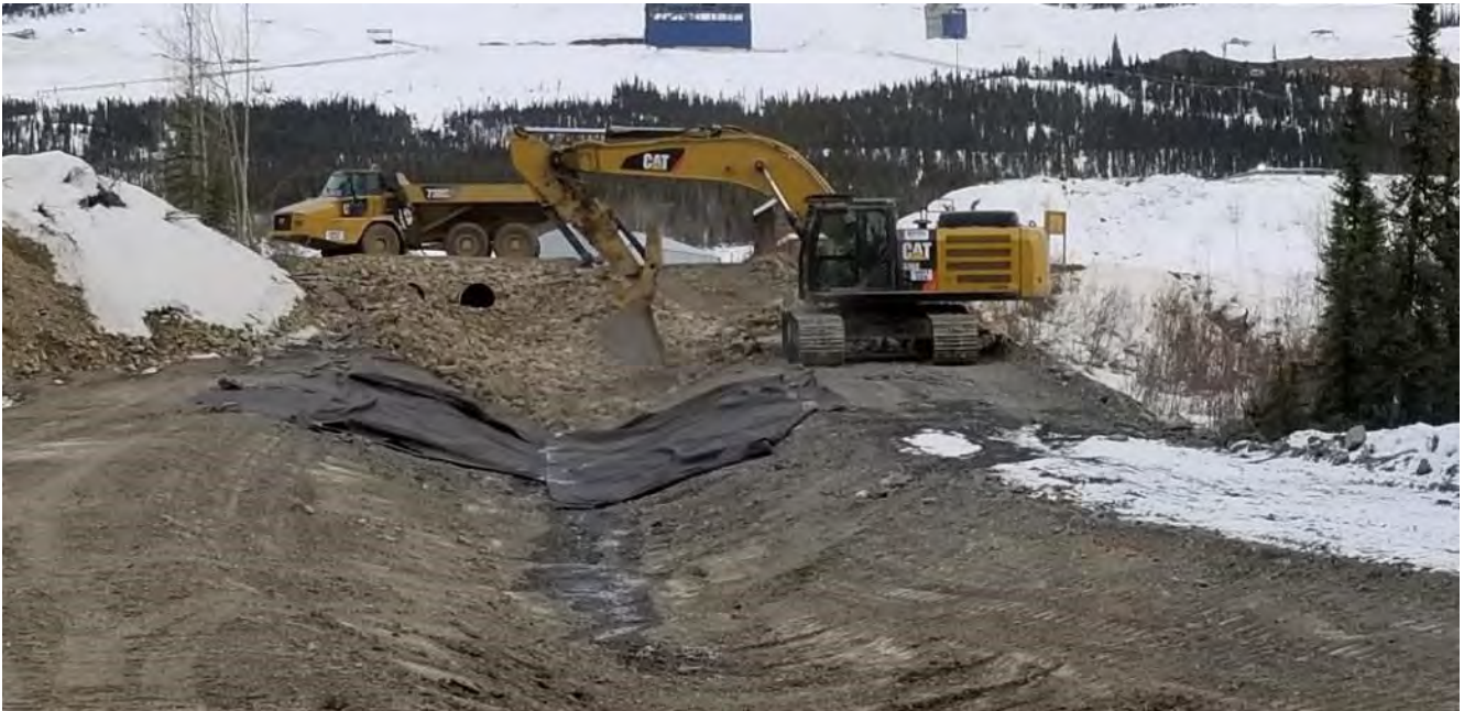
Photo 2.1-2: Ditch C Rip Rap Installation - March 17, 2019
