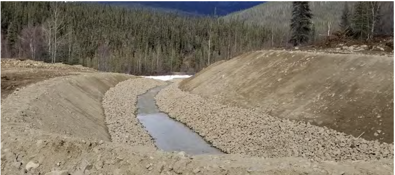
Photo 2.1-3: Ditch C Construction Complete - April 20, 2019
