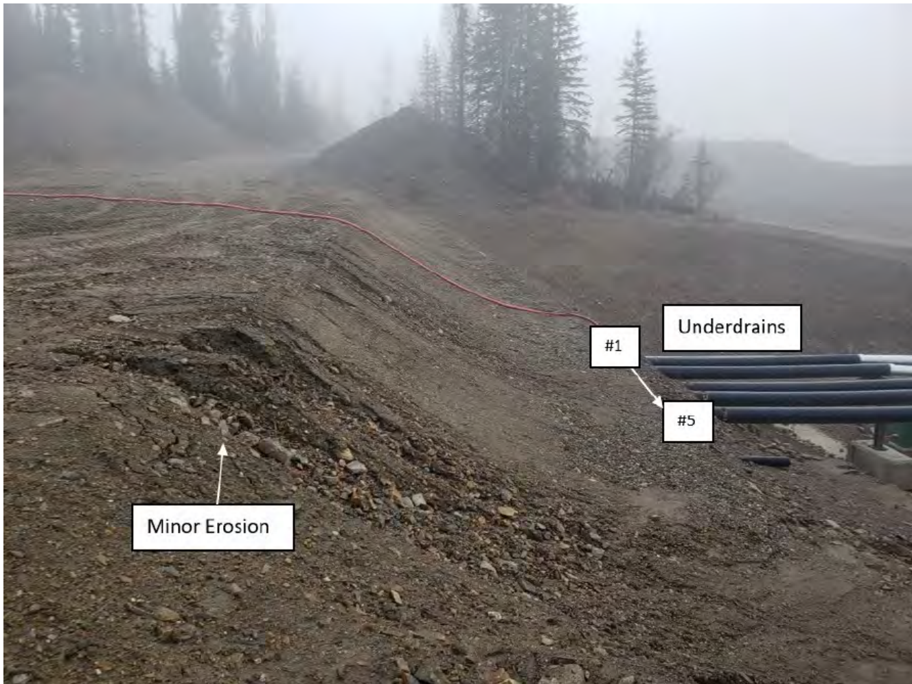
Photo 4.3-2: HLF Underdrain Outlet Between Dam and Monitoring Vault Looking East
