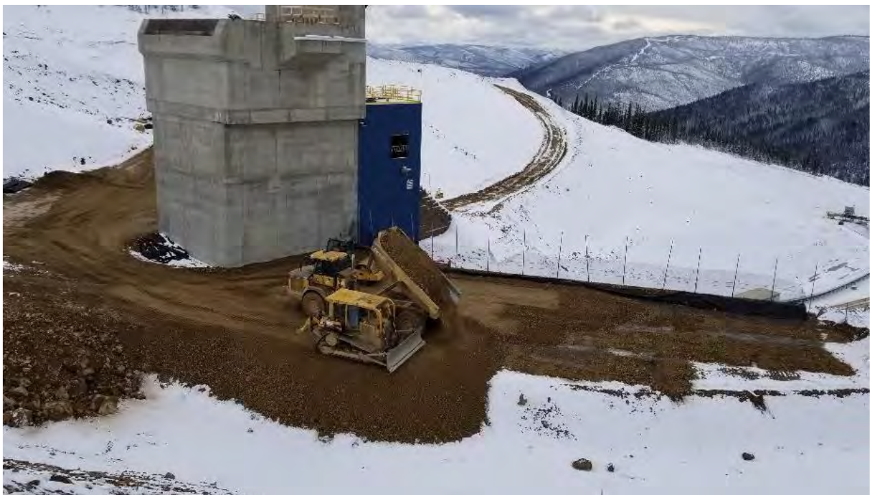
Photo 2.1-9: Primary Crusher MSE Wall Construction - April 24, 2019
