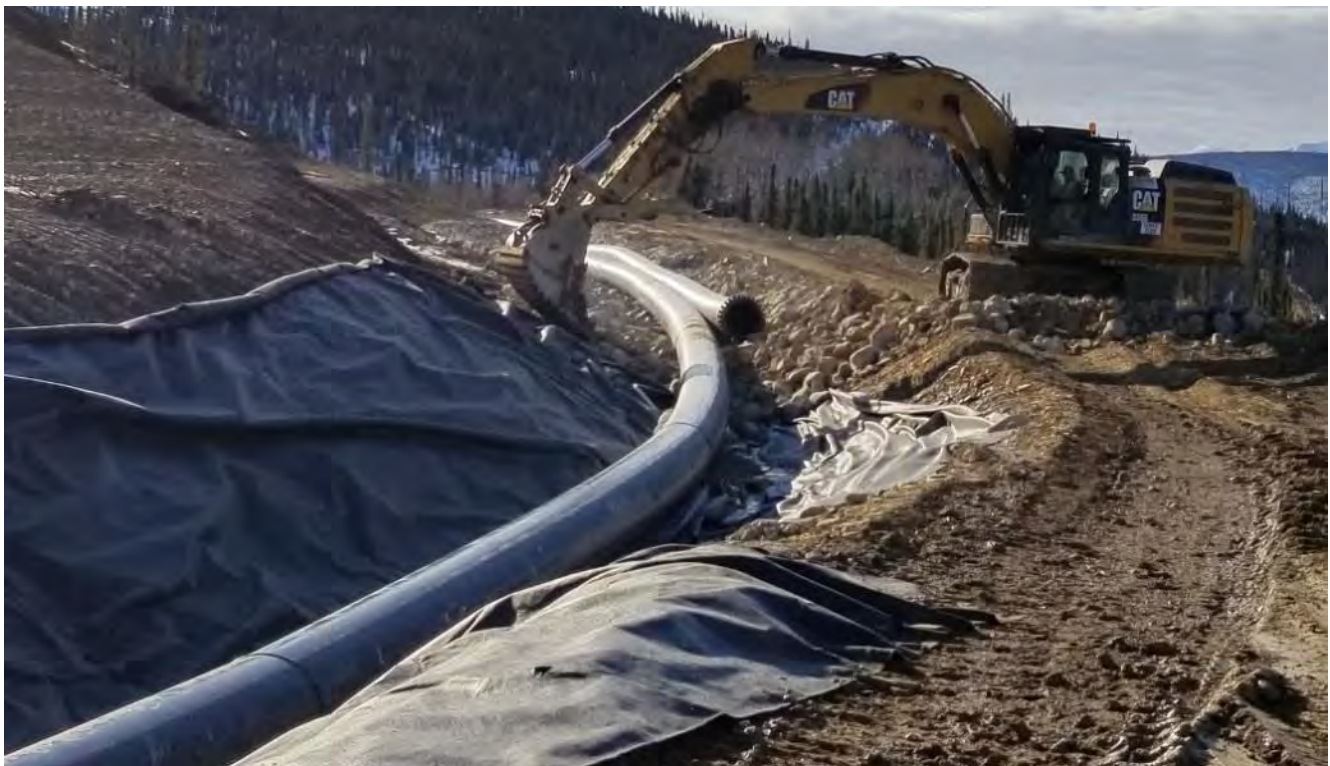
Photo 2.1-1: Ditch A Rip Rap and HDPE Pipe Installations - March 28, 2019
