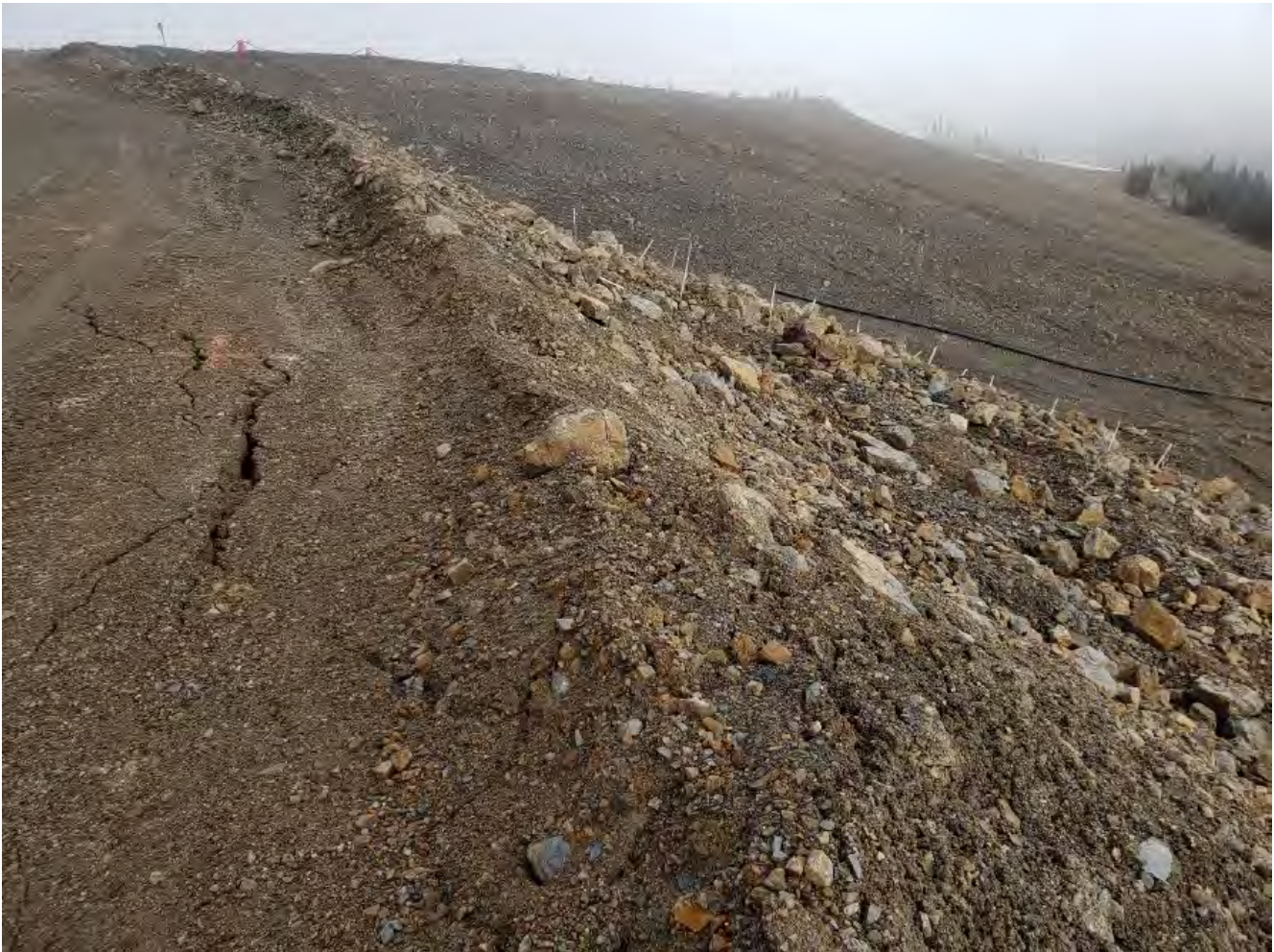
Photo 4.3-4: Upper Portion of HLF Spillway Access Road
