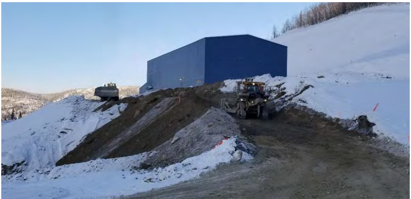
Photo 2.1-5: ADR to HLF Road Construction - February 19, 2019
