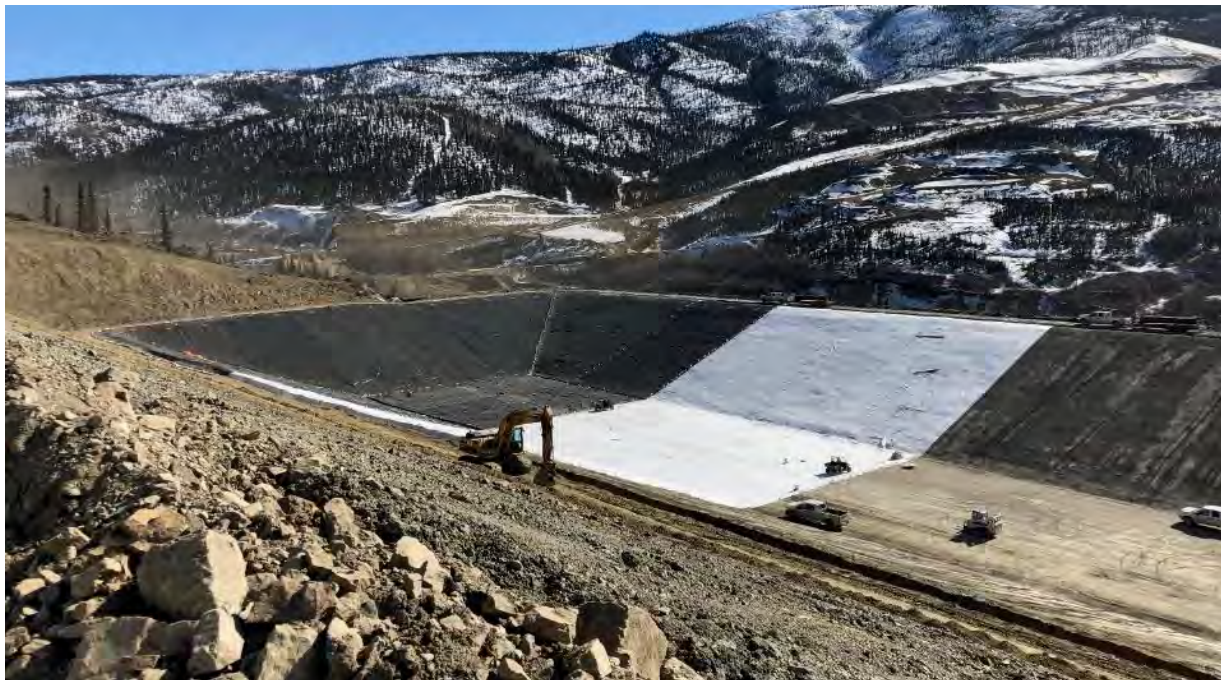
Photo 2.1-18: Events Pond Liner Installation - April 3, 2019
