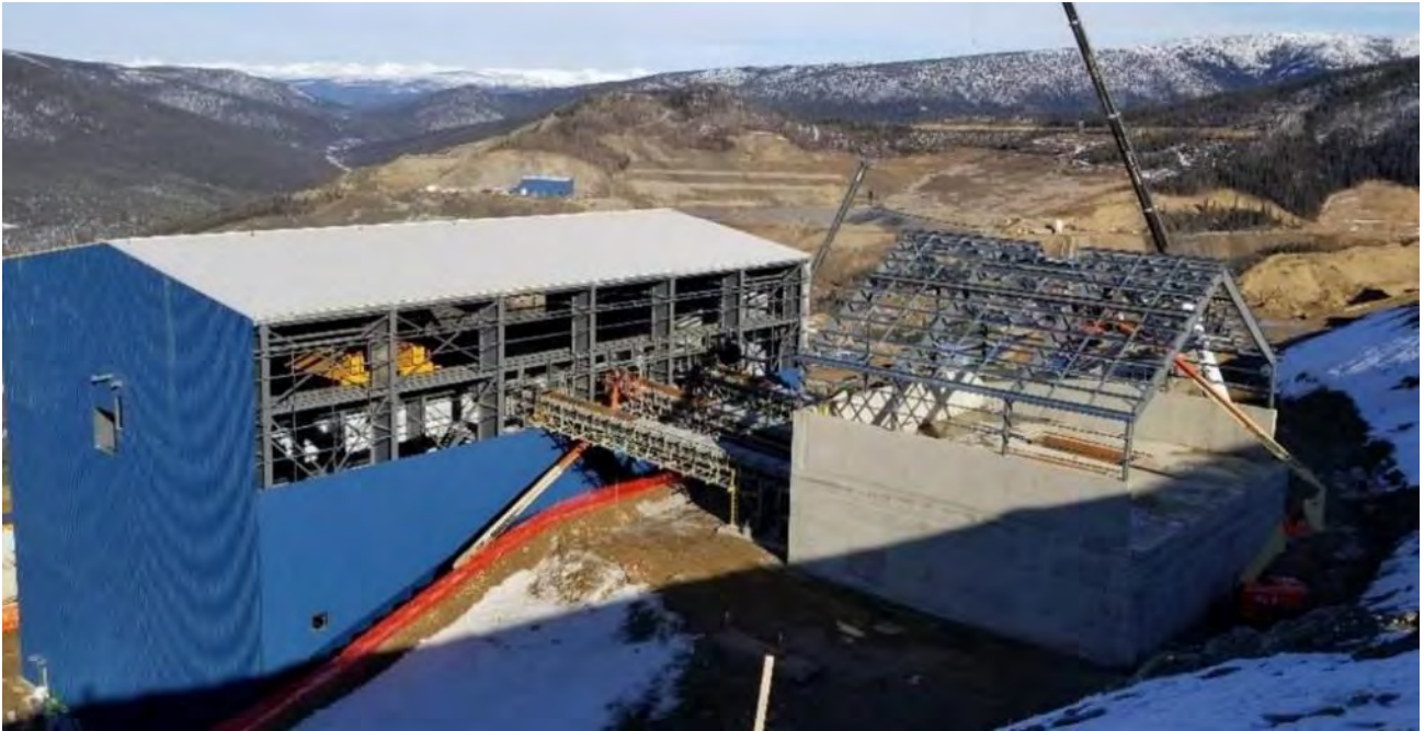
Photo 2.1-8: Secondary and Tertiary Crushing Facility - March 31, 2019
