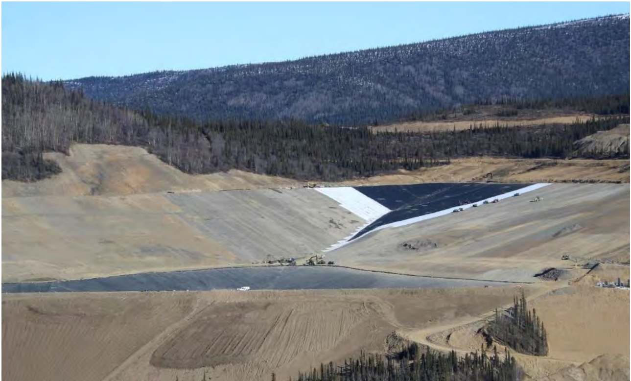
Photo 2.1-19: HLF Liner Deployment in Phase 1A Area - May 2, 2019
