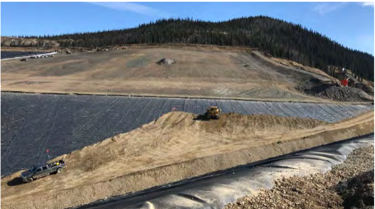
Photo 2.1-20: In-Heap Pond Area ODF Placement - May 10, 2019
