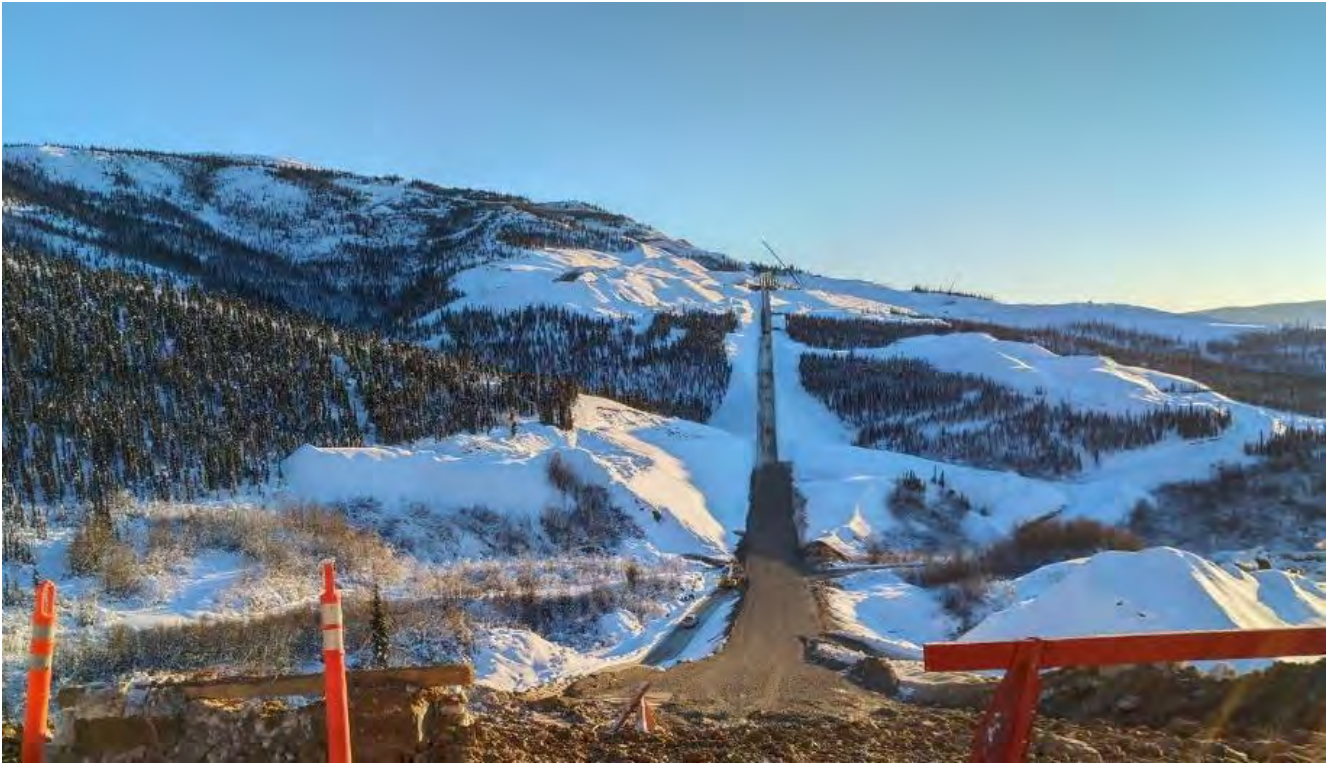
Photo 2.1-12: Overland Conveyor Grading Completion - February 1, 2019
