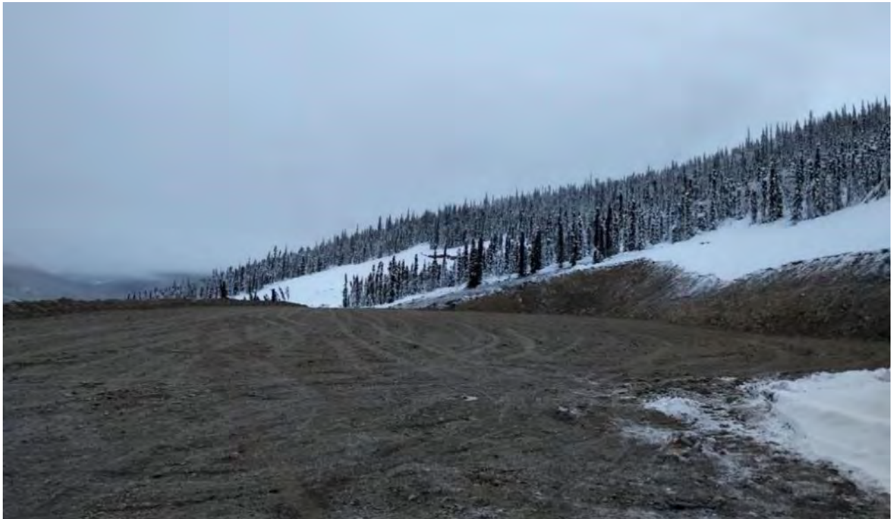
Photo 2.1-15: Explosives Area Pad Grading - January 24, 2019
