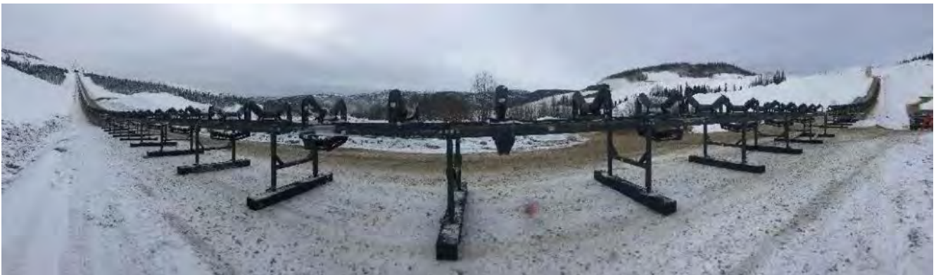
Photo 2.1-13: Overland Conveyor Structure Installation - February 28, 2019
