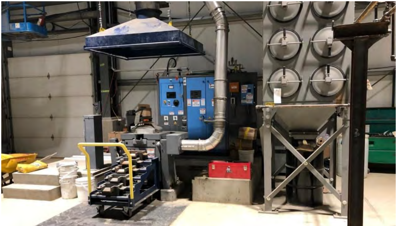
Photo 2.1-7: ADR Furnace Installation - April 6, 2019
