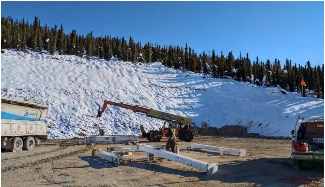
Photo 2.1-16: Erecting Explosives Silo Frame - March 5, 2019
