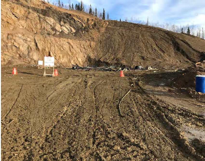
Photo 19 Eagle Pit – Entrance to Inert Waste Storage Area
