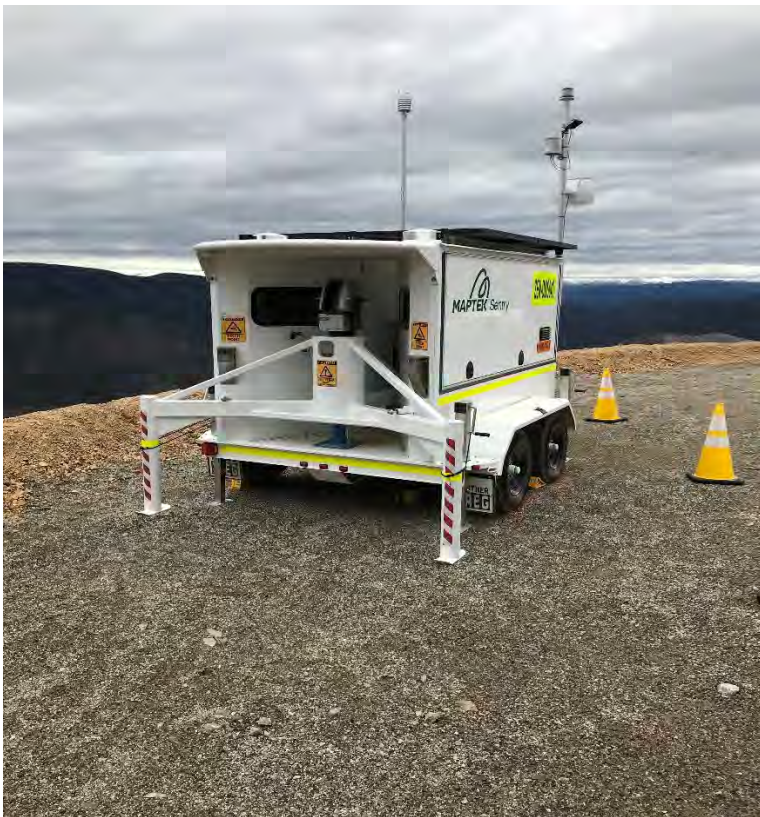
Photo 6 MAPTEK Sentry Lightning Detection System, Showing Sensor
