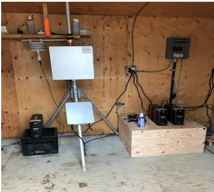
Photo 2 Air Quality Monitoring Station AQ2 –(Inside of Building) – Near Eagle Creek
