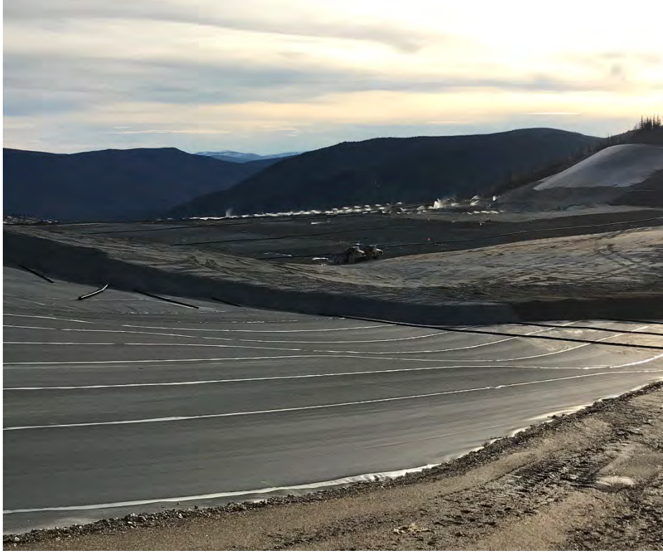
Photo 25 HLF Under Construction, Looking south-southwest from South End of Phase 3
