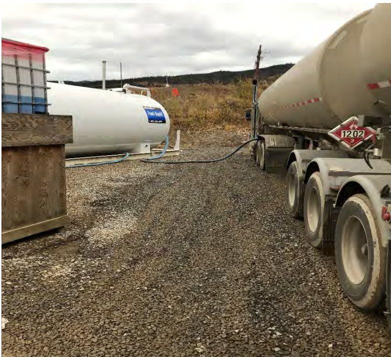
Photo 18 Diesel Fuel Delivery to Storage Tank. Note drainage ditch just ahead of truck, no secondary containment
