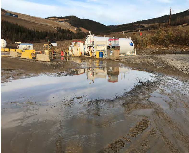
Photo 17 Gasoline and Diesel Fuel Storage Tanks. Note drainage ditch beyond tanks on photo right-centre
