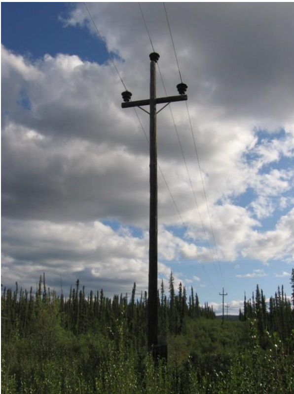
Photo 6.9-1: Typical Tangent Pole
