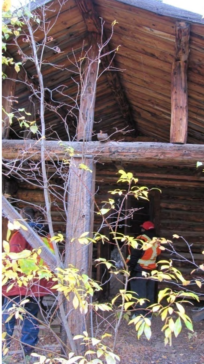
Plate 28: Site 2 structure, view west of the front of the structure; note porch with extended overhanging roof
