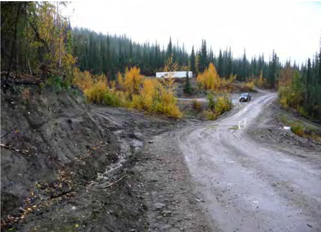
Note: View to the north. Intact deposits on west side of road.
