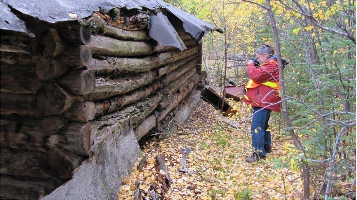
Plate 31: Site 2 structure, exterior view of north wall
