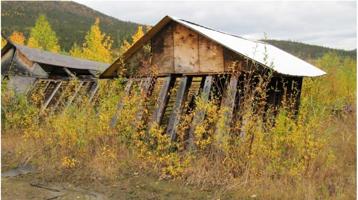
Plate 17: Site 1, view west at core structures [3]
