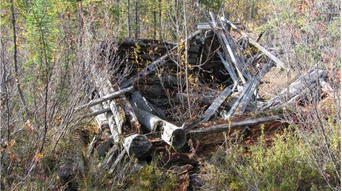
Plate 35: Site 3 structure, view west
