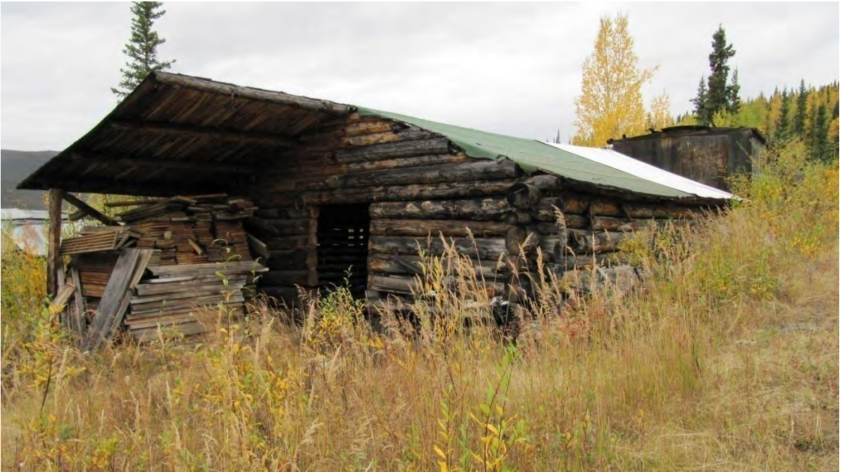
Plate 4: Site 1, view northwest of log structure [5]; note more recently constructed roof extension over front of the structure
