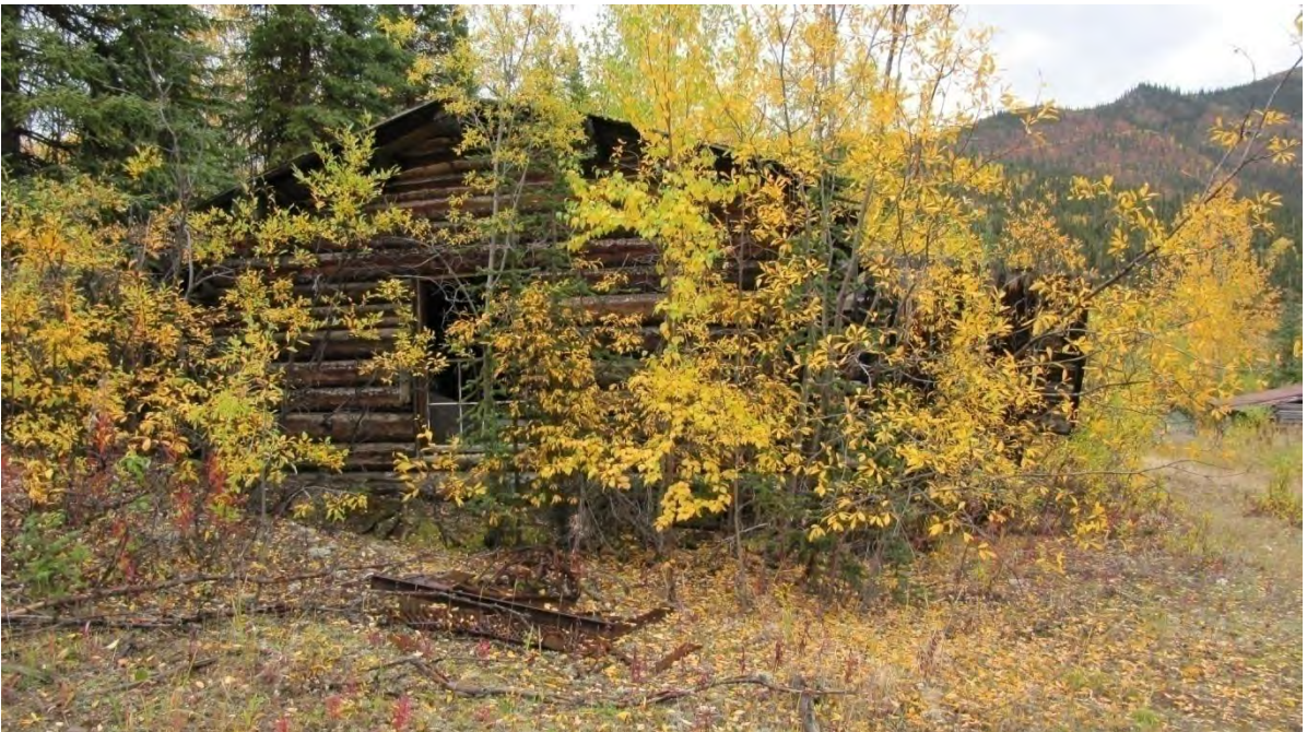
Plate 8: Site 1, view south of back side of log structure [7]
