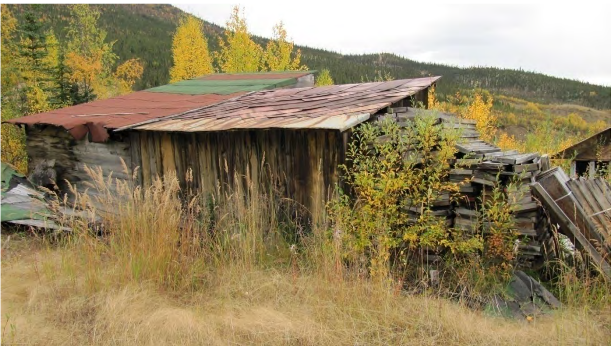
Plate 12: Site 1, view southwest showing the back side and partial metal roof of the plank structures [4]
