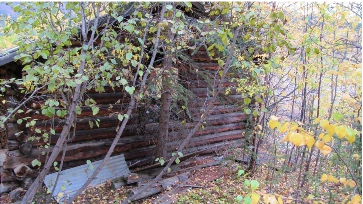
Plate 32: Site 2 structure, exterior view of back (west) wall
