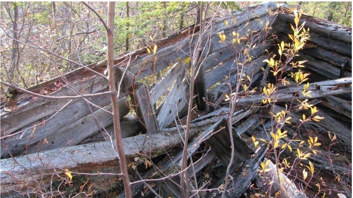
Plate 36: Site 3 structure, view southwest; note window opening on south wall
