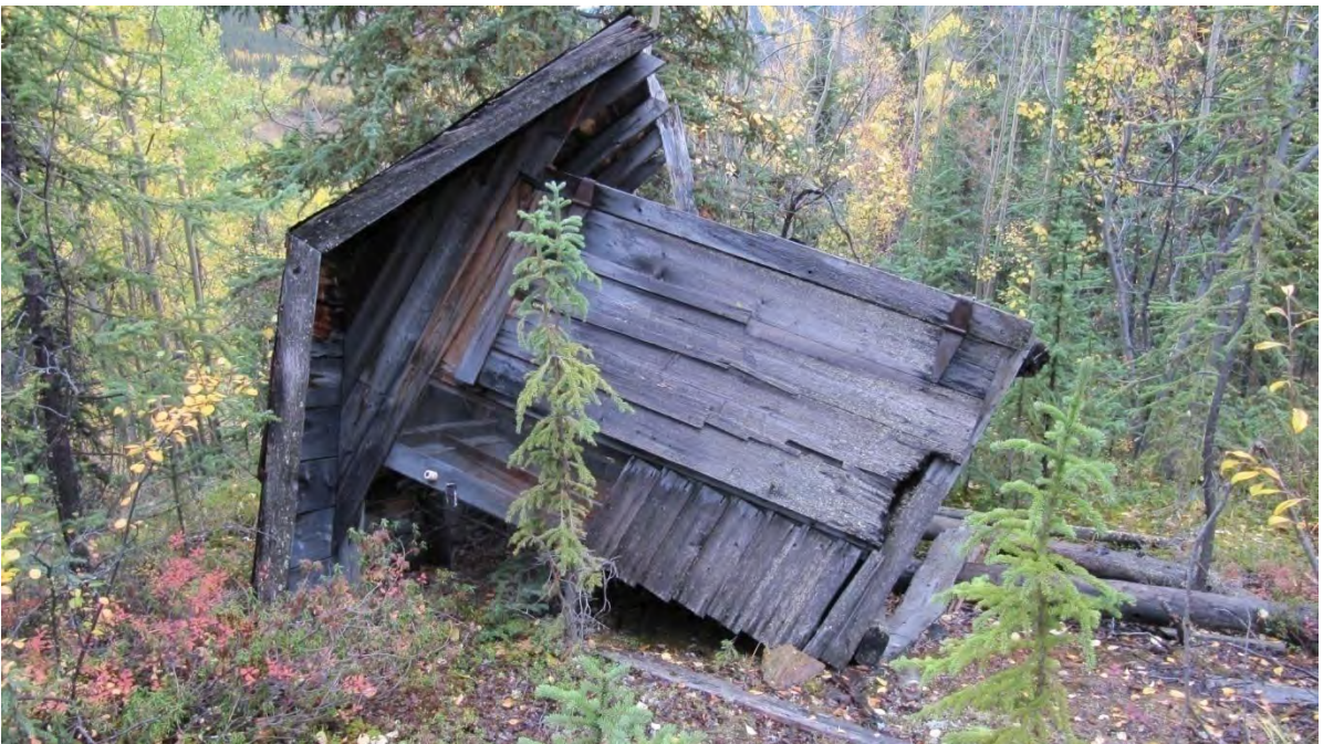
Plate 23: Site 1, small shack [10], view west
