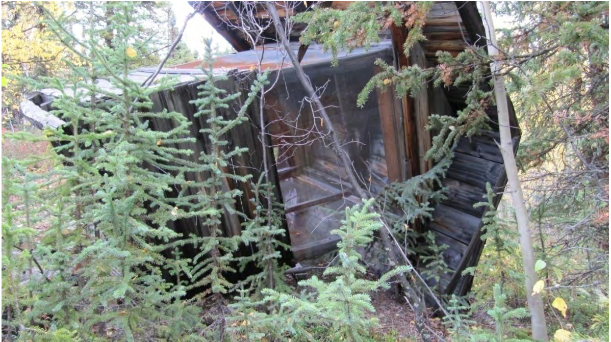
Plate 24: Site 1, small shack [10], view east
