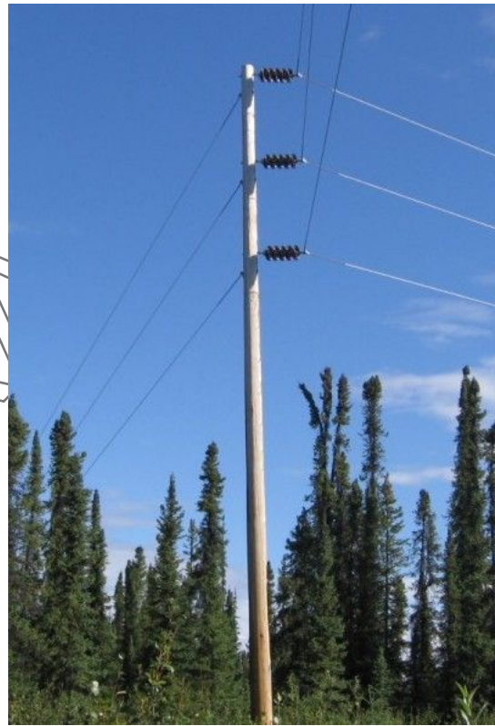
Photo 6.9-2: Typical Running Angle Pole
