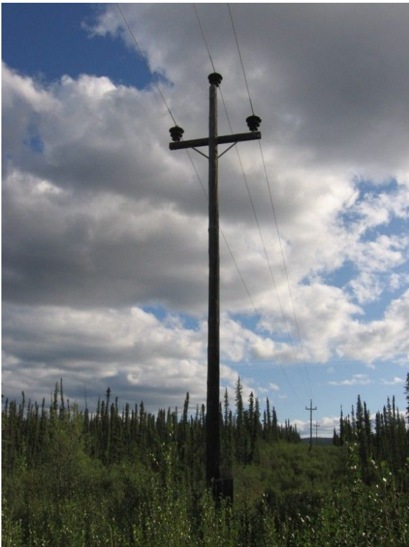
Photo 6.9-1: Typical Tangent Pole
