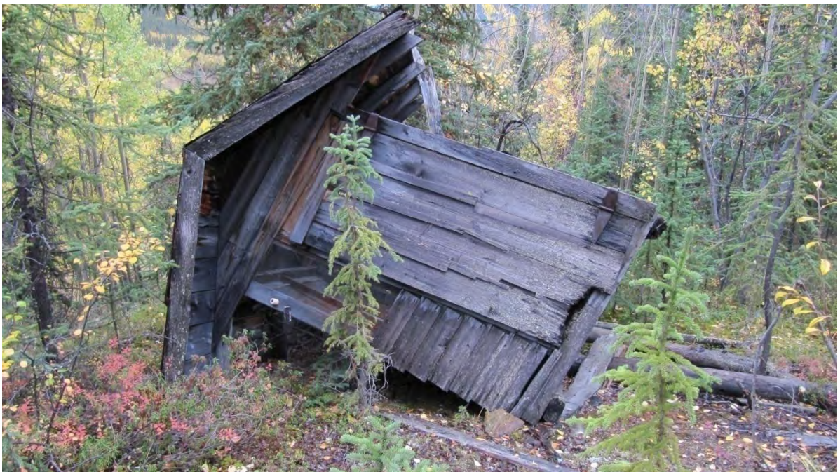
Plate 23: Site 1, small shack [10], view west
