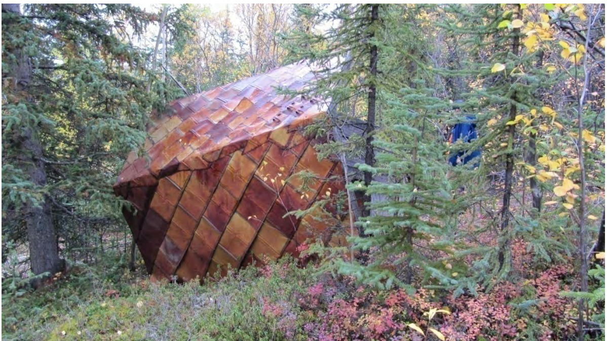
Plate 25: Site 1, metal roof of small shack [10], view north
