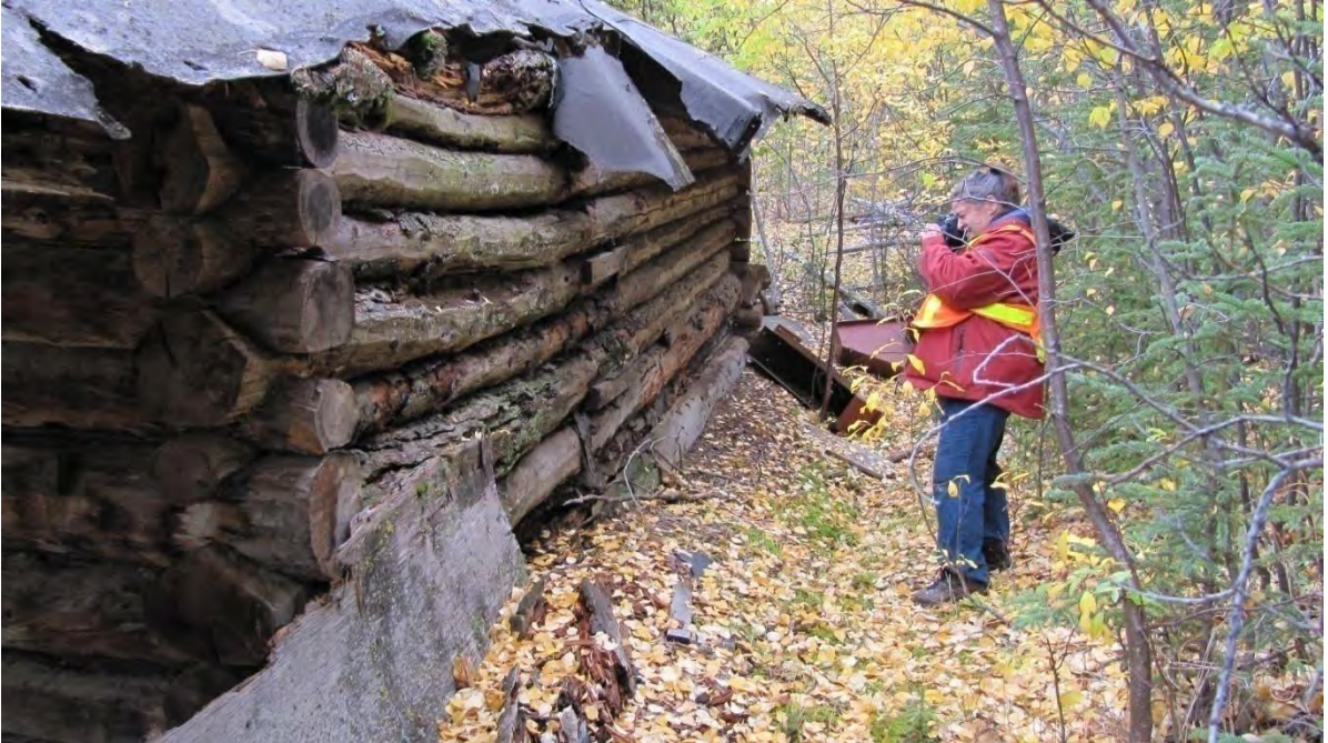
Plate 31: Site 2 structure, exterior view of north wall
