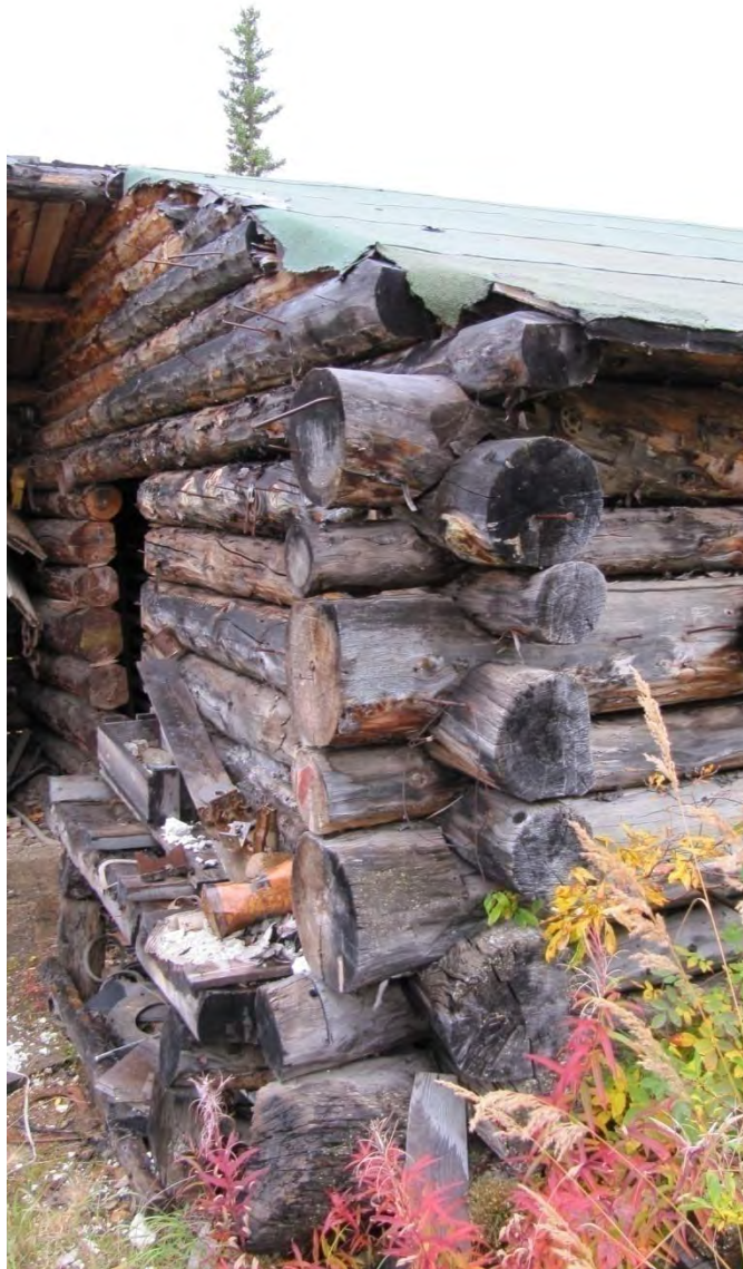
Plate 6: Site 1, log structure [5], view northwest at structure details
