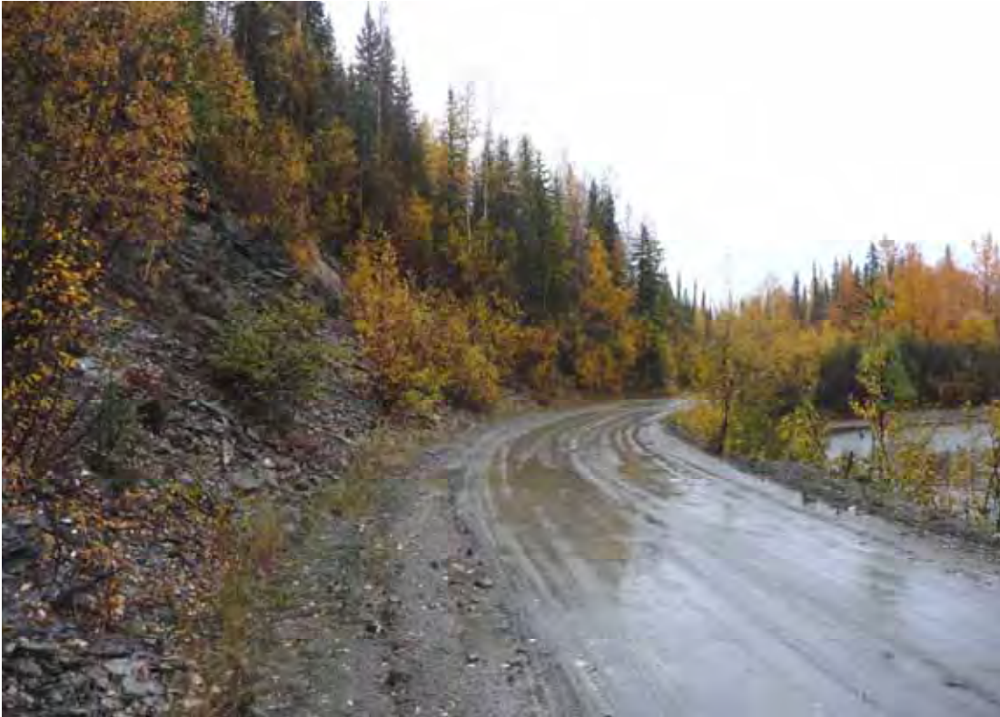
Note: View to the north along roadcut through phyllite.
