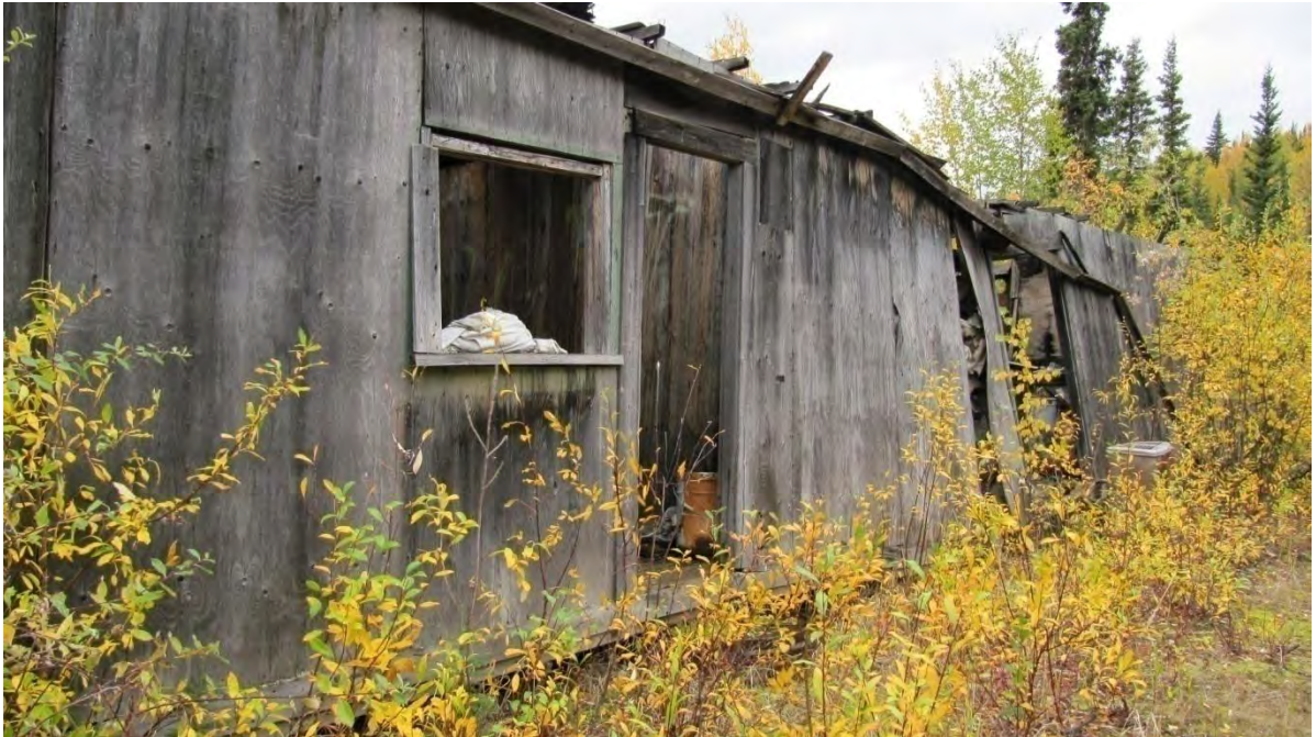
Plate 15: Site 1, plank/board/plywood structure [6], view northwest
