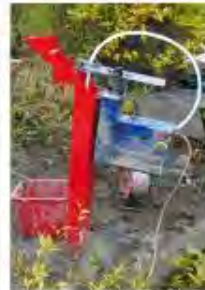
Installation of groundwater monitoring well
