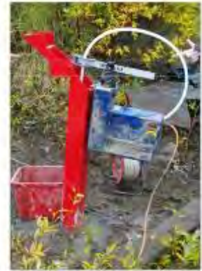
Developing monitoring well, summer 2009
