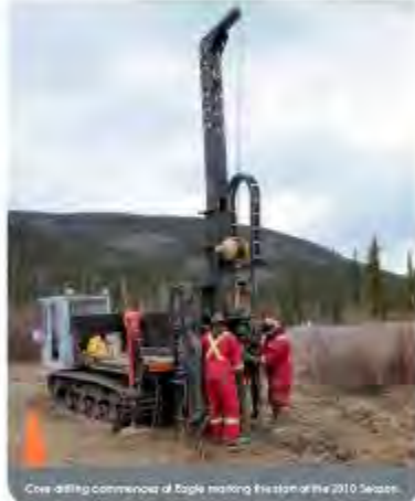
Cove drilling commences at Eagle making first hole in the 2010 season.
