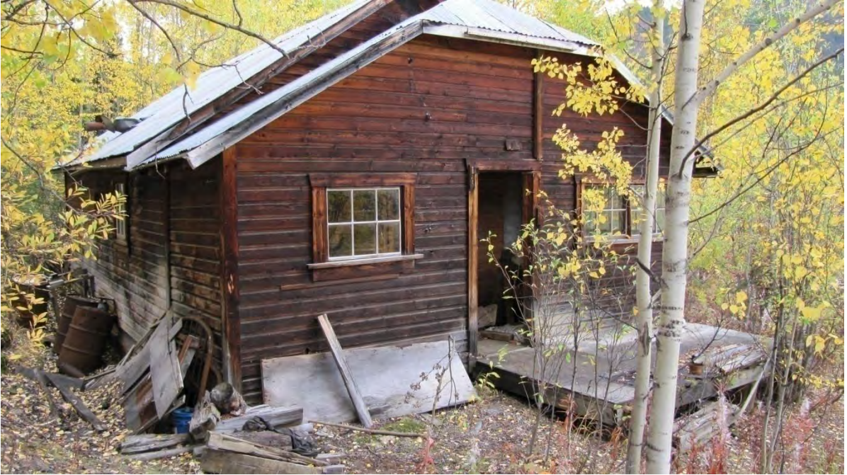
Plate 19: Site 1, house [8], view southeast
