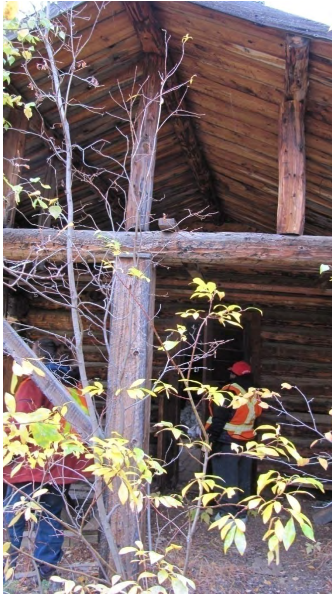
Plate 28: Site 2 structure, view west of the front of the structure; note porch with extended overhanging roof
