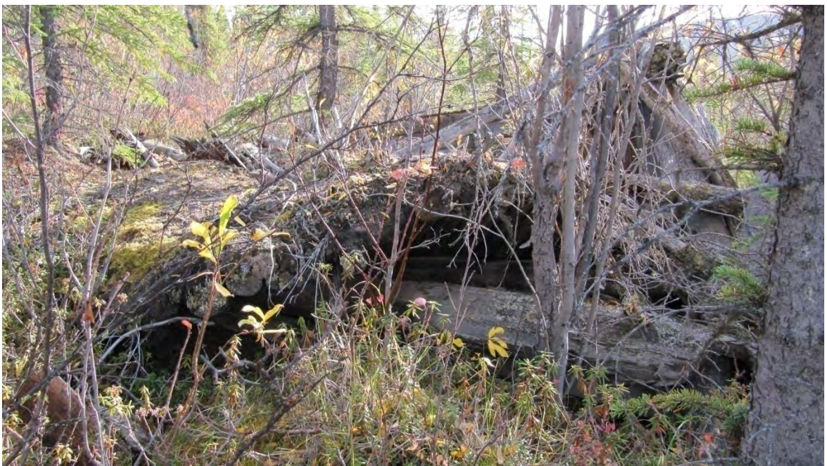
Plate 34: Site 3 structure, view south; note the sod roof
