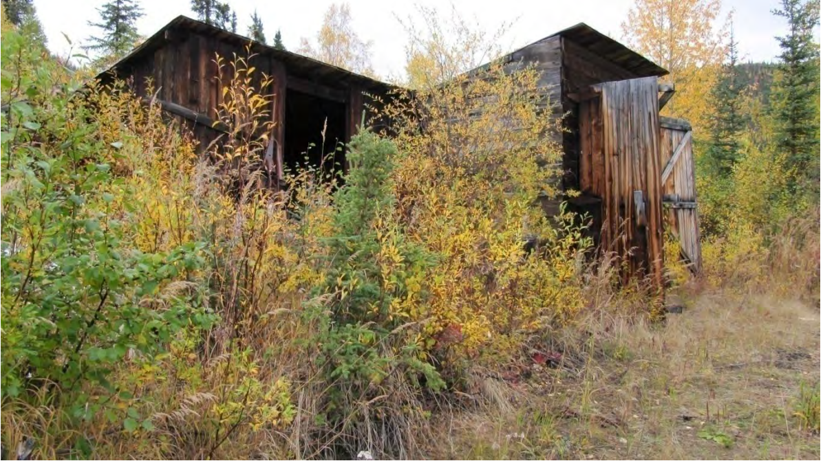
Plate 11: Site 1, view southeast of plank shacks [4]
