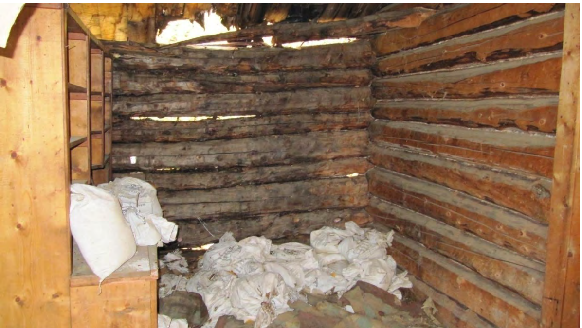
Plate 30: Site 2 structure, interior view of north wall
