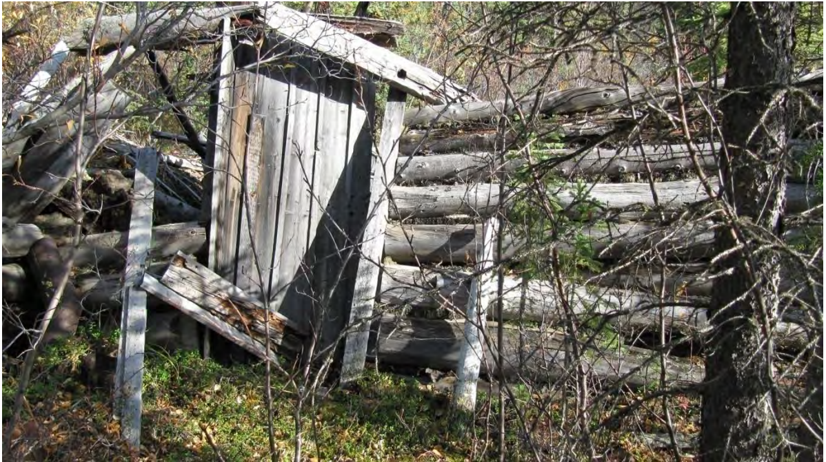
Plate 33: Site 3 structure, view east showing the front (door) of the cabin
