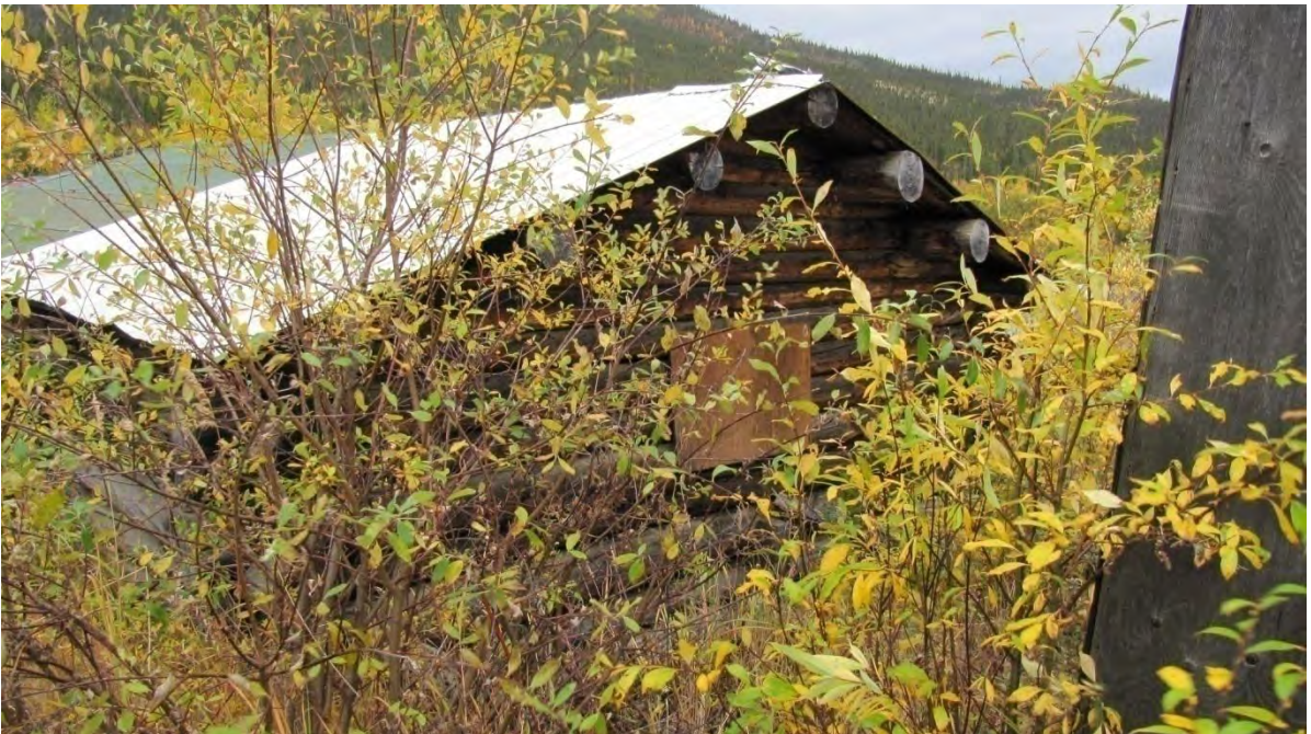
Plate 5: Site 1, back side of log structure [5], view southwest
