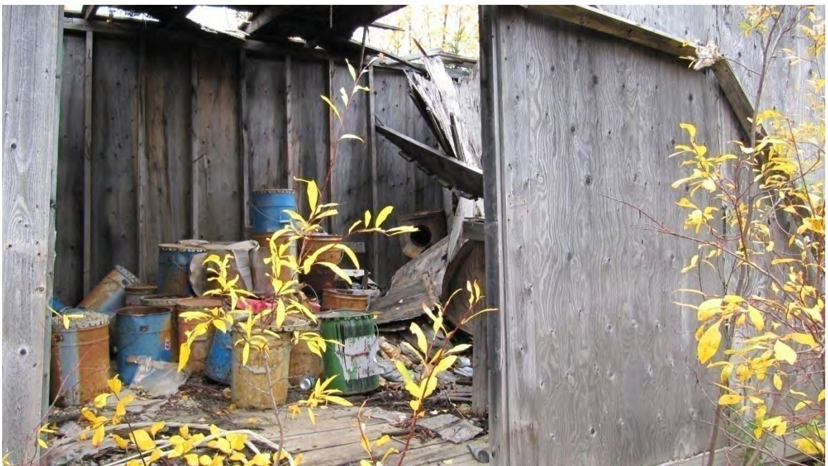
Plate 16: Site 1, interior view west of structure [6]
