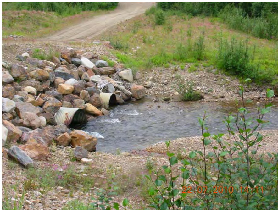
Photograph 6 Proposed location of overflow CSP
