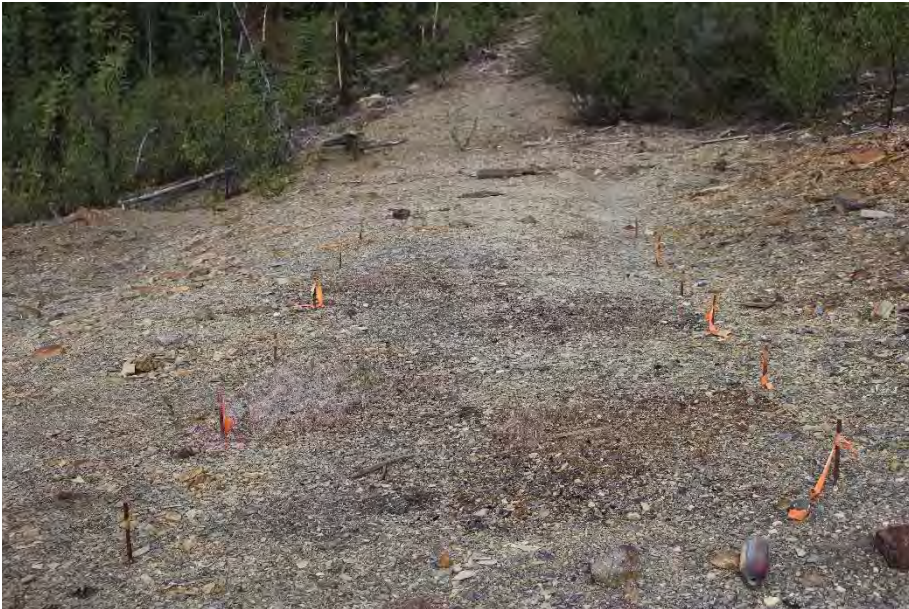
Photo # 14: Overall view of Block 3 on the Waste Rock site.
