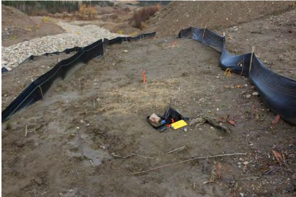
Installed willow staking, Sept 2019
