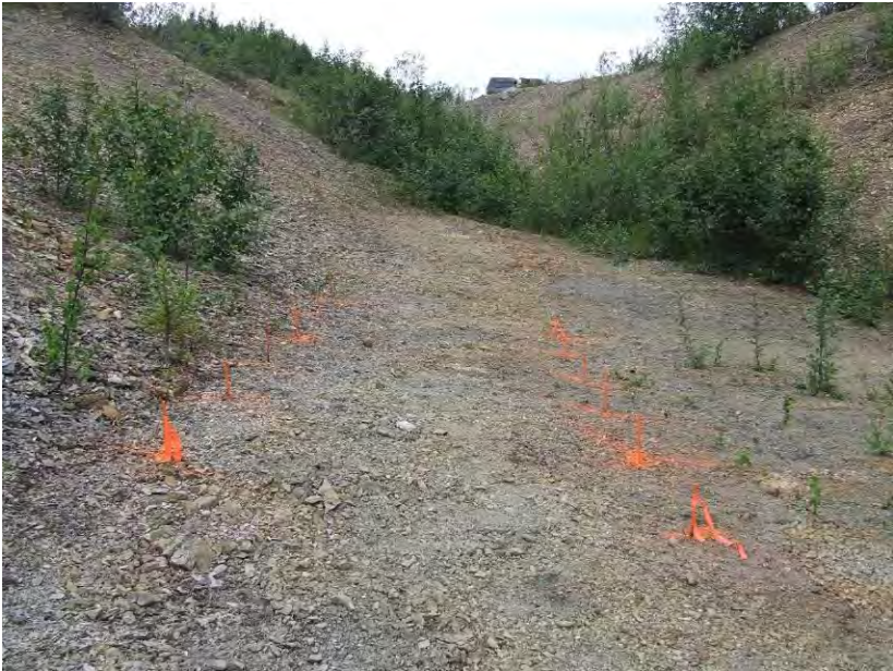
Photo #1: Trench - Block #1 staked out, July 2012
