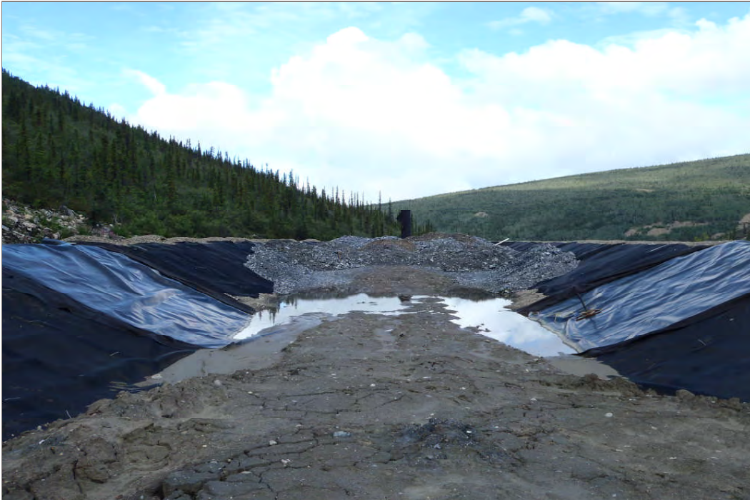
Photo 3: Partially completed PAG Waste Storage Facility (Facing north – July 28, 2011)
