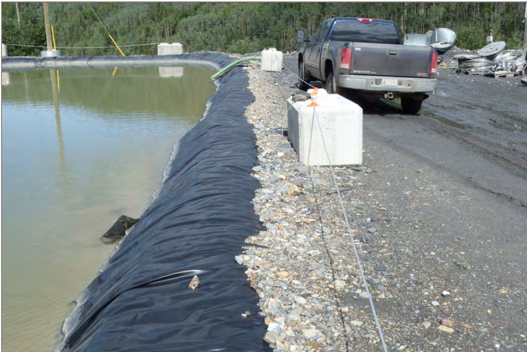
Photo 10: Liner anchoring trench and berm (Facing north – July 28, 2011)
