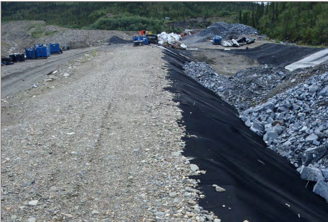
Photo 4: Liner anchoring trench along east berm (Facing south – July 28, 2011)
