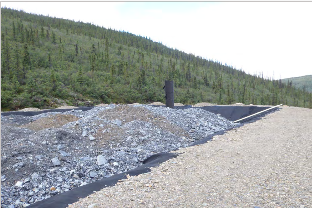
Photo 2: Geotextile wrapped vertical culvert, waste piles, completed portion of liner system (Facing north – July 28, 2011)
