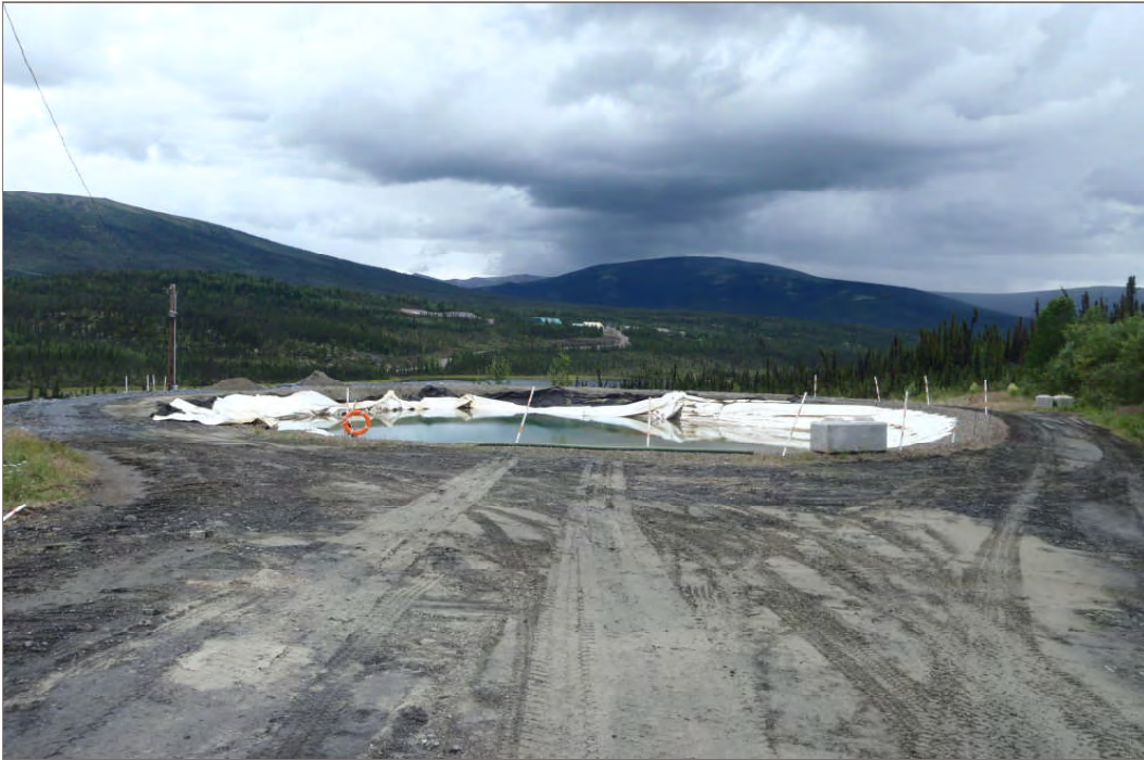
Photo 19: Galkeno 900 water treatment pond liner falling into pond (Facing south – July 28, 2011)
