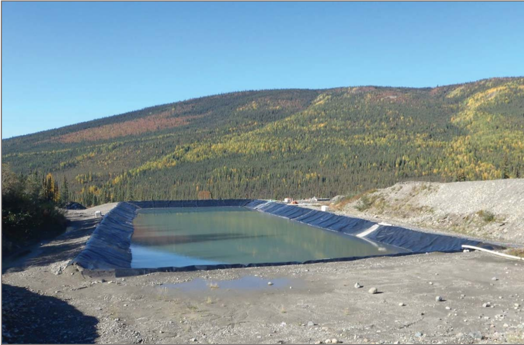
Photo 19: Mill Water Storage Pond Approximately 2.0 m of freeboard in mill water storage pond Facing west – September 10, 2013
