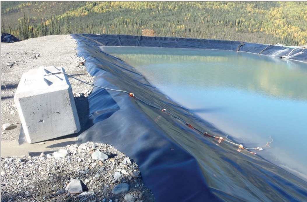
Photo 22: Mill Water Storage Pond Safety rope for exiting pond Facing west – September 10, 2013
