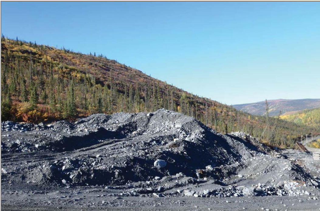
Photo 10: Bellekeno Waste Rock Pile Overview of waste rock pile Facing west – September 10, 2013
