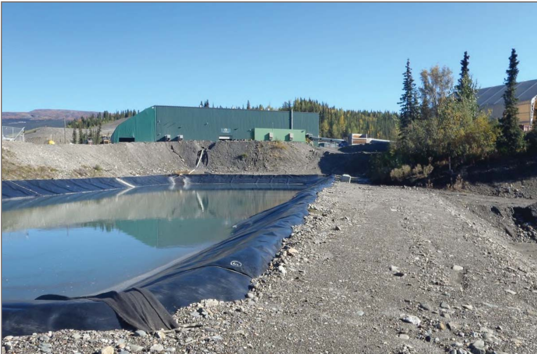
Photo 20: Mill Water Storage Pond Stable perimeter berm Facing east – September 10, 2013
