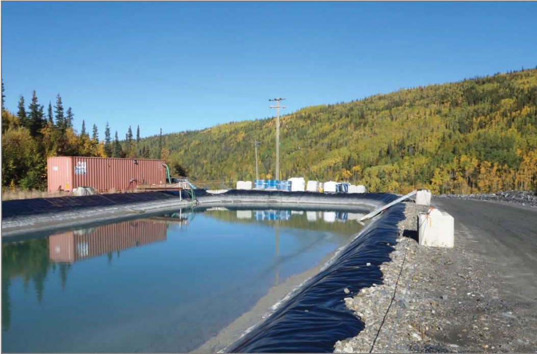
Photo 7: Bellekeno 625 Water Treatment Ponds Approximately 1.5 m freeboard in pond two Facing north – September 10, 2013
