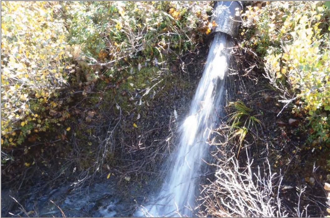
Photo 9: Bellekeno 625 Water Treatment Ponds Discharge point requiring rip-rap armouring for erosion protection Facing south – September 10, 2013
