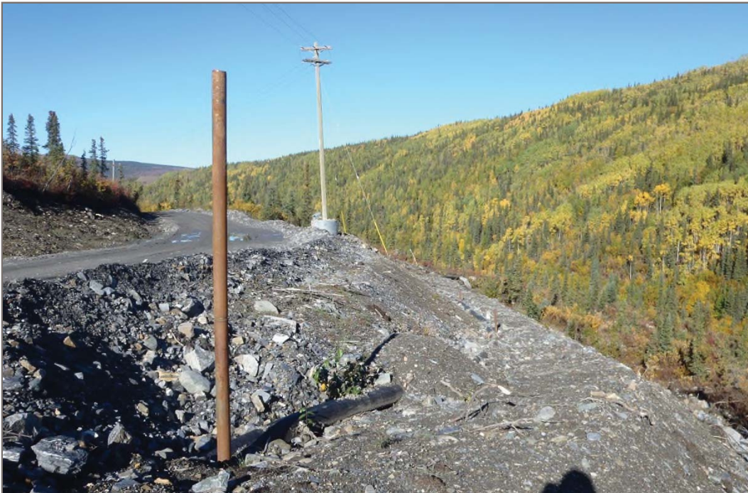
Photo 8: Bellekeno 625 Water Treatment Ponds Partially buried discharge line Facing west – September 10, 2013
