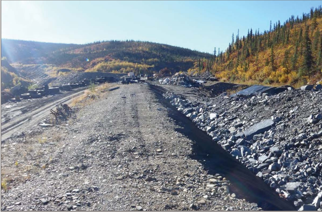
Photo 1: PAG Waste Storage Facility Perimeter berm Facing south – September 10, 2013
