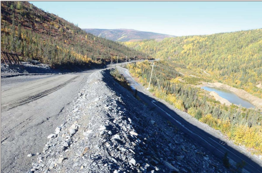
Photo 12: Bellekeno Waste Rock Pile Stable pile sideslopes Facing west – September 10, 2013
