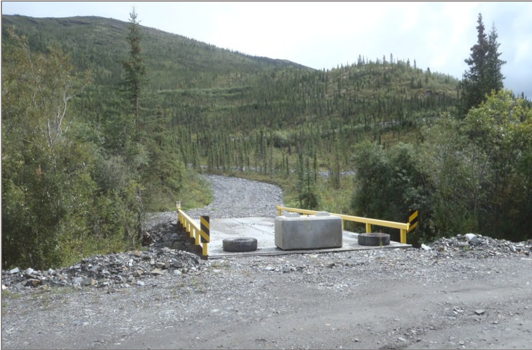
Photo 13: Lightning Creek Bridge Abutments (Onek Road) Bridge overview Facing south – August 12, 2014
