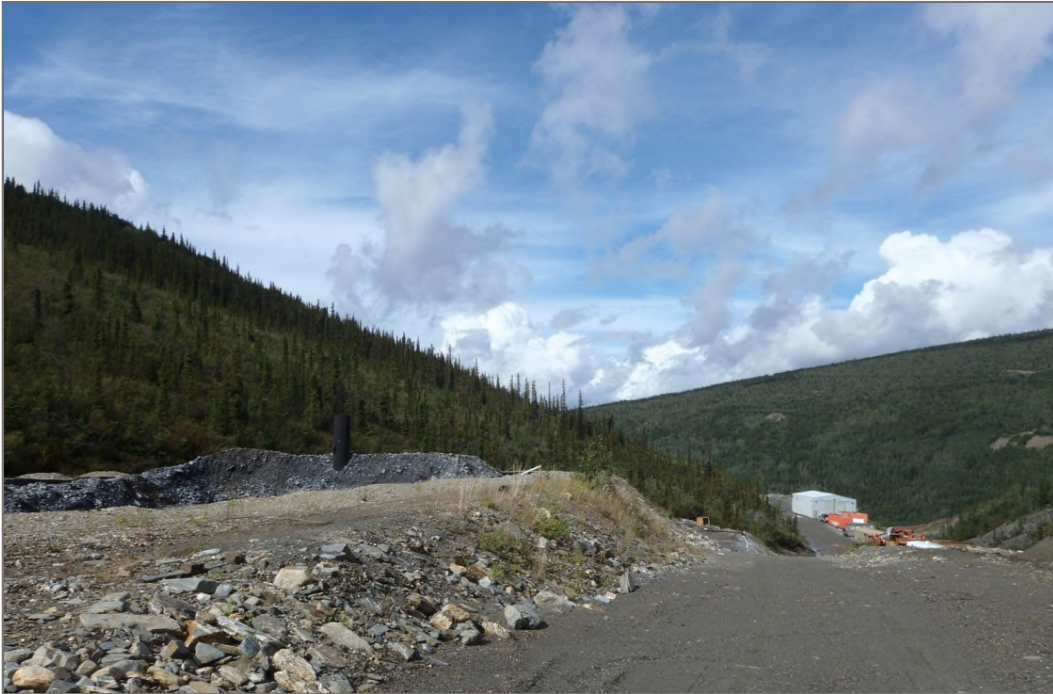
Photo 1: PAG Waste Storage Facility Facility berms and sideslopes Facing north – August 12, 2014
