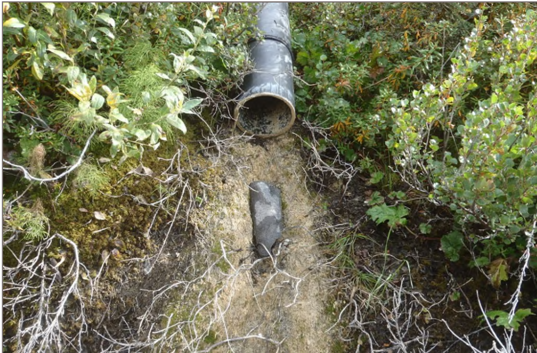
Photo 10: Bellekeno 625 Water Treatment Ponds Discharge location Facing south – August 12, 2014
