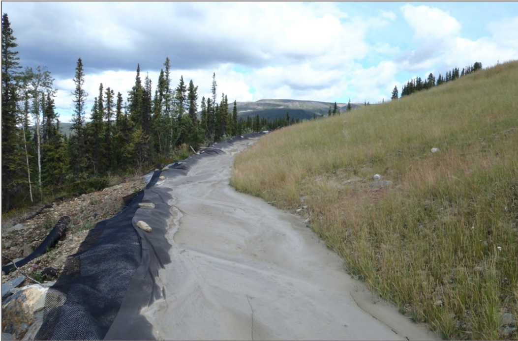
Photo 25: Dry Stacked Tailings Facility Tailings in the surface water runoff collection system Facing north – August 13, 2014
