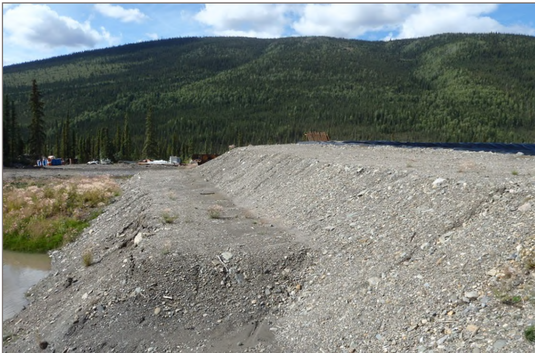
Photo 20: Mill Water Storage Pond Stable berm sideslope Facing west – August 13, 2014
