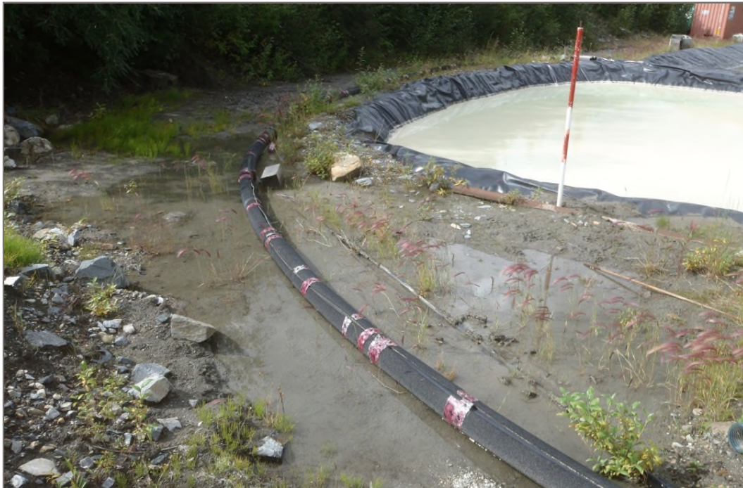
Photo 8: Bellekeno 625 Water Treatment Ponds Surface water and sediment accumulation outside southwest corner of primary pond Facing west – August 12, 2014
