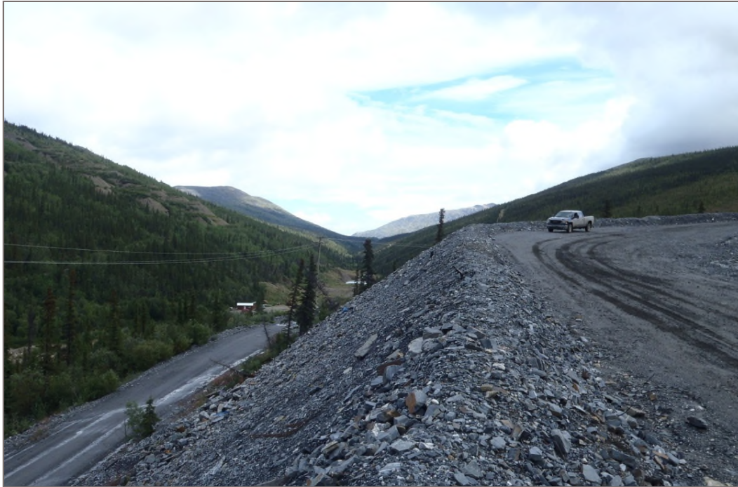
Photo 11: Bellekeno Waste Rock Pile Intact sideslopes Facing east – August 12, 2014
