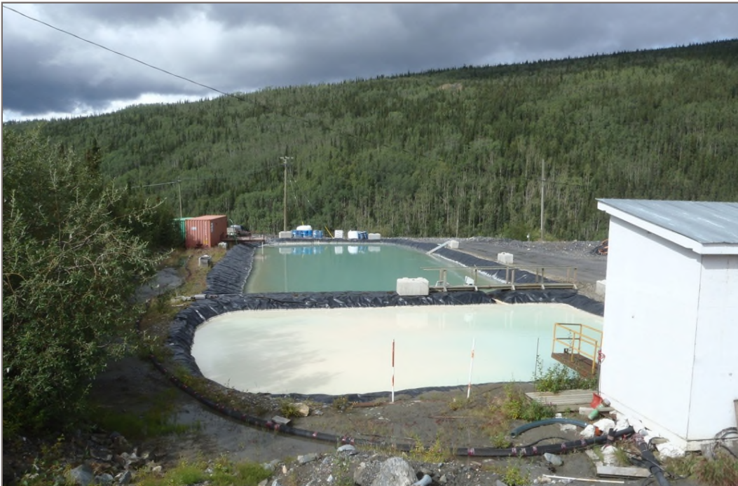
Photo 6: Bellekeno 625 Water Treatment Ponds Facility overview Facing north – August 12, 2014
