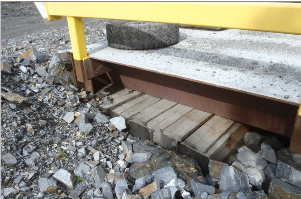
Photo 14: Lightning Creek Bridge Abutments (Onek Road) Stable timber bridge abutments Facing west – August 12, 2014
