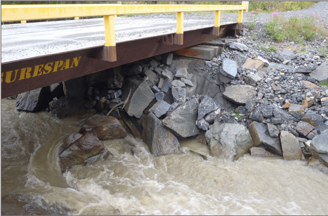
Photo 11: Lightning Creek Bridge Abutments (Onek Road) Displaced rip-rap on downstream side of south abutment Facing South - August 10, 2015
