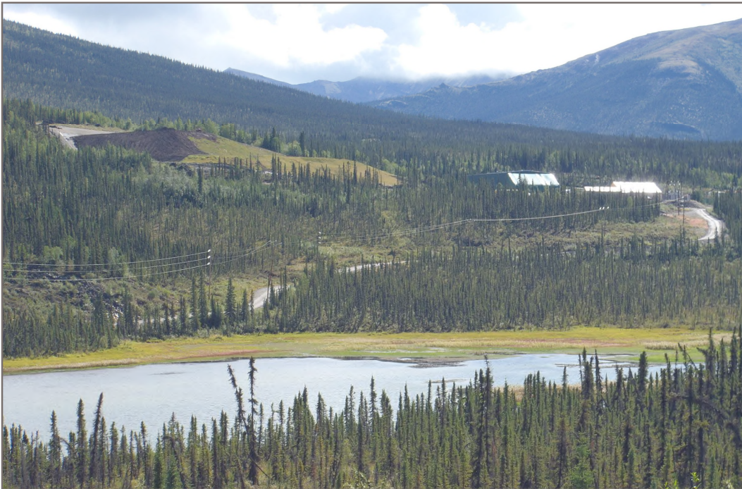
Photo 16: Dry Stacked Tailings Facility Regraded and covered tailings facility Facing East - August 11, 2015
