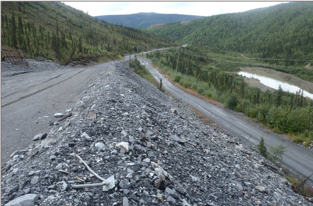
Photo 4: Bellekeno Waste Rock Pile Stable waste rock pile sideslope Facing West - August 10, 2015
