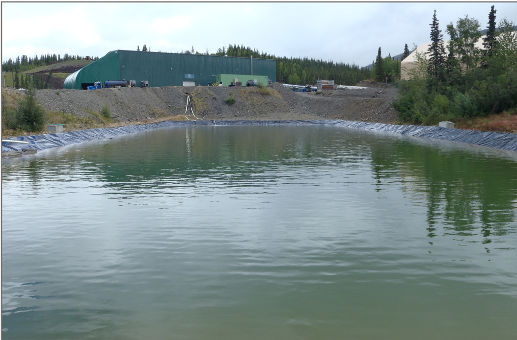
Photo 14: Mill Water Storage Pond Water level in pond Facing East - August 11, 2015
