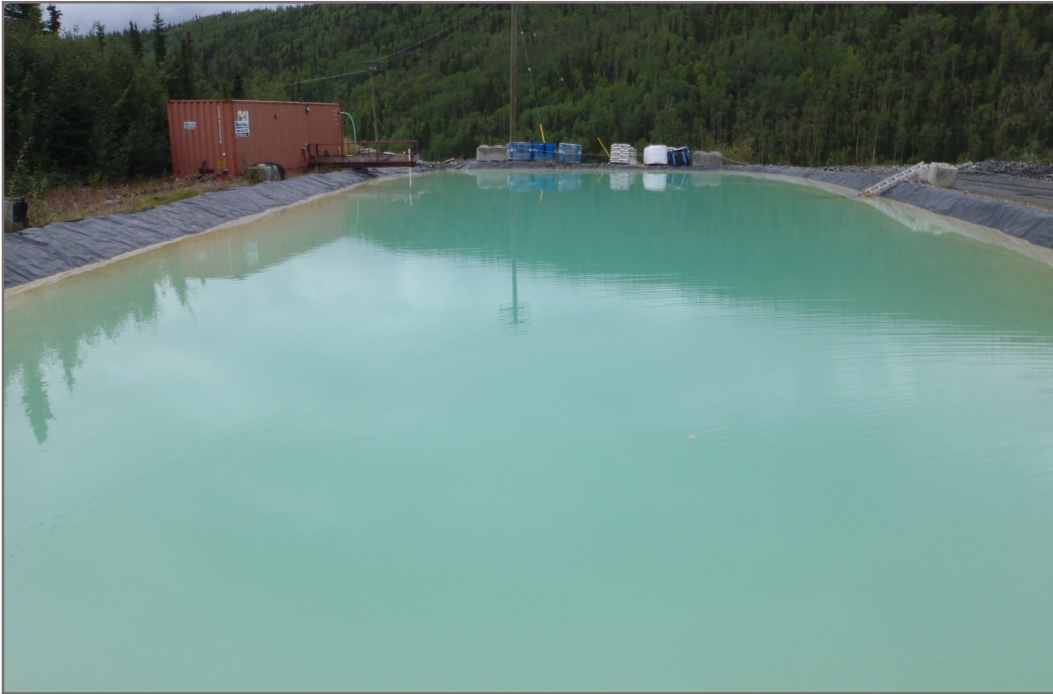
Photo 7: Bellekeno 625 Water Treatment Ponds Reduced freeboard at north end of secondary pond Facing North - August 10, 2015
