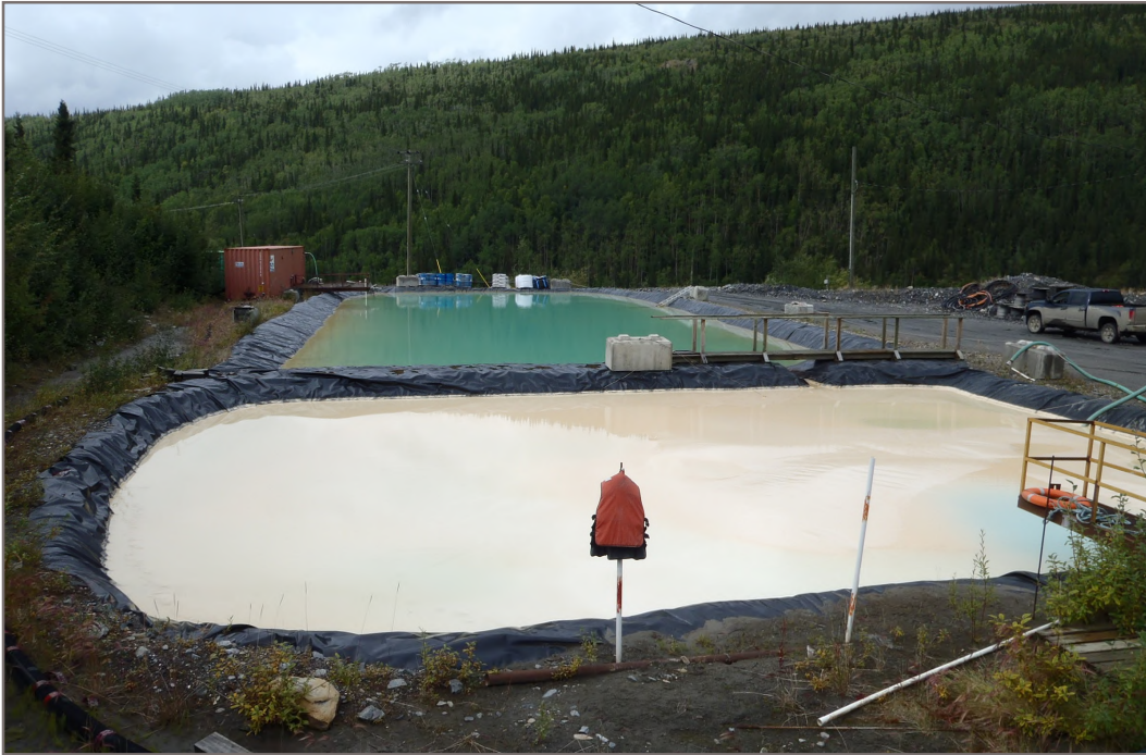
Photo 5: Bellekeno 625 Water Treatment Ponds Facility overview Facing North - August 10, 2015
