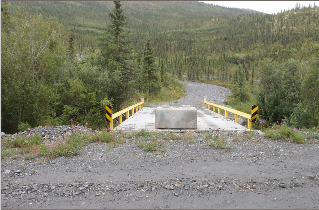
Photo 9: Lightning Creek Bridge Abutments (Onek Road) Bridge overview Facing South - August 10, 2015
