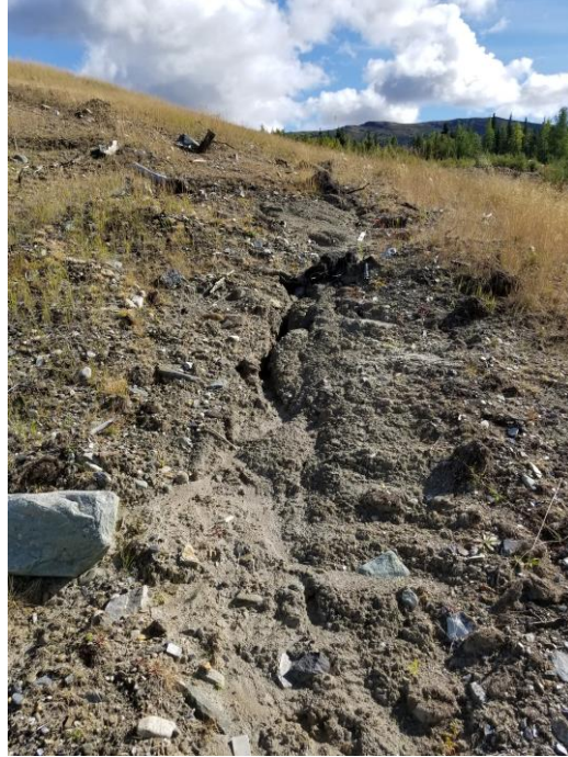
Photo 9: DSTF Visible Erosion and Deposition August 24, 2017
