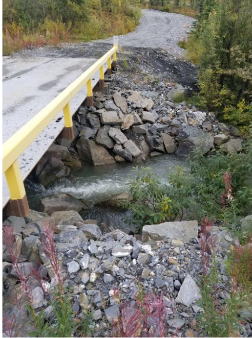
Photo 5: Lightning Creek Abutments Onek Road August 24, 2017
