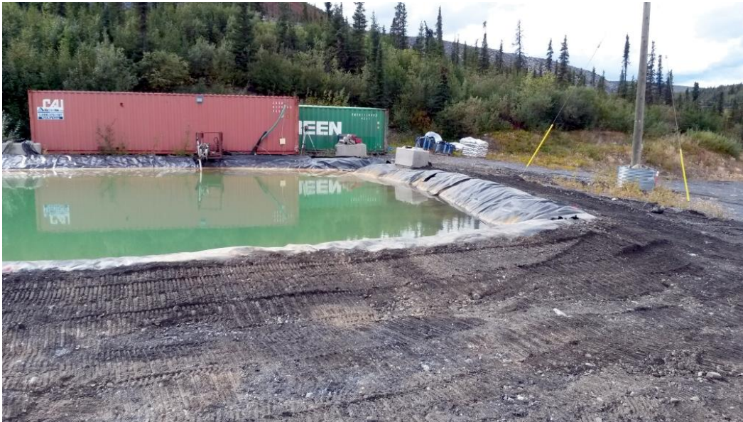
Photo 2: Bellekeno 625 Water Treatment Ponds North Perimeter Berm Facing South – August 24, 2017
