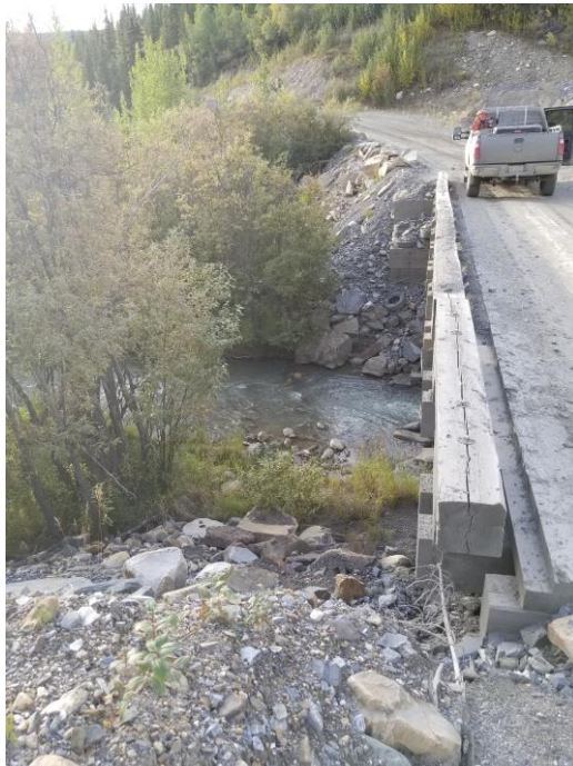
Photo 6: Lightning Creek Abutments Bellekeno Haul Road August 24, 2017
