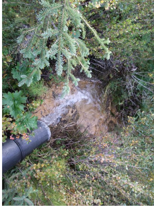
Photo 3: Bellekeno 625 Water Treatment Ponds Water Discharge August 24, 2017
