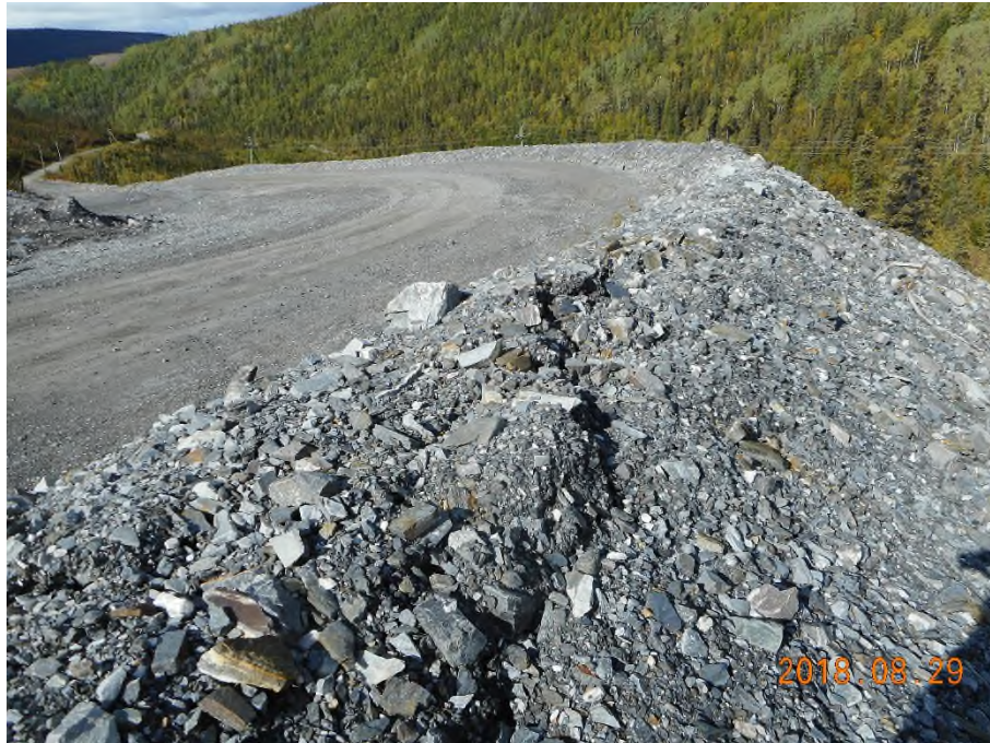
Photo 2: Bellekeno waste rock dump used as foundation for access road
