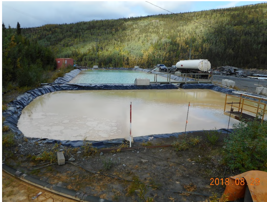
Photo 3: Bellekeno 625 water treatment ponds – discharge is from the far end of the facility
