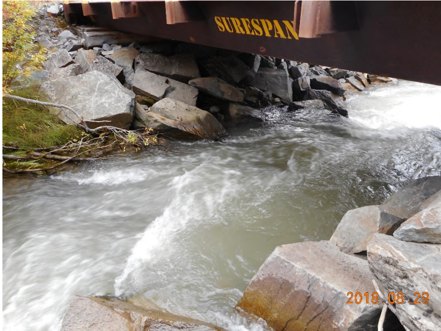
Photo 4: Well armoured bridge abutments at Lightning Creek crossing by the Onek road.
