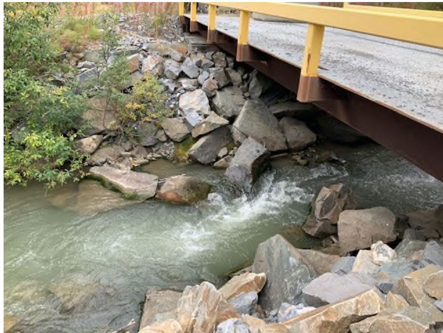
Photo 6 - Lightning Creek Bridge Abutments, Onek Road (August 20/19)
