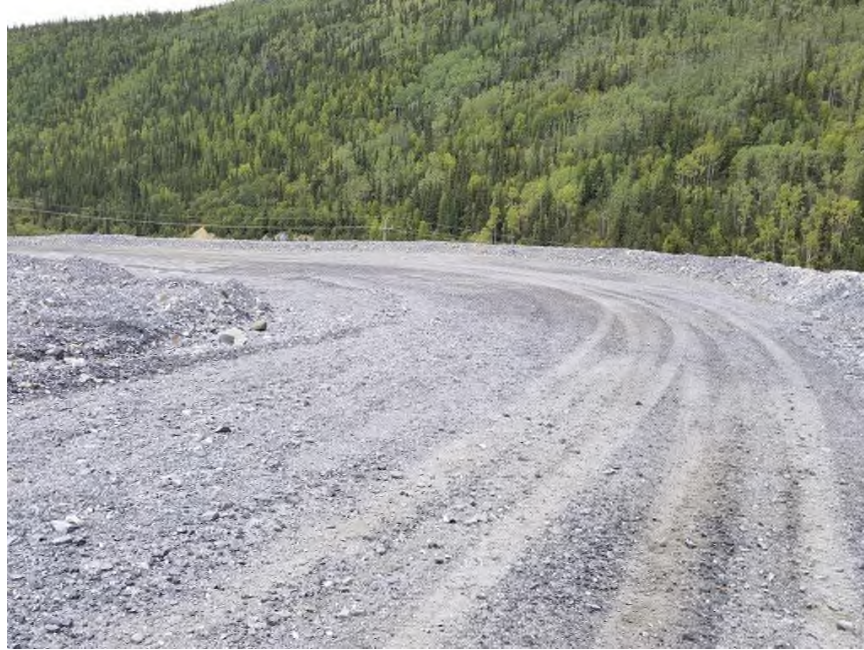
Photo 2 – Bellekeno Road Waste Rock Pile (August 20/19)
