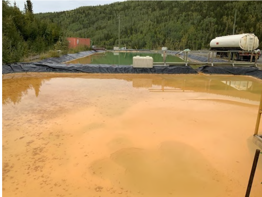
Photo 3 - Bellekeno 625 Water Treatment Ponds (August 20/19)
