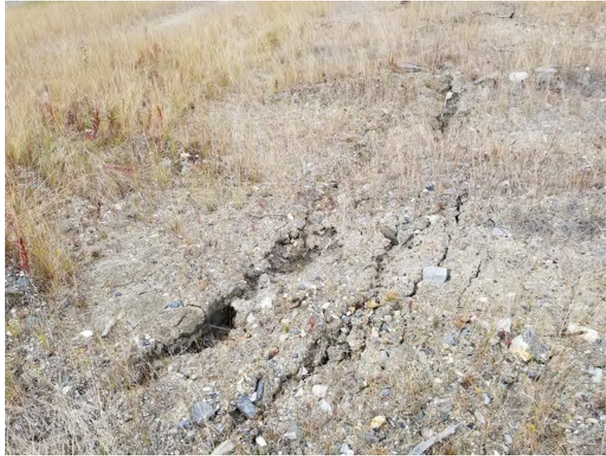
Photo 9 - DSTF Circular Instability (August 20/19)
