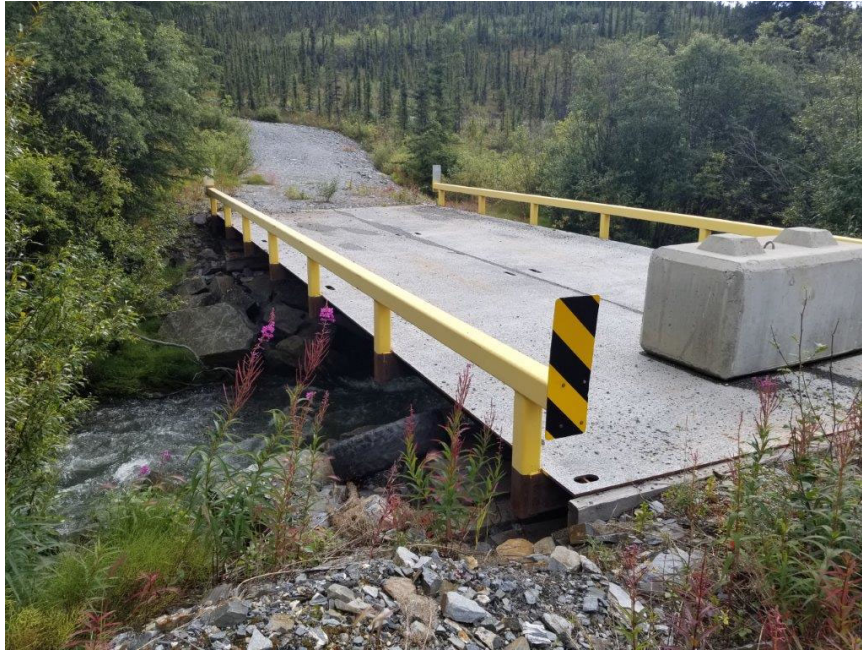
Photo 6 - Lightning Creek Bridge Abutments, Onek Road (August 18/20)
