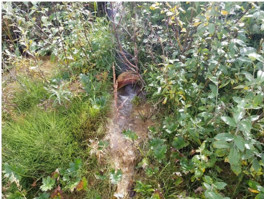
Photo 4 - Bellekeno 625 Water Treatment Ponds, Discharge Location (August 18/20)
