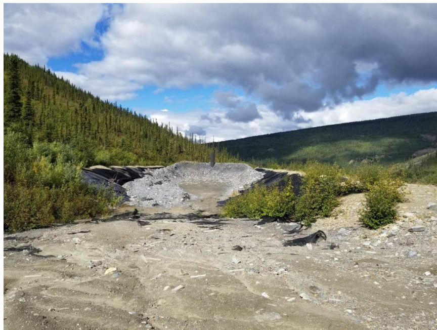
Photo 1 - Bellekeno PAG Storage Facility (August 18/20)
