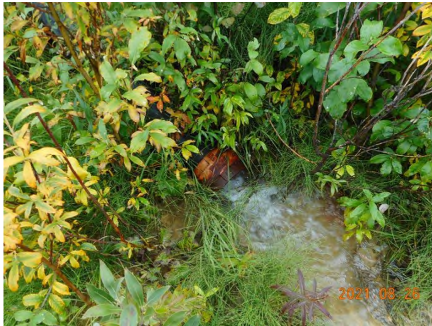
Photo 4: Bellekeno 625 Water Treatment Ponds, Discharge Location (August 26/21)
