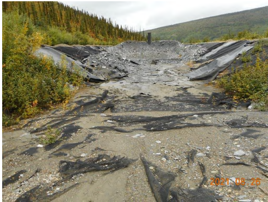
Photo 1: Bellekeno PAG Storage Facility (August 26/21)
