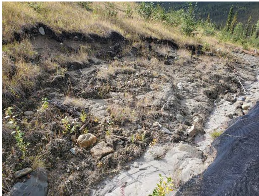
Photo 12: DSTF Shallow Failure into Runoff Collection Ditch (August 26/21)
