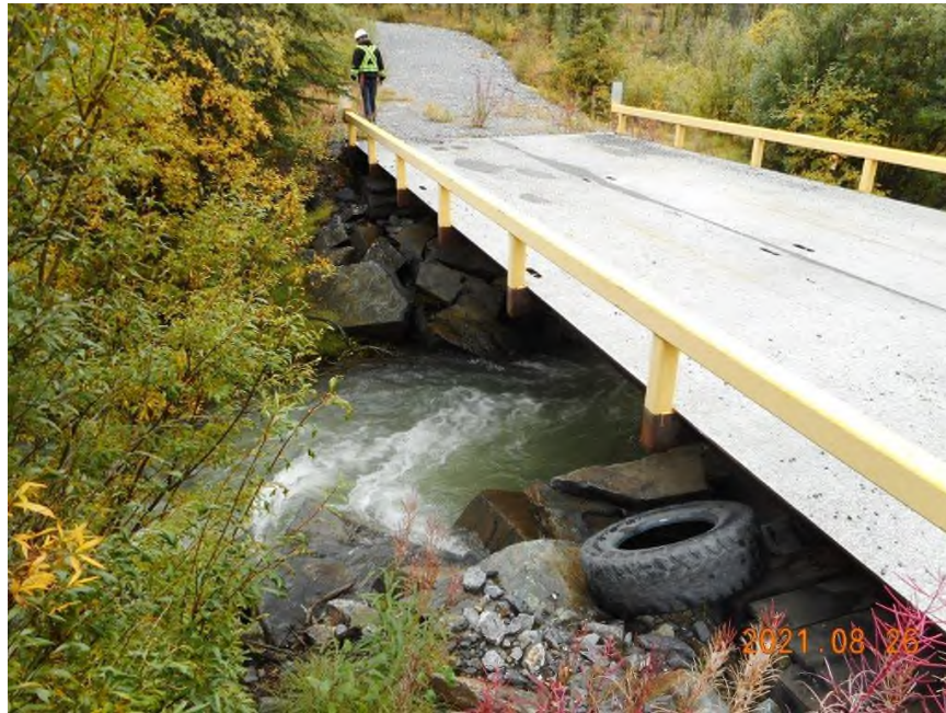
Photo 6: Lightning Creek Bridge Abutments, Onek Road (August 26/21)
