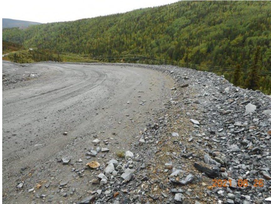
Photo 2: Bellekeno Road Waste Rock Pile/Haul Road (August 26/21)
