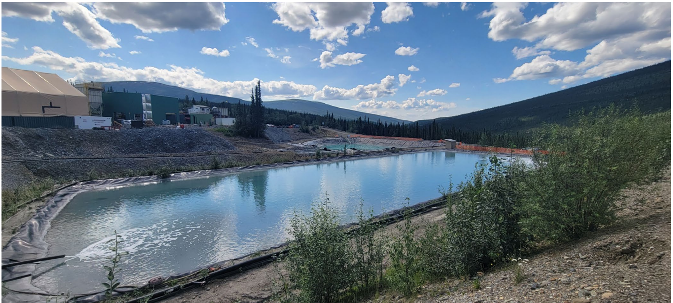
Photo 10: Fill Water Storage pond – facing south (I. MacIntyre, July 20, 2023)
