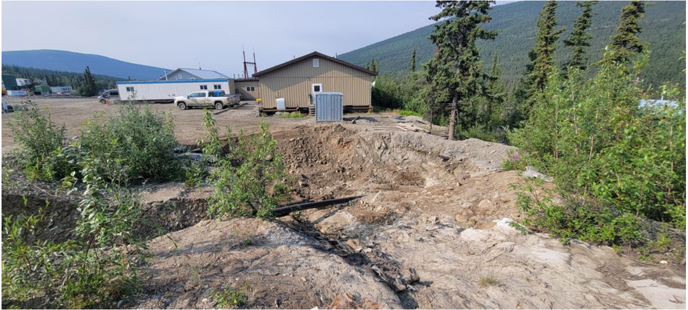
Photo 17: DSTF Phase 1 collection sump after cleaning of sediment build up. Liner was later installed. Facing southwest. (I. MacIntyre, July 22, 2023)
