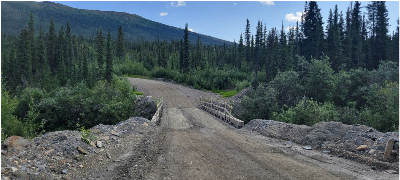
Photo 6: Lightning Creek Bridge – Bellekeno Haul Road (I. MacIntyre, July 30, 2023)
