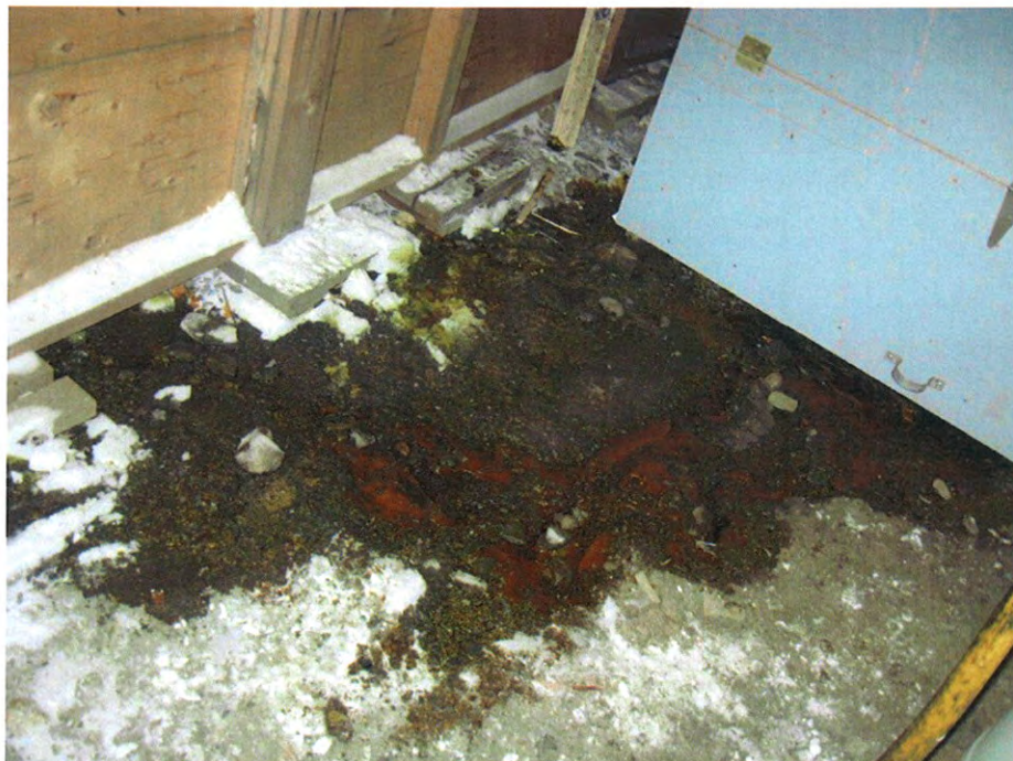
BK 625 Ferric Chloride on Floor of Reagent Shed
