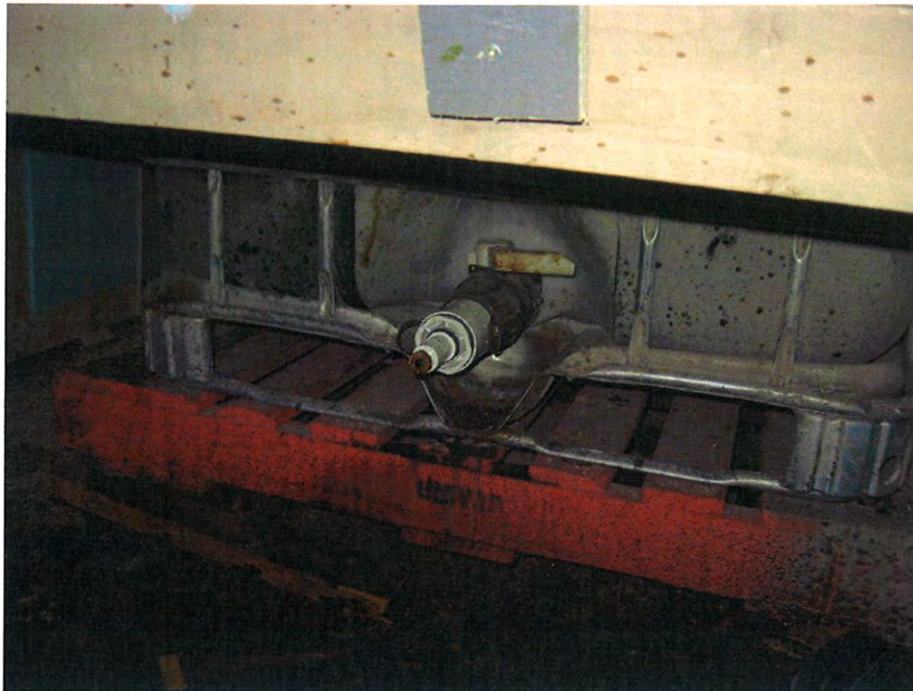
BK625 Corroded Brass Fitting on Ferric Chloride Tank
