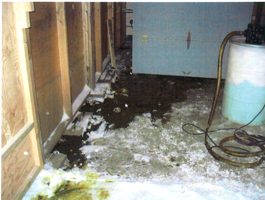
BK625 Ferric Chloride Spillage Inside Reagent Shed
