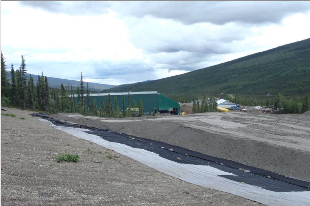
Photo 17: Gravel drainage blanket, geosynthetic clay liner, geonet, geotextile, and tailings placed within the DSTF (Facing south – July 28, 2011)
