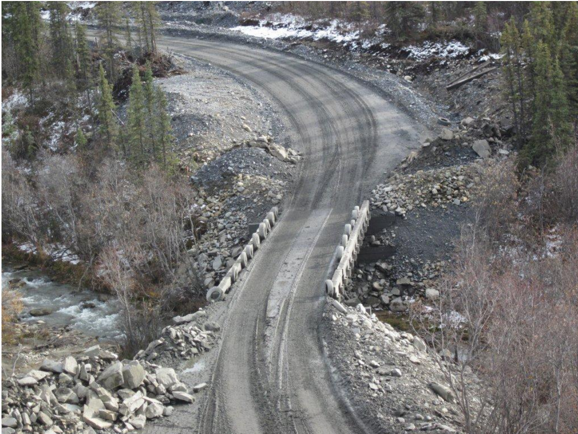
Figure 3-33 Lightning Creek Bridge
