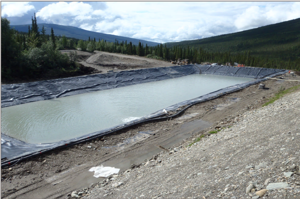
Photo 14: Mill water storage pond and berms appeared stable (Facing west – July 28, 2011)
