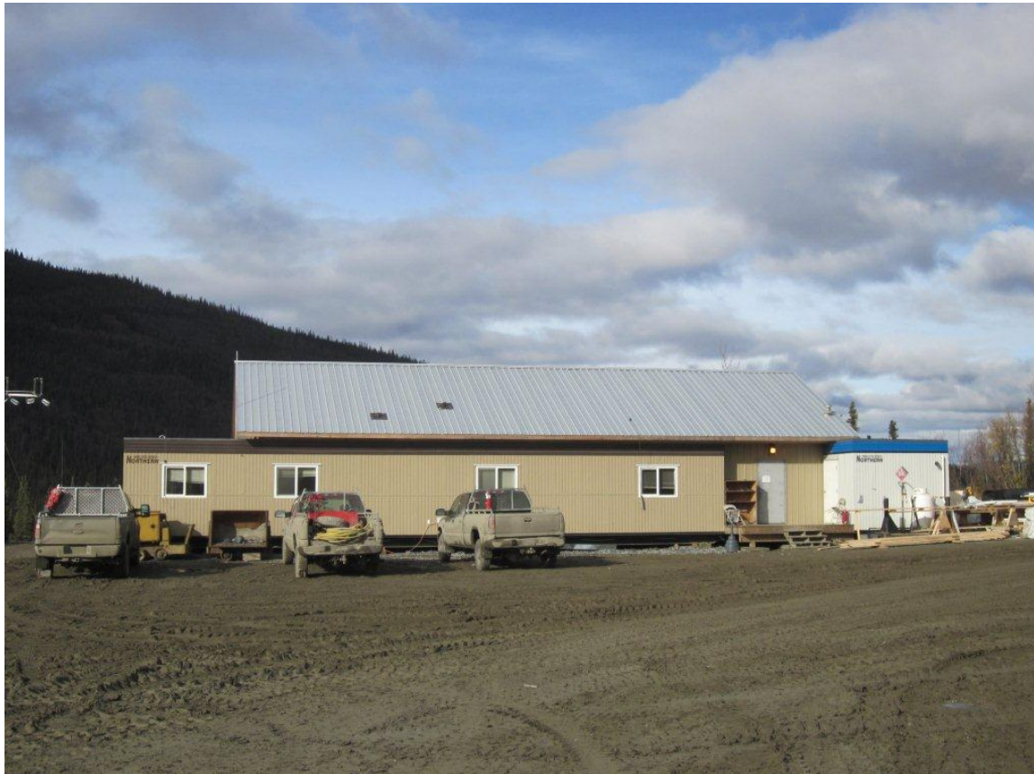
Figure 3-6 Mill Office and Dry
