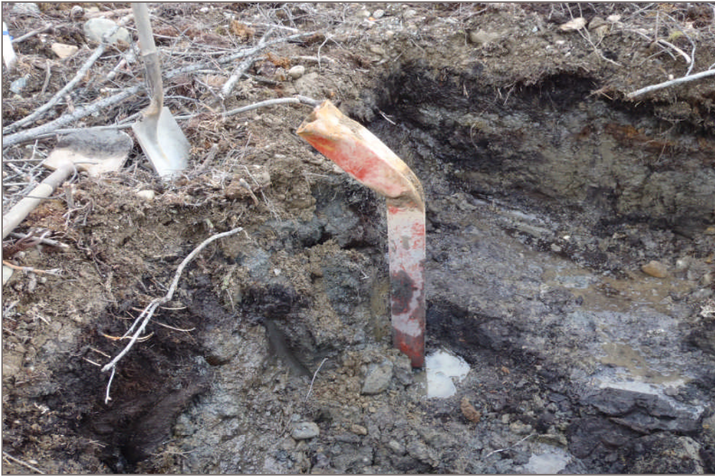
Photo 1: Borehole BH28 – Damaged slope indicator kinked at ground surface. September 28, 2011.
