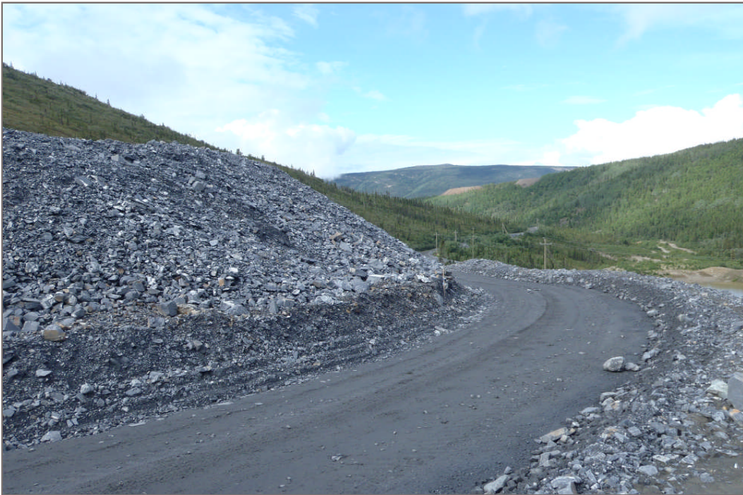
Photo 6: Bellekeno Mine haul road and waste rock pile (Facing west – July 28, 2011)
