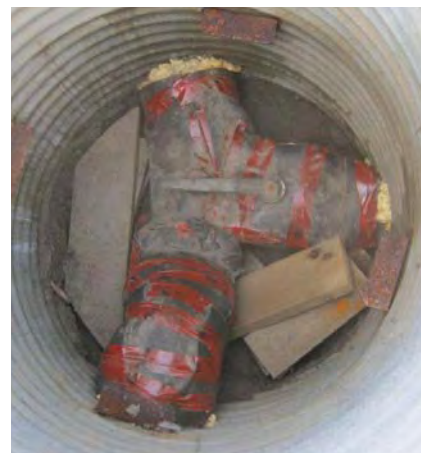
FIGURE 2 – INLET VALVE
