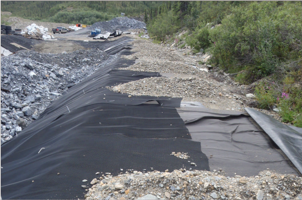
Photo 5: Loose material piled on top of west berm to hold liner in place (Facing south – July 28, 2011)
