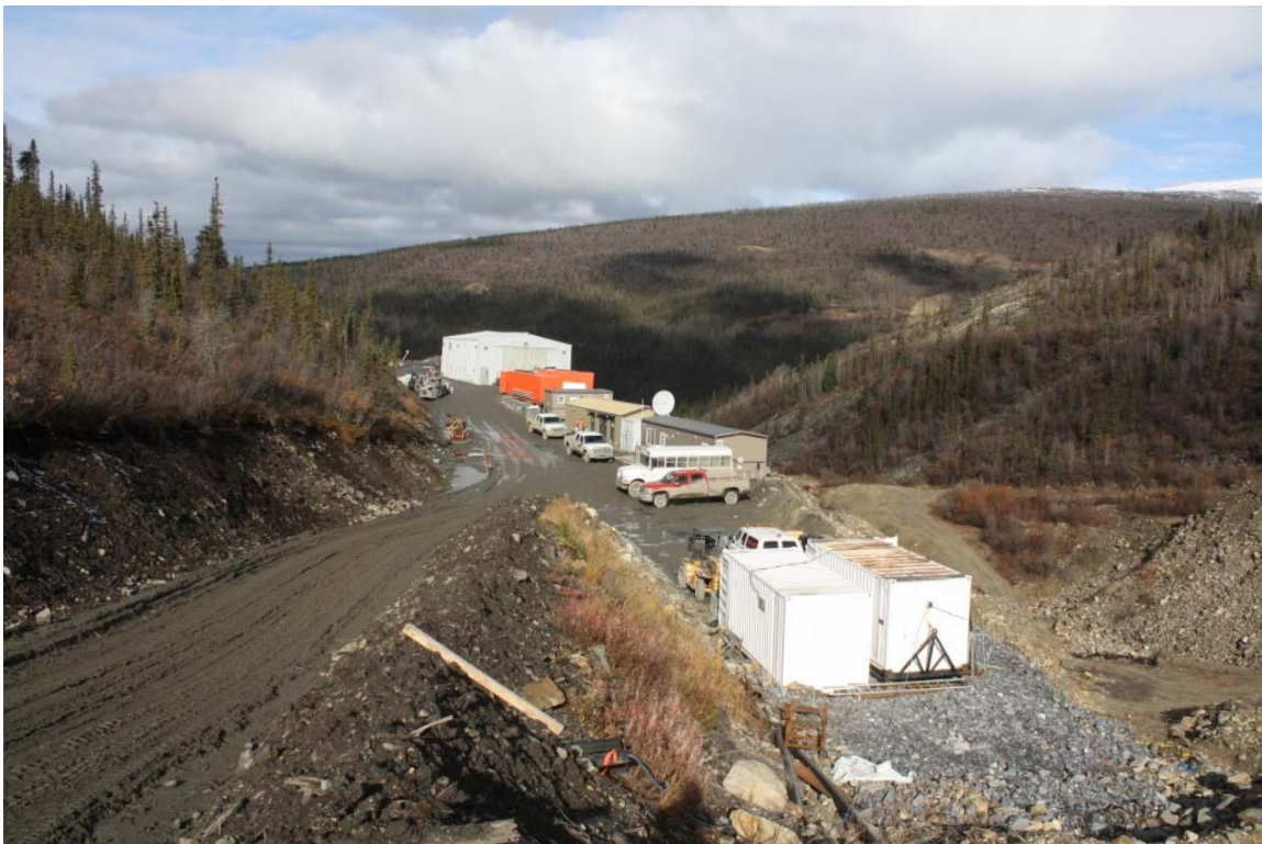
Figure 2-3 Bellekeno East Surface Facilities
