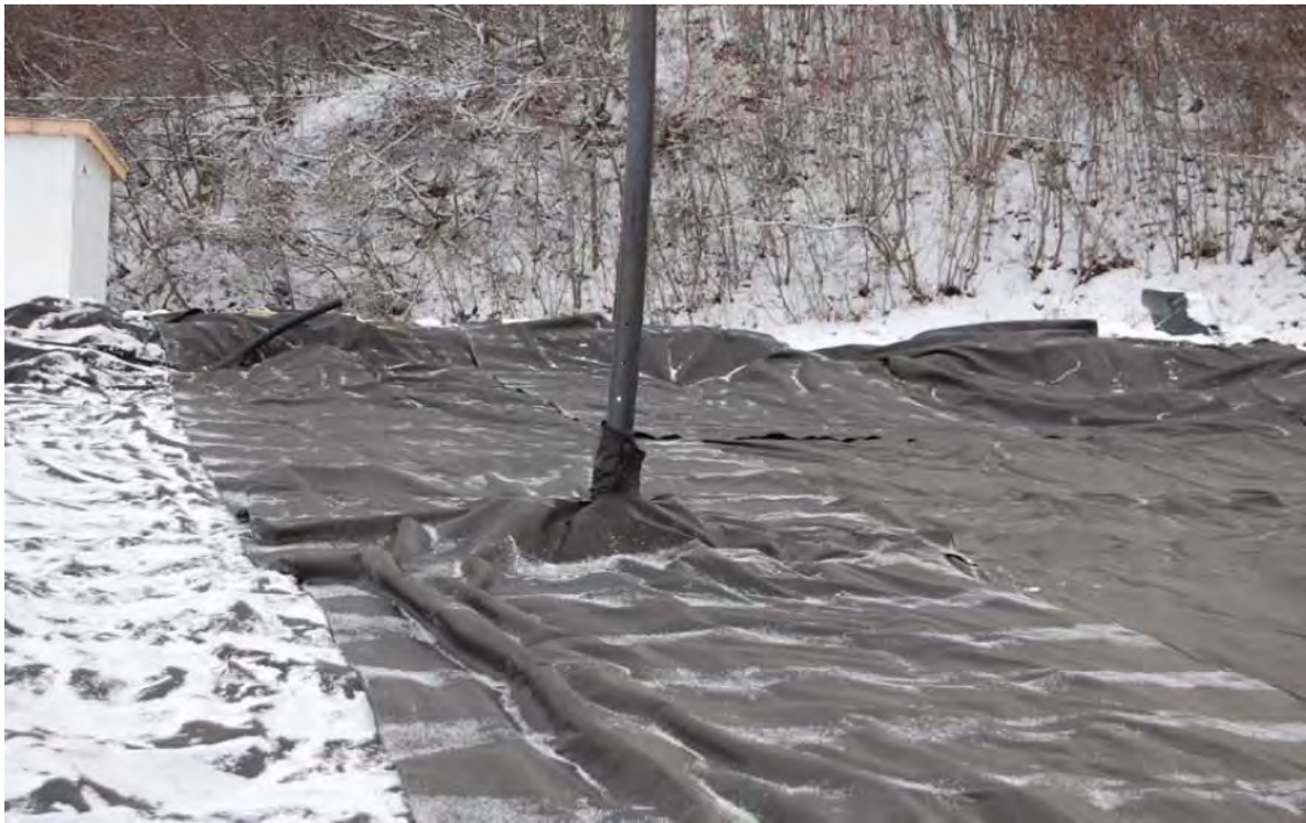
FIGURE 6 – BIOREACTOR STANDPIPE
