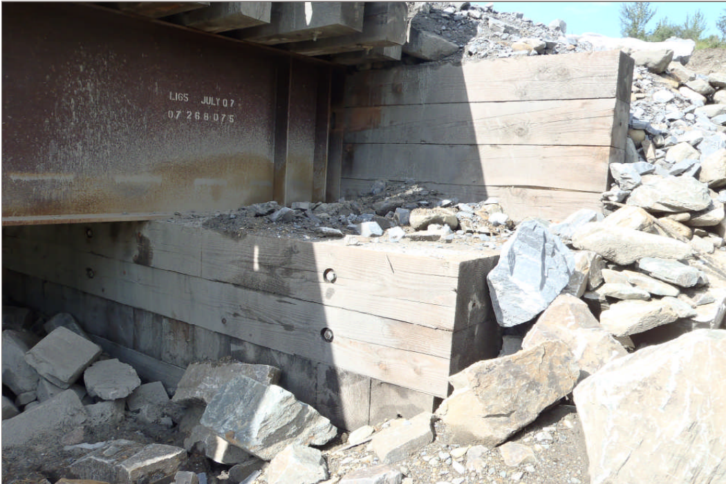
Photo 11: Lightning Creek bridge, north abutment (Facing west – July 28, 2011)
