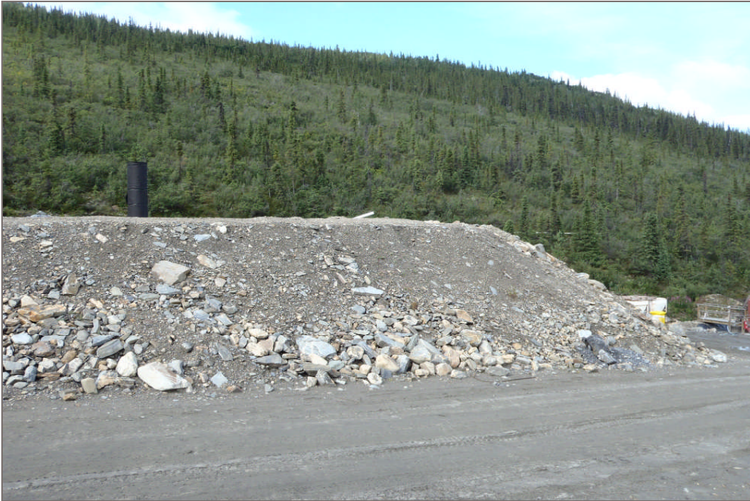
Photo 1: PAG Waste Storage Facility perimeter berm (Facing northwest – July 28, 2011)
