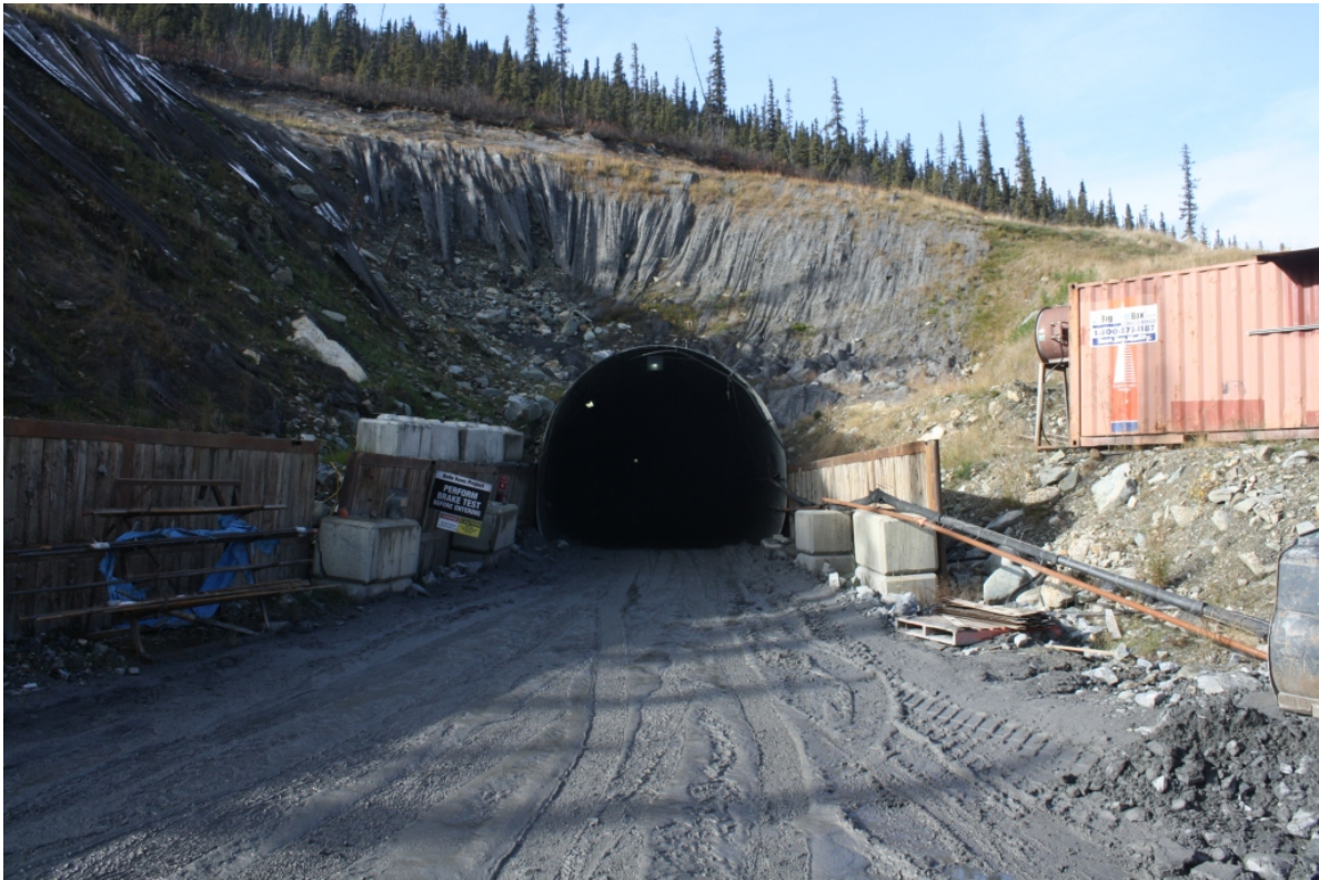
Figure 2-1. Bellekeno East Portal
