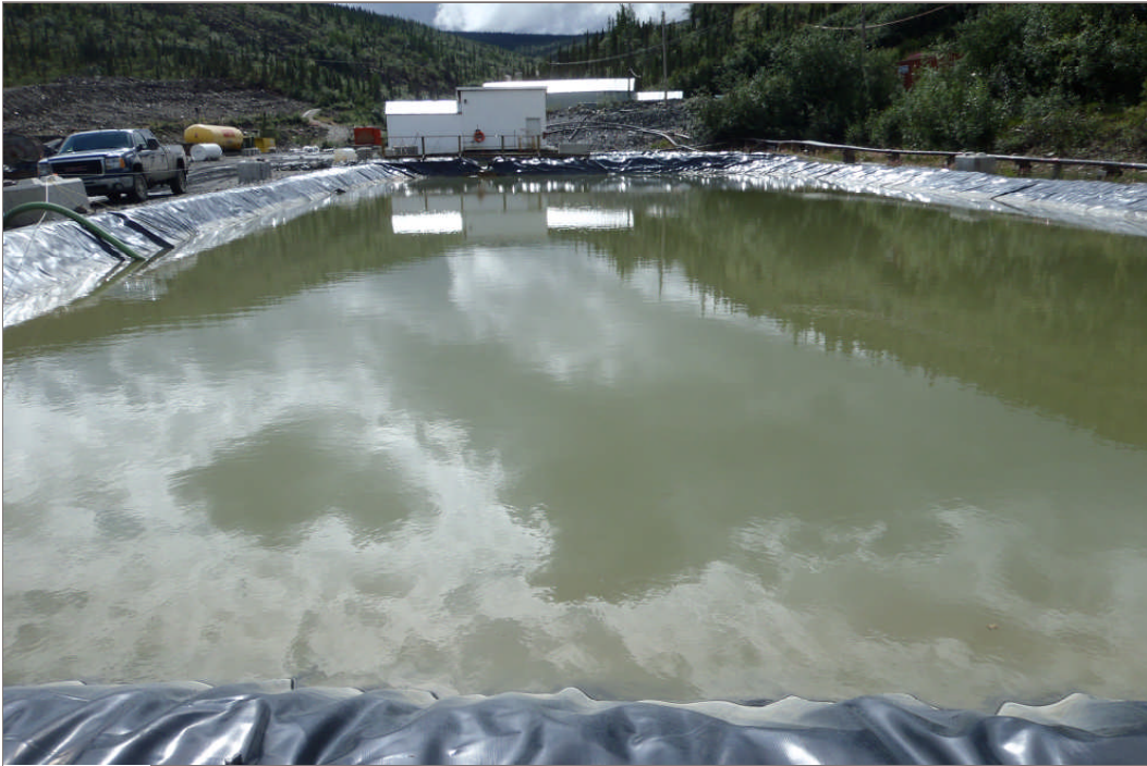
Photo 9: Bellekeno 625 water treatment pond liner system (Facing south – July 28, 2011)
