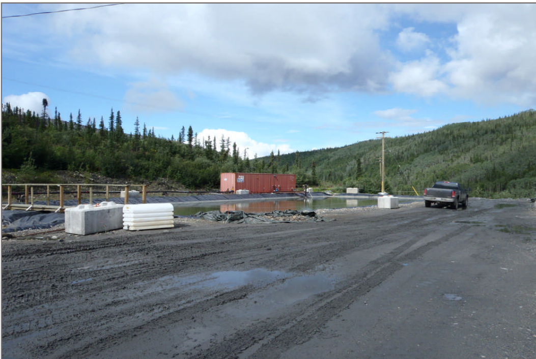
Photo 8: Bellekeno 625 water treatment pond and surrounding structures (Facing north – July 28, 2011)
