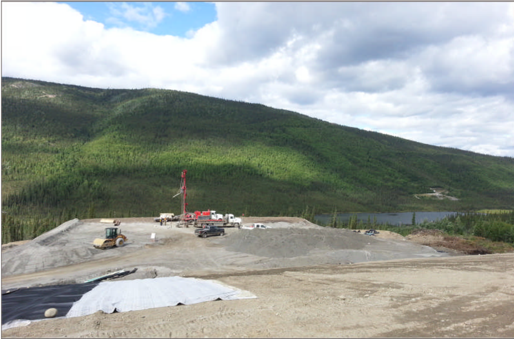
Photo 1: DSTF Lower Bench - Instrumentation Location Facing West August 2, 2012
