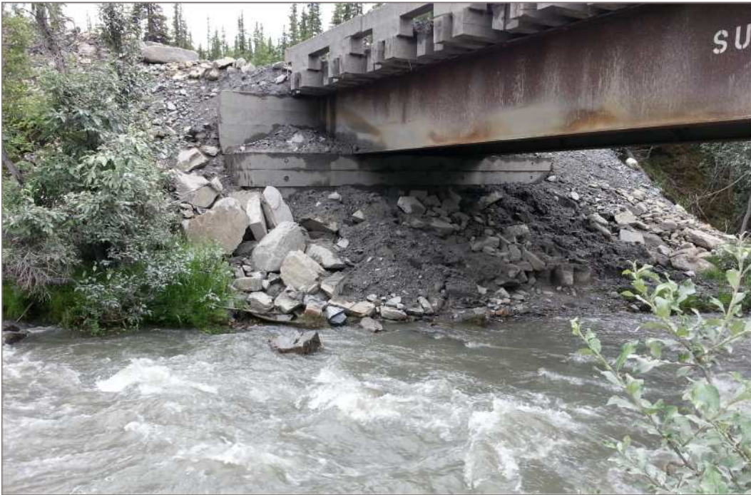
Photo 10: Lightning Creek Bridge Abutments Facing East July 13, 2012
