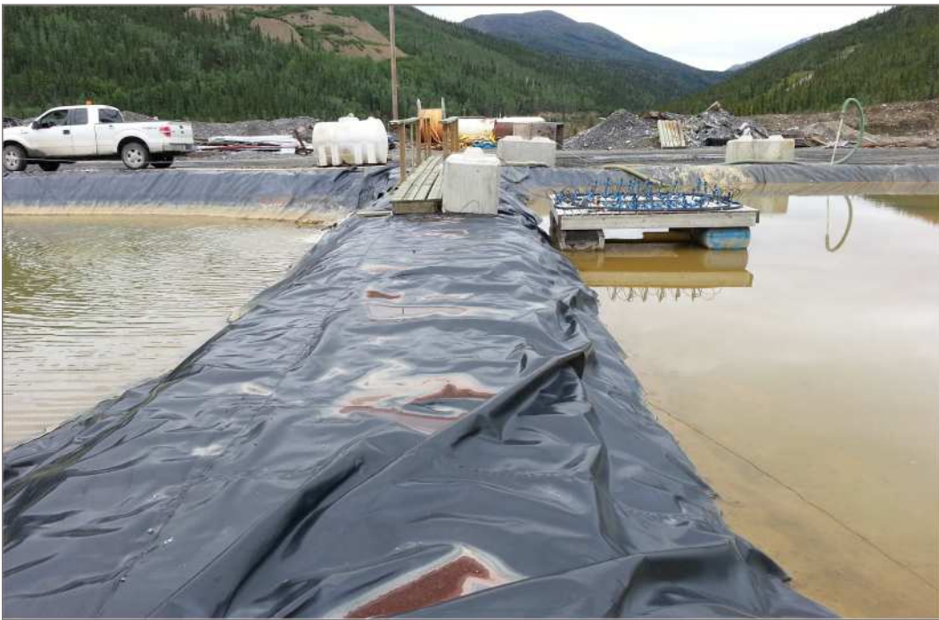
Photo 6: Belkeno 625 Water Treatment Pond July 13, 2012
