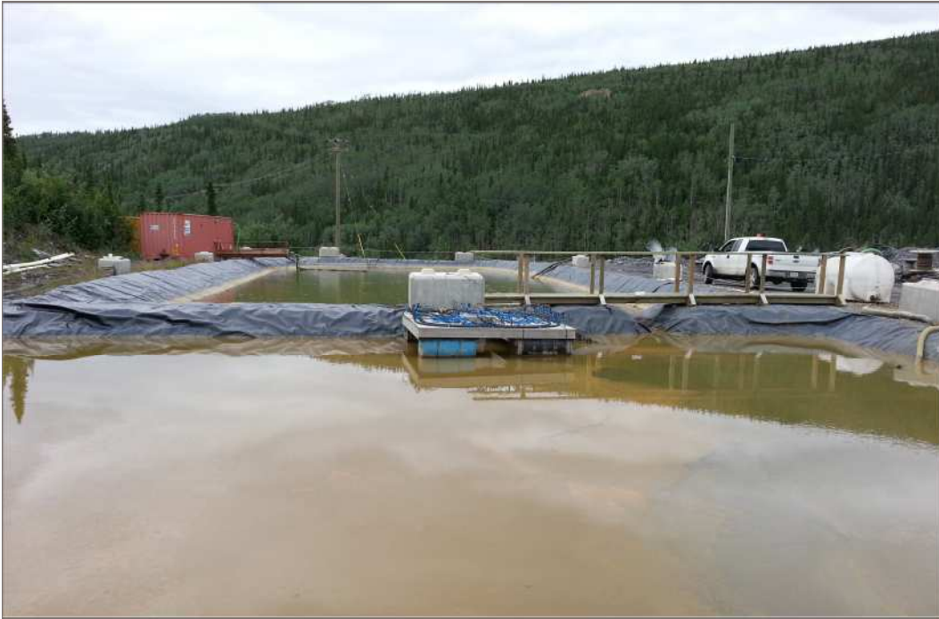
Photo 5: Belkeno 625 Water Treatment Pond July 13, 2012
