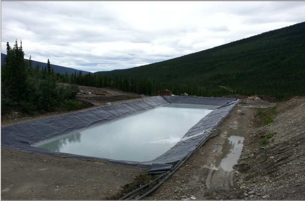
Photo 13: Mill Water Storage Pond July 13, 2012
