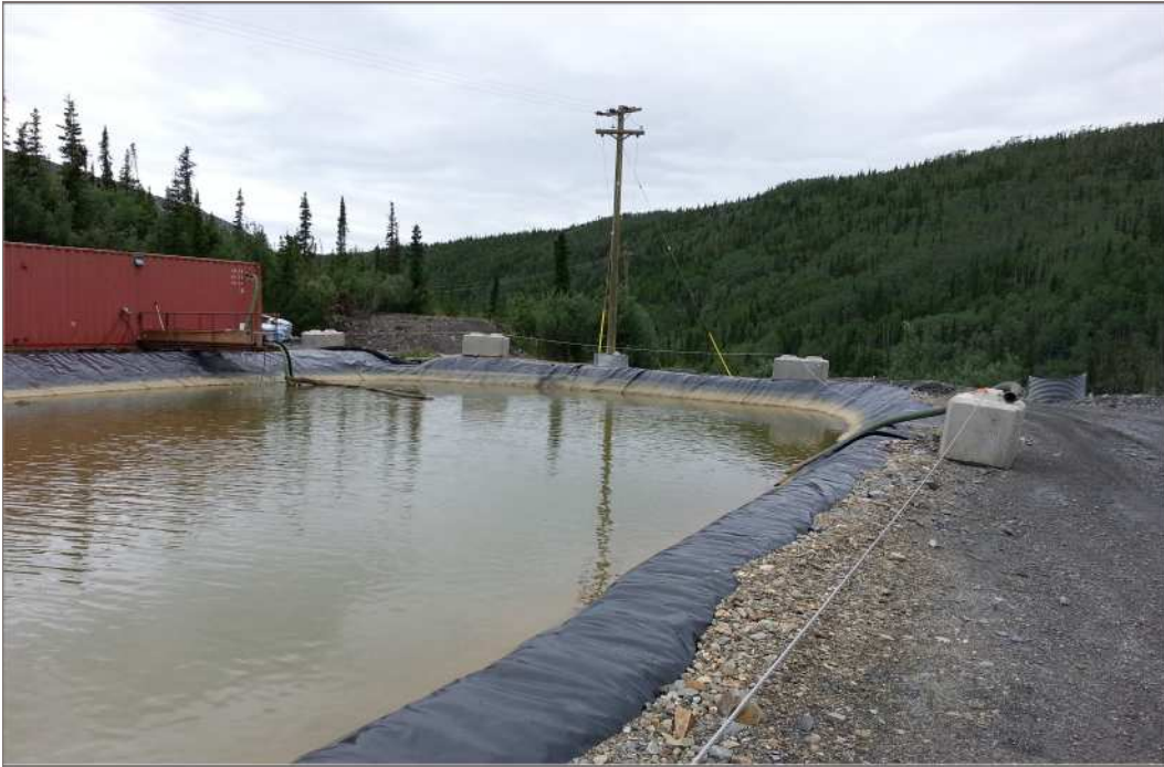
Photo 7: Belkeno 625 Water Treatment Pond July 13, 2012
