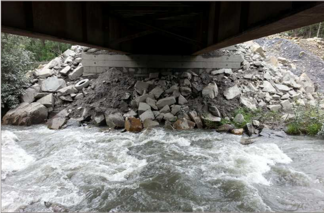
Photo 11: Lightning Creek Bridge Abutments Facing West July 13, 2012
