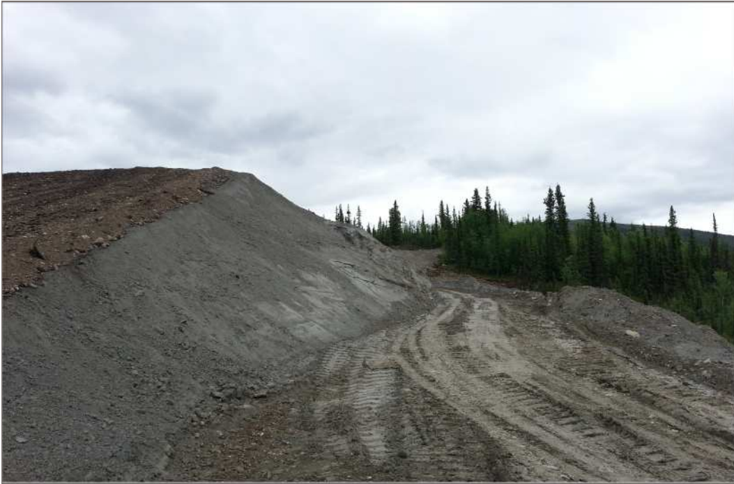
Photo 19: DSTF Lower Bench South slope and haul road July 13, 2012
