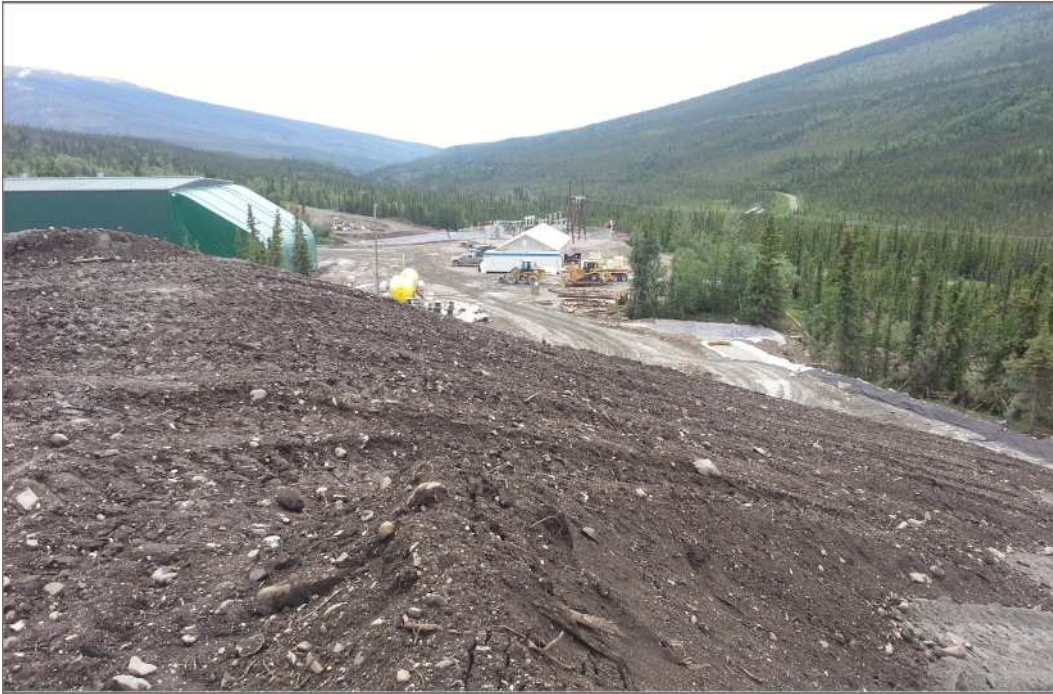
Photo 17: DSTF Lower Bench Early stages of cover placement July 13, 2012
