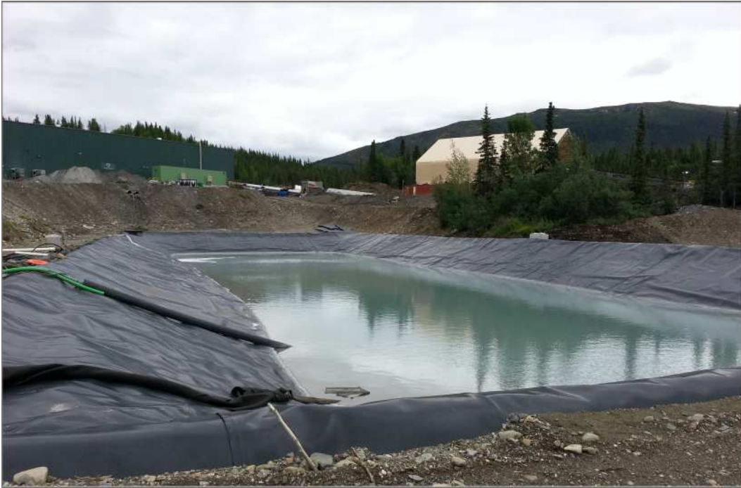
Photo 15: Mill Water Storage Pond July 13, 2012
